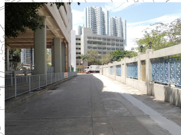
PHOTO 2143: ACCESS ROAD (DATE TAKEN: 12 MAY 2021)
