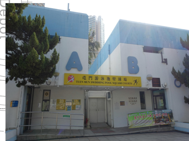
PHOTO 4728: TUEN MUN SWIMMING POOL SQUASH COURTS (DATE TAKEN: 25 JANUARY 2021)
