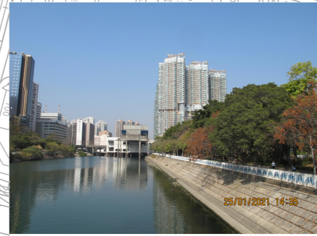
PHOTO 0991: TUEN MUN RIVER CHANNEL (DATE TAKEN: 25 JANUARY 2021)
