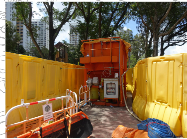
PHOTO 6970: MATERIALS STORAGE AREA AND CHEMICAL DOSING UNIT AT WORKS SITE OF CONTRACT NO. DC/2018/09 (DATE TAKEN: 21 MAY 2021)
