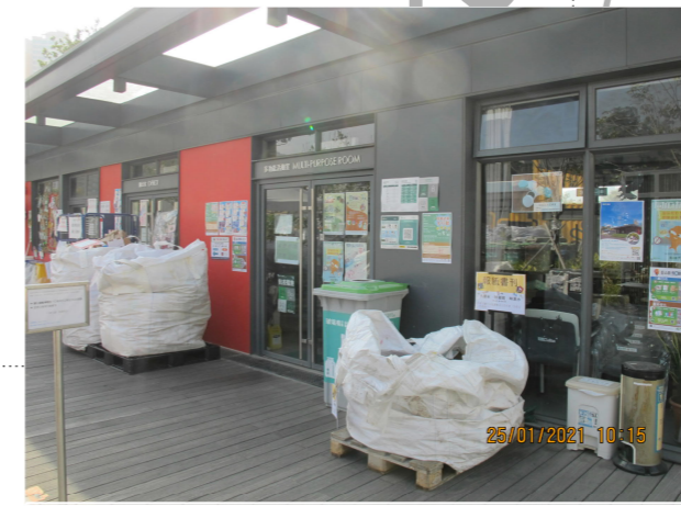
PHOTO 5655: OFFICE AND MULTI-PURPOSE ROOM OF TUEN MUN COMMUNITY GREEN STATION (SITE TME-S1) (DATE TAKEN: 25 JANUARY 2021)
