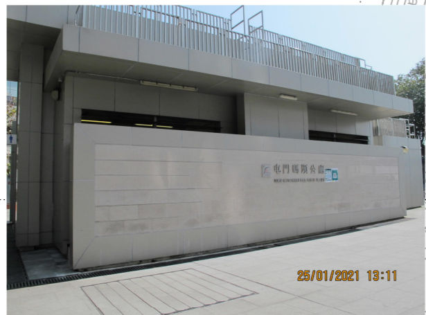
PHOTO 0939: TUEN MUN FERRY PIER PUBLIC TOILET (DATE TAKEN: 25 JANUARY 2021)
