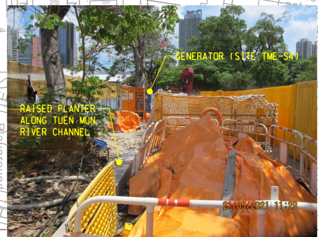
PHOTO 7456: WORKS AREA OF CONTRACT NO. DC/2018/09 (DATE TAKEN: 21 MAY 2021)
