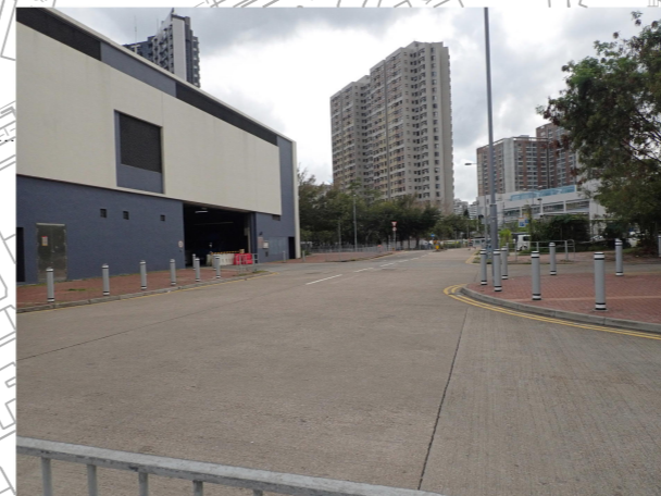
PHOTO 2520: ACCESS ROAD (DATE TAKEN: 17 MAY 2021)
