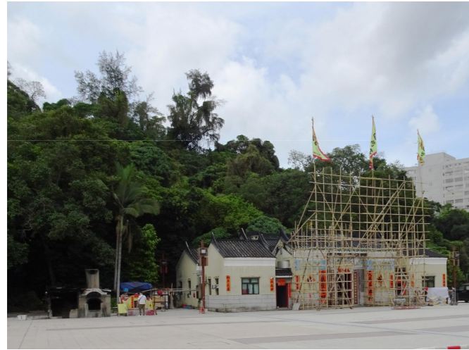
LR 2 - LANDSCAPE AREA IN TIN HAU TEMPLE AND ADJACENT HILLSIDE
