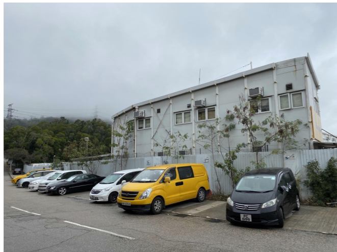
LR 6.6 - VEGETATION ALONG THE EDGES OF THE CONSTRUCTION WORKS AREA
