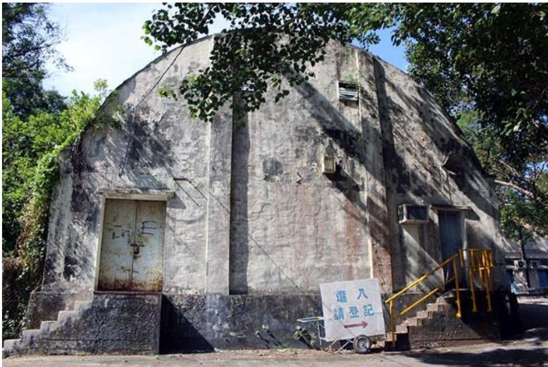
Rear elevation of Kesarbahadur Halls
