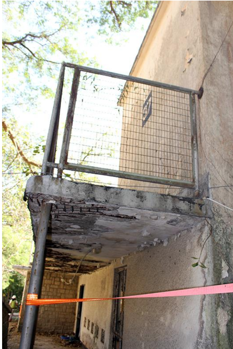
The northern wall of Kesarbahadur Hall
