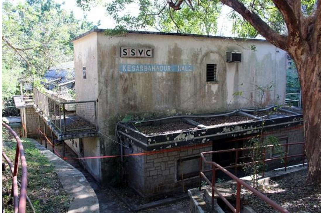
General view of Kesarbahadur Hall
