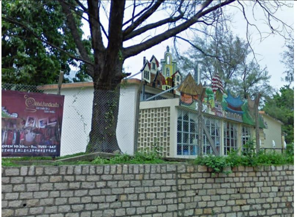
General view of building from Castle Peak Road looking generally north; note protruding addition to the south.
