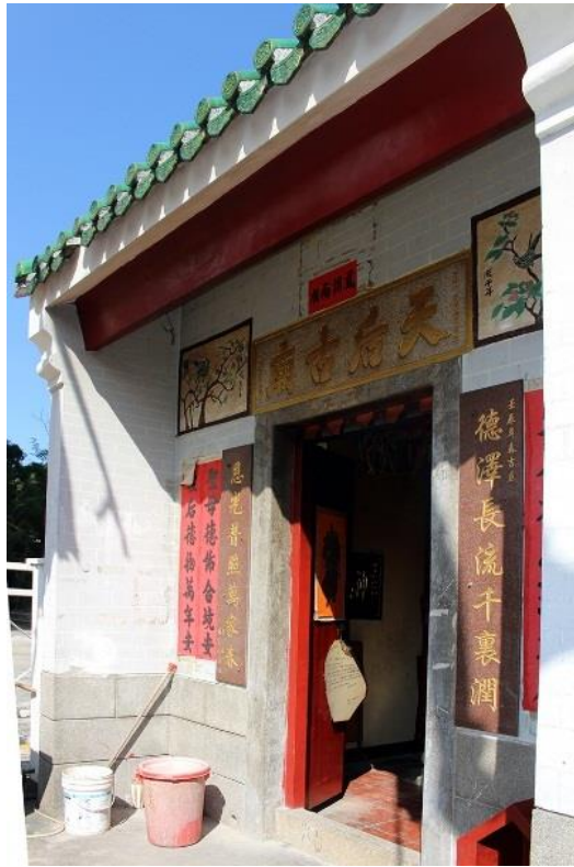
Front façade of Tin Hau Temple
