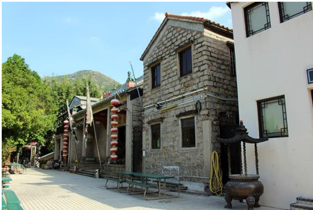
Additional buildings to both sides of Shing Miu. Left: office block; Right: Tai Sui Din
