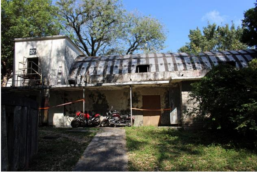
The southern wall of Kesarbahadur Hall
