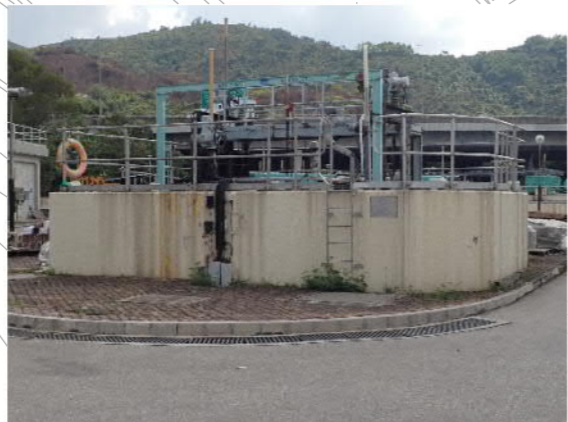
PHOTO 2185: DISUSED INLET CHAMBER (DATE TAKEN: 14 MAY 2021)
