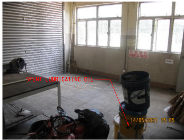
PHOTO 7307: FORMER WORKSHOP IN ADMINISTRATION BUILDING (DATE TAKEN: 14 MAY 2021)
