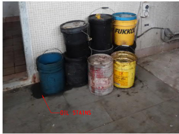
PHOTO 6907: EXISTING CHEMICAL STORAGE AREA IN FORMER SOLIDS HANDLING STATION (DATE TAKEN: 14 MAY 2021)
