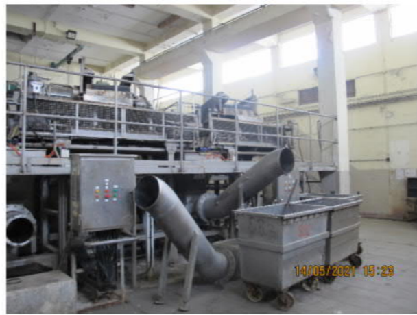
PHOTO 7345: FORMER SOLIDS HANDLING STATION (DATE TAKEN: 14 MAY 2021)
