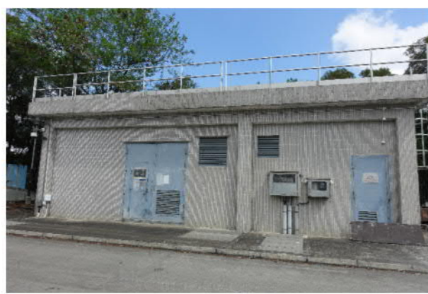
PHOTO 6870: EXISTING TRANSFORMER HOUSE (INACCESSIBLE) (DATE TAKEN: 14 MAY 2021)
