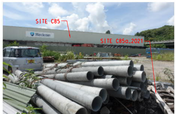
PHOTO 7486: SUSPECTED WAREHOUSE (SITE C85) & SUSPECTED OPEN AREA STORAGE (SITE C85a_2021) (DATE TAKEN: 25 AUGUST 2021)
