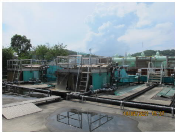
PHOTO 7352: DISUSED FINE SCREEN CHAMBER (DATE TAKEN: 14 MAY 2021)
