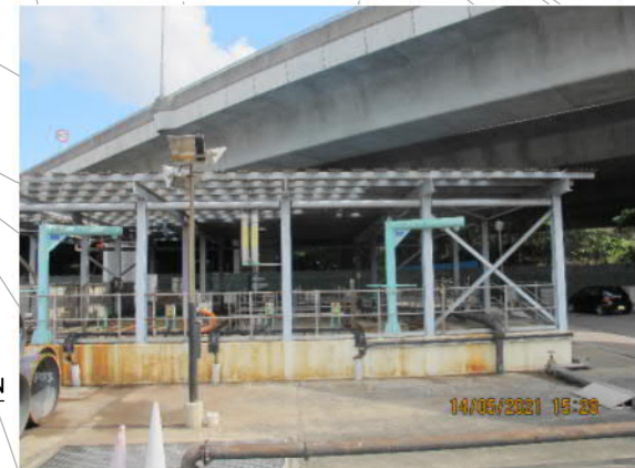
PHOTO 7358: DISUSED WATER STORAGE TANK (DATE TAKEN: 14 MAY 2021)
