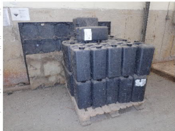
PHOTO 2242: BLEACH STORAGE AREA IN FORMER SOLIDS HANDLING STATION (DATE TAKEN: 14 MAY 2021)
