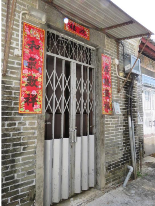
Façade of No.23, looking southwest.
