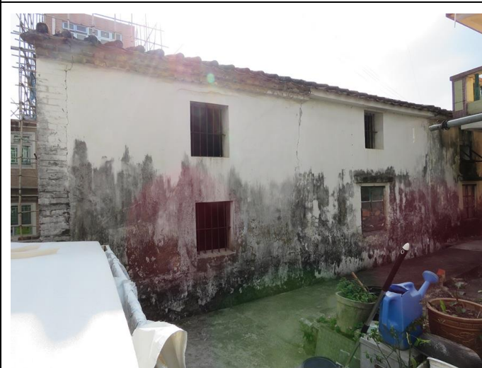
Back view of HB-06, showing northeast elevation, looking west.
