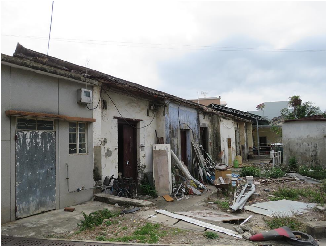
Front view of HB-43, looking southeast.
