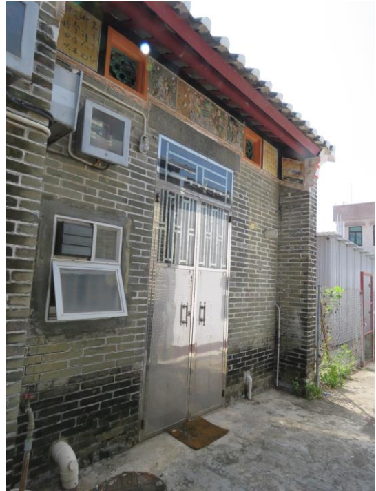
Façade of No.22, looking southwest.
