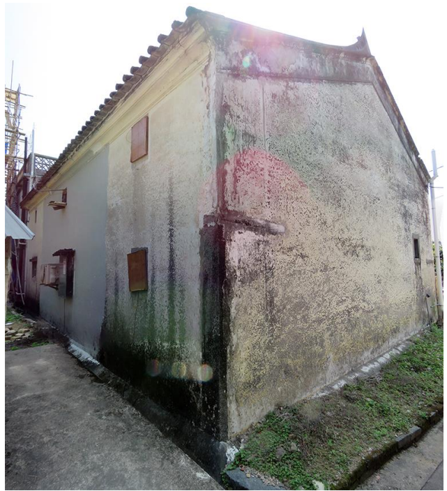
Back and side view, showing northeast and northwest elevations, looking south.
