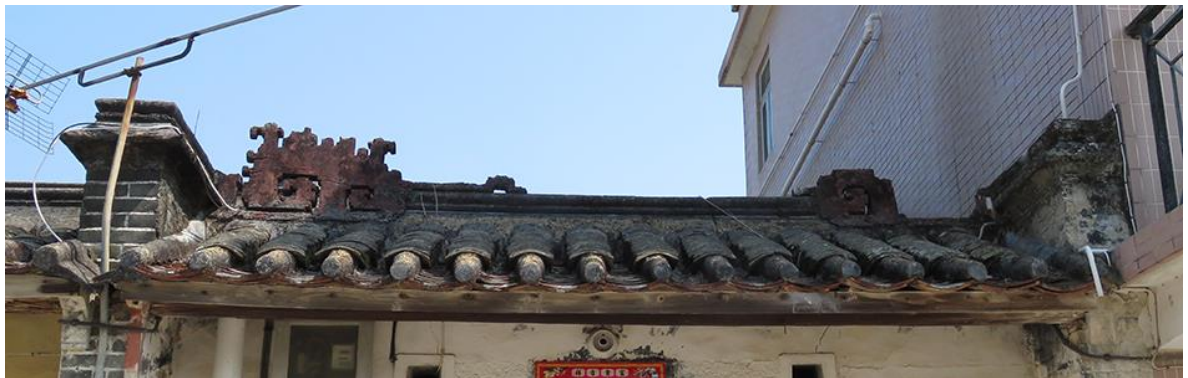
Other details: Roof of No. 2
