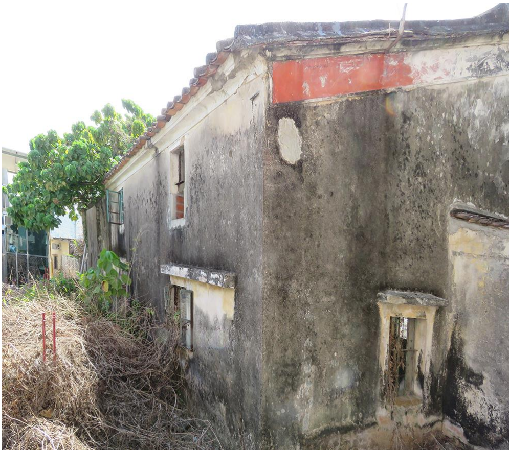
Back view of HB-52, showing northeast elevation, looking south.
