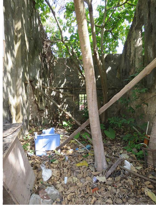
Internal view of ruin No.134, looking northeast.
