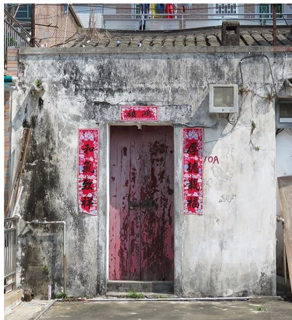
Close up of the façade (No. 10A)
