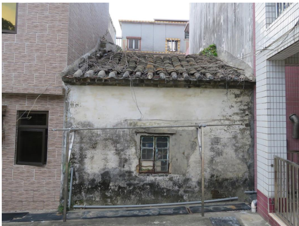
Back view HB-63, showing east elevation, looking west.
