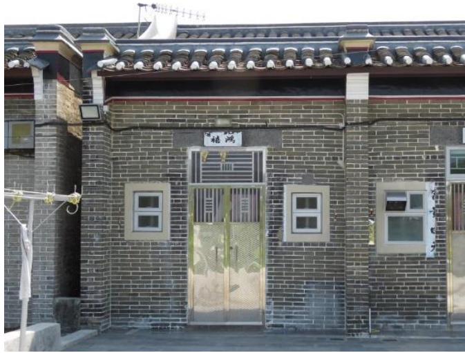
Close up of the façade of No.35 (Middle bay)
