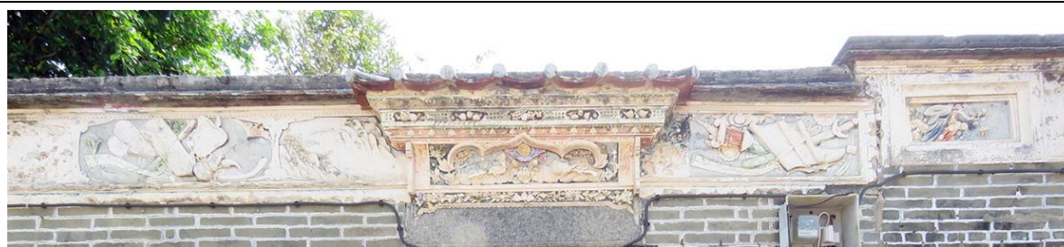
Example of plaster moulding on façade wall
