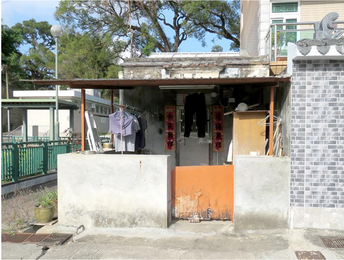
Front view of HB-26, looking northeast.
