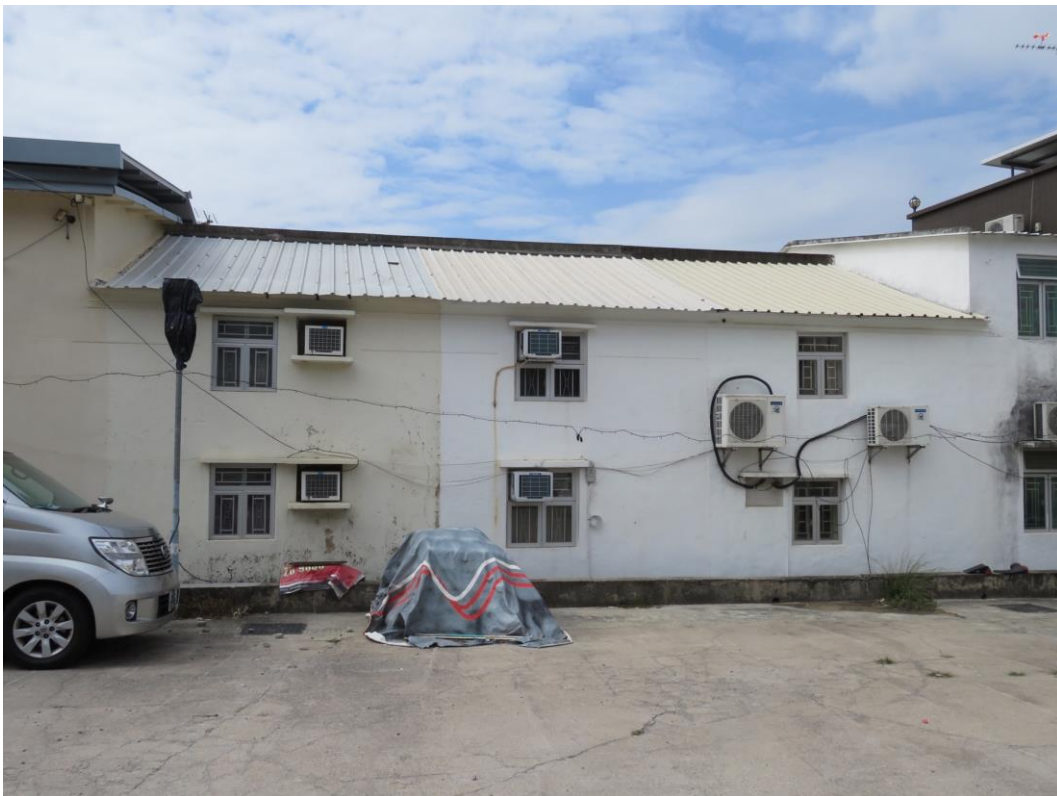
Back view of HB-46, showing northeast elevation, looking southwest.
