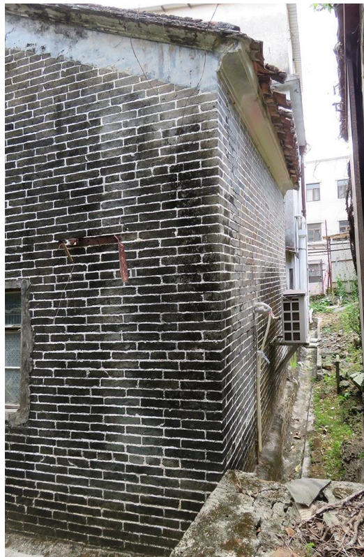
Back view of HB-60, showing northwest elevation, looking southwest.
