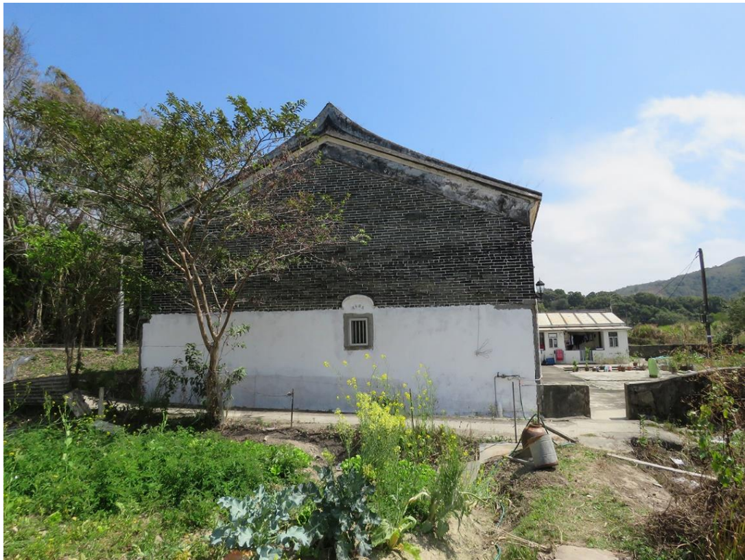
Side view of GB-08, showing northwest elevation, looking southeast.
