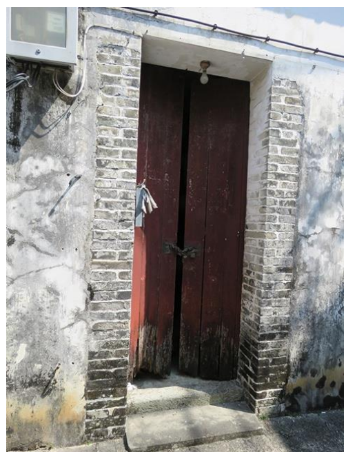
Façade of No.15, looking southeast.
