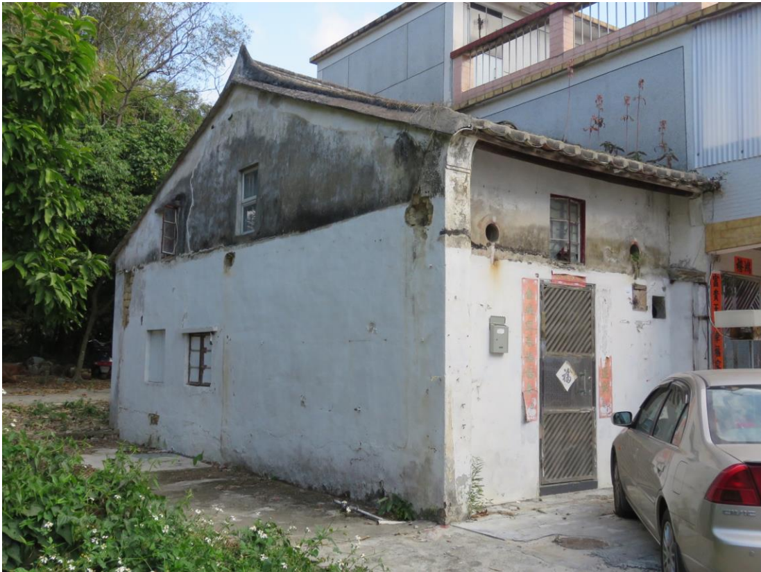
General view of HB-65, showing northwest elevation and façade, looking southeast.
