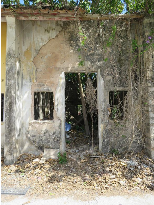
Façade of ruin next to No.134, looking northeast.
