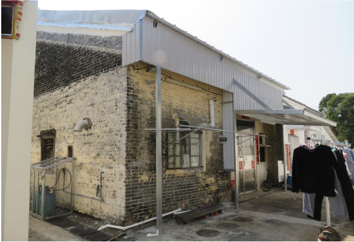
Front view of HB-18, looking southwest.
