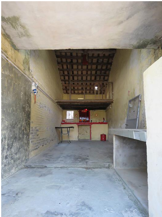
Internal view HB-34, looking south-south-east.
