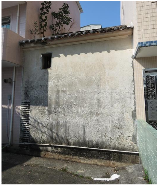
Back view of HB-31, showing south elevation, looking north.
