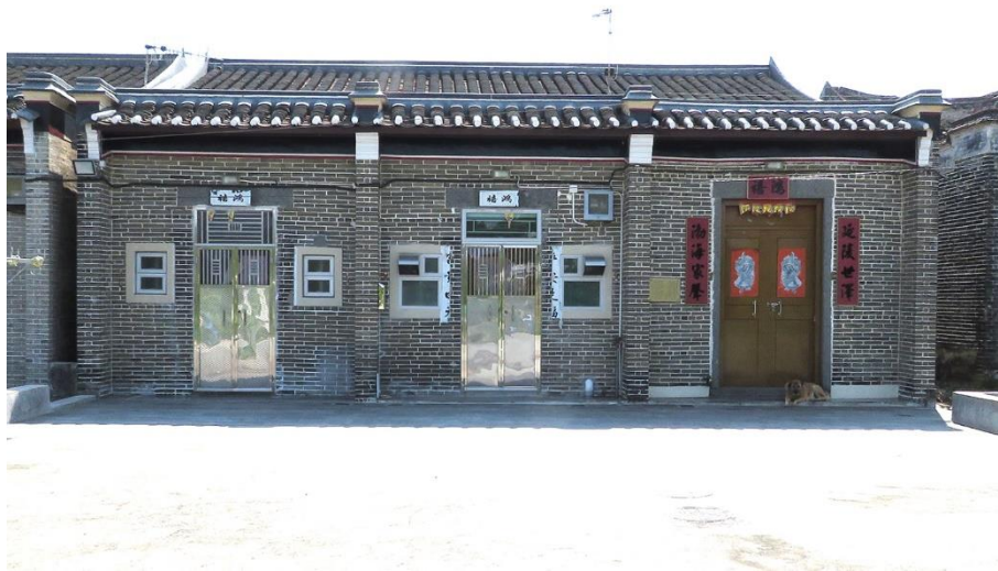
Façade view of No.35, looking southeast.
