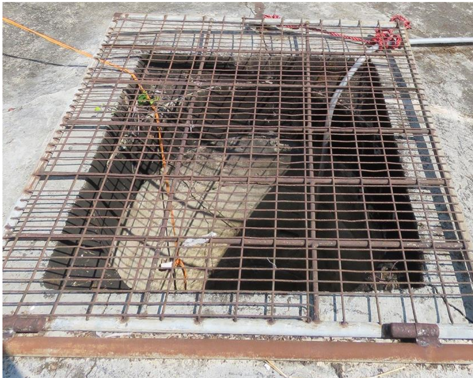
Stone lining of the well, looking northeast.
