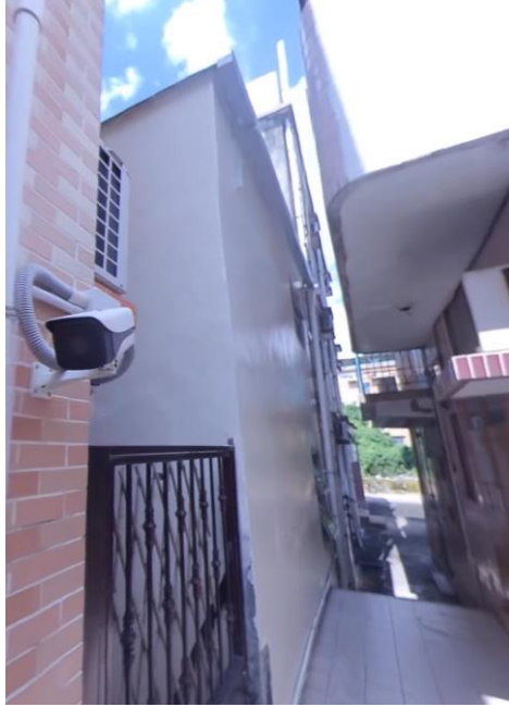
Newly renovated rear of No.8
