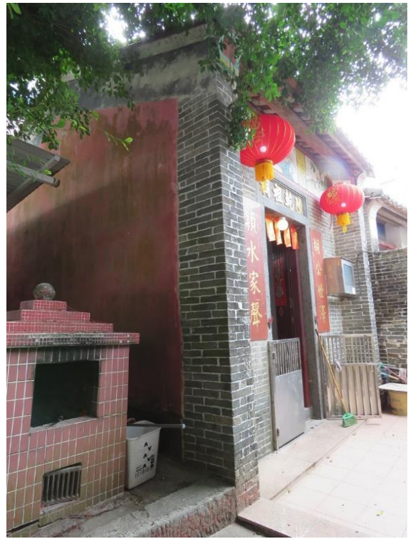
Side view of GB-07, showing north elevation, looking southeast.
