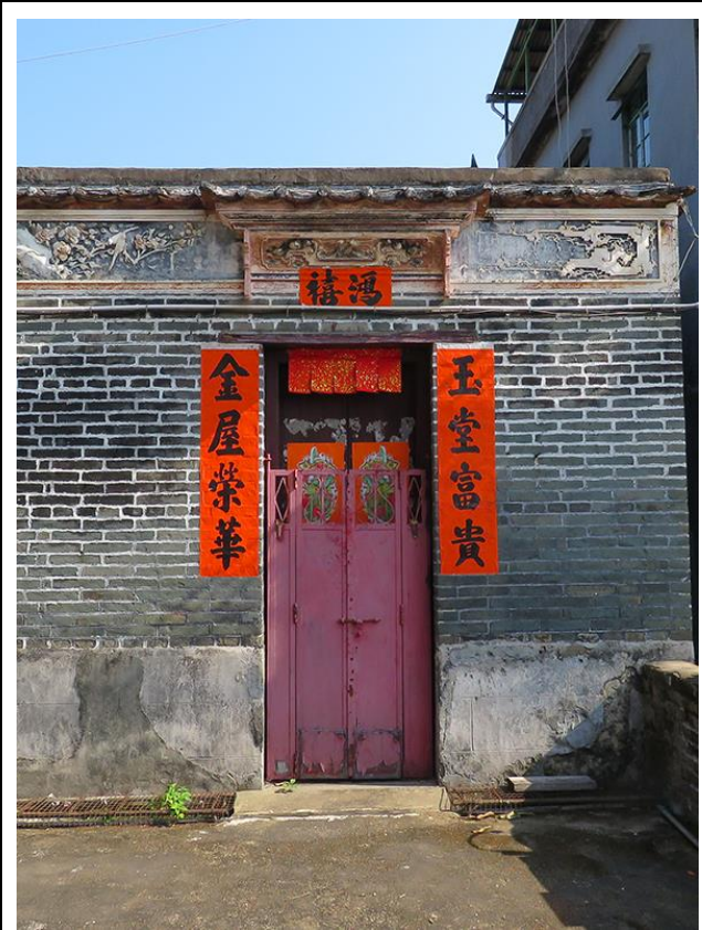
Close up of the façade (No. 41A)
