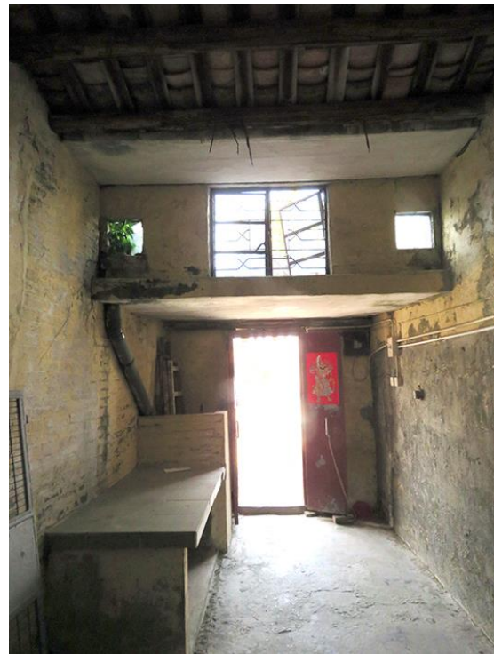
Internal view HB-34, looking north-north-west.
