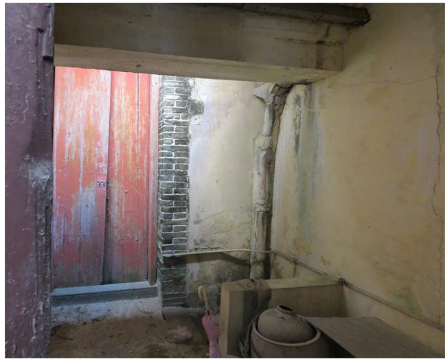
Internal view of HB-31, looking south.
