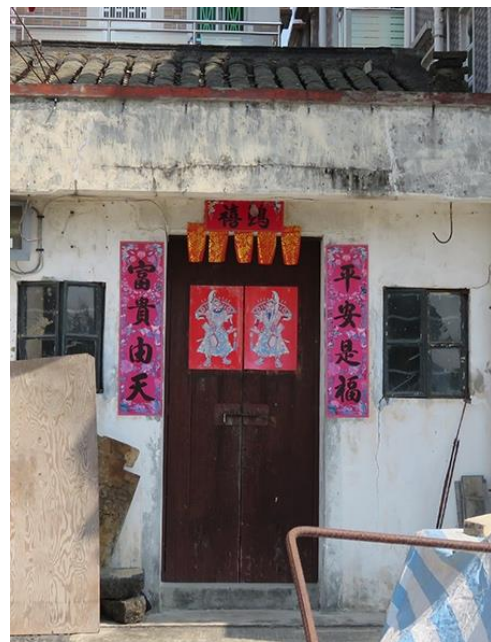
Close up of the façade (No.10)
