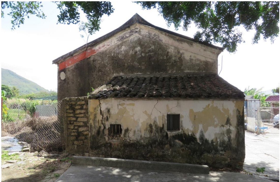
Side view of HB-52, showing northwest elevation, looking southeast.
