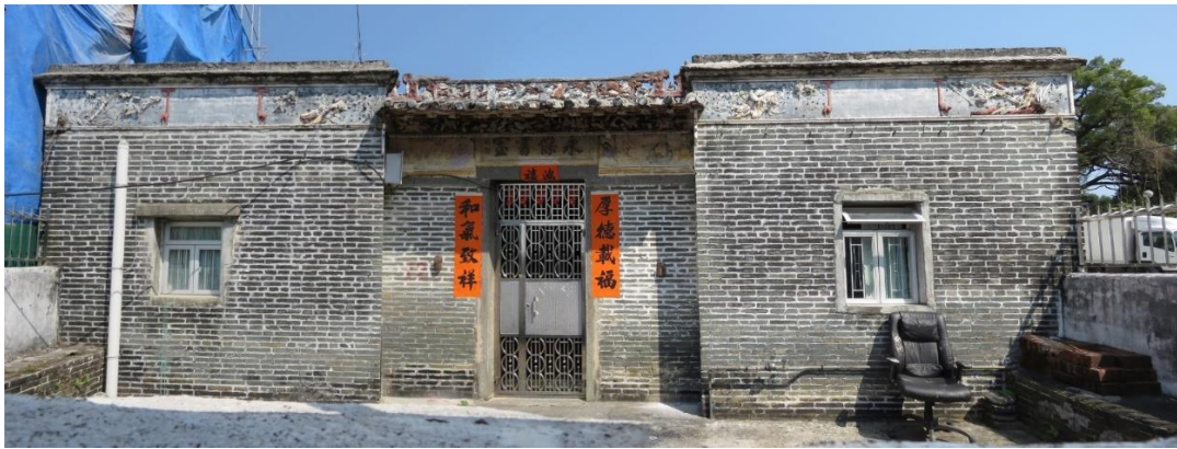
Façade view, looking northeast.
