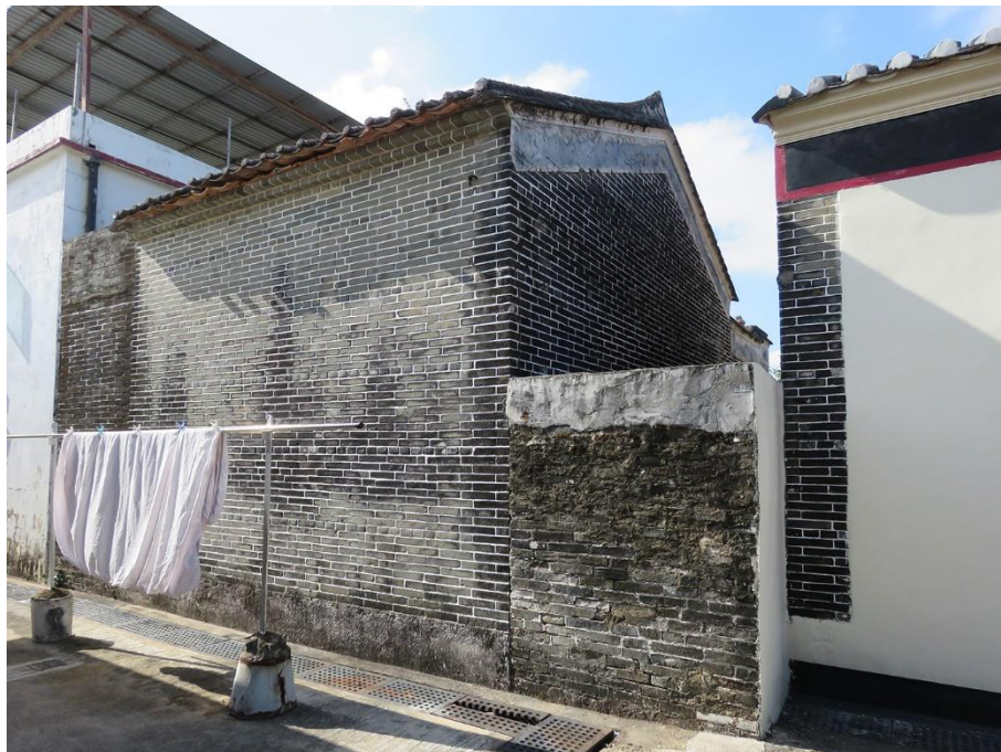
Back View, showing the southeast elevation, looking northwest.
