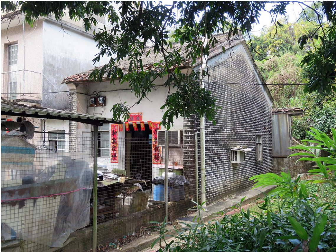
General view of HB-60, showing façade and northeast elevation, looking northwest.
