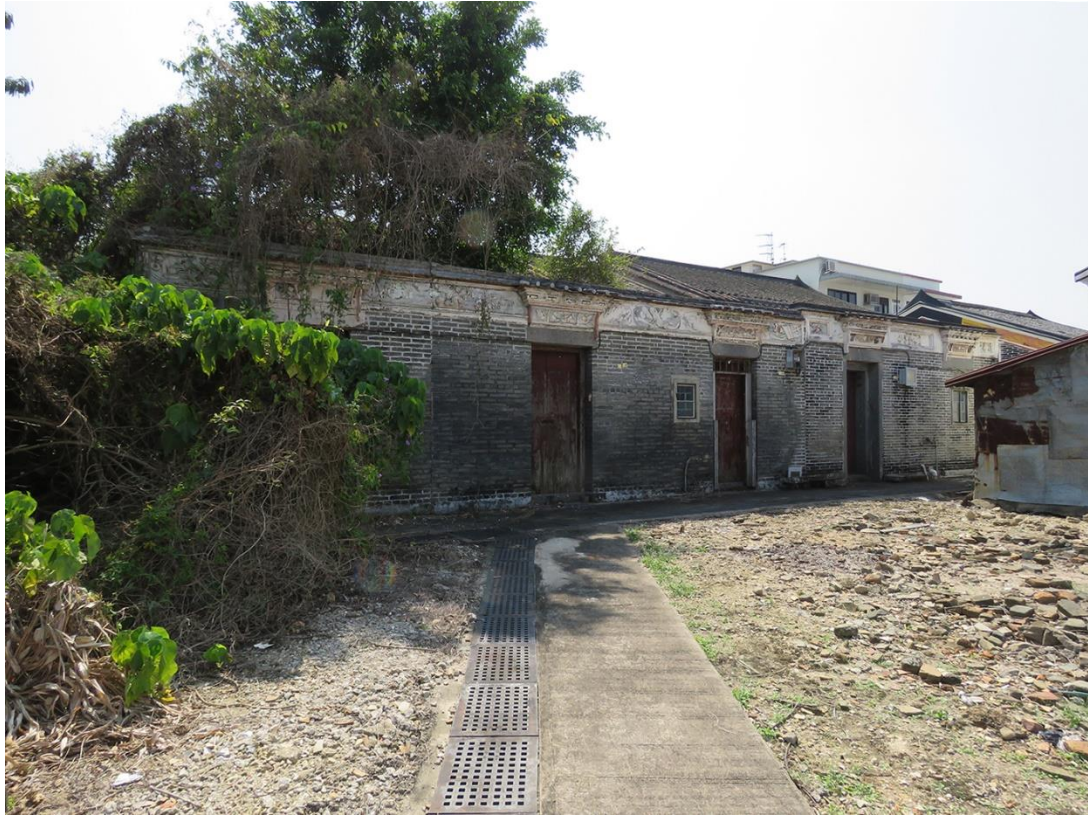
General view of GB-05, looking southwest.
