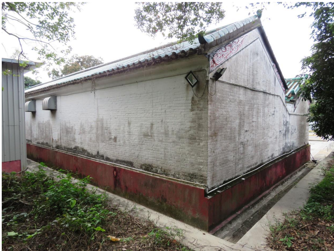
Rear view of GB-09, looking northwest
