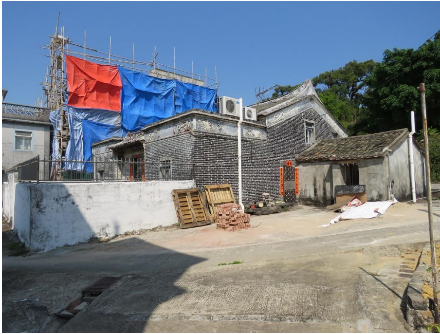
Side view of GB-01, showing façade and southeast elevation, looking northeast.
