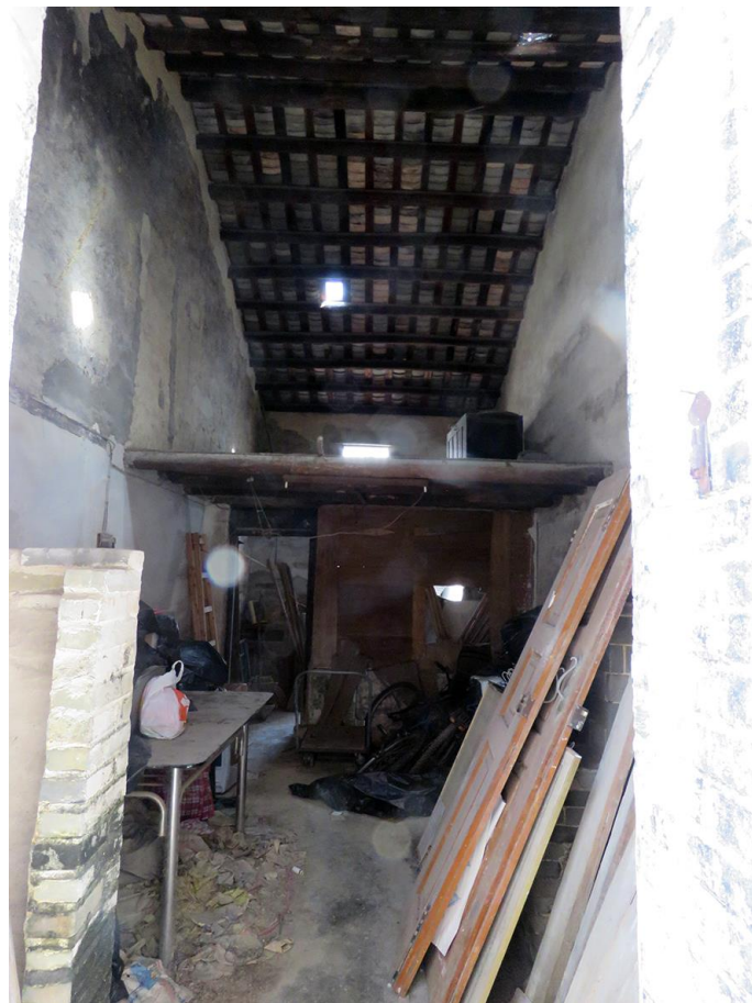
Internal view of No.17, looking northeast.
