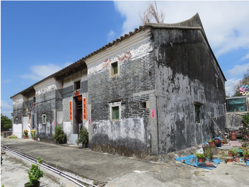
Side view of GB-08, showing southeast elevation, looking northwest.
