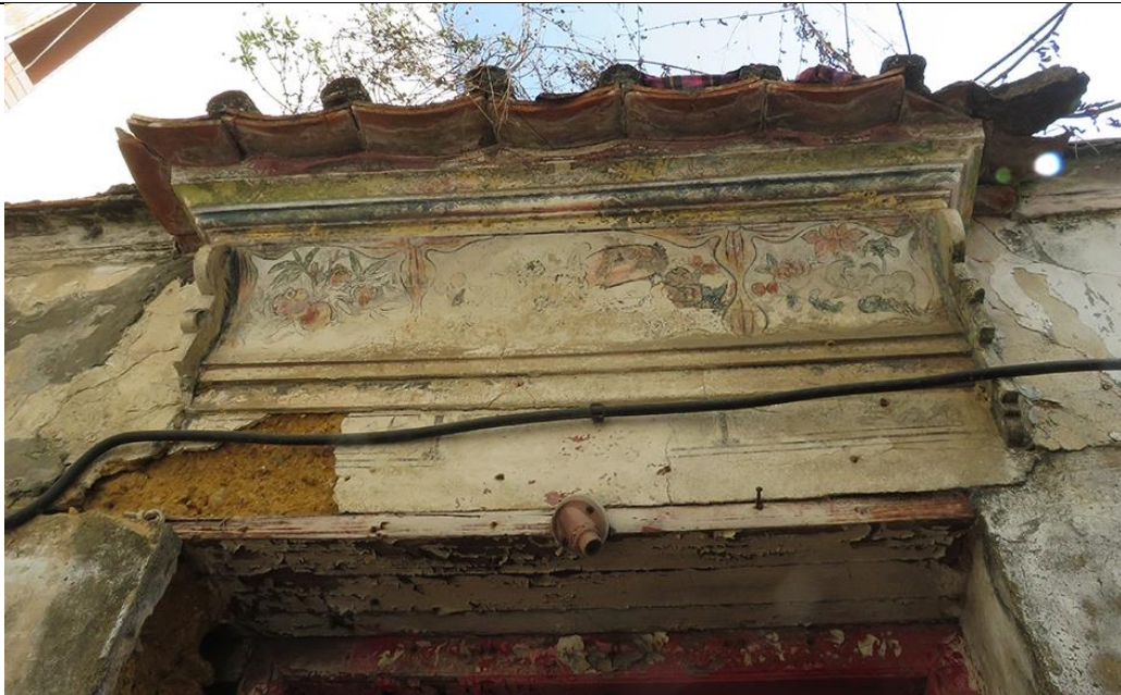
Painting on door canopy of No.12B
