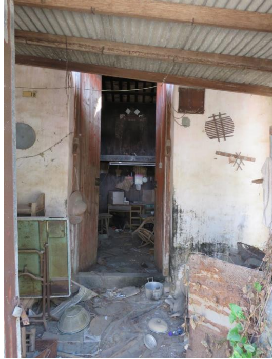
Façade of No.18, looking southeast.
