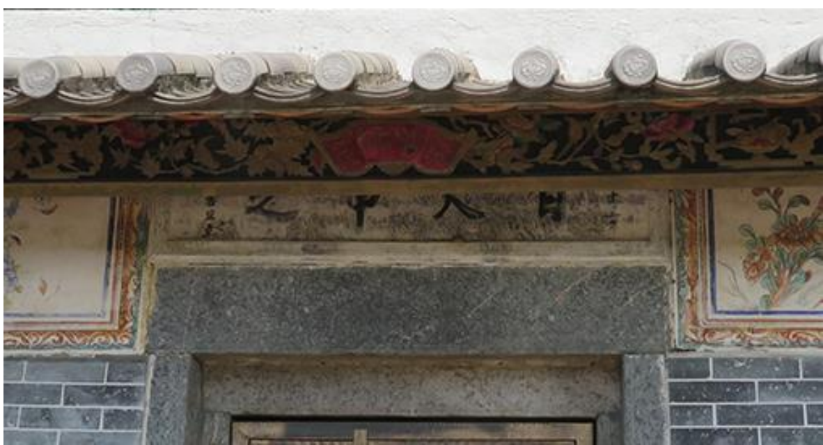
Close up of the façade (No.23)
