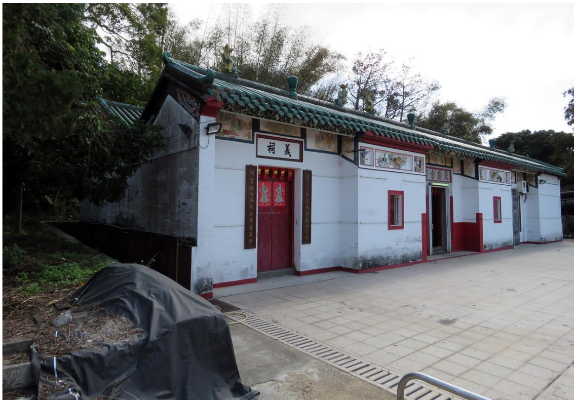
Side view of GB-09, showing façade and northeast elevation, looking southwest.
