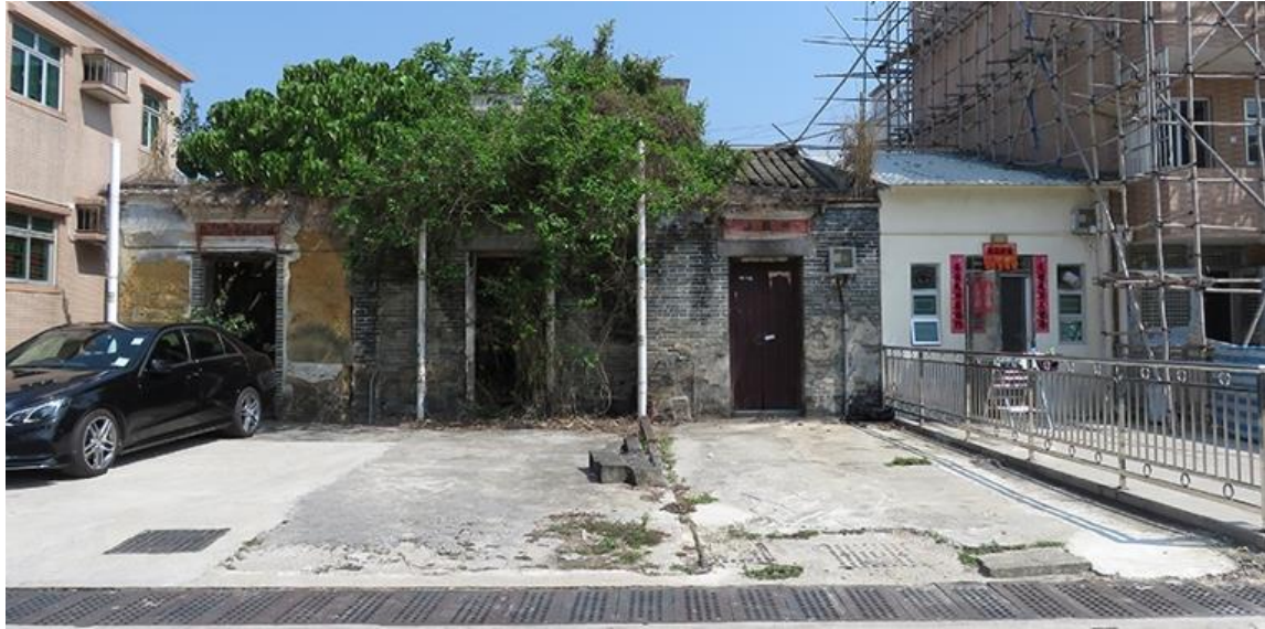
Front view of HB-03, looking northeast.
