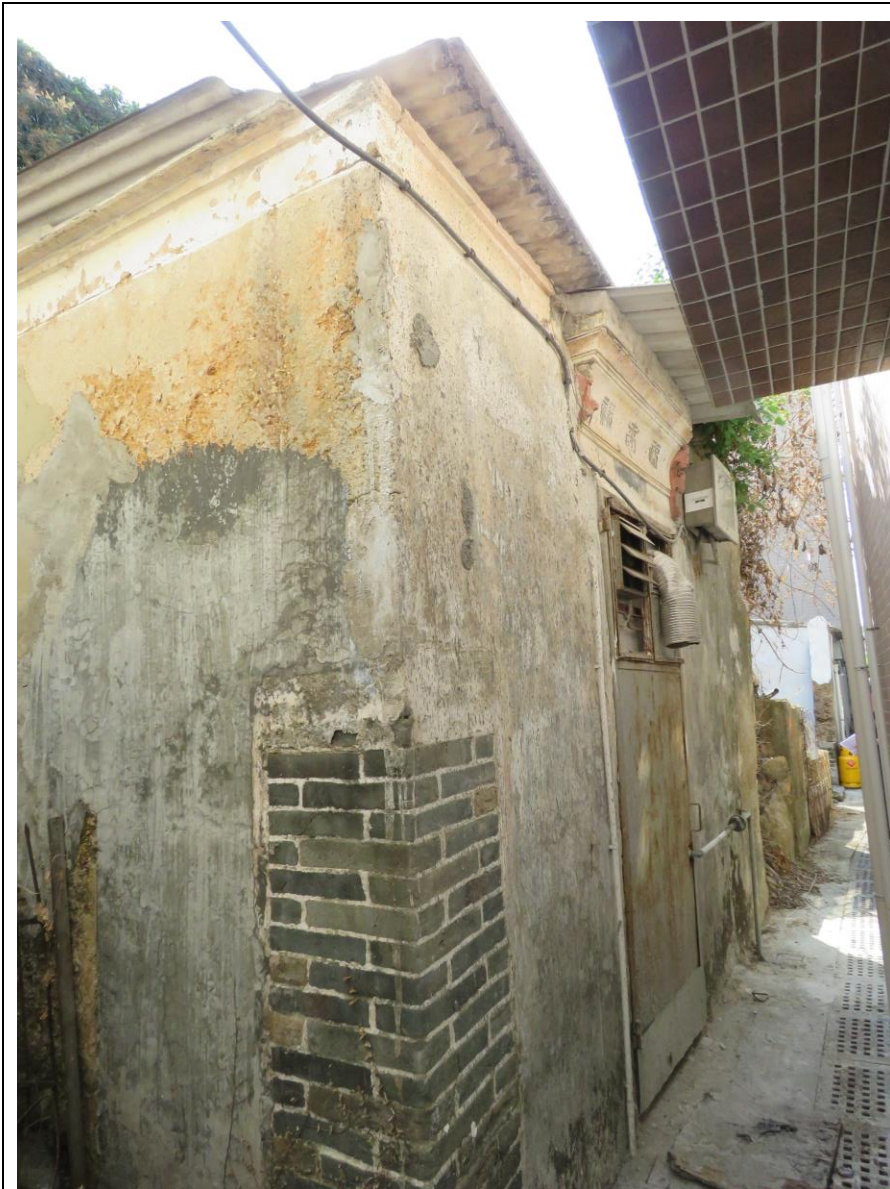
Front view of HB-32, looking southwest.
