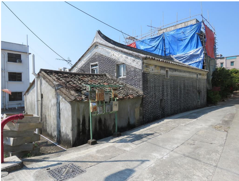
Side and back view of GB-01, showing southeast and northeast elevations, looking northwest.
