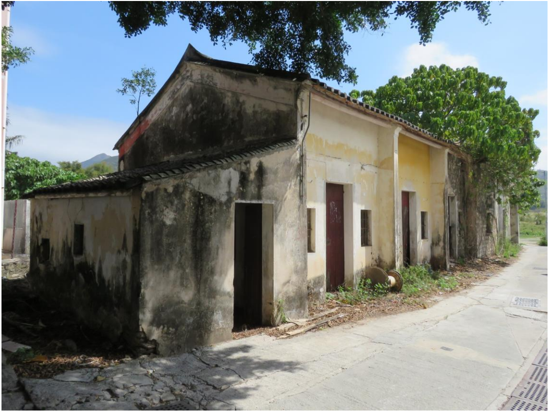
General view of HB-52, looking southeast.
