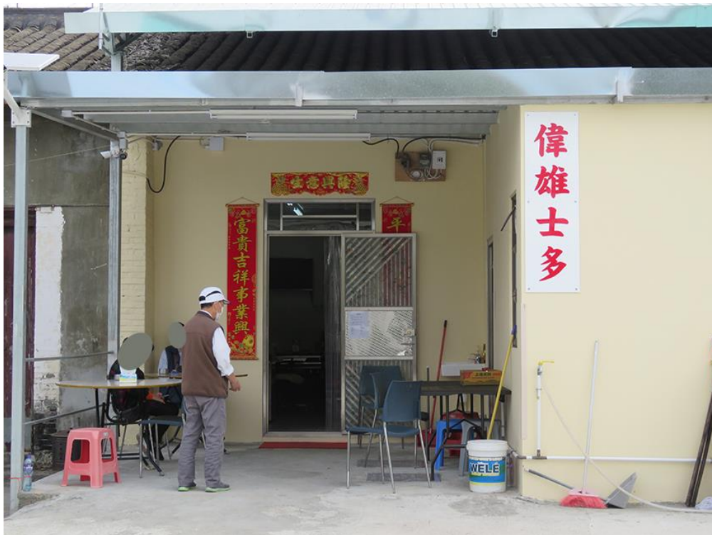
Façade view of No.56, looking east.
