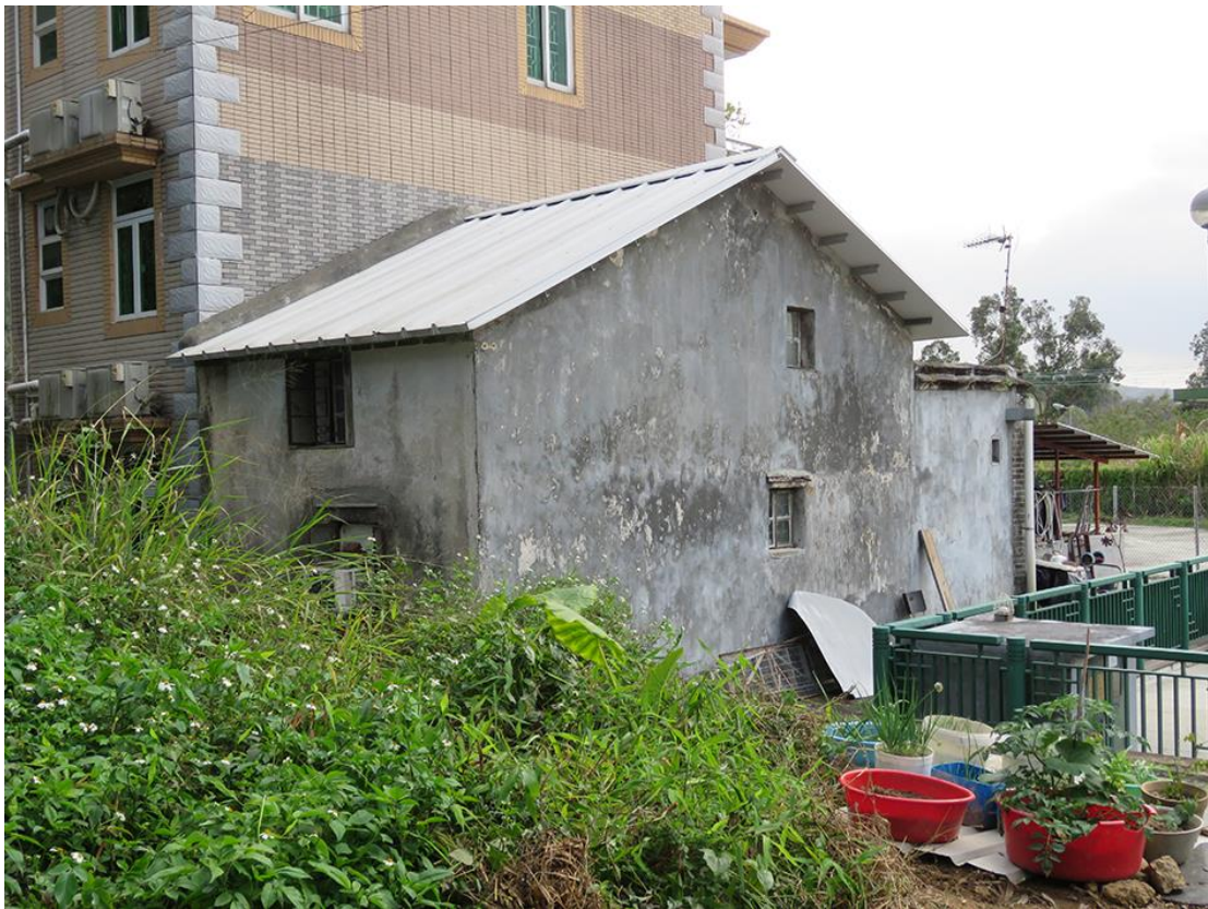
Back and side view, HB-26, showing northeast and northwest elevations, looking south.
