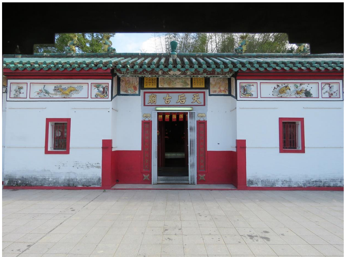
Façade of Tin Hau Temple, looking southeast.
