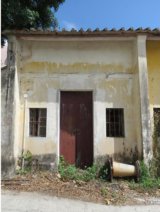
Façade view of No.133, looking northeast.
