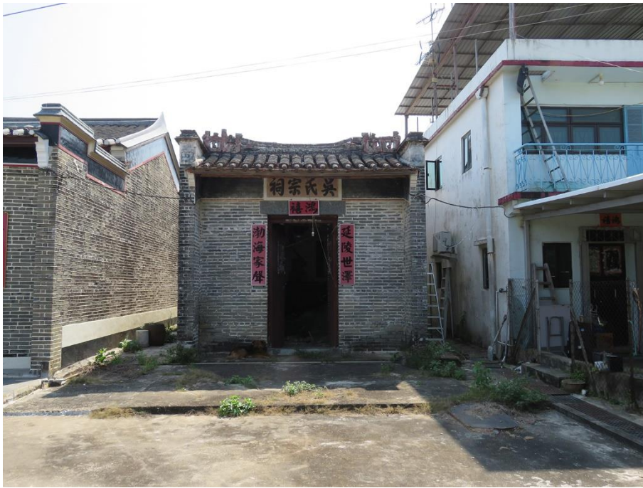
Façade view of GB-02, looking southeast.
