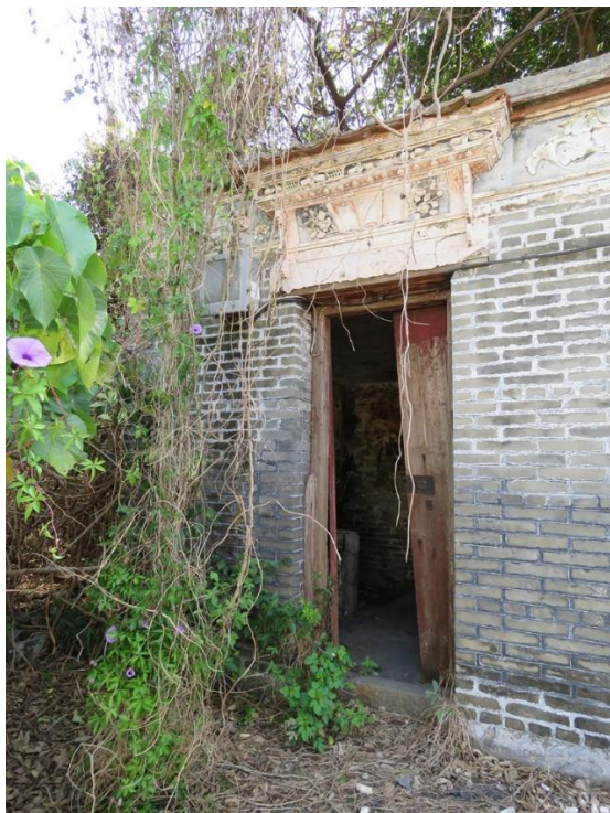
Façade of No.27, looking southeast.
