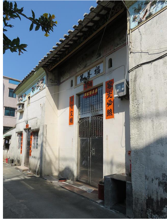
Front view of No. 9, looking north.
