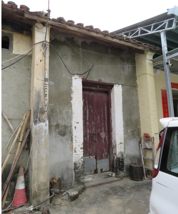
Façade view of No.55, looking southeast.
