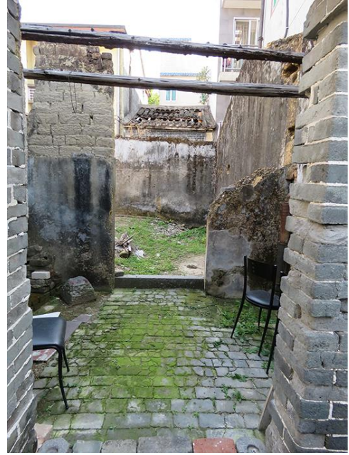
Internal view of ruin, looking southeast.
