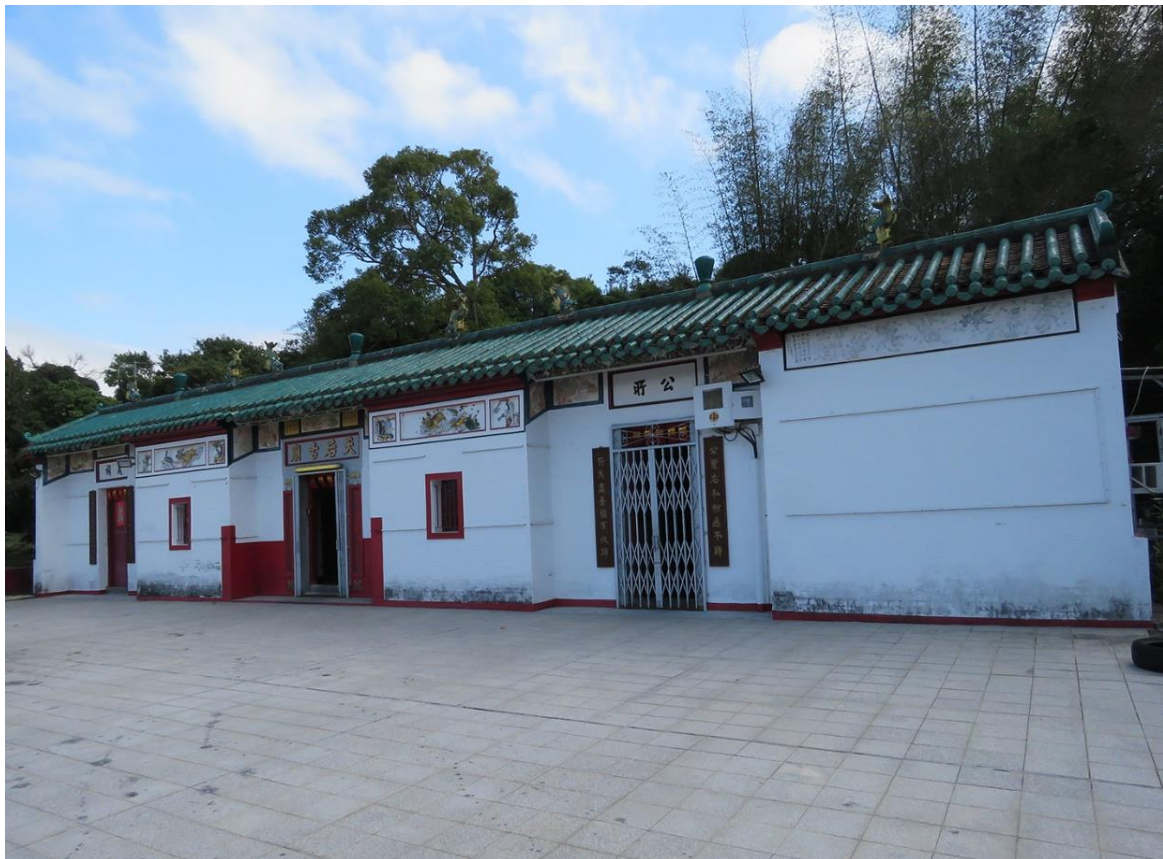
Façade view of GB-09, looking southeast.
