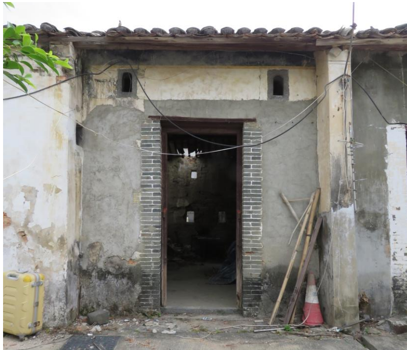
Façade view of No.54, looking east.
