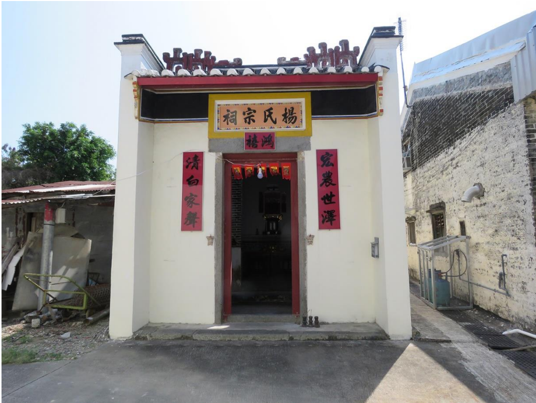
Façade view of GB-04, looking southeast.
