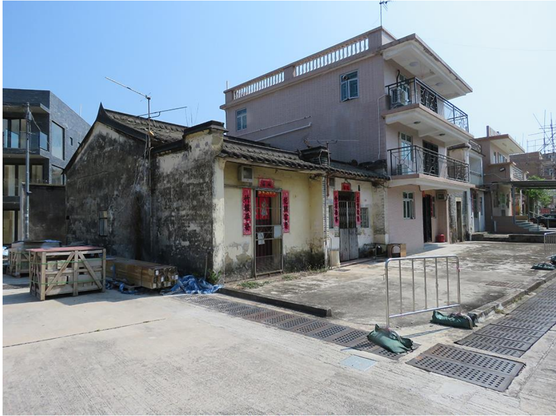
General view of HB-01, showing front and northwest elevations, looking east.
