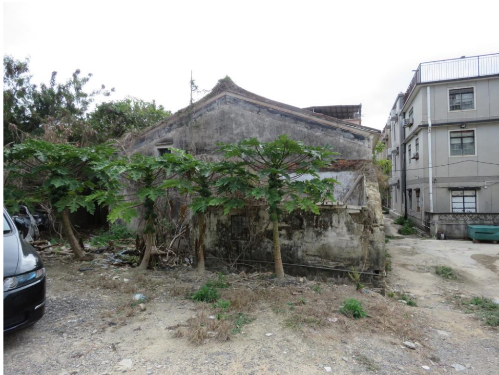
Side view of HB-16, showing northwest elevation, looking southeast.
