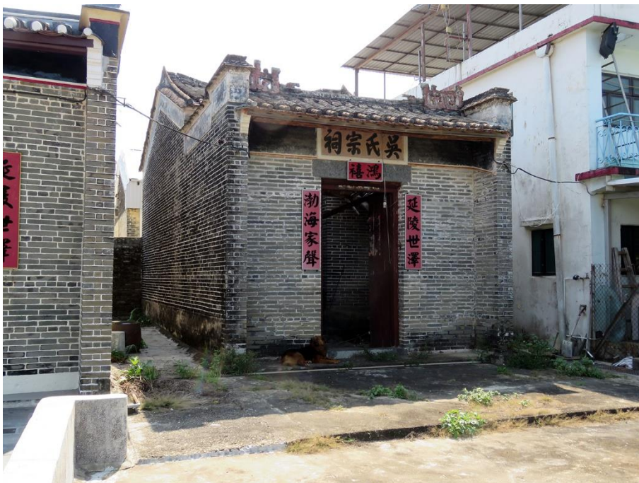
Side view of GB-02, showing façade and northeast elevation, looking southwest.
