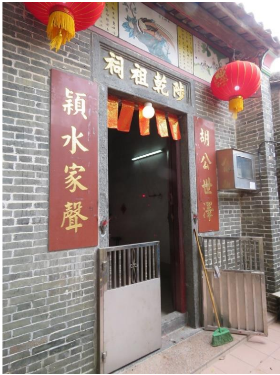
Façade view of GB-07, looking southeast.
