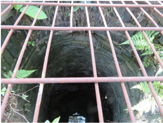
Brick lining of HB-24, looking southwest.
