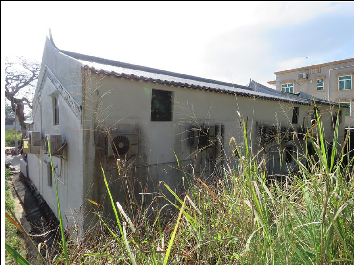
Side and back view, showing southeast and northeast elevations, looking no
