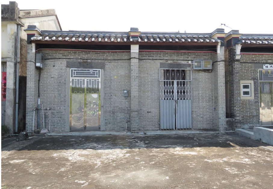
Façade view of GB-03, looking southeast.
