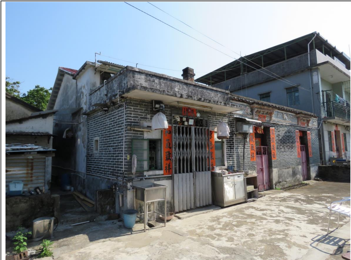
General view of HB-37, showing northeast elevation and façade, looking south.
