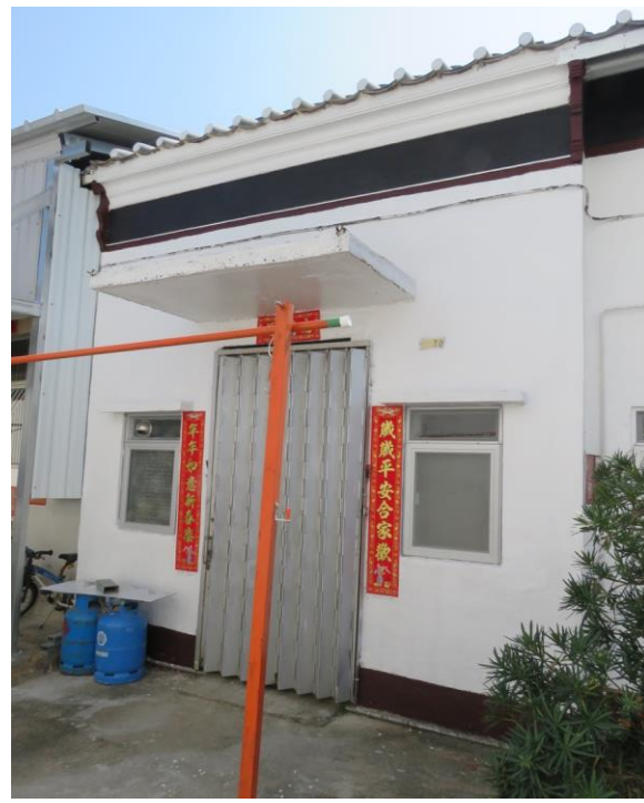
Façade of No.30, looking southeast.
