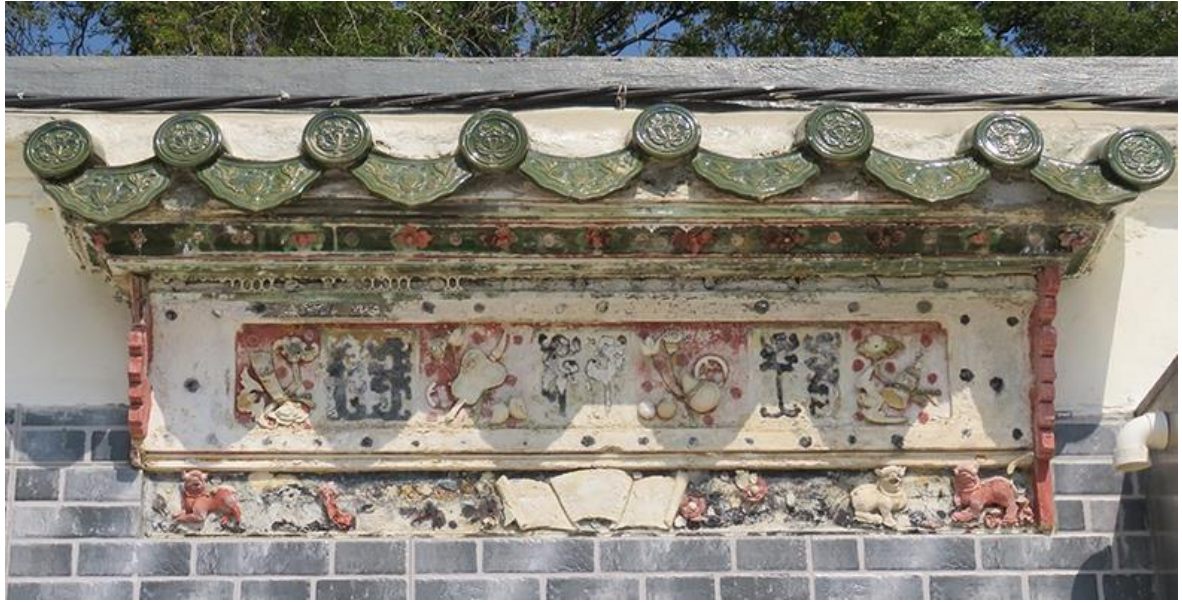
Close up of the façade (No.20)
