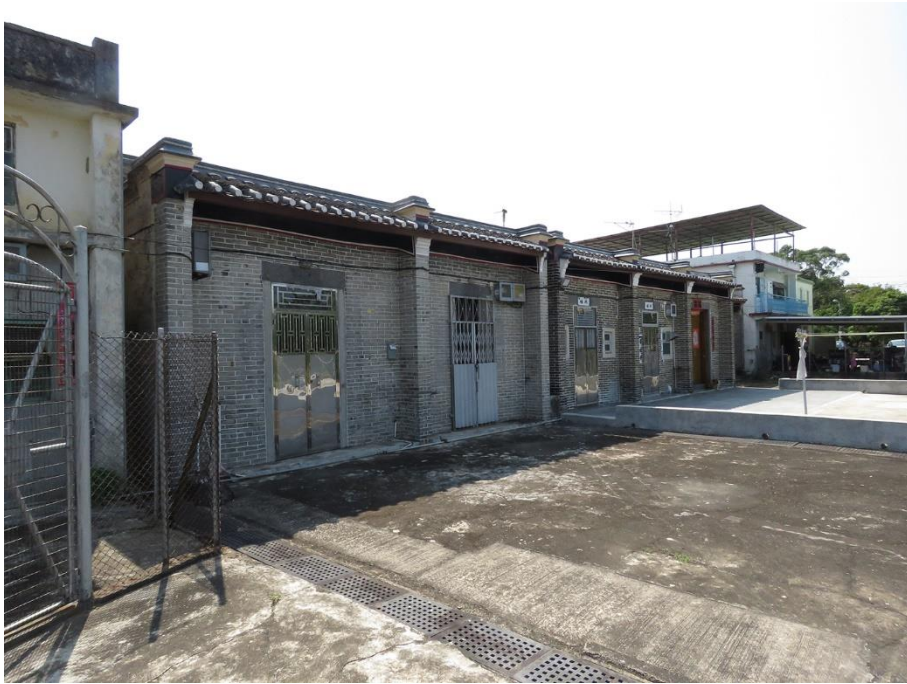
General view of GB-03, looking southwest.
