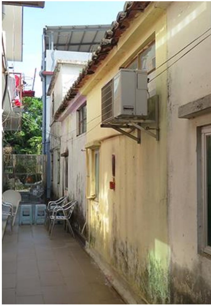
Back view, showing northeast elevation, looking southeast.
