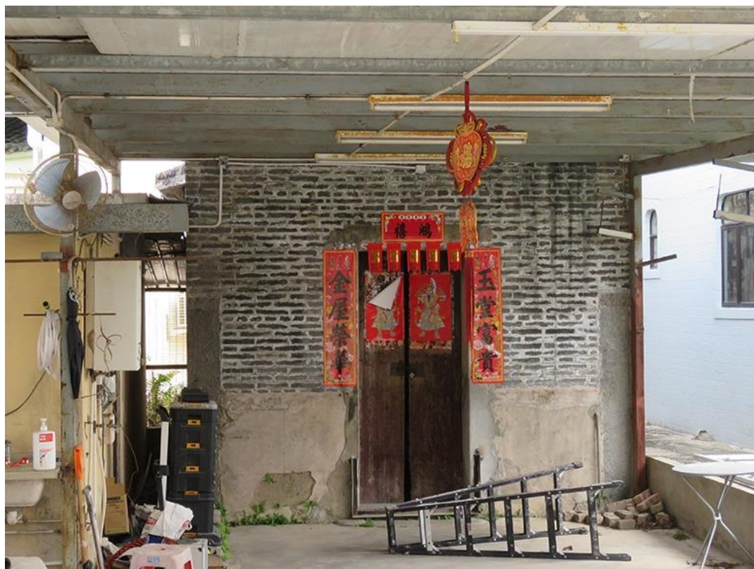
Front view of HB-44, looking northeast.
