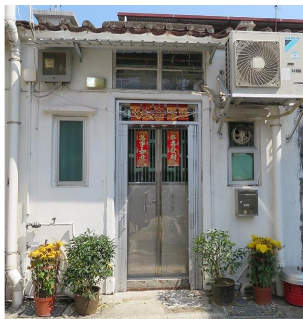
Close up of façade (No. 23B)
