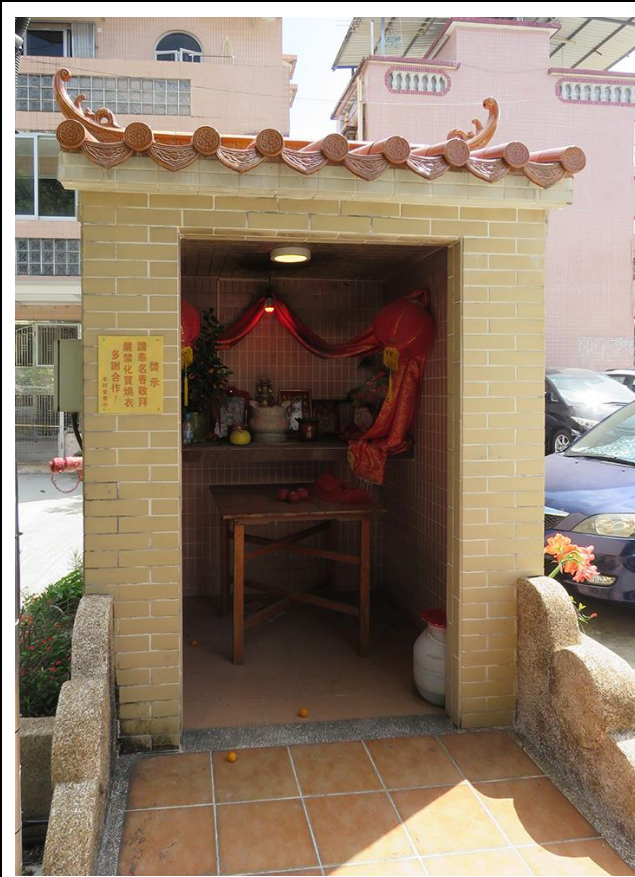
Front view of HB-51, looking east-south-east.
