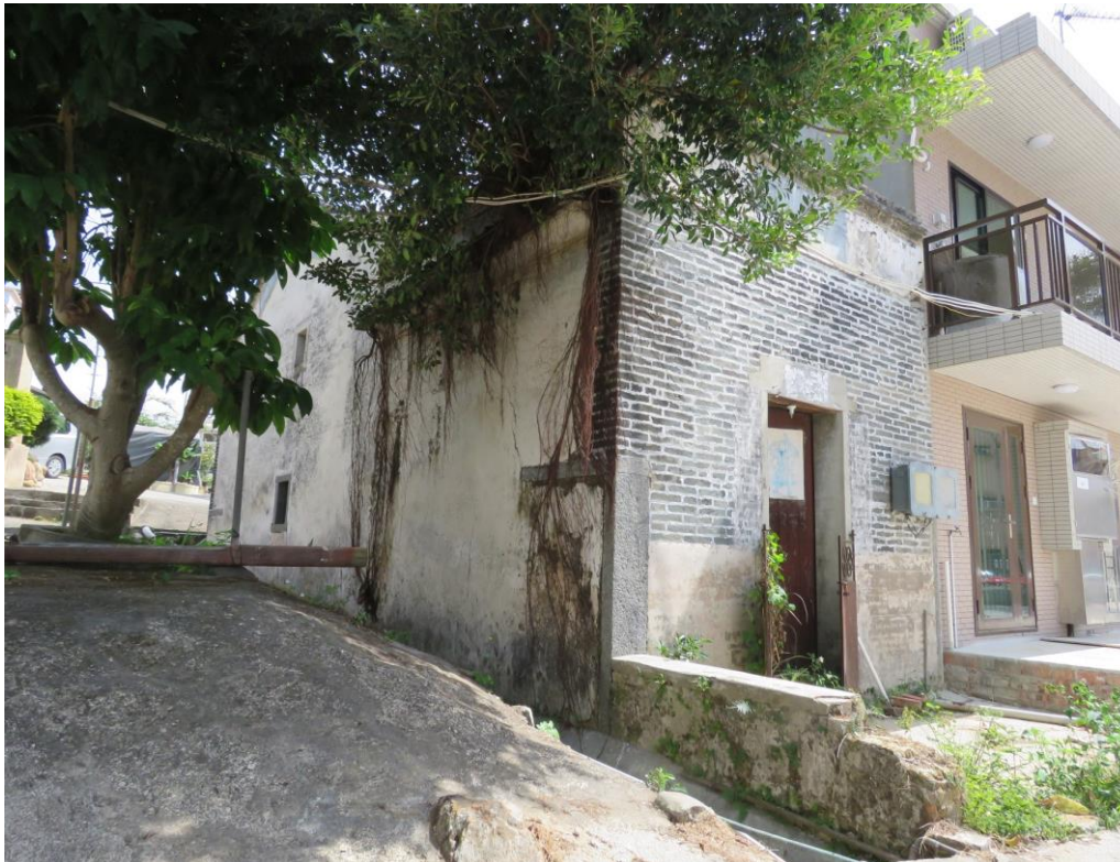
Side and front view, showing northwest elevation and façade, looking east.
