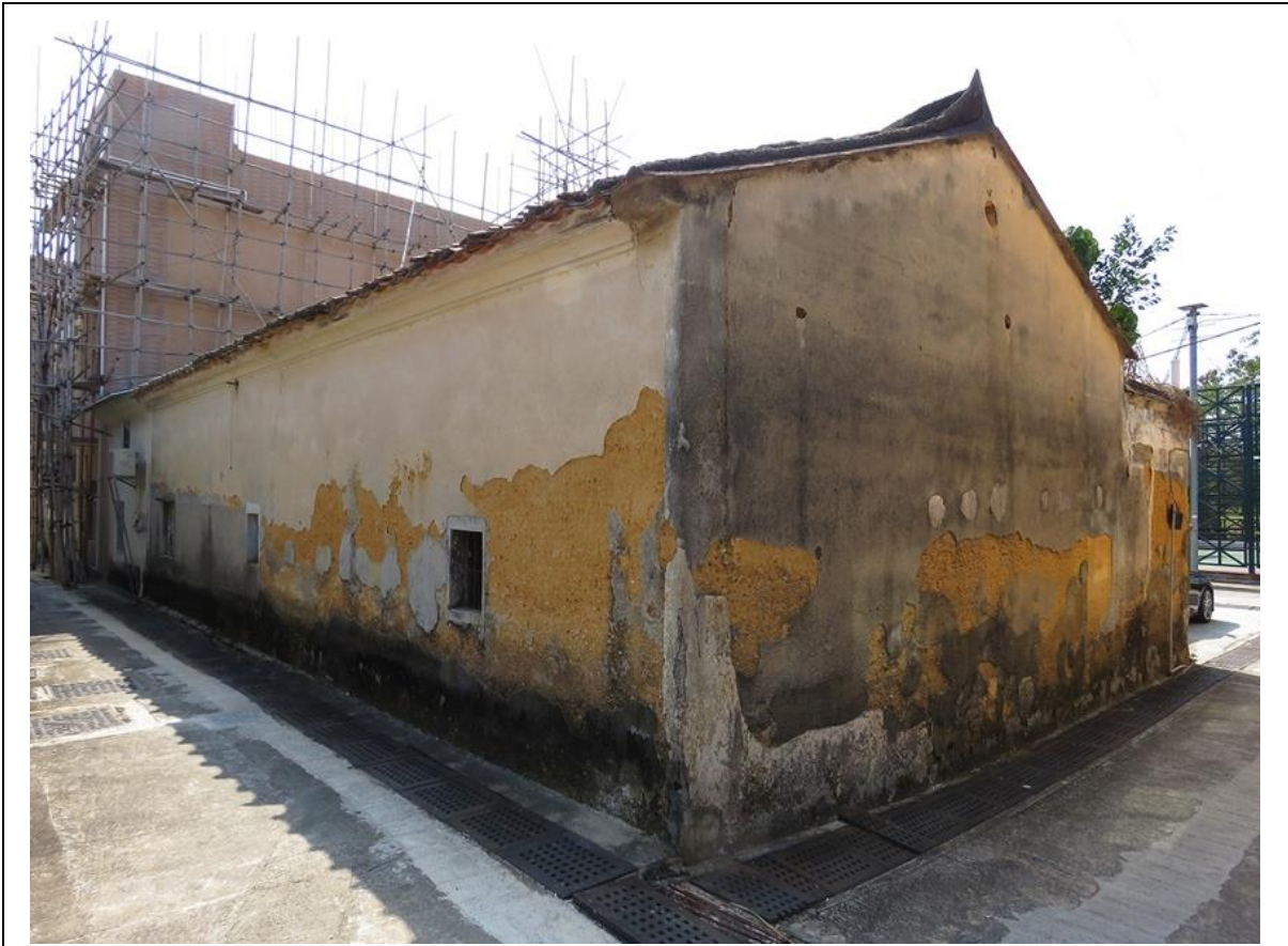
Back and side view, showing northeast and northwest elevations, looking south.
