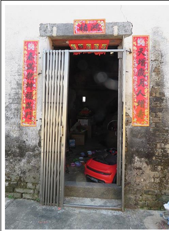
Close up of the façade (No.21A)
