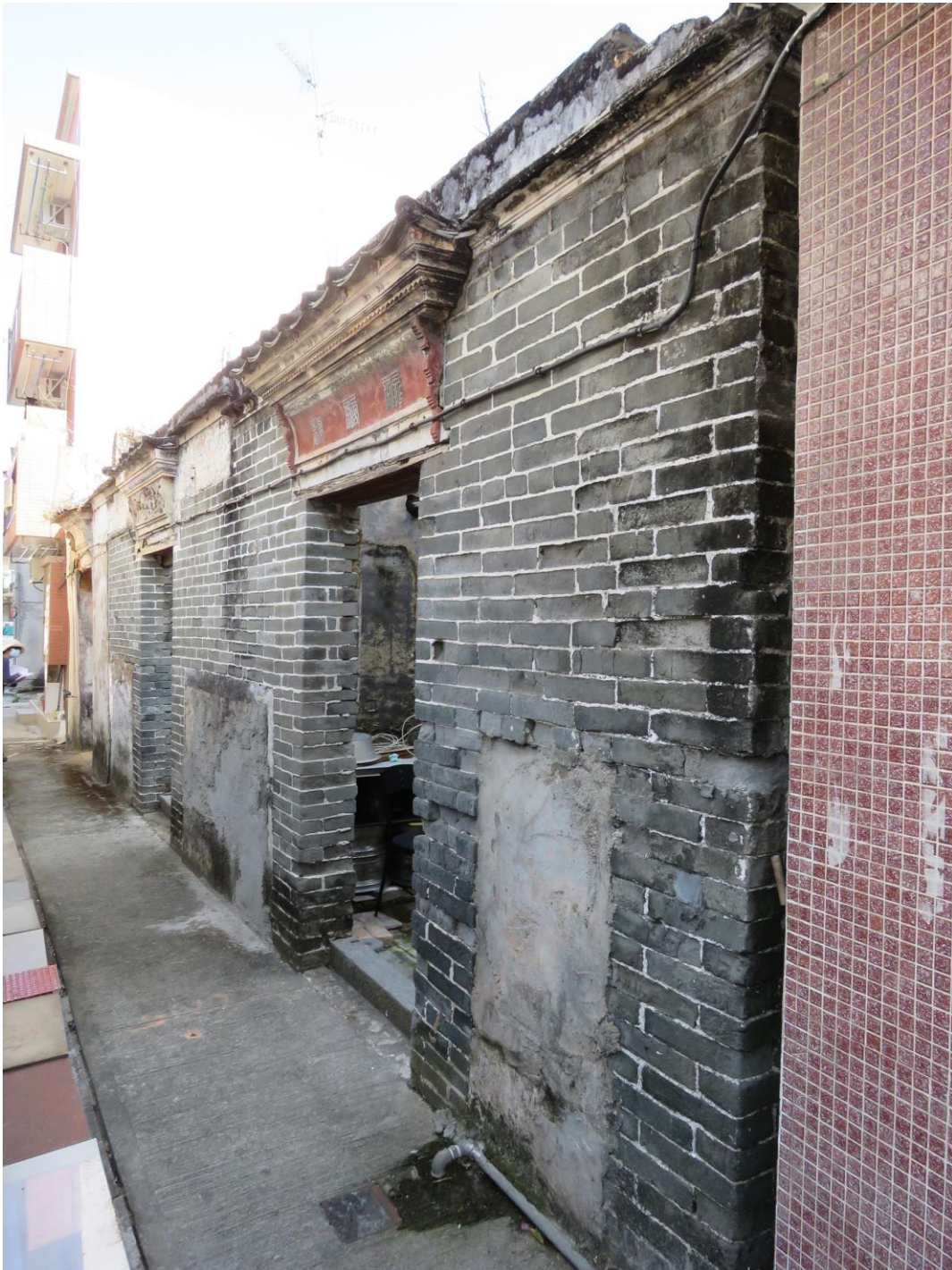
Front view of HB-39, looking southeast.
