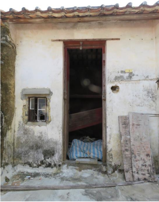
Façade of northeast bay of No.17, looking southeast.
