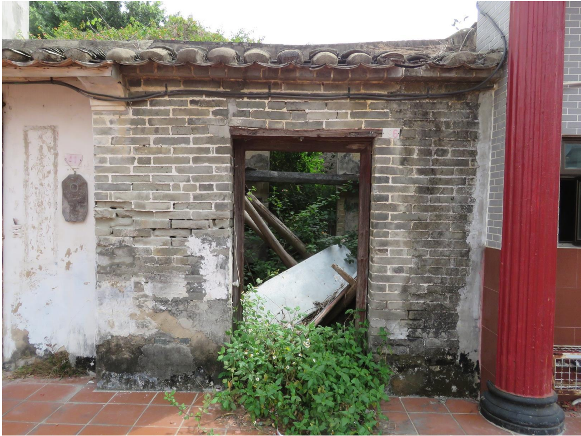
Façade view of No.96, looking east-southeast.
