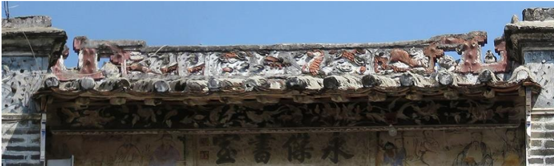
Decoration of door canopy
