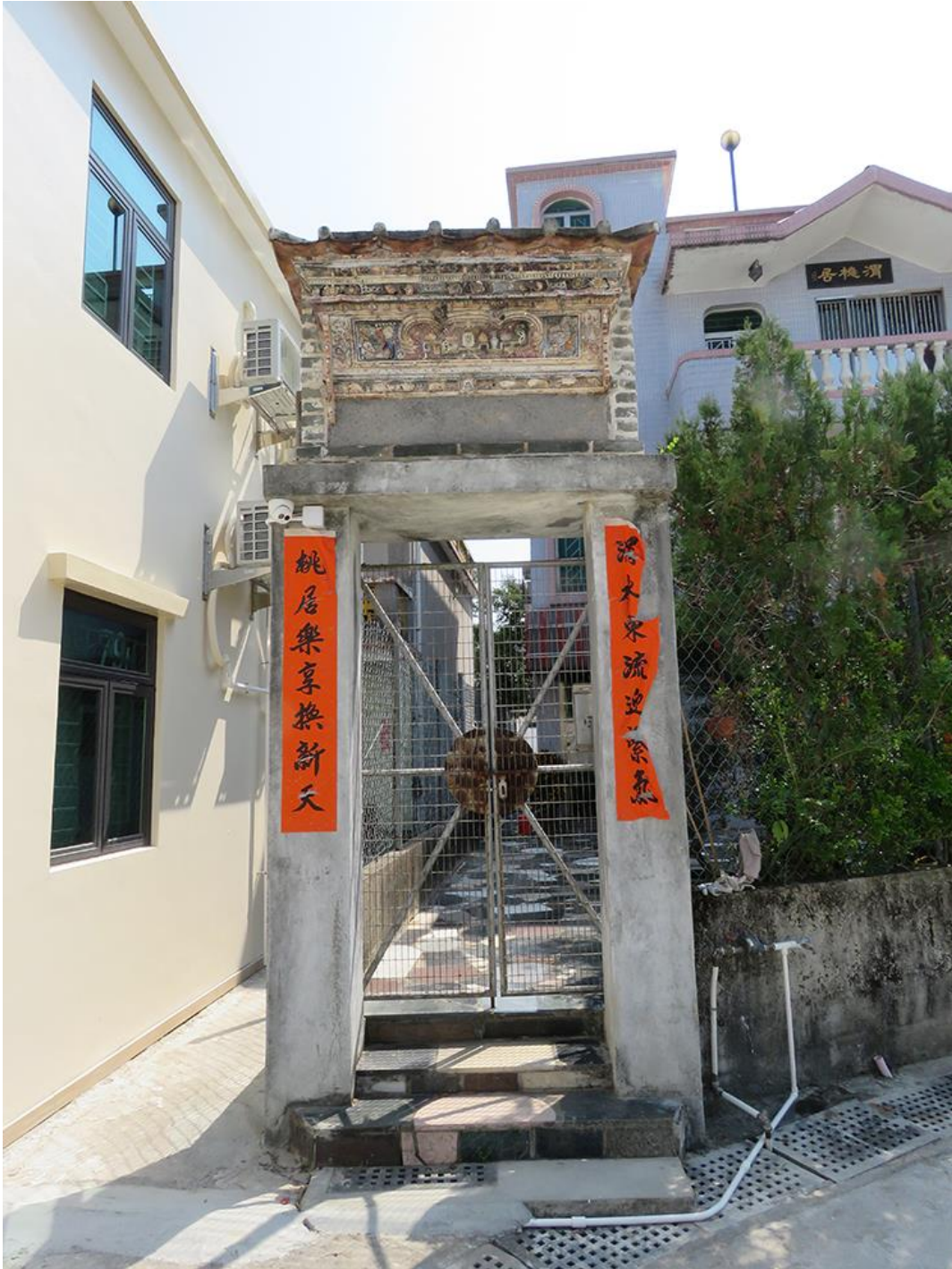
Front view of HB-23, looking southeast.
