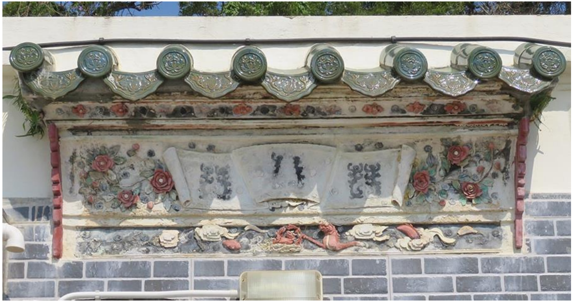
Close up of the façade (No.20)
