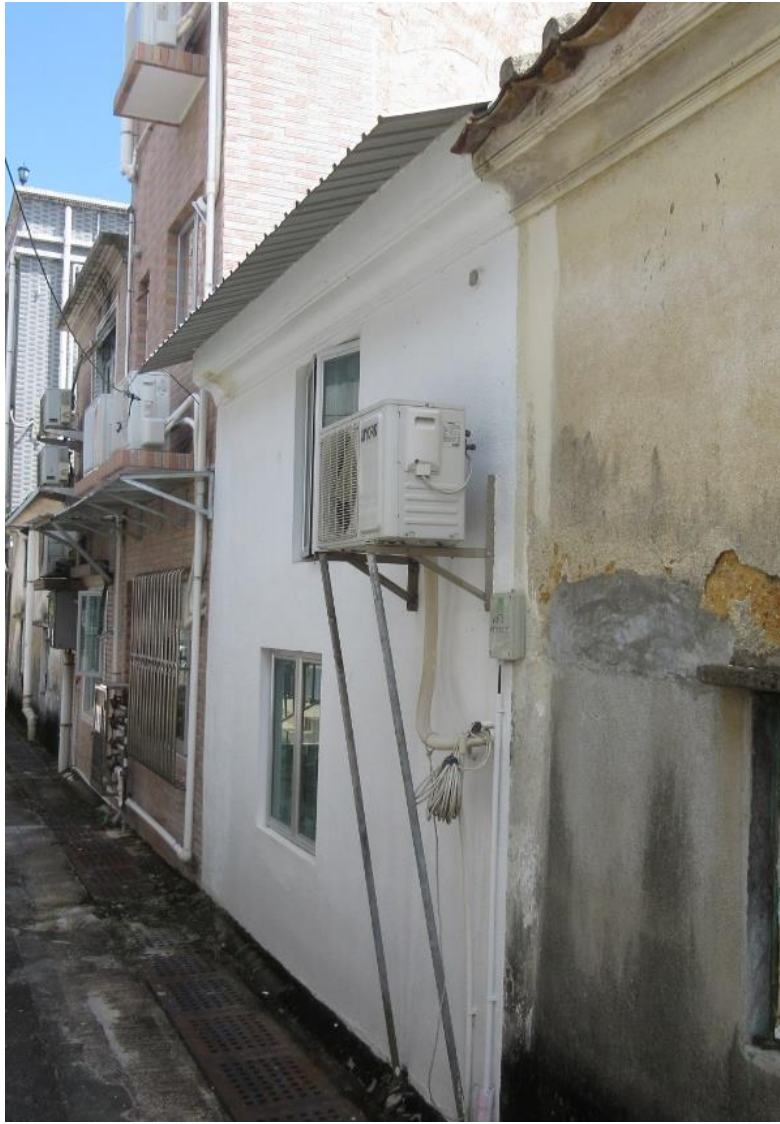
Rear view of HB-66, looking west.
