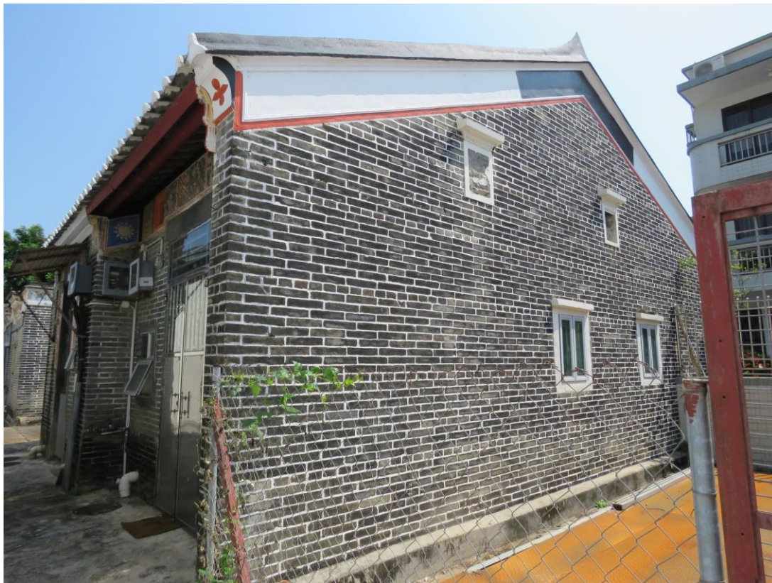
Front and side view, showing façade and northwest elevations, looking southeast.
