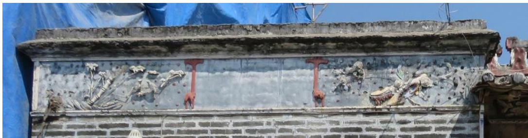
Plaster moulding on façade wall
