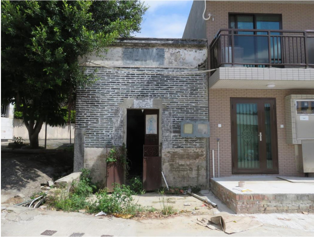
Front view of HB-47, looking northeast.
