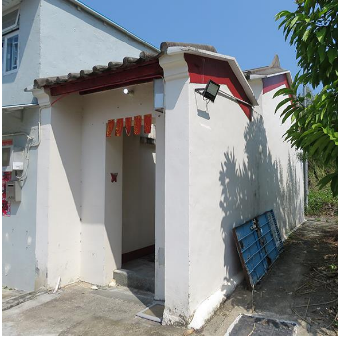
Front and side view of HB-08, showing façade and southeast elevation, looking north.
