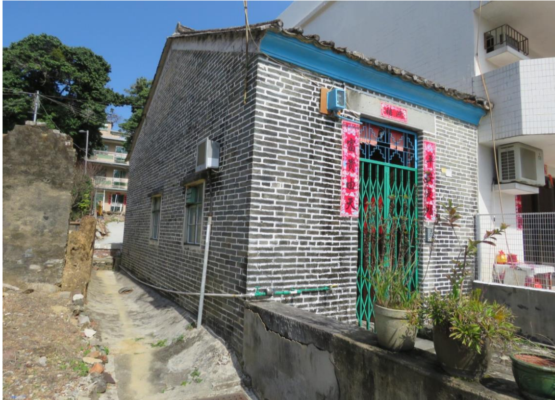
Side view of HB-19, showing northwest elevation, looking northeast.
