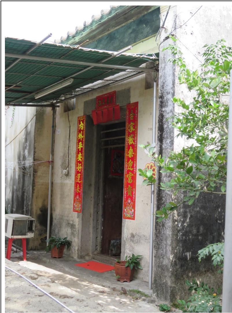
Close up of façade of the south-eastern end unit
