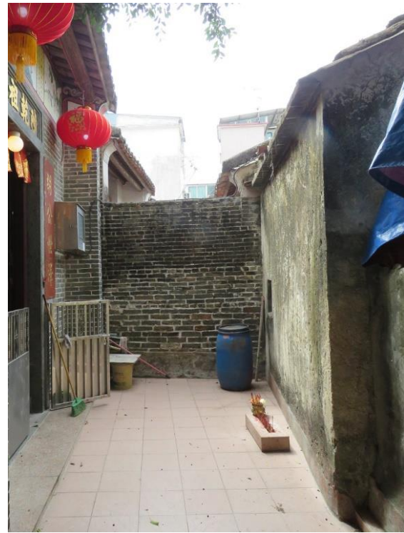
Side wall of GB-06, looking southwest.
