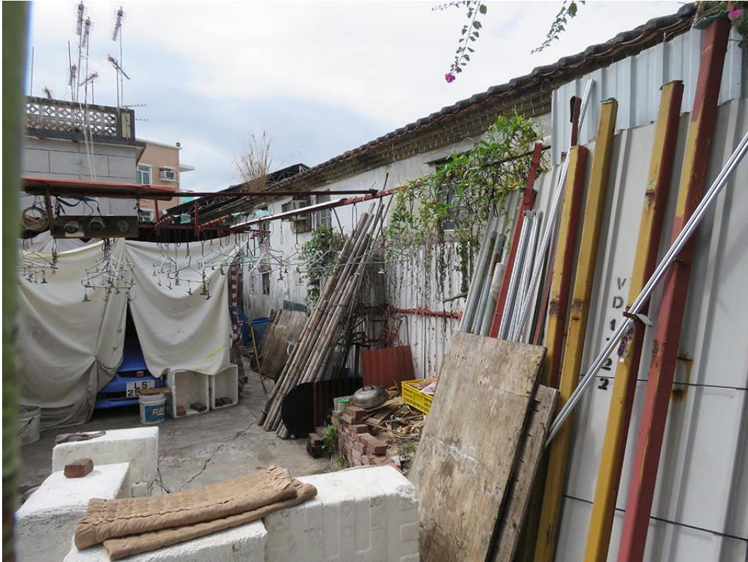
Back view of HB-43, showing east elevation, looking south.
