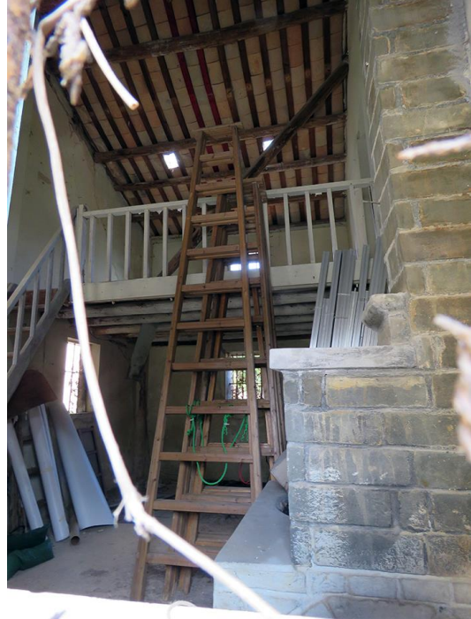
Internal view of No.133, looking northeast.
