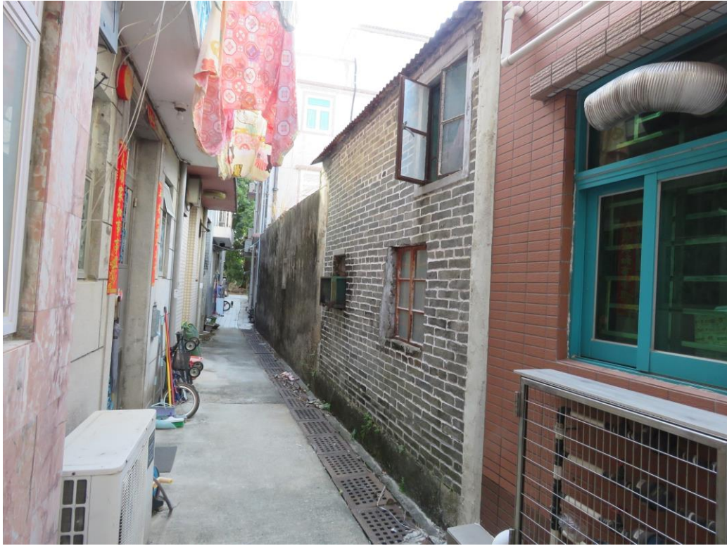
Back view of HB-39, showing south elevation, looking northwest.
