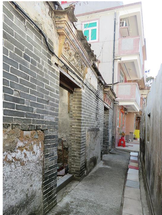
Façade of No.12A, looking southwest.
