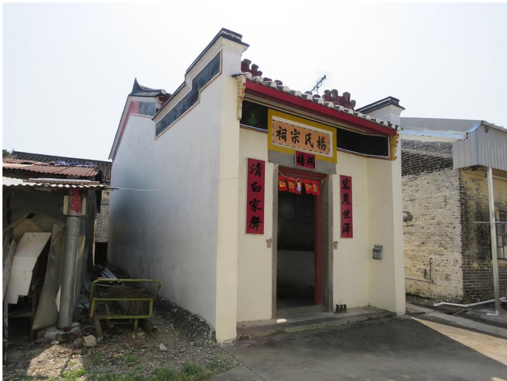
Side view of GB-04, showing façade and northeast elevation, looking southwest.
