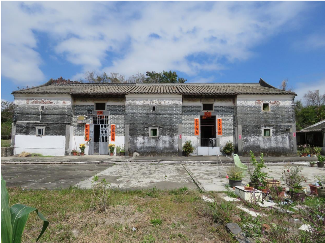
Front view of GB-08, looking northeast.
