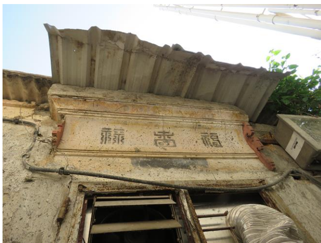
Close up of the façade
