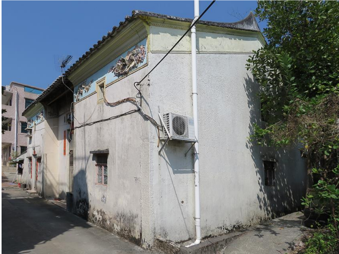
General view of HB-28, showing façade and southeast elevation, looking north.
