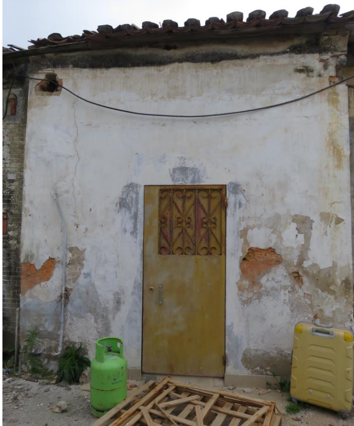
Façade view of No.53B, looking east.
