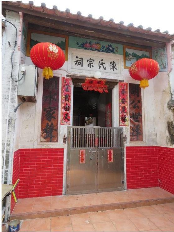
Façade view of GB-06, looking southeast.
