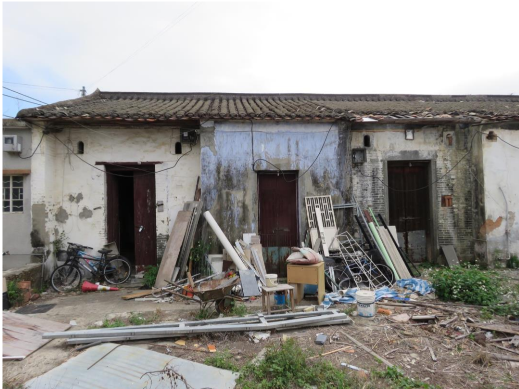
Façade view of No.51, 52 and 53, looking east.
