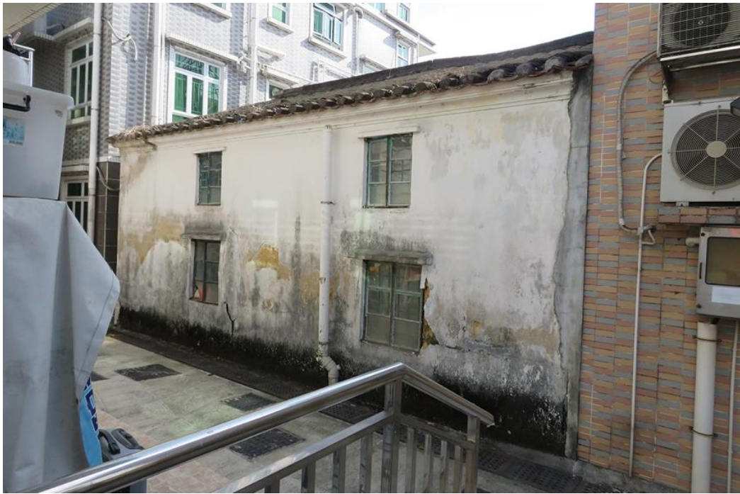
Back view of HB-04, showing northeast elevation, looking southeast.
