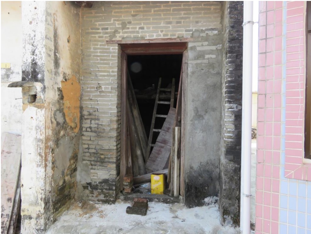
Façade of southwest bay of No.17, looking southeast.
