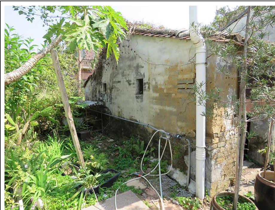
Side view, showing façade and northwest elevation, looking east.
