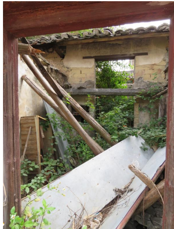
Internal view of No.96, looking east-southeast.
