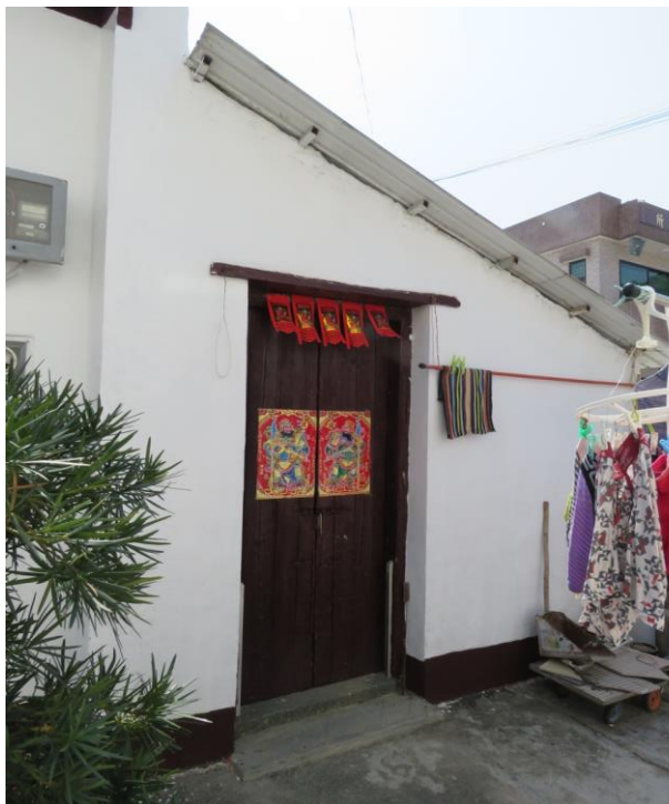
Façade of side building of No.31, looking southwest.
