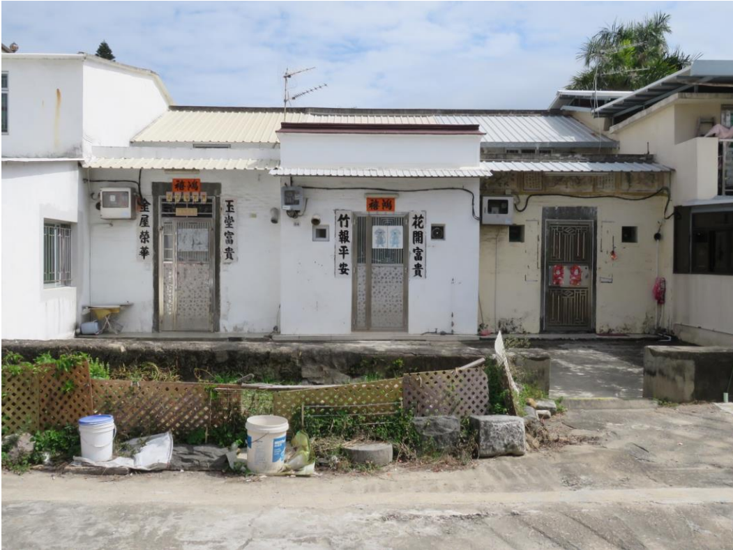
Front view of HB-46, looking northeast.
