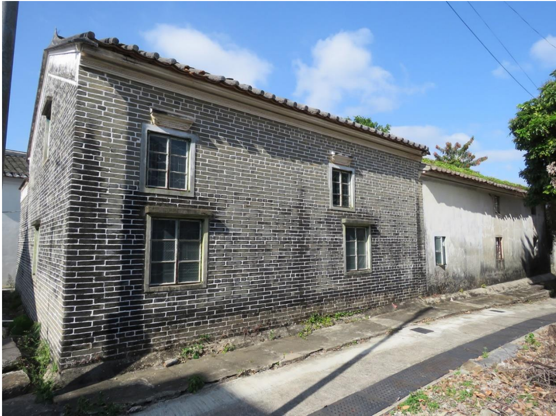
Back view, showing southeast elevation, looking northeast.
