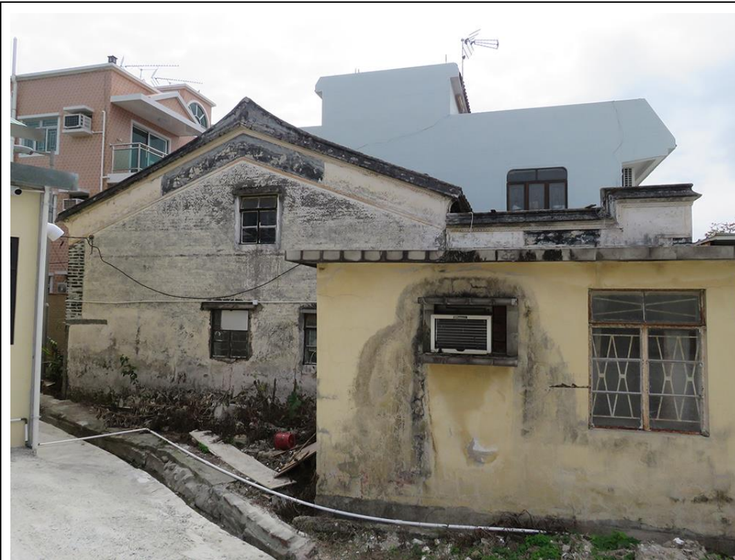
Side view of HB-44, showing northwest elevation, looking southeast.
