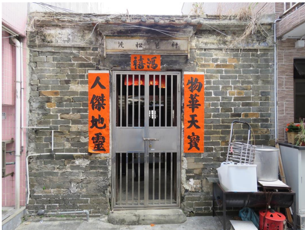
Front view of HB-63, looking east-south-east.
