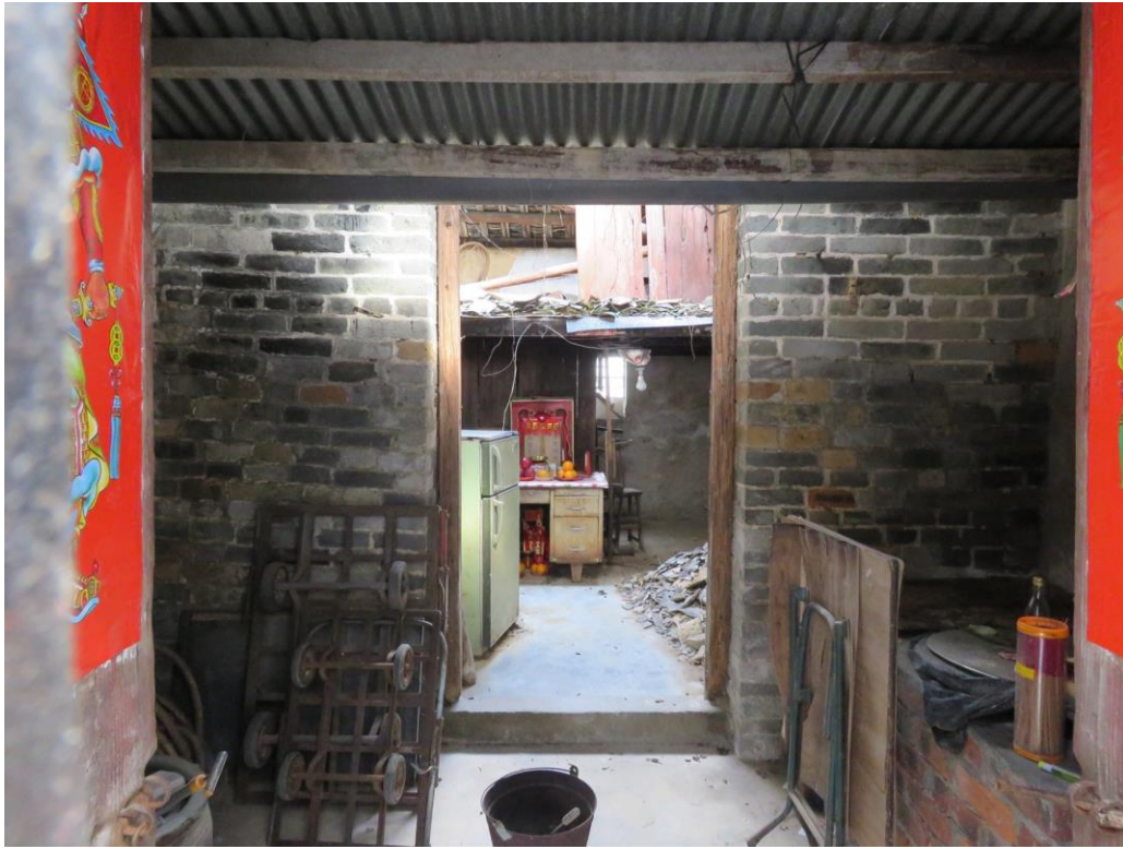
Internal view of HB-63, looking east-south-east.
