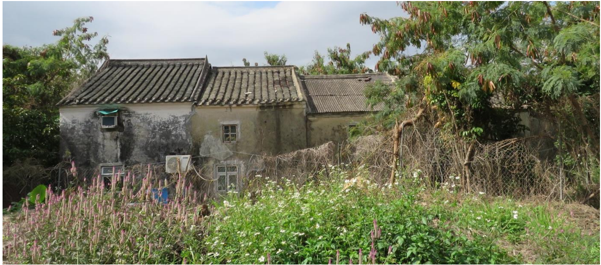
Back view of HB-15, showing northeast elevation, looking southwest.
