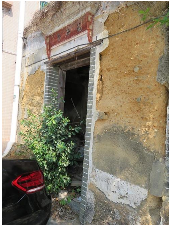
Façade of No. 6A, looking northwest.
