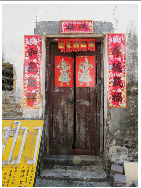
Close up of the façade (No.21)
