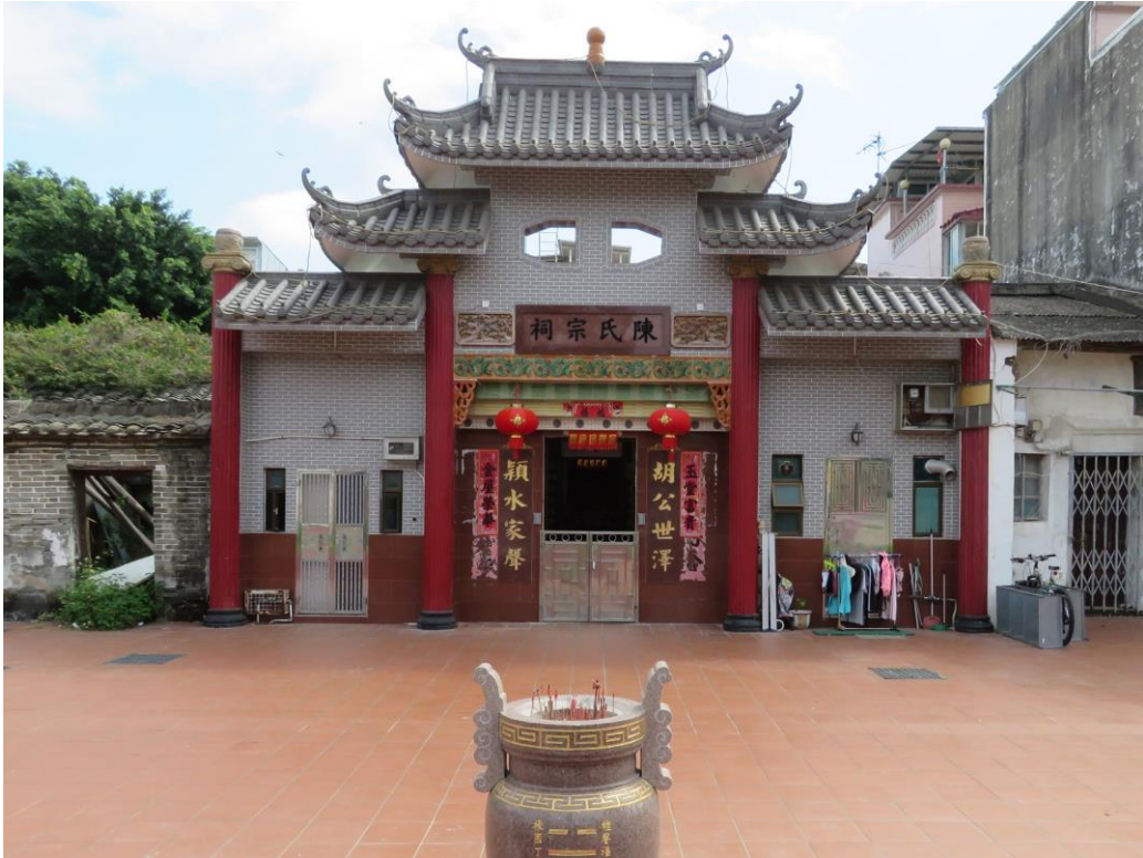
Front view of HB-49, looking southeast.
