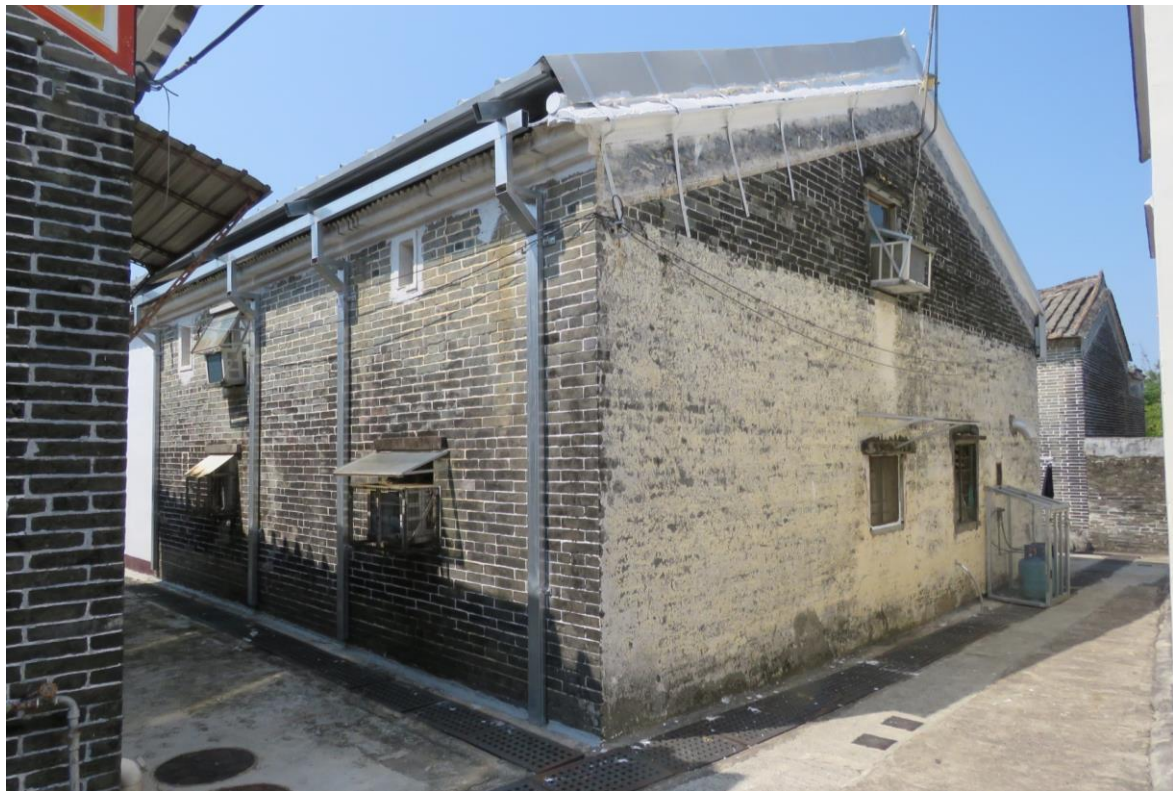
Side and back view, showing northeast and southeast elevations, looking northwest.
