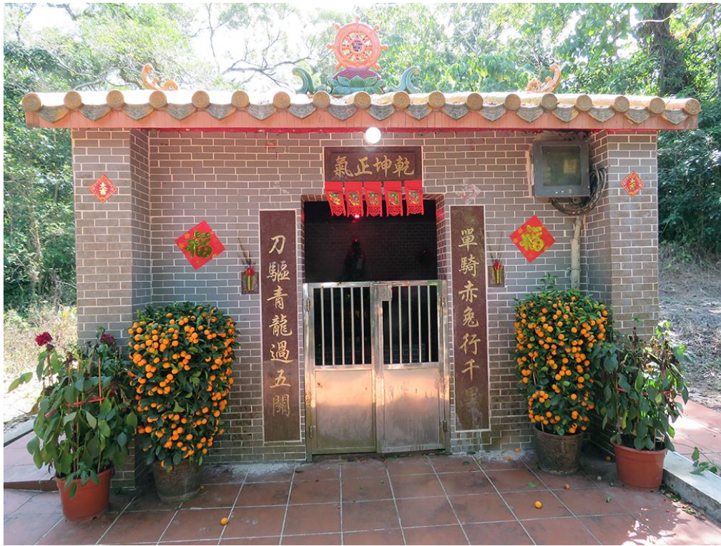
Front view of HB-56, looking southeast.
