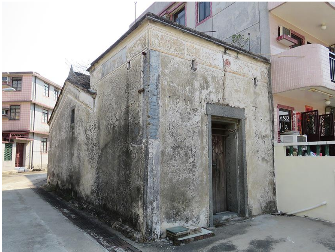
General view of HB-35, showing northeast elevation and façade, looking southwest.
