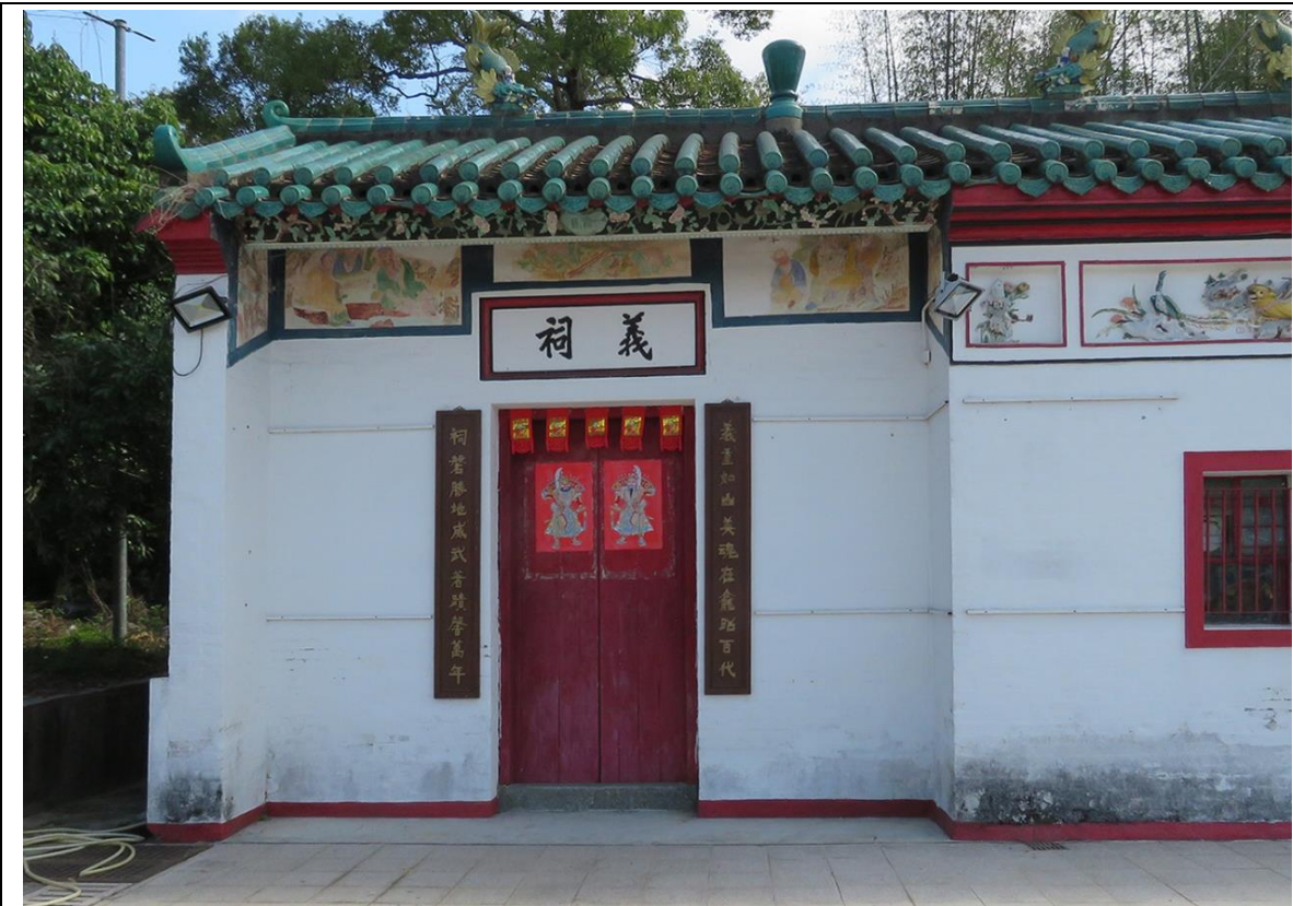
Façade of Yee Tsz, looking southeast.
