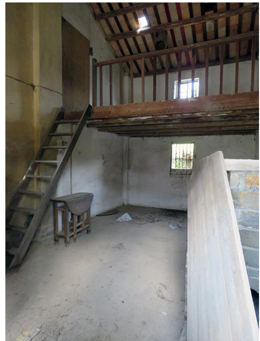
Internal view of No.134, looking northeast.
