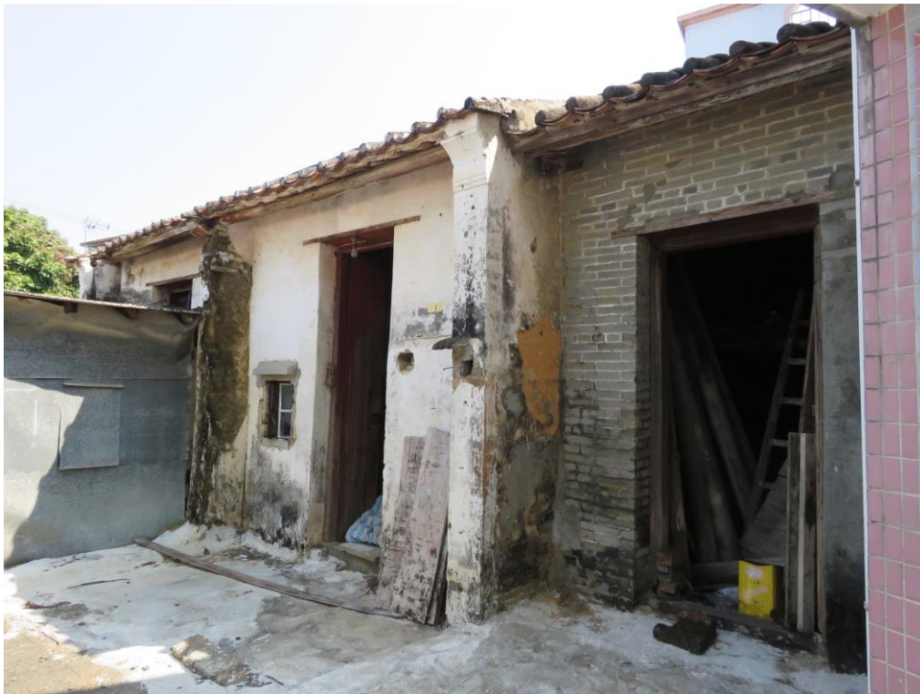
Façade view of HB-21, looking southeast.
