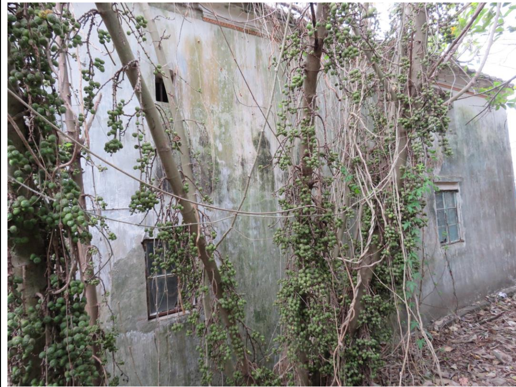
Back view of HB-16, showing northeast elevation, looking northwest.
