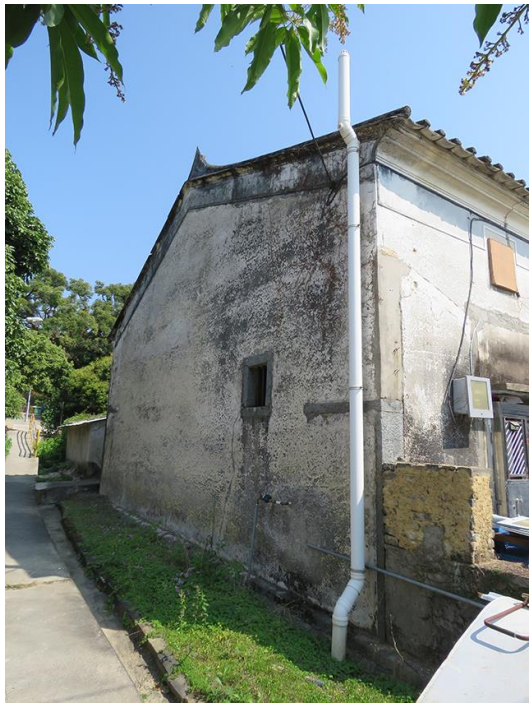
Side view of HB-29, showing northwest elevation, looking southeast.
