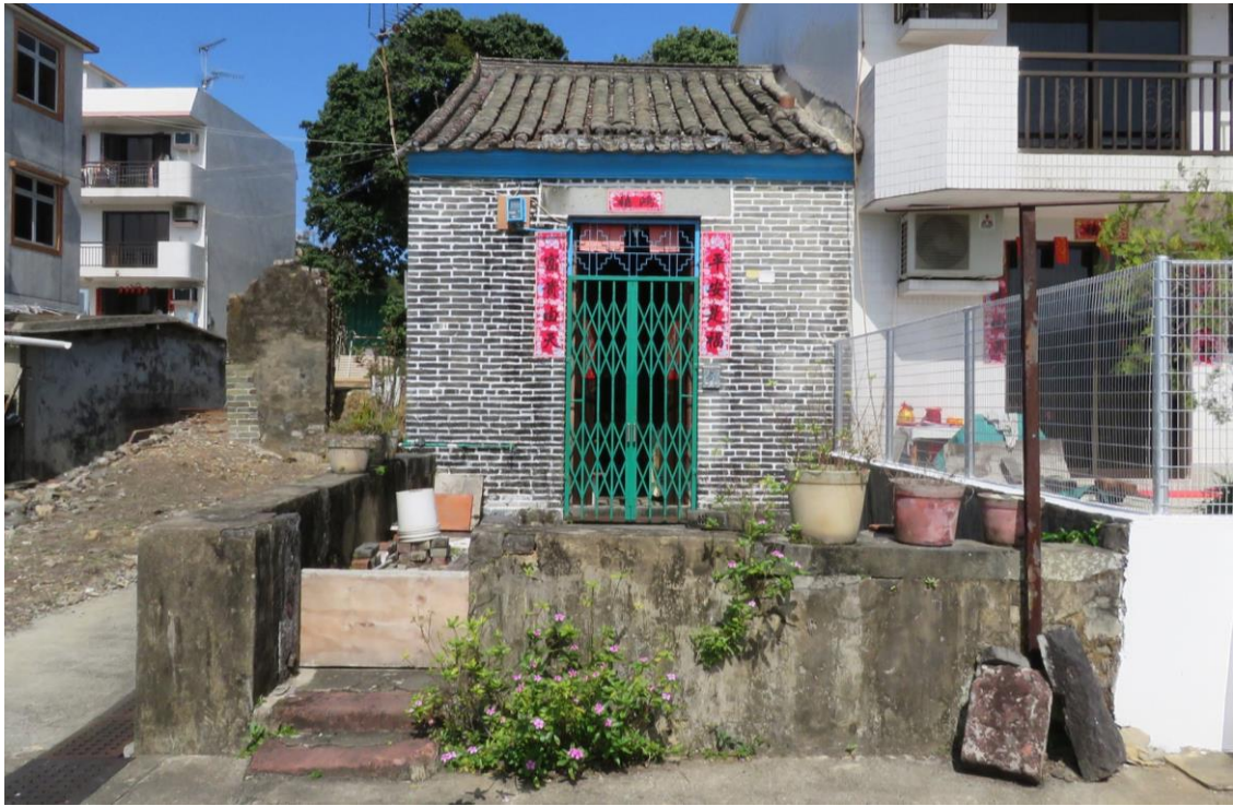
Front view of HB-19, looking northeast.
