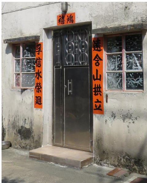
Close up of the right entrance façade
