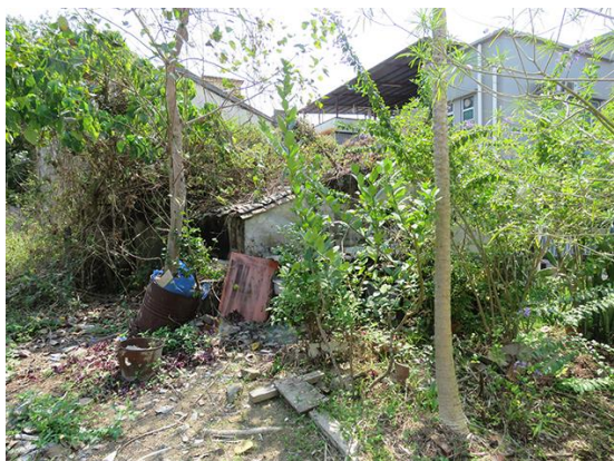
Back view, showing northeast elevation, looking south.
