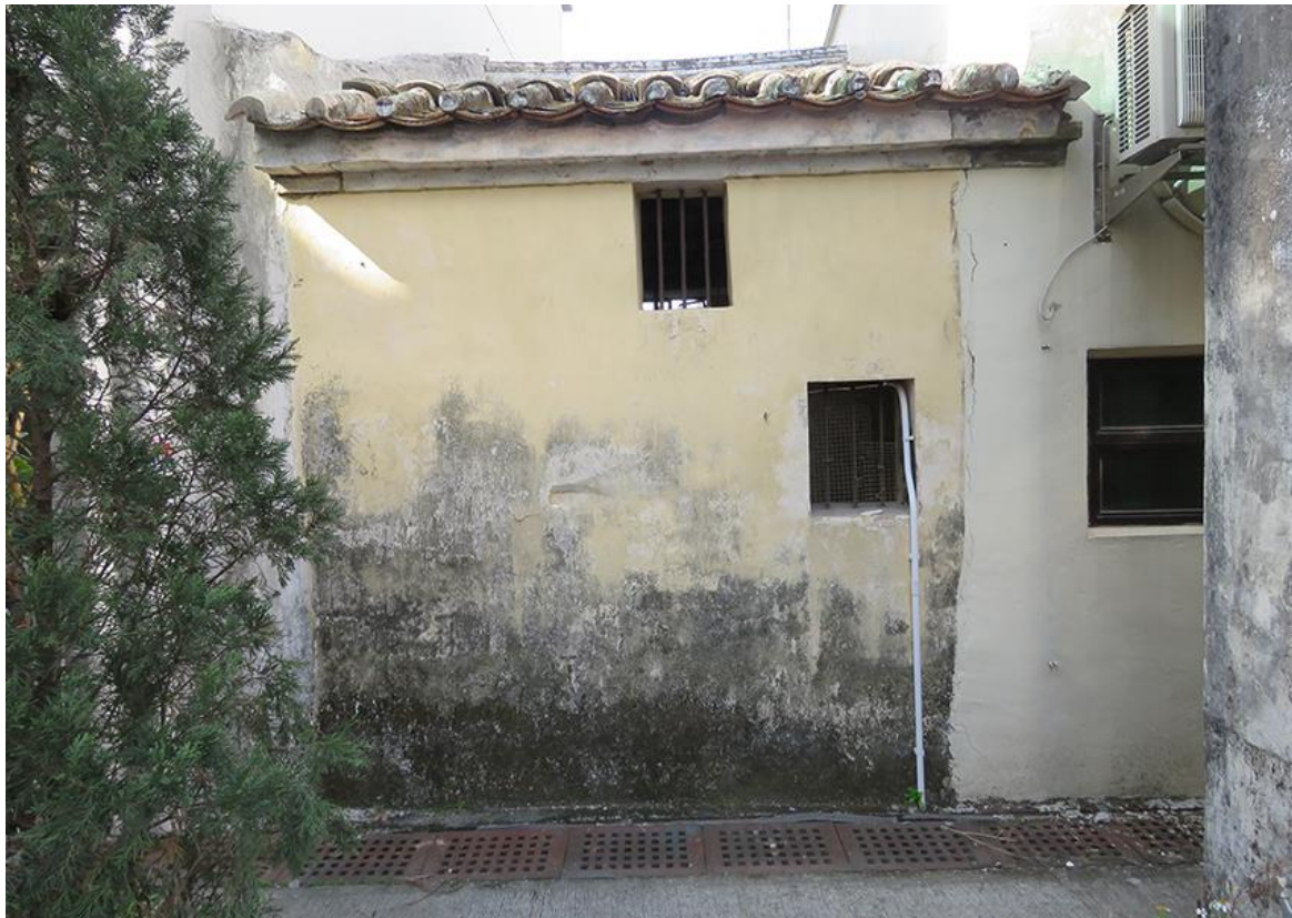
Back view of HB-34, showing south-south-east elevation, looking north-north-west.
