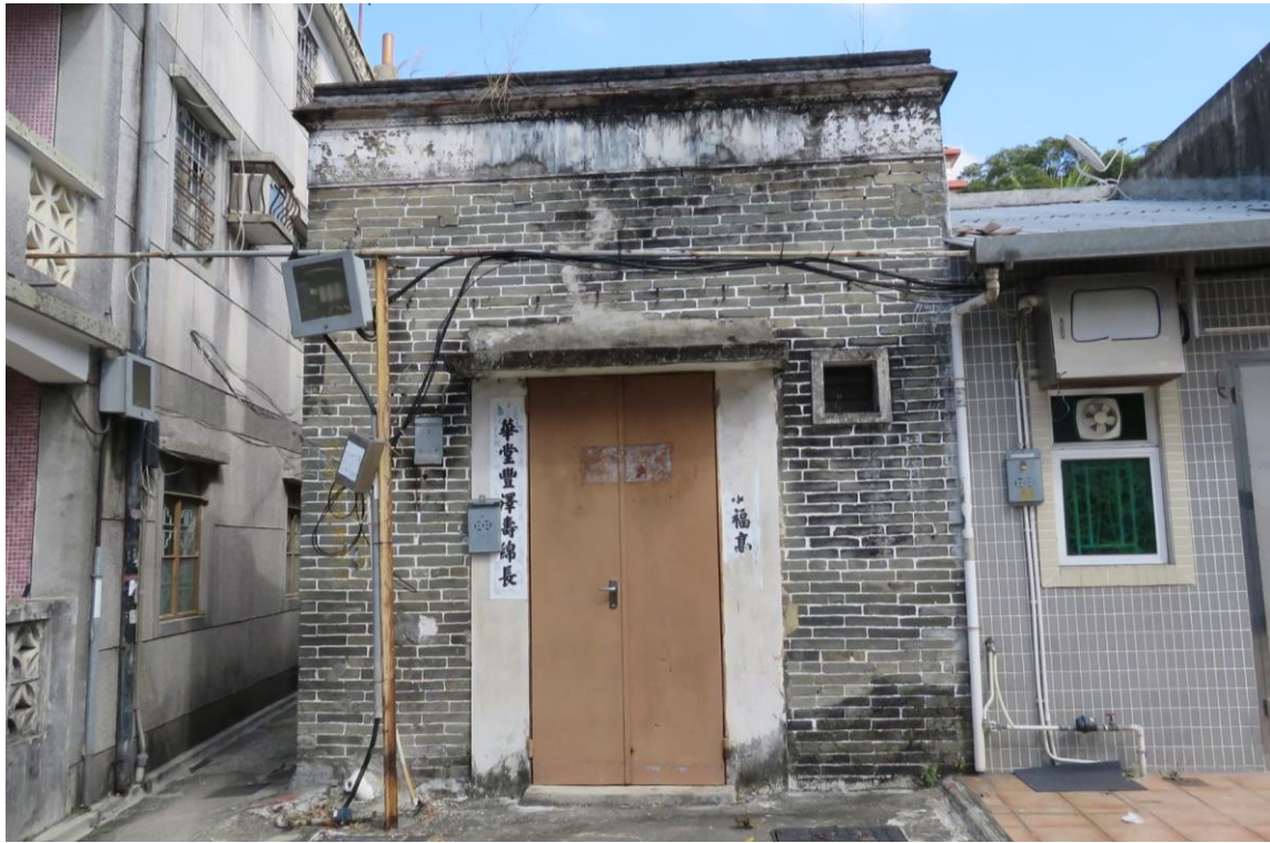
General view of HB-10, looking east.
