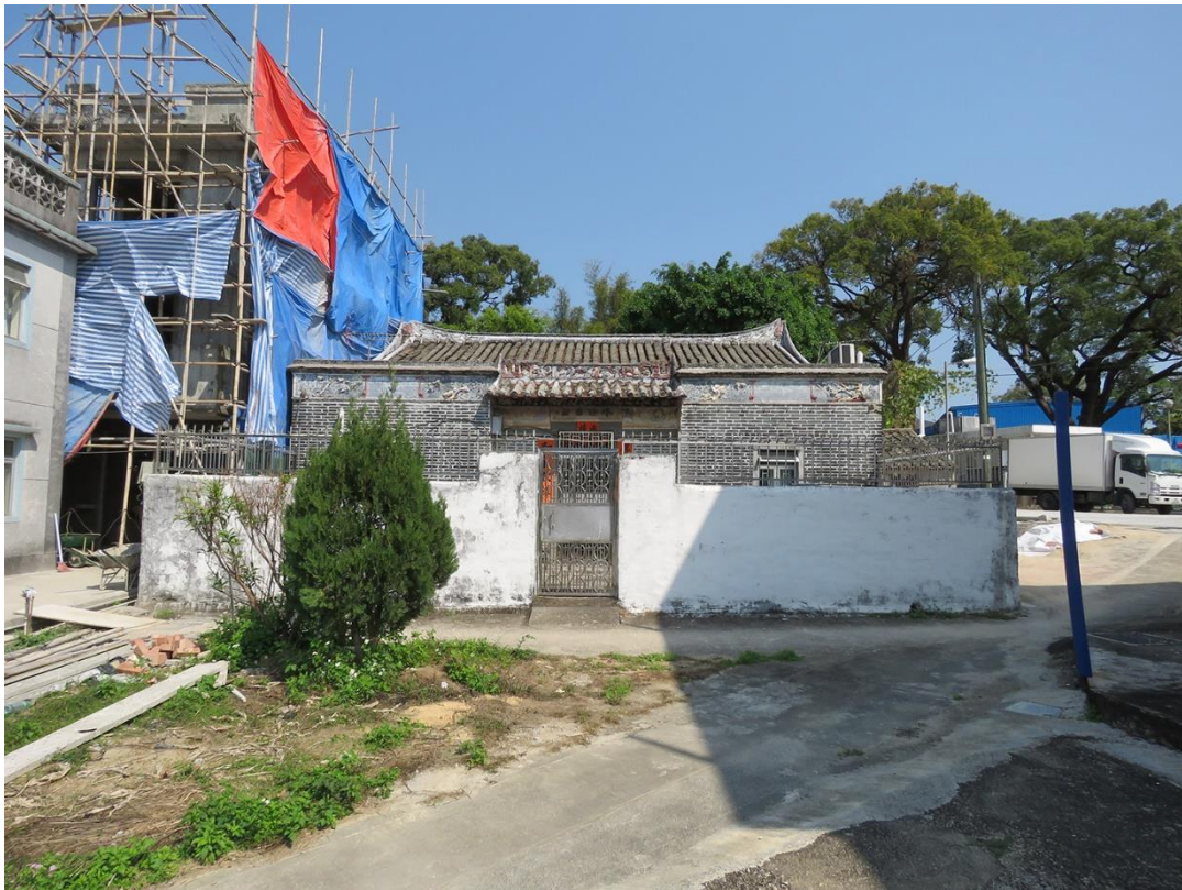
Front view of GB-01, looking northeast.
