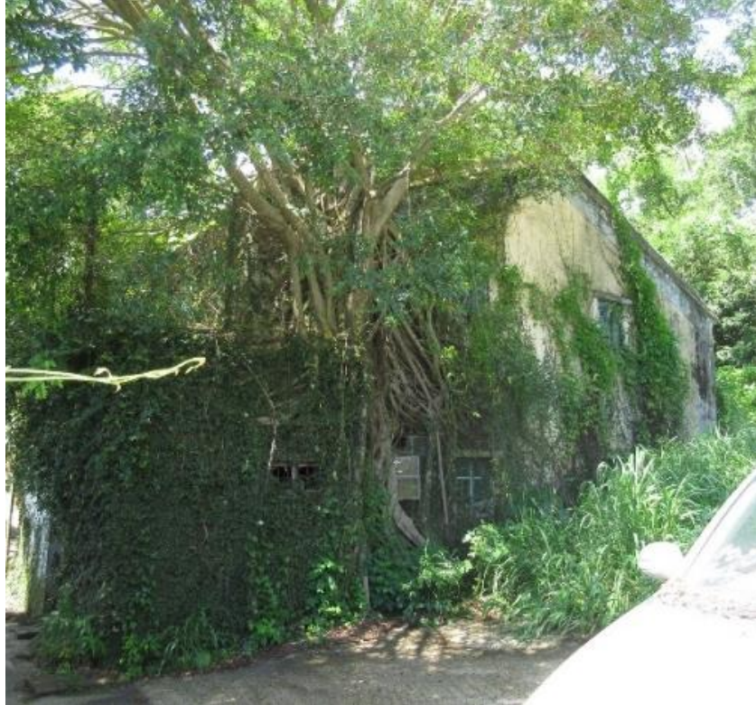
Side view, showing northeast and northwest elevations, looking south.
