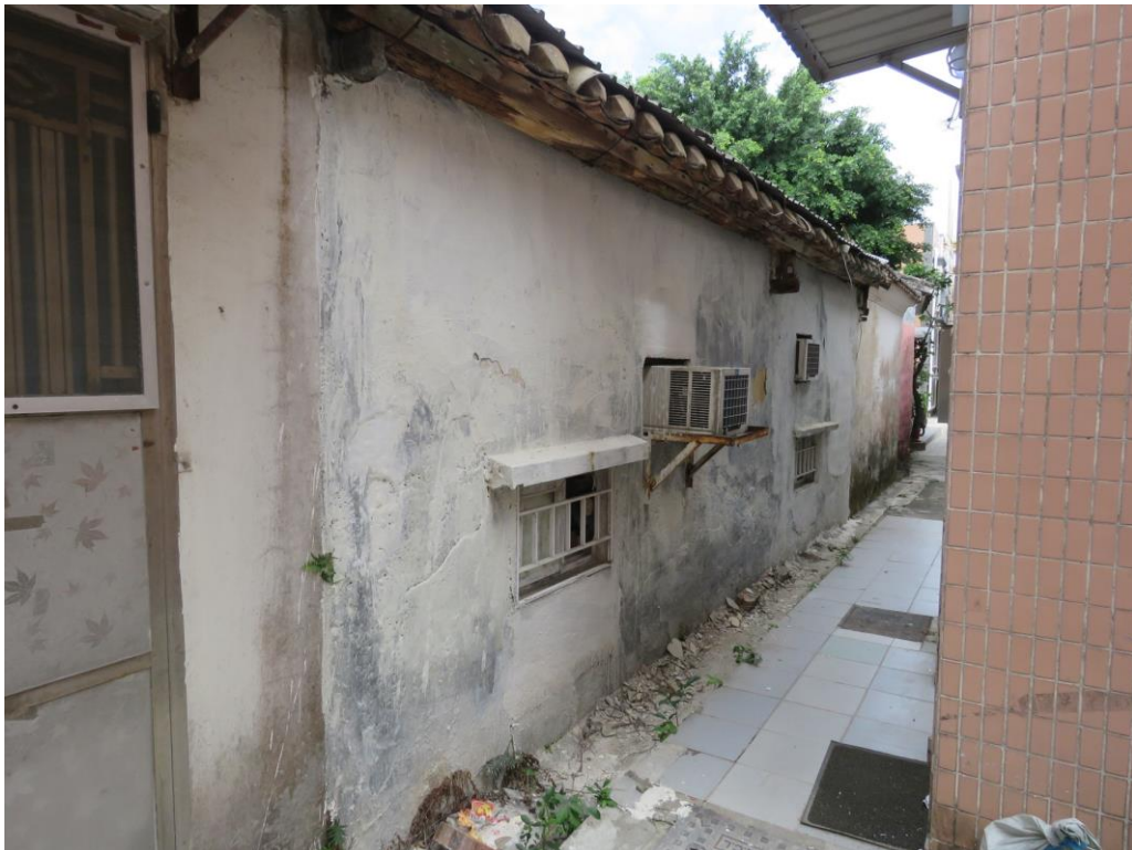
Back view of HB-49, showing southeast elevation, looking north.
