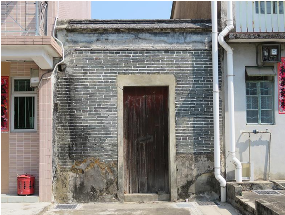
Front view of HB-02, looking northeast.
