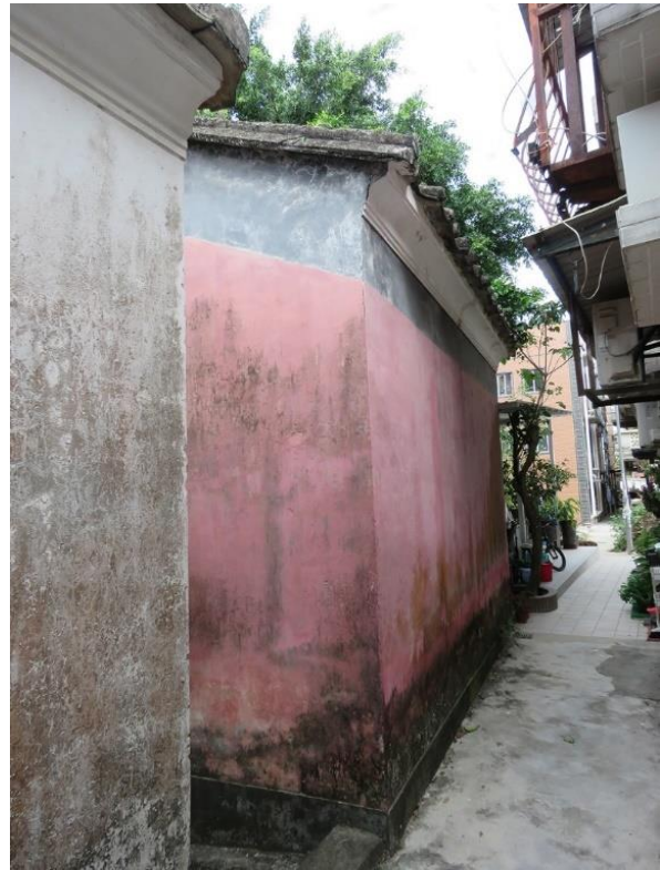
Back view GB-07, showing east elevation, looking north.
