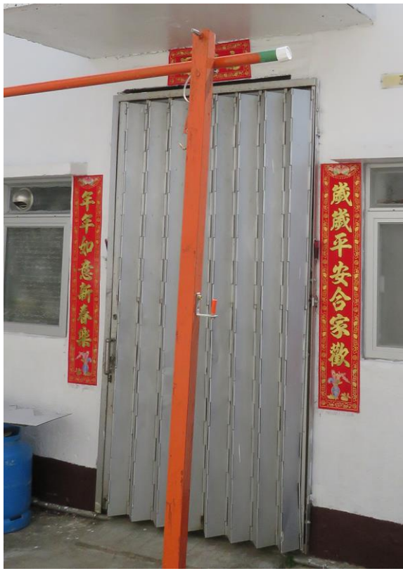
Close up of the façade (No.30)
