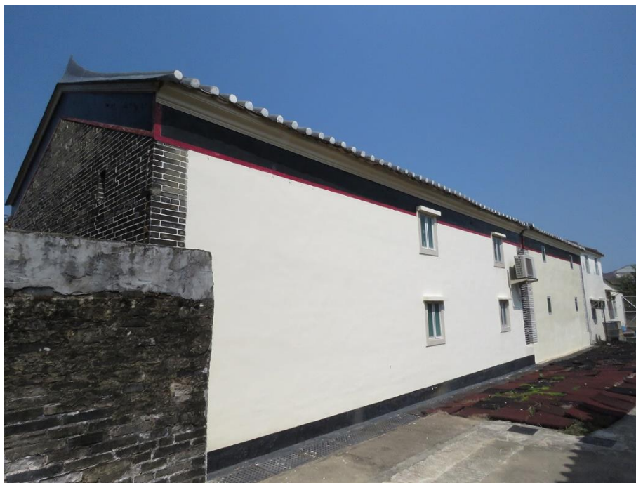
Back and side view, showing southeast and southwest elevations, looking northeast.
