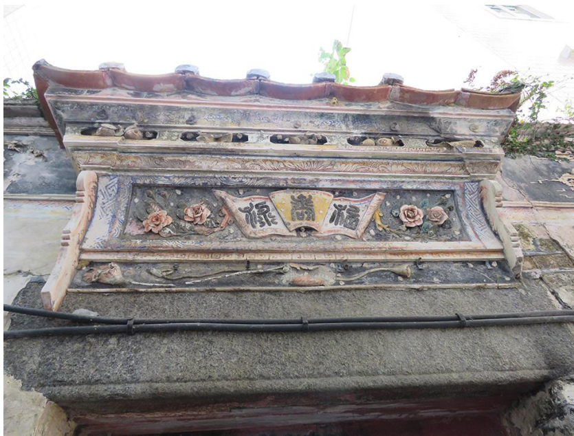
Close up of the façade
