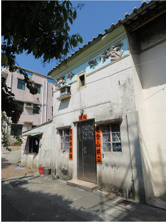
Front view of No. 8, looking northeast.
