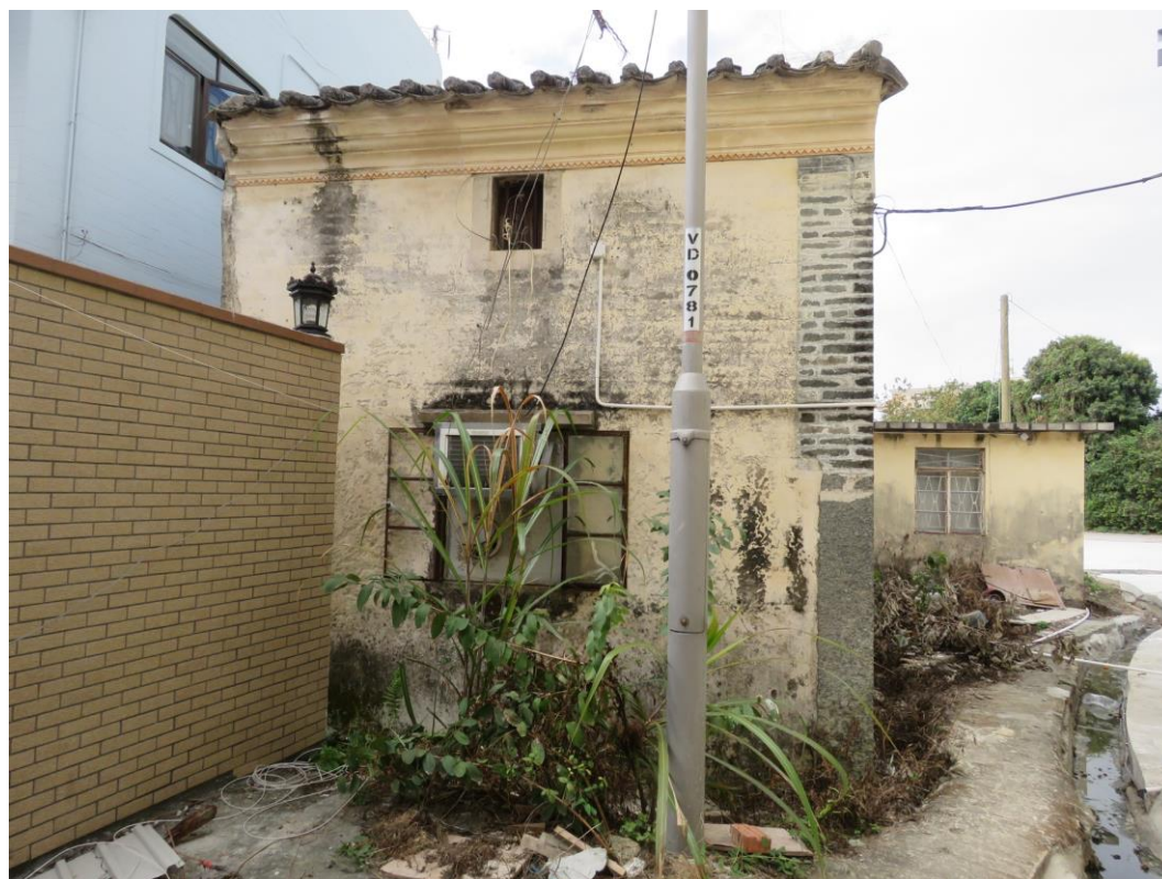
Back view of HB-44, showing northeast elevation, looking southwest.
