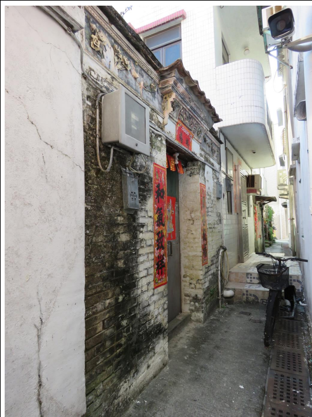
Front view of HB-36, looking southwest.
