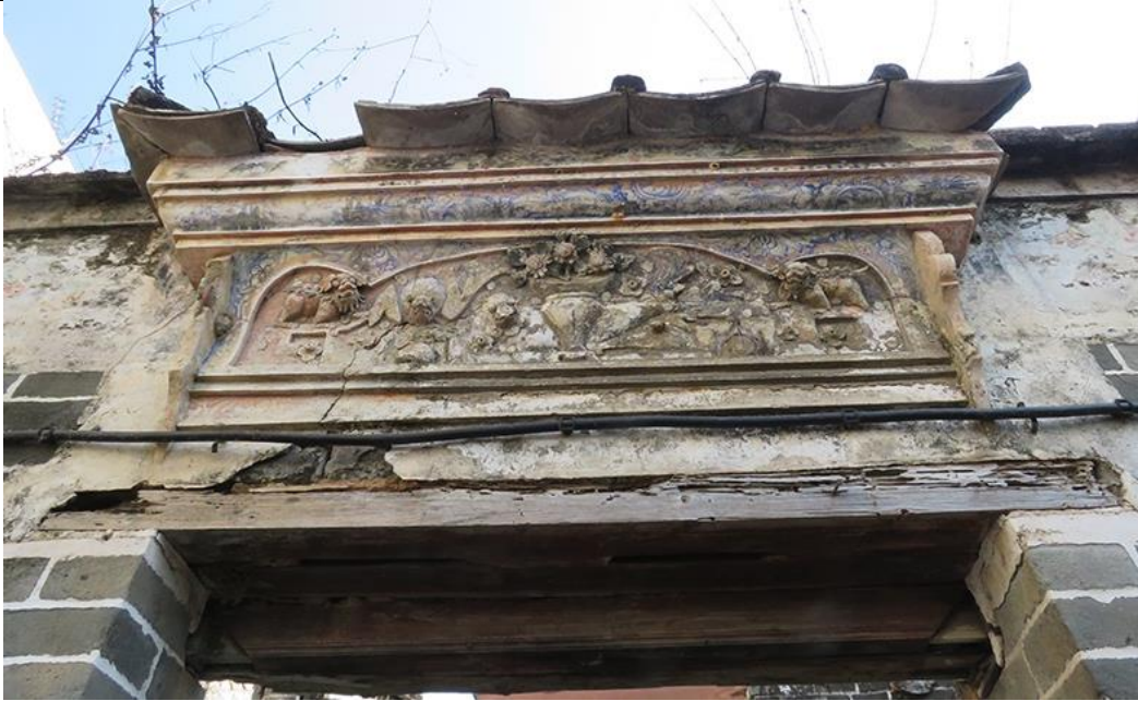
Plaster moulding on door canopy of No.12A
