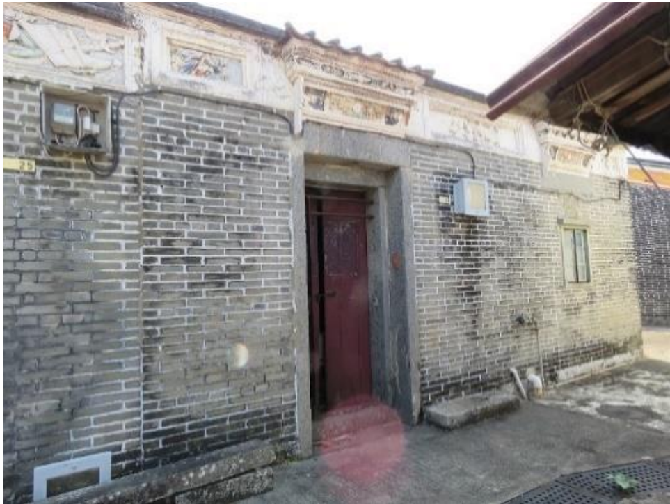
Façade of No.24, looking southwest.
