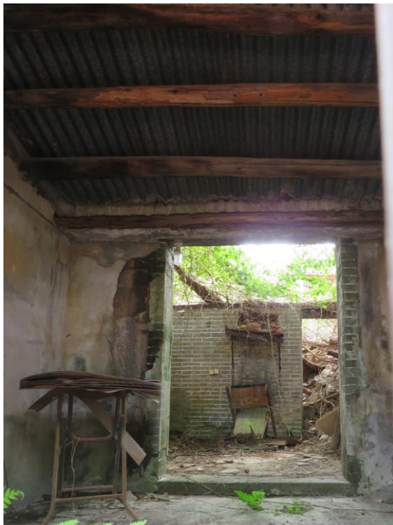
Internal view of No.95, looking east-southeast.
