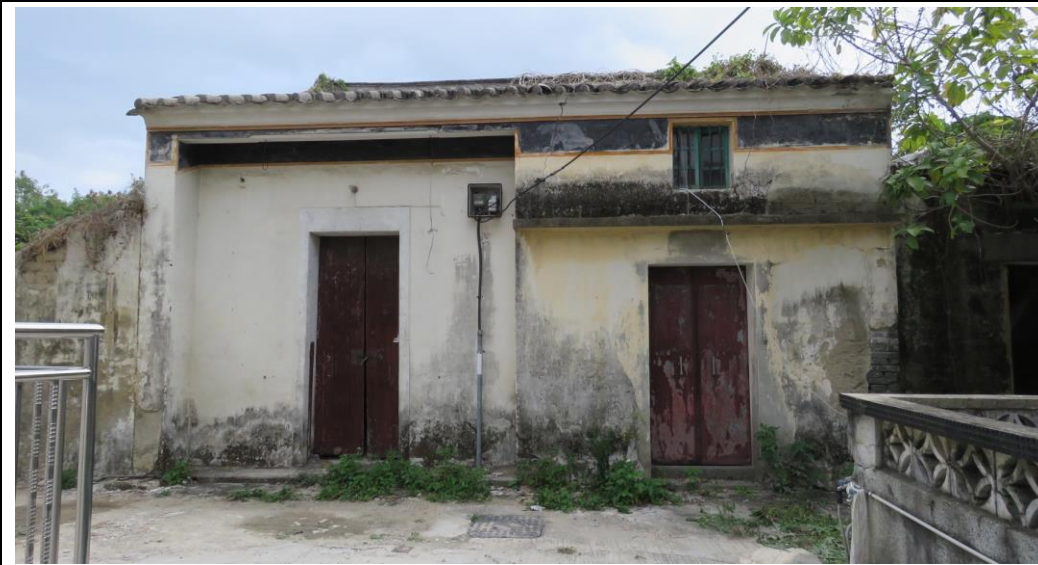
Façade view of HB-16, looking northeast.
