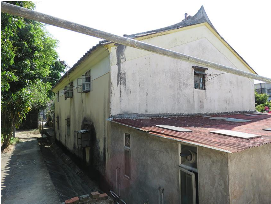
Back and side view, showing northeast and northwest elevations, looking southwest.
