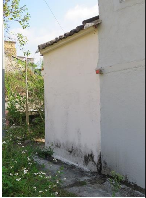
Back view of HB-08, showing northeast elevation, looking southeast.
