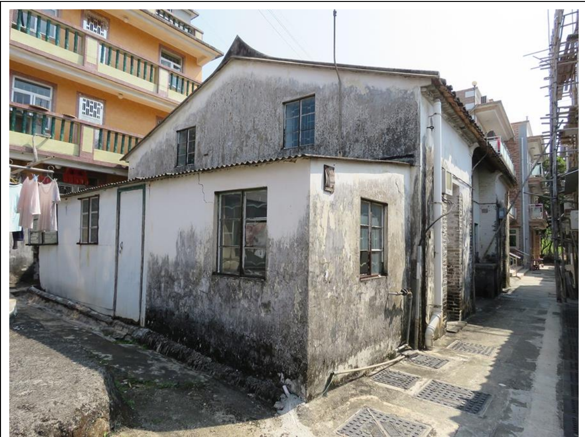
Side view of HB-06, showing northwest elevation, looking east.
