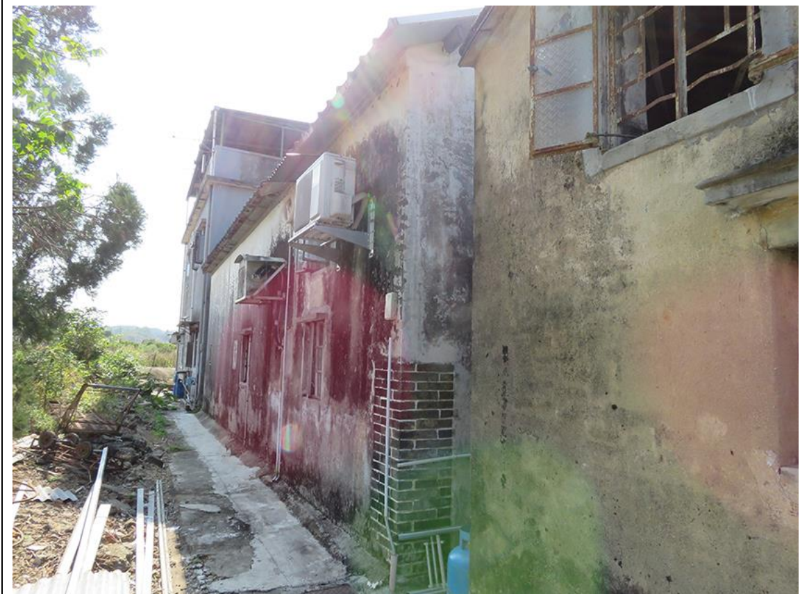
Back view of HB-37, showing southeast elevation, looking southwest.
