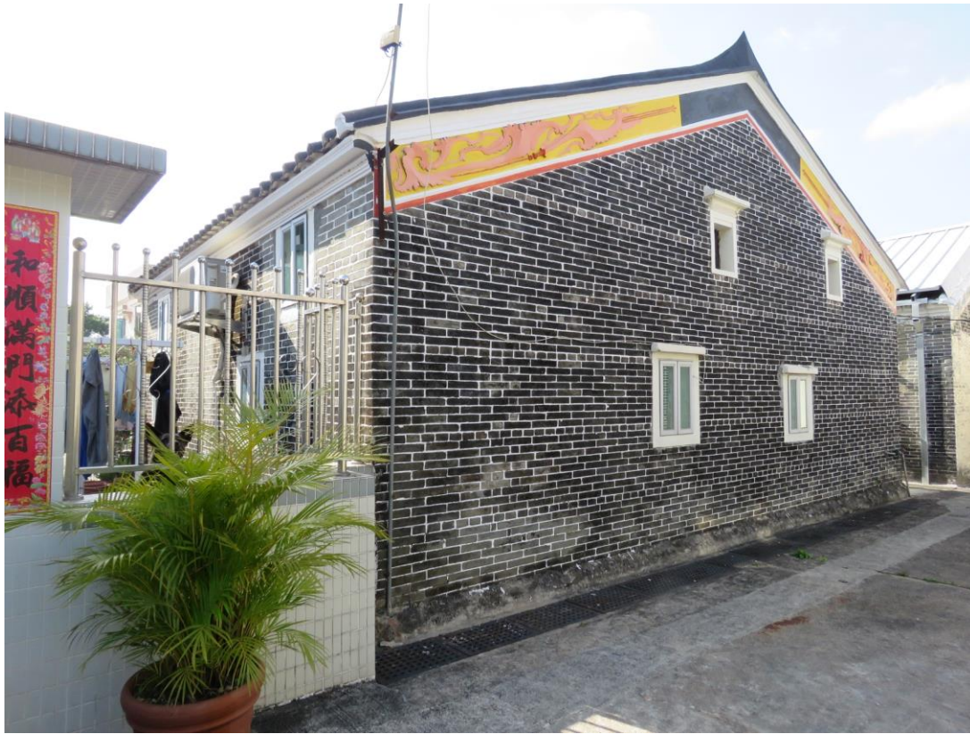
Back and side view of HB-20, showing southeast and northeast elevations, looking northwest.
