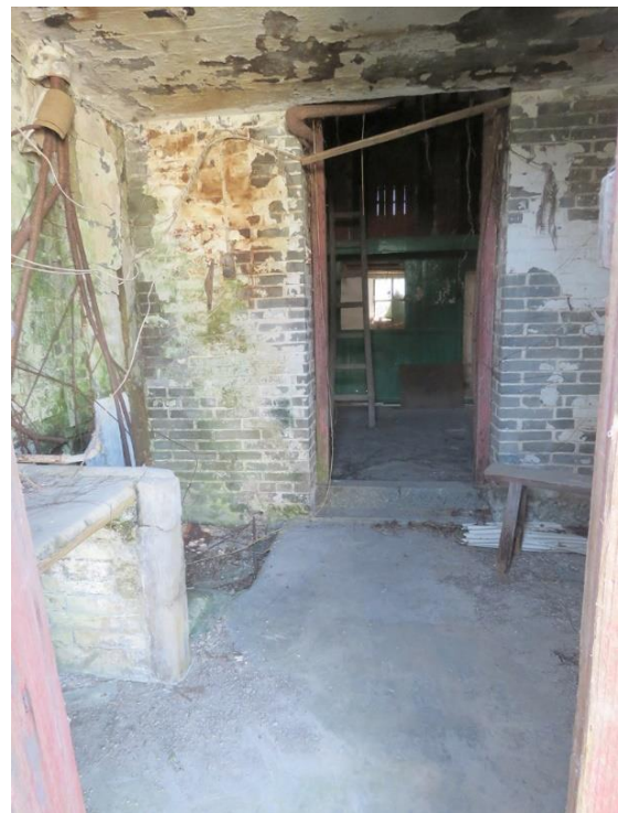
Internal view of No.27, looking southeast.
