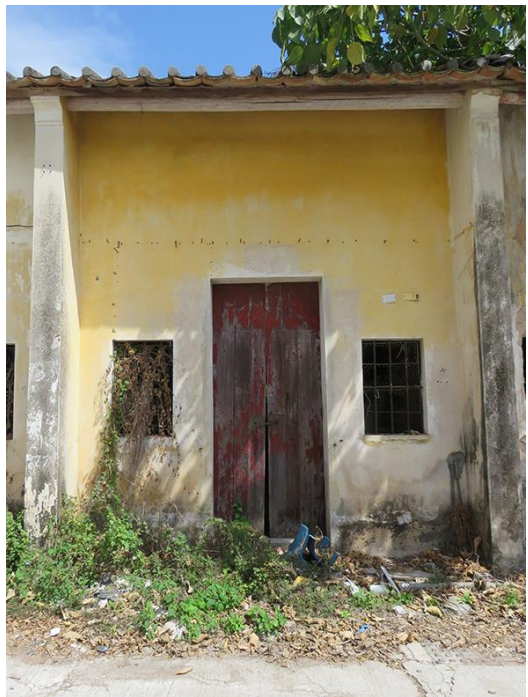
Façade view of No.134, looking northeast.
