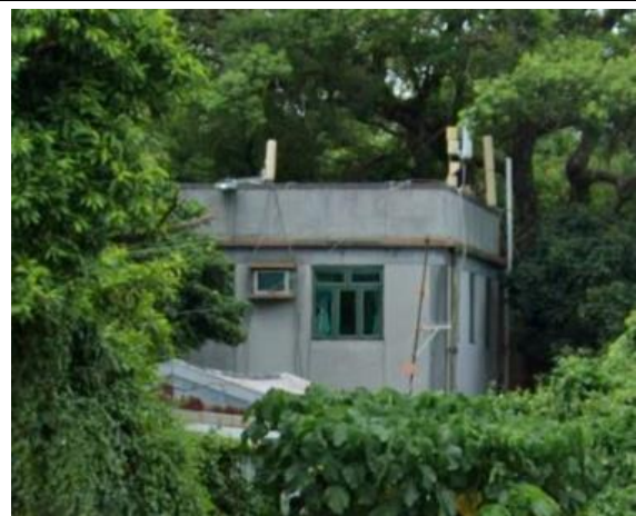
NSR 18 – Village House in Tai Po Tin
