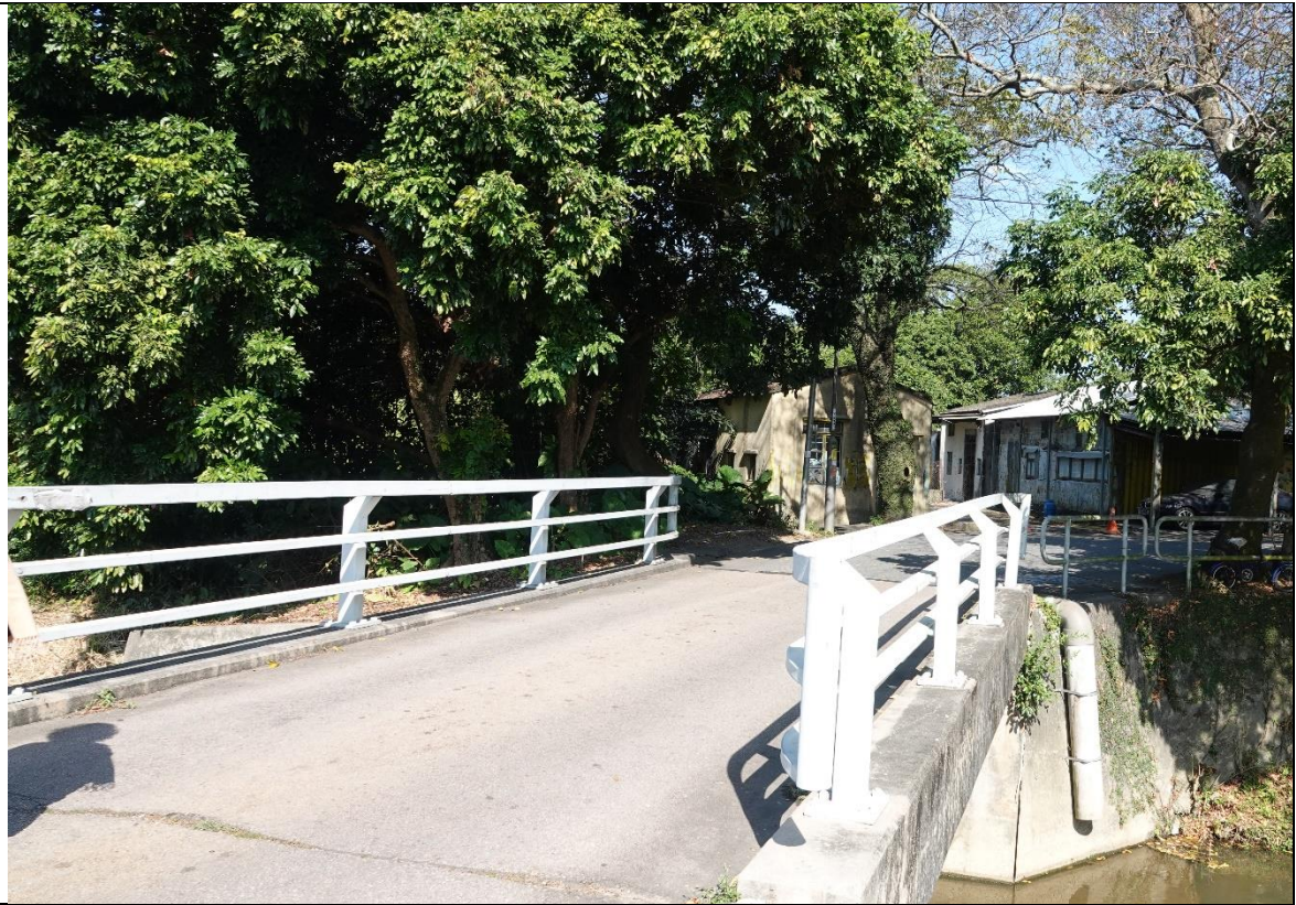
Photograph: 7 | Location of Proposed Vehicular Crossing
