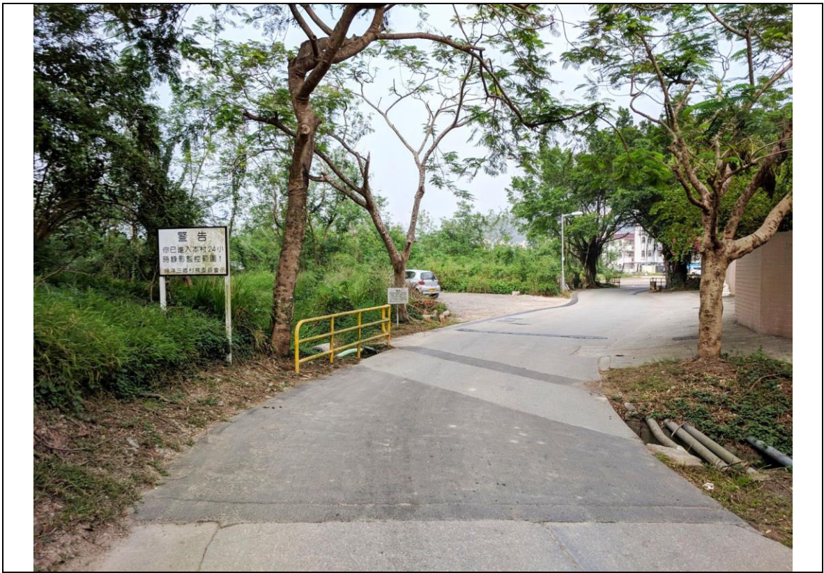
Photograph: 13 Existing vehicle road - Proposed U-channel/Rectangular Channel
