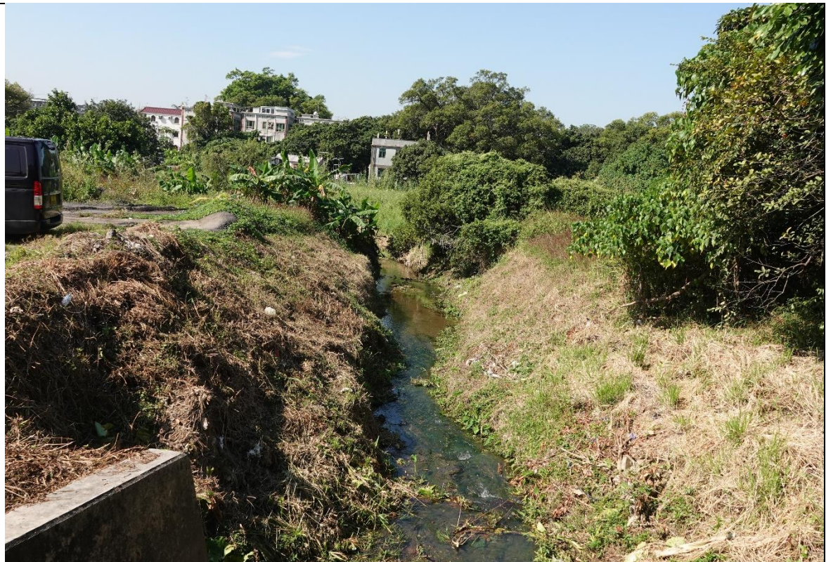
Photograph: 8 | View of the existing nullah
