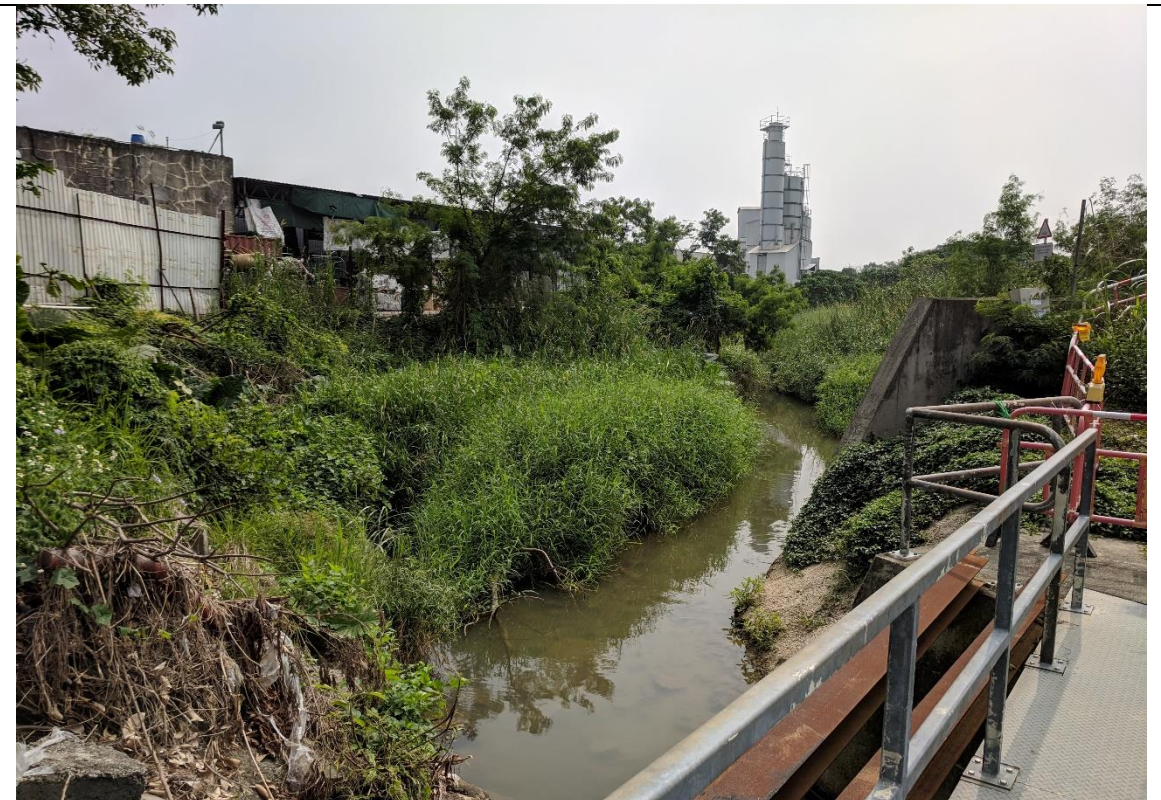
Photograph: 10 | Location of Proposed Footway Crossing
