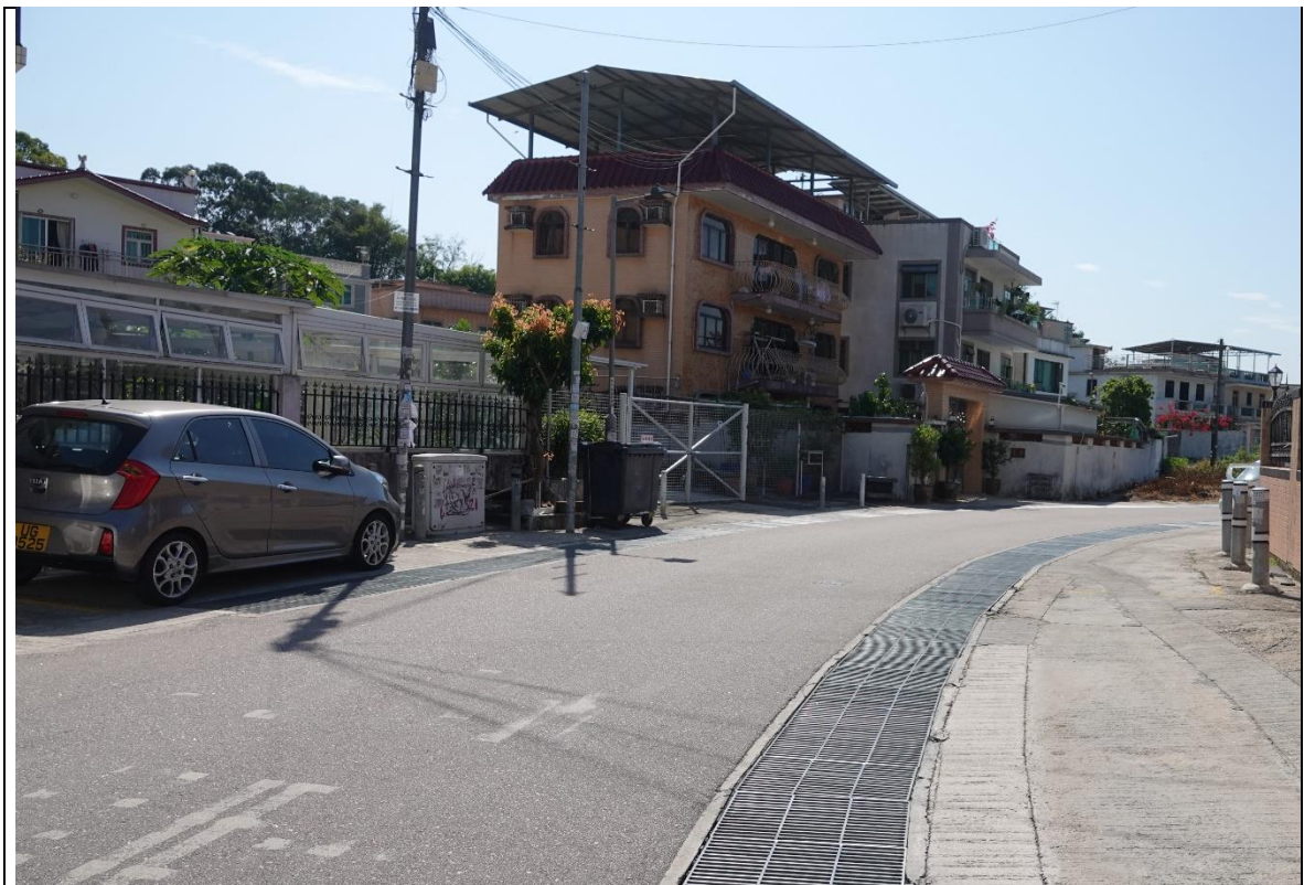
Photograph: 14 Existing vehicle road - Proposed U-channel/Rectangular Channel
