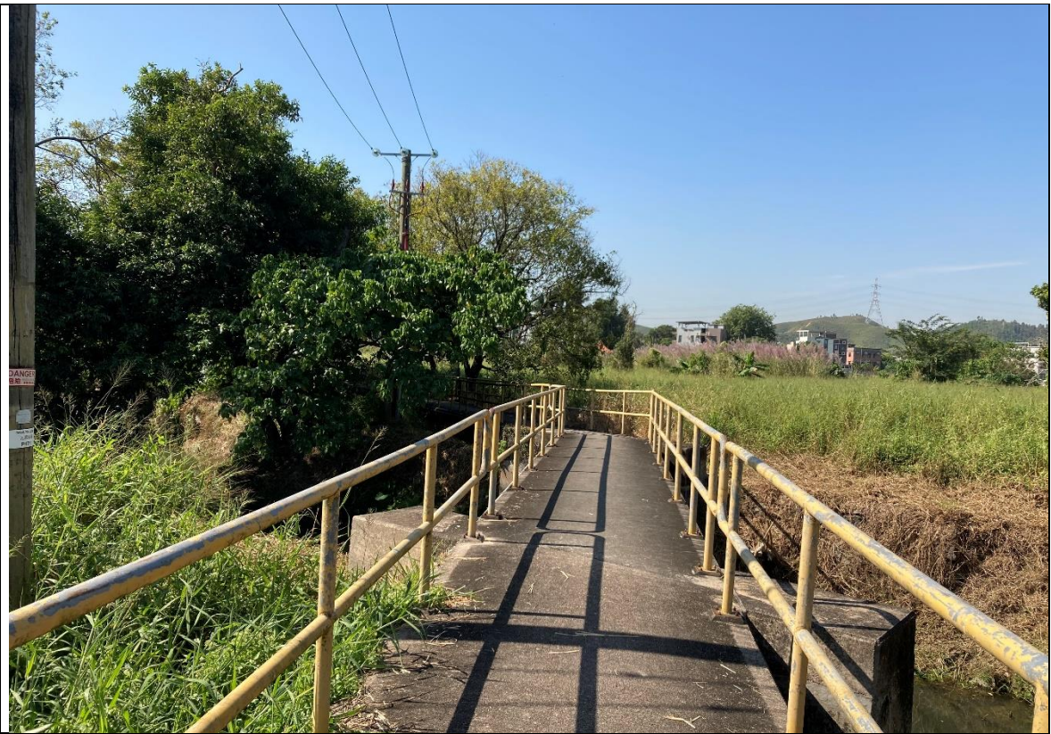
Photograph: 11 | Location of Proposed Footway Crossing
