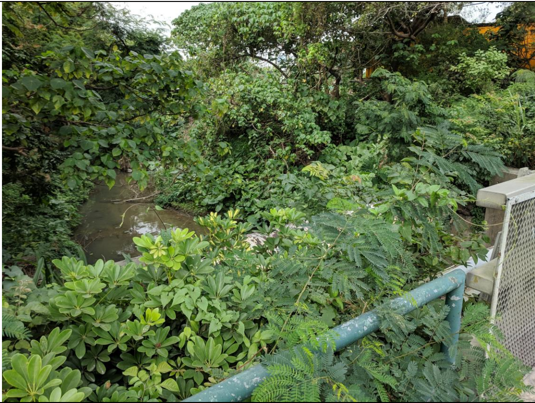
Photograph: 5 | View of the existing nullah
