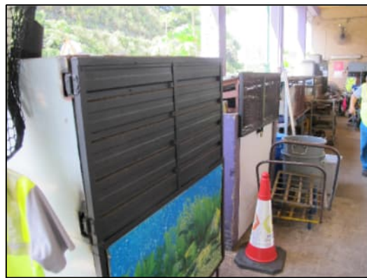
PHOTO 9713: CHEMICAL WASTE STORAGE AREA IN VEHICLE MAINTENANCE WORKSHOP IN ADMINISTRATION BUILDING (DATE TAKEN: 25 AUGUST 2020)
