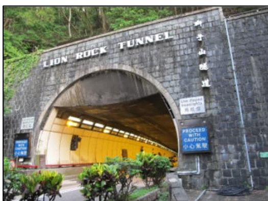
PHOTO 9846: LION ROCK TUNNEL (DATE TAKEN: 25 AUGUST 2020)
