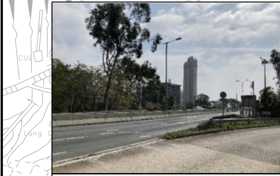
PHOTO 3047: LION ROCK TUNNEL ROAD NEAR LAMP POST BF1962 (DATE TAKEN: 12 FEBRUARY 2022)
