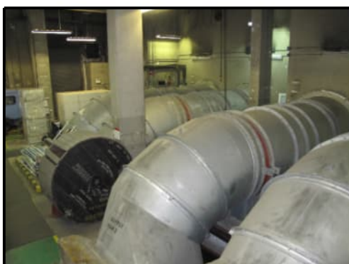
PHOTO 9876: VENTILATION BUILDING K2 (DATE TAKEN: 25 AUGUST 2020)
