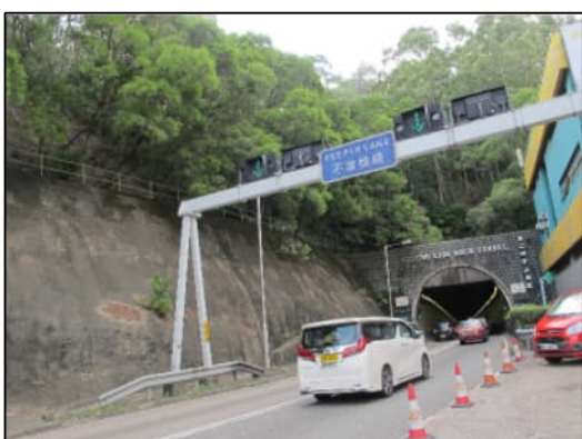
PHOTO 9893: SECOND LION ROCK TUNNEL (DATE TAKEN: 25 AUGUST 2020)
