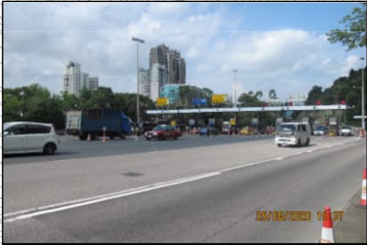
PHOTO 4370: LION ROCK TUNNEL TOLL PLAZA (DATE TAKEN: 25 AUGUST 2020)
