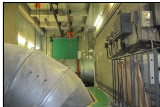
PHOTO 9836: VENTILATION BUILDING S1 (DATE TAKEN: 25 AUGUST 2020)
