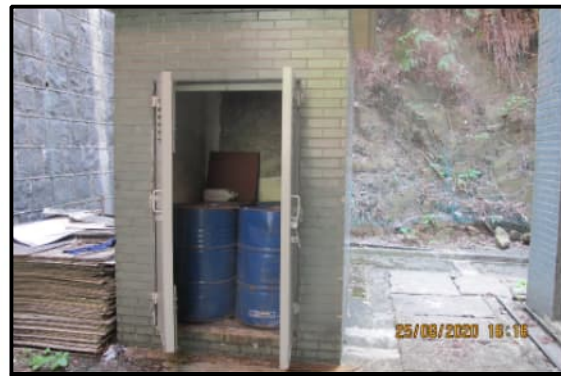
PHOTO 4430: CHEMICAL WASTE STORAGE AREA OF VENTILATION BUILDING S1 (DATE TAKEN: 25 AUGUST 2020)
