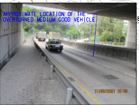
PHOTO 7761: LUNG CHEUNG ROAD UNDERNEATH EXISTING VEHICULAR BRIDGE (DATE TAKEN: 11 JUNE 2021)
