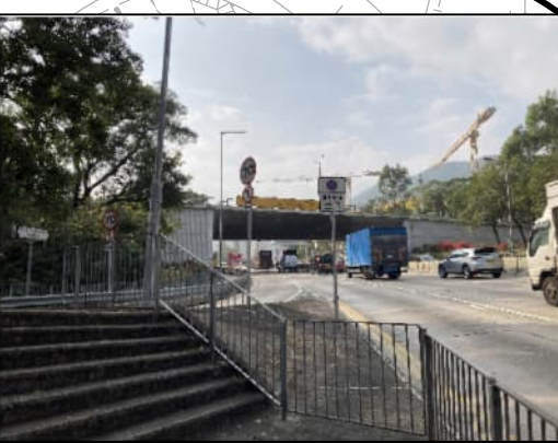
PHOTO 2486: LUNG CHEUNG ROAD AND EXISTING VEHICULAR BRIDGE (DATE TAKEN: 7 JANUARY 2022)
