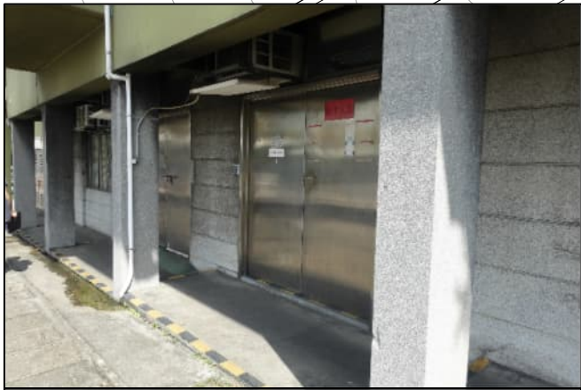
PHOTO 2643: E&M BUILDING (DATE TAKEN: 25 AUGUST 2020)
