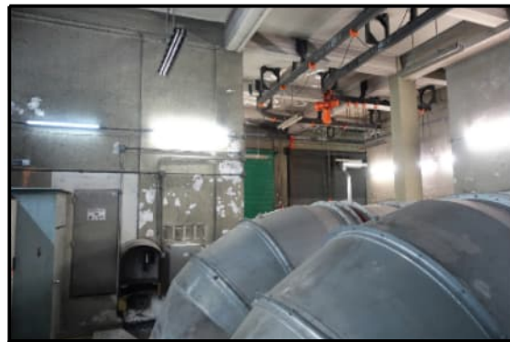
PHOTO 2784: VENTILATION BUILDING S1 (DATE TAKEN: 25 AUGUST 2020)
