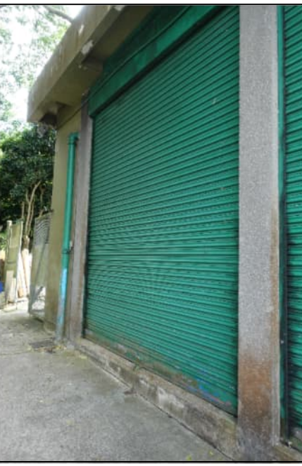
PHOTO 2726: E&M BUILDING (DATE TAKEN: 25 AUGUST 2020)
