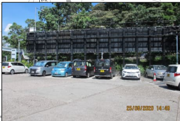
PHOTO 4351: CAR PARK OF ADMINISTRATION BUILDING (DATE TAKEN: 25 AUGUST 2020)
