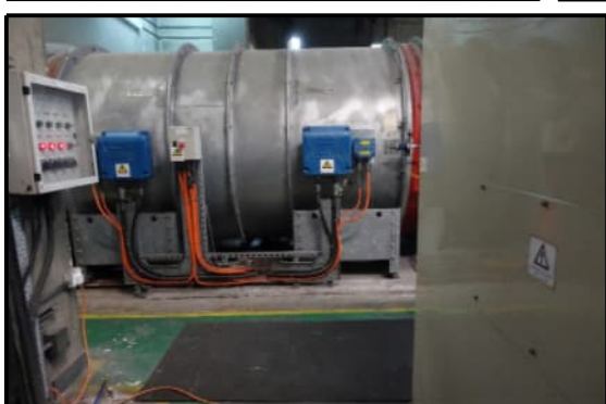
PHOTO 2836: VENTILATION BUILDING K2 (DATE TAKEN: 25 AUGUST 2020)
