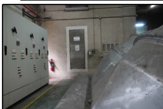
PHOTO 2865: VENTILATION BUILDING K1 (DATE TAKEN: 25 AUGUST 2020)
