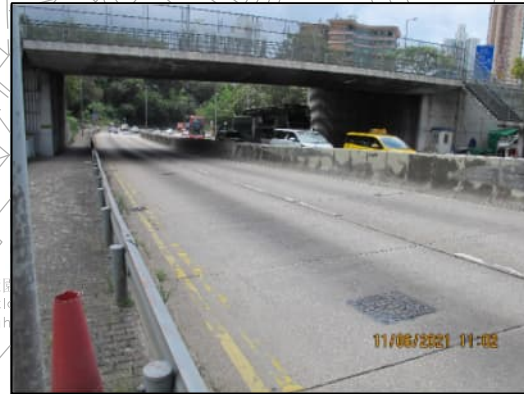
PHOTO 7797: LUNG CHEUNG ROAD AND EXISTING VEHICULAR BRIDGE (DATE TAKEN: 11 JUNE 2021)
