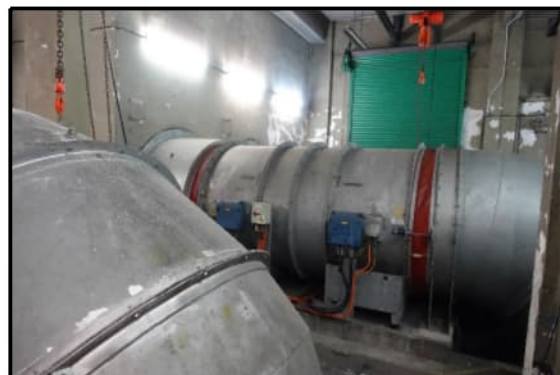
PHOTO 2772: VENTILATION BUILDING S1 (DATE TAKEN: 25 AUGUST 2020)
