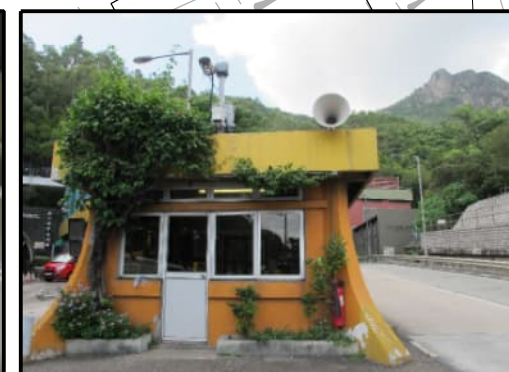
PHOTO 9852: CONTROL ROOM (DATE TAKEN: 25 AUGUST 2020)
