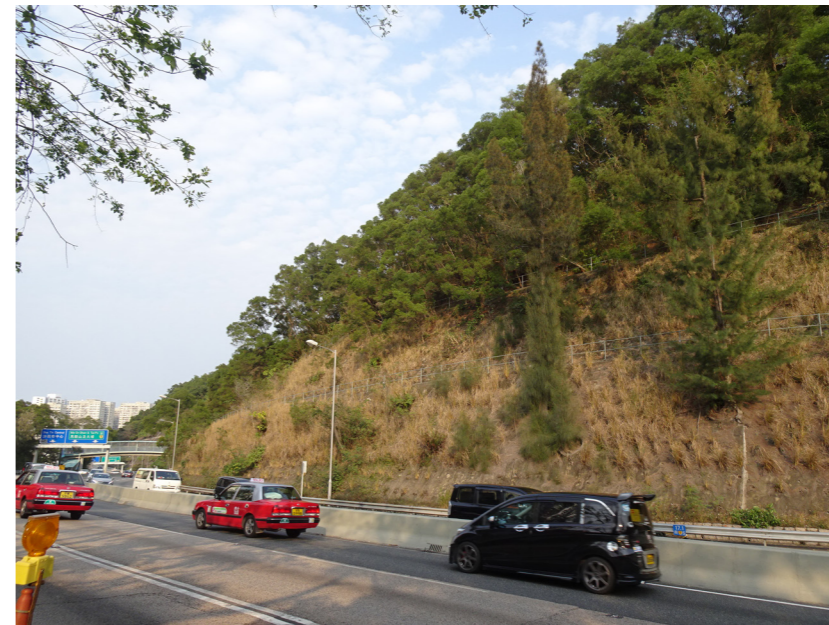
LR-3.2 VEGETATION ON ROADSIDE ENGINEERED SLOPES FROM TAI WAI TO SHA TIN TAU
