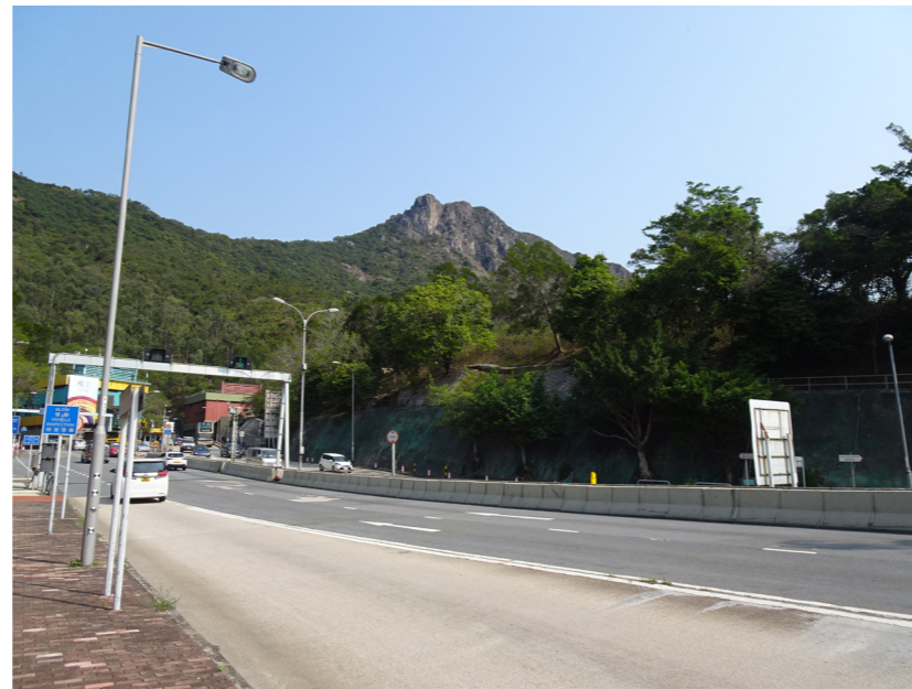
LR-3.1 VEGETATION ON ROADSIDE ENGINEERED SLOPES IN KOWLOON TONG
