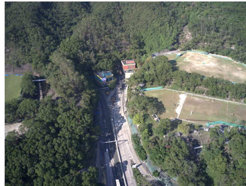
LR-6.1 VEGETATED AREAS IN SERVICE RESERVOIRS AND ASSOCIATED LANDSCAPE AREAS IN KOWLOON SIDE
