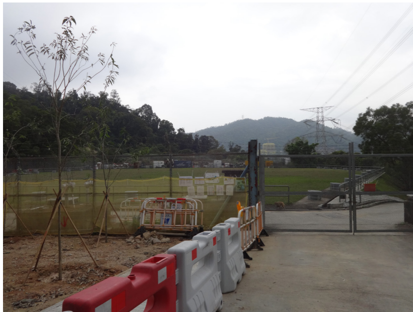
LR-6.2 VEGETATED AREAS IN SHATIN SOUTH FRESH WATER SERVICE RESERVOIR AND ASSOCIATED LANDSCAPE AREAS
