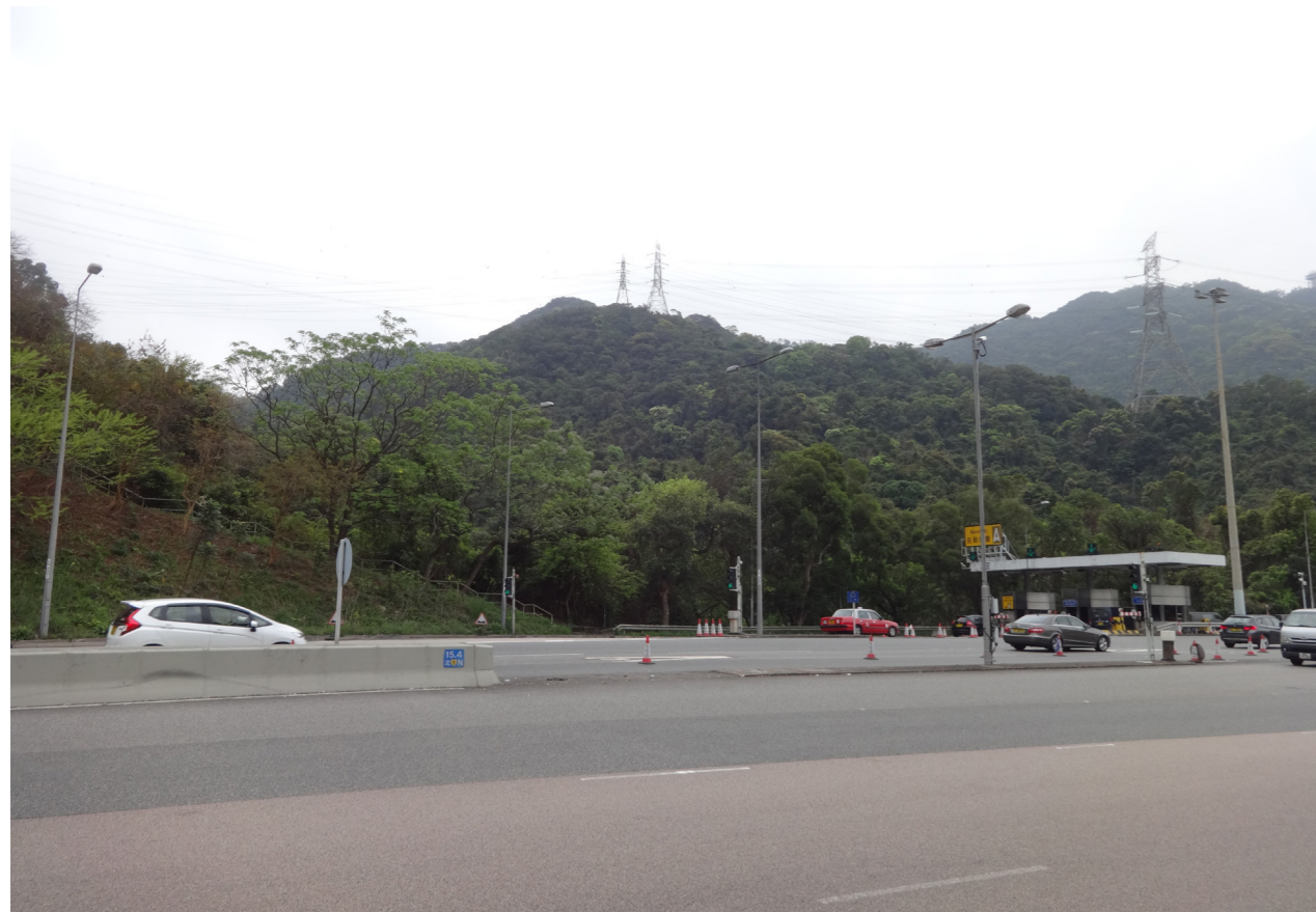
VP3 TOLL PLAZA VIEW OF TAI WAI SIDE
