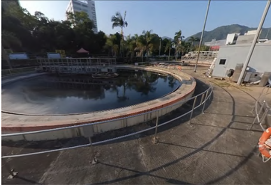
Photo WP-39: Primary Sedimentation Tanks of West Plant - The tanks are located on concrete paved floor in good condition with no oil stain/stressed vegetation observed.
