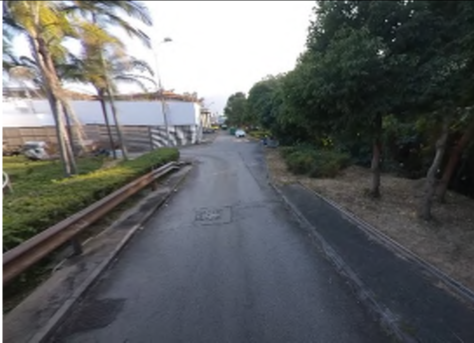
Photo WP-41: Road next to Primary Sedimentation Tanks of West Plant - The road is paved with concrete in good condition with no oil stain observed.
