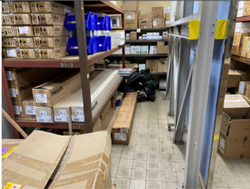
Photo WP-18: Control and Storage House (Storage Room on First Floor) - Most of the equipment are stored on steel racks, some are being put on the floor inside cardboard box. The floor is paved with ceramic tile and concrete. No damage/ broken parts is observed, and no oil stain/leakage is observed.
