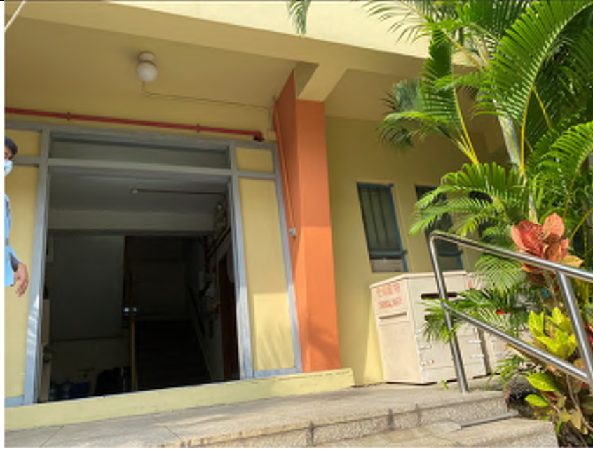
Photo WP-1: Old Administration Building (External View) – It is a two-storey building located on concrete paved floor in good condition. No oil stain/ leakage is observed.
