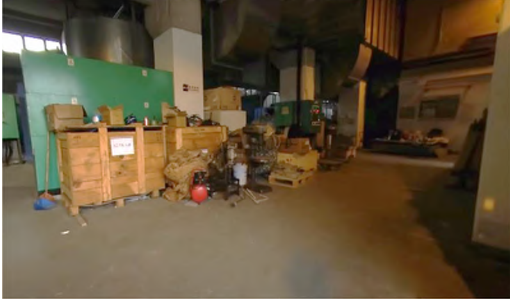
Photo EP-28: Central Building Complex – The first floor of the Central Building Complex is paved with concrete and some equipment were stored here inside the wooden box/on the wooden panel. Some other equipment are placed on the floor. No oil stain/leakage is observed.
