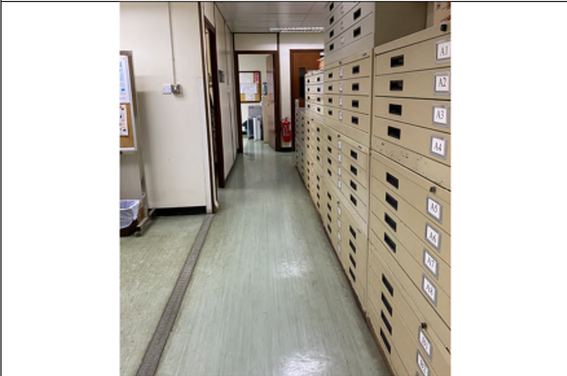
Photo WP-14: Administrative Building (First Floor) - The floor is paved with flooring plate and concrete in good condition floor. This floor is mainly used for office and administration works.No oil stain/ spillage is observed.
