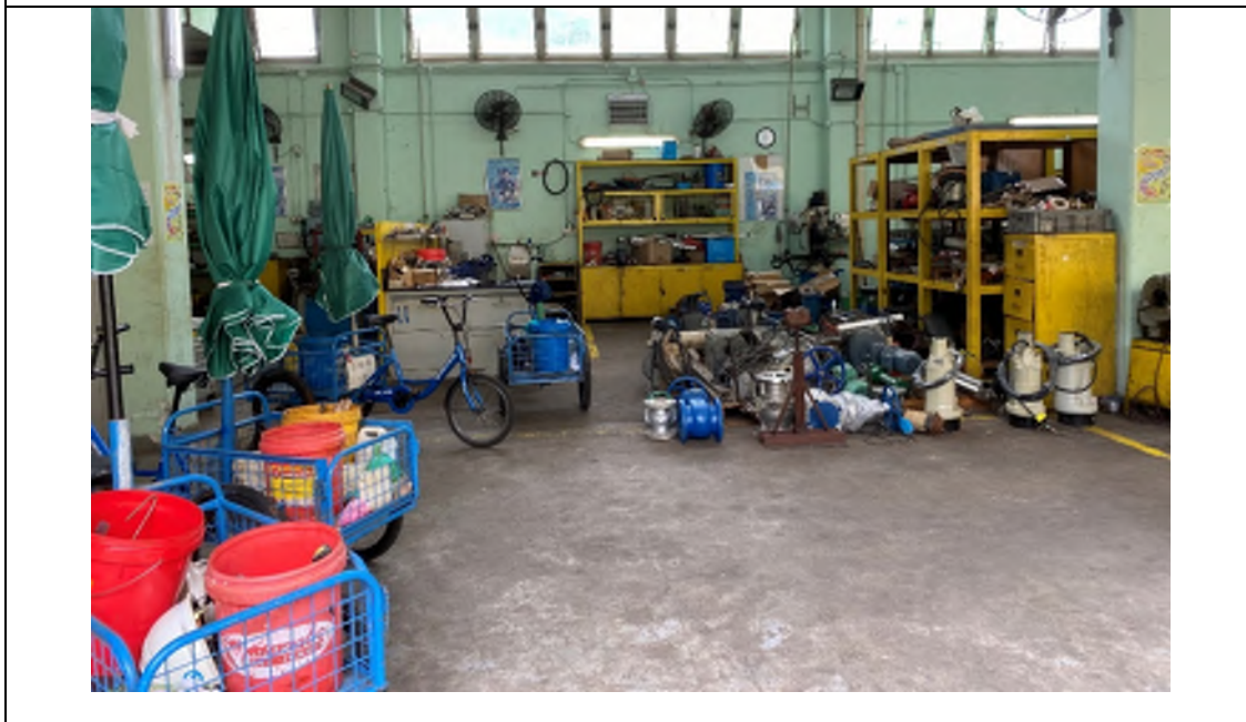
Photo WP-10: Maintenance Building – The floor is paved with concrete, small tools and equipment are placed on racks. Some other equipment was placed on the floor, there are some bicycle carrying cleaning tools parked here. No oil stain / leakage is observed.
