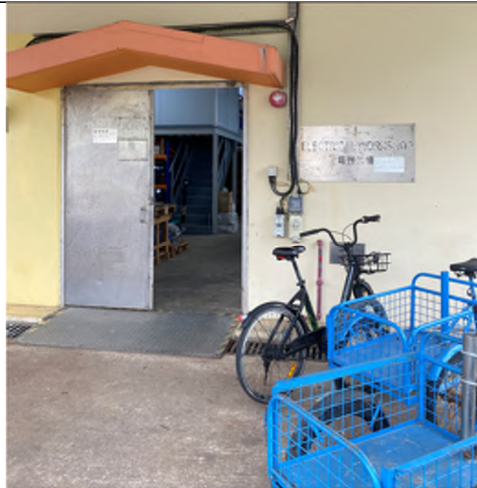
Photo WP-4: Electrical Workshop (External View) – No oil stain / floor leakage observed.
