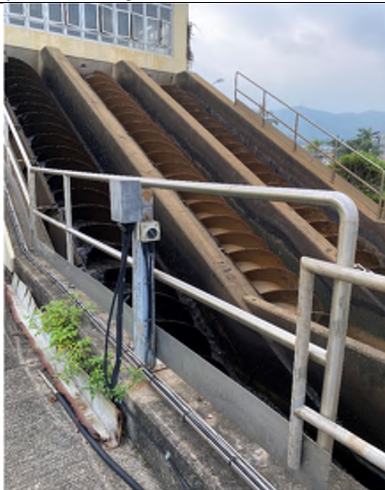
Photo EP-18: Inlet Pumping Station of East Plant (External View of Screw Pumps) – The pumps are located on concrete paved floor at 3.4 m above the ground level. All accessible surfaces around the pumps are paved with concrete, steel panels are installed to prevent spillage. No observation of oil stain/ leakage is anticipated.
