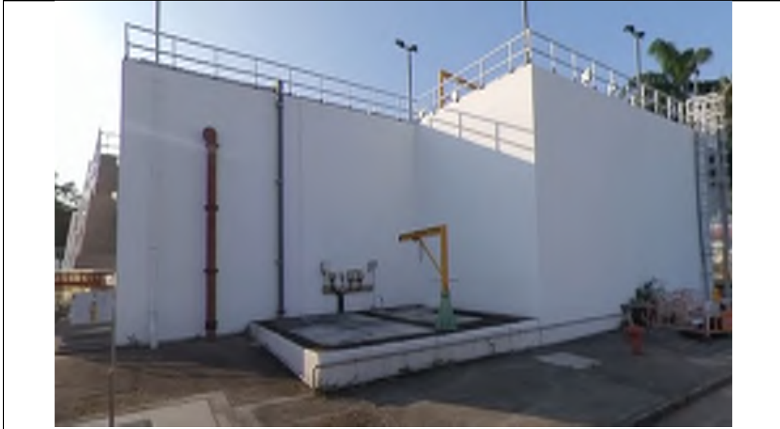
Photo WPS-13: Filtrate Treatment Units – The Filtrate Treatment Units is constructed with concrete located on concrete paved ground in good condition with no oil stains / stressed vegetation or potentially contaminating activities observed in the area.
