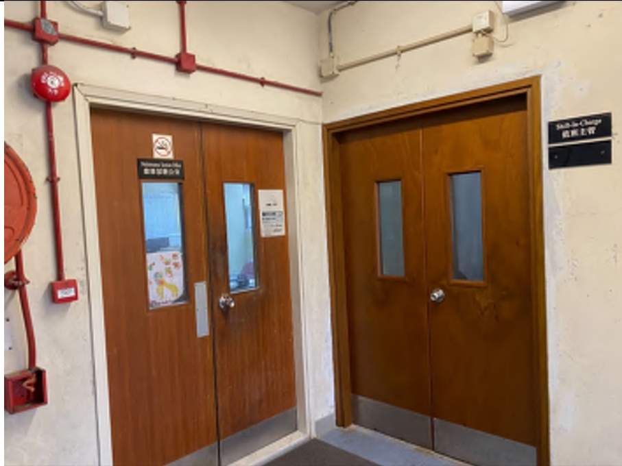
Photo WP-3: Old Administration Building – The second floor of the Old Administration Building is paved with concrete slab, the Maintenance Section Office is located on the second floor.
