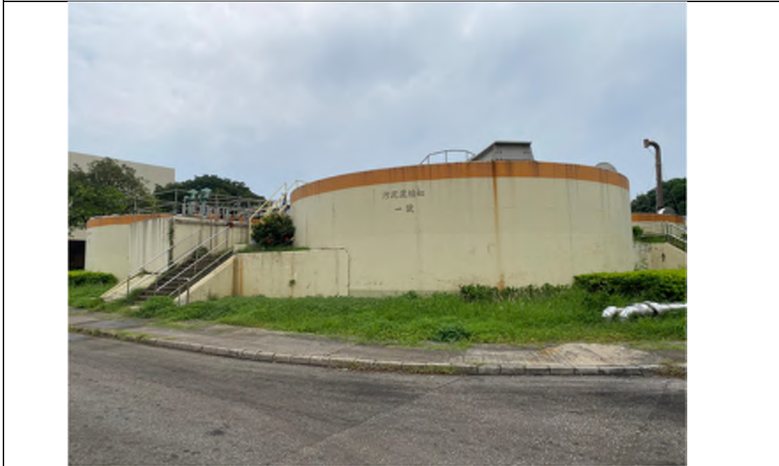
Photo WPS-14: Primary Sludge Gravity Thickeners of West Plant– The thickeners are located on concrete paved floor with vegetation surrounding in good condition. No oil stain is observed.
