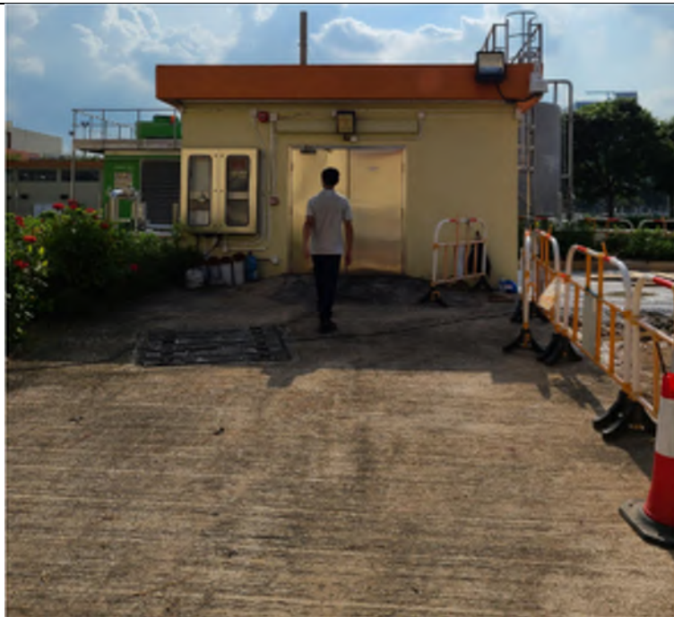
Photo EP-41: Chemical Store – The chemical store is located on concrete paved floor. No oil stain/ leakage is observed.
