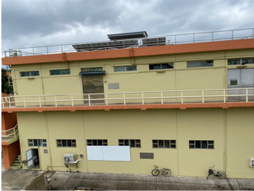
Photo WP-17: Control and Storage House (External View) – It is a two-storey building with the storage room of equipment on the ground floor and the control room on the second floor. The building is located on concrete paved floor, water stain was observed, no oil stain/leakage is observed.
