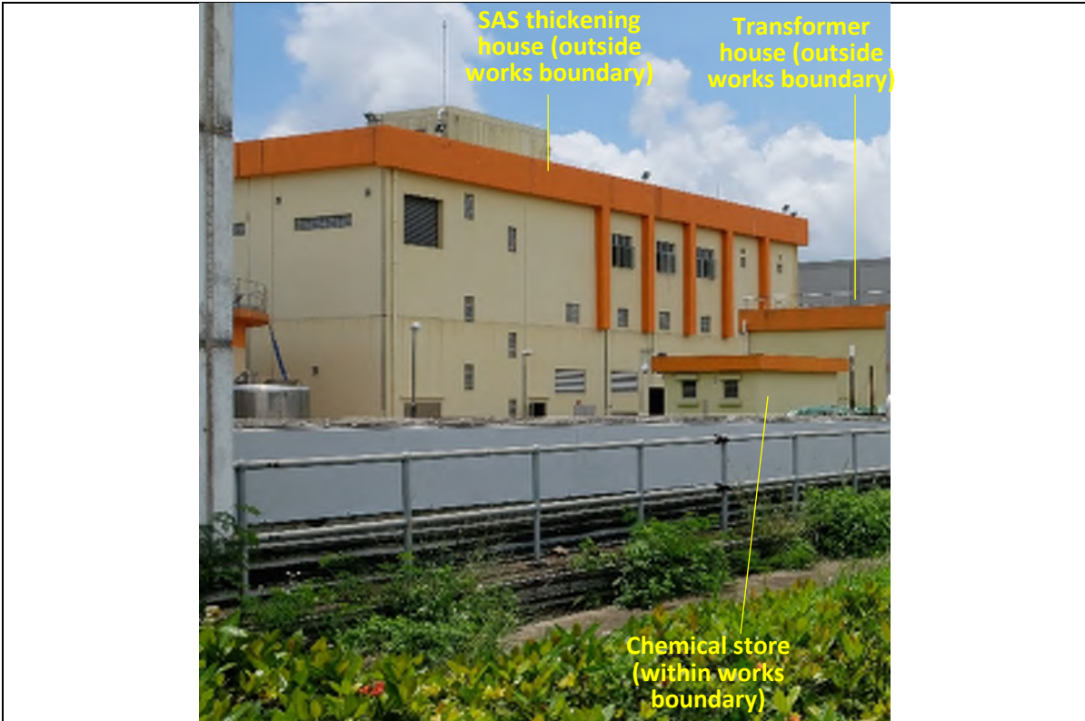
Photo V1: TPSTW facilities outside the proposed excavation works limit, including the SAS Thickening House and Transformer House, are enclosed within concrete building.
