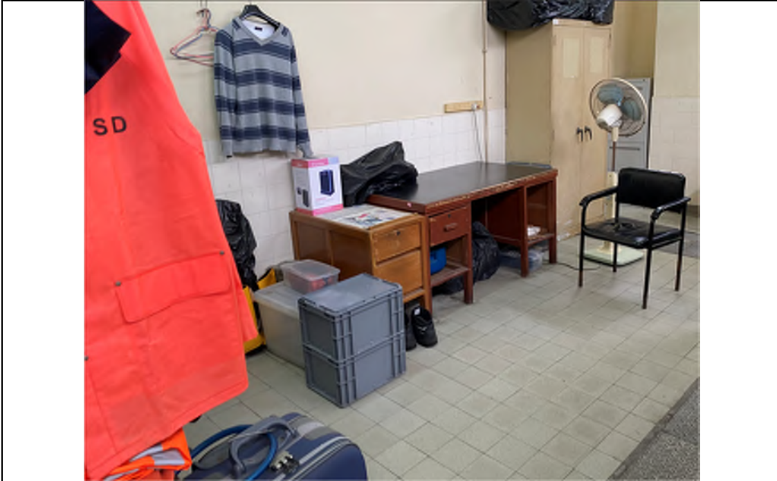
Photo WP-21: Control and Storage House (Staff Room on Second Floor) – It is next to the Control Room. The floor is paved with ceramic tile and concrete in good condition. No oil stain/leakage is observed.
