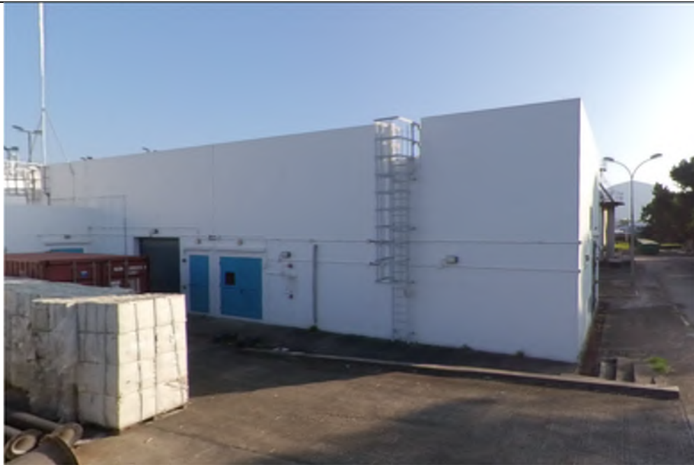
Photo WPS-12: Filtrate Treatment Complex – It is located on concrete paved panel in good condition, no oil stain is observed.
