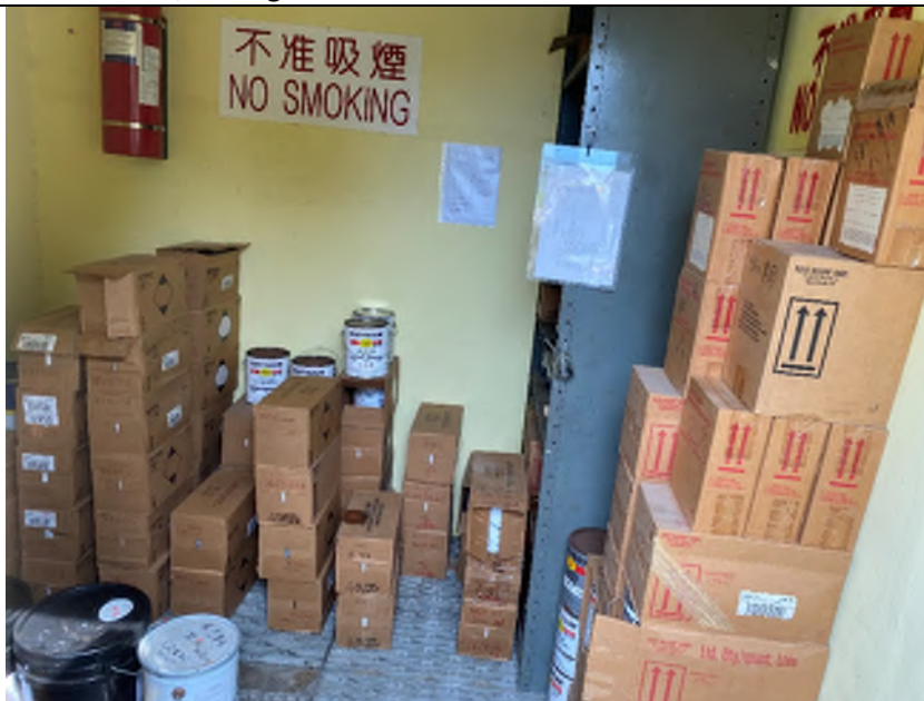
Photo WP-24: Dangerous Goods (DG) Store – Paint were stored inside the DG Store. Some paint were placed on the steel panel inside the container and the cardboard box; Some were stored inside the steel rack. No oil stain/leakage is observed.
