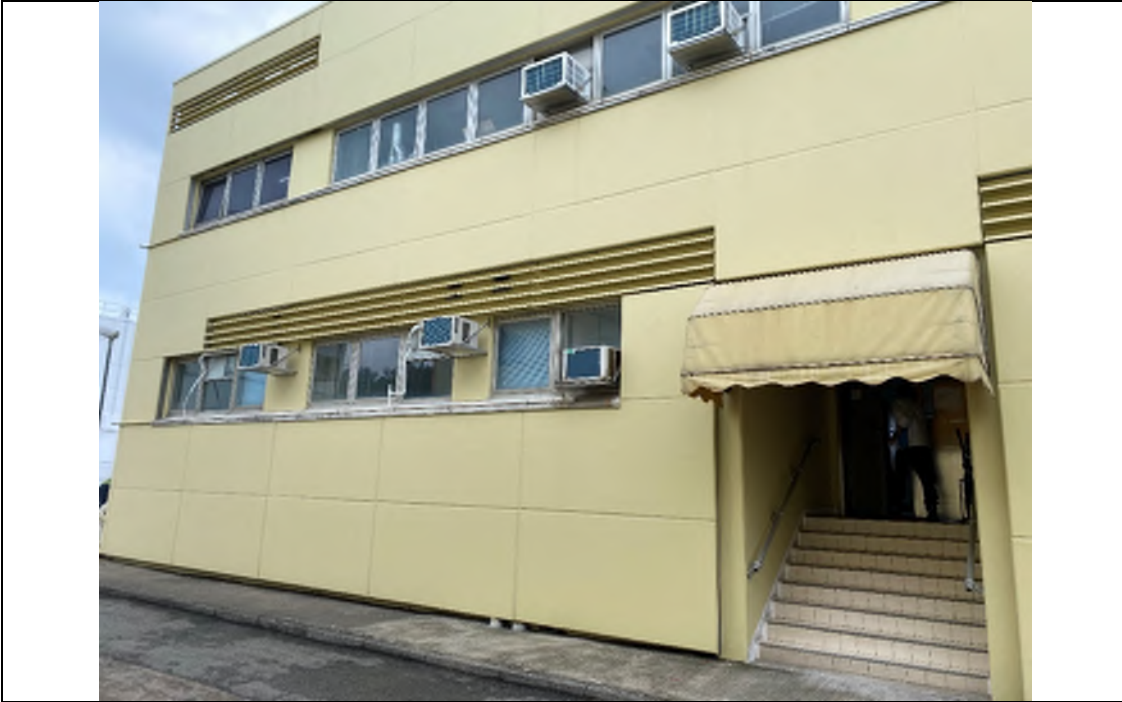
Photo WP-13: Administrative Building (External view) - The building is a two-storey building located on concrete paved floor in good condition. No oil stain/leakage is observed.
