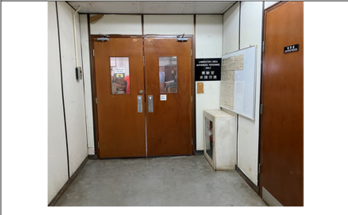
Photo WP-16: Administrative Building (Second Floor) - The Laboratory is located on this floor next to the Switch Room on concrete paved floor in good condition
