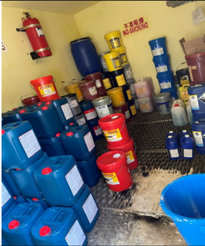
Photo WP-23: Dangerous Goods (DG) Store – The soluble cutting oil, hydraulic oil, lubricant oil, gear oil were stored inside the DG store. DG were located on steel panel and concrete paved floor. No oil stain/ leakage is observed.
