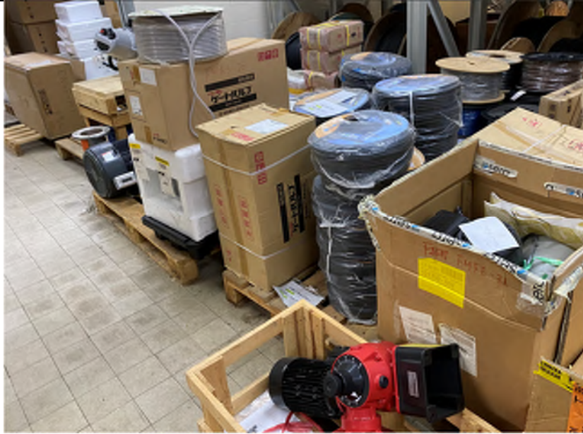
Photo WP-19: Control and Storage House (Storage Room on First Floor) - Equipment (electronic wire) was being put on wooden panel or wooden box. The floor is paved with ceramic tile and concrete in good condition. No oil stain/leakage is observed.
