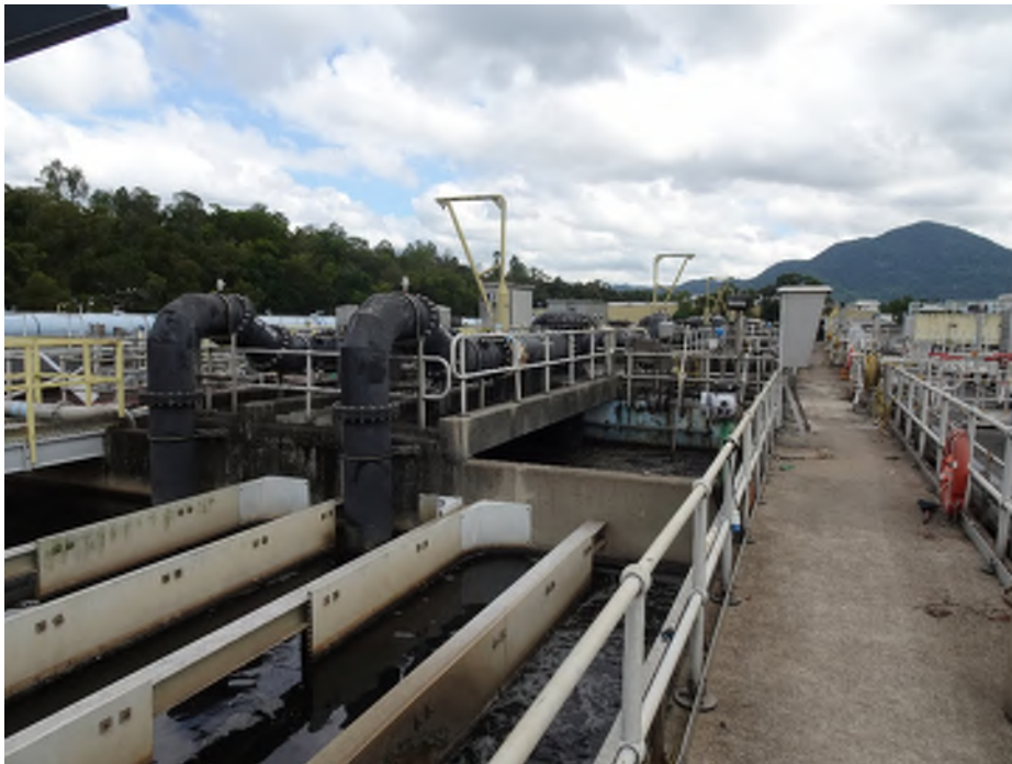
Photo V9: Aeration Tanks of East Plant – The tanks are constructed with concrete, and located below ground level. The assessable road is paved with concrete. Water stain caused by handling of sludge is observed, no oil stain/ spillage observed.
