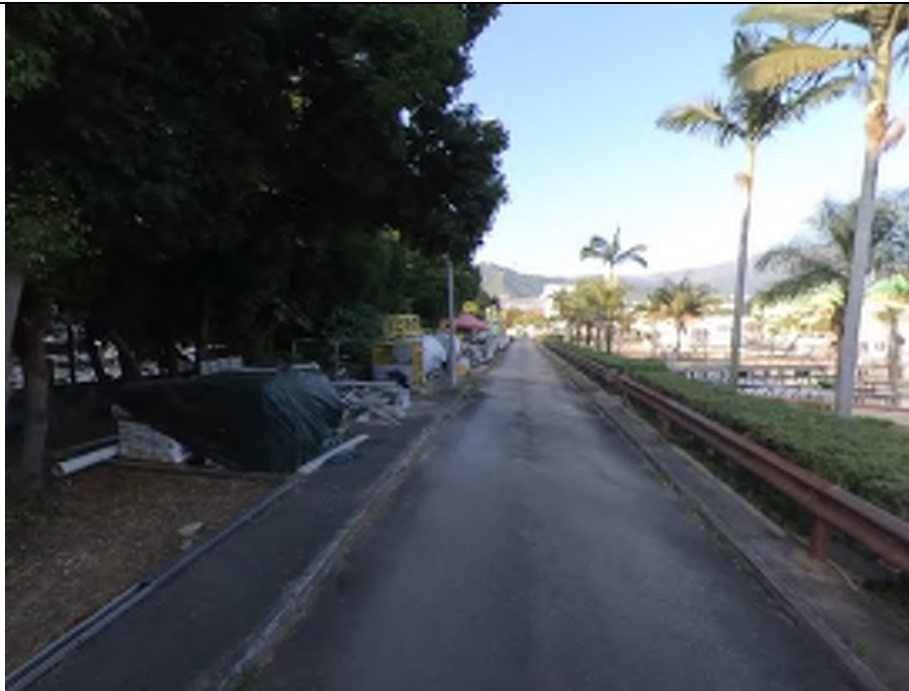
Photo WP-40: Road next to Primary Sedimentation Tanks of West Plant – The road is paved with concrete in good condition with no oil stain observed.
