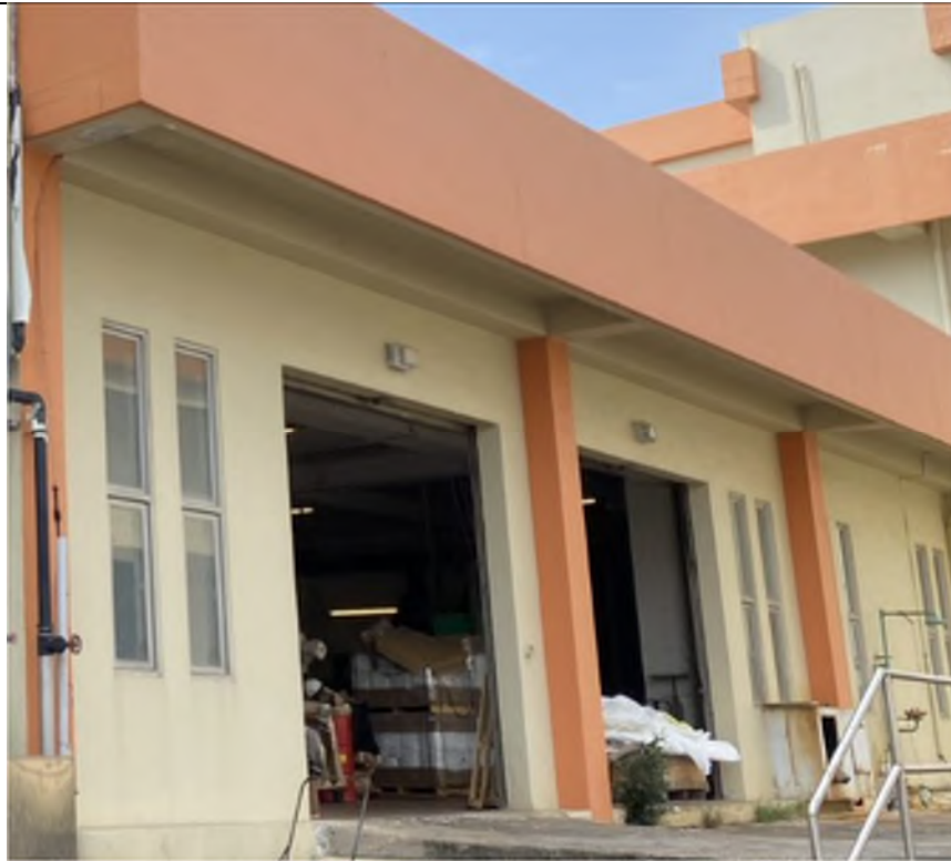
Photo WPS-18: Chemical House –The Chemical House is paved with concrete floor in good condition with no oil stain observed.
