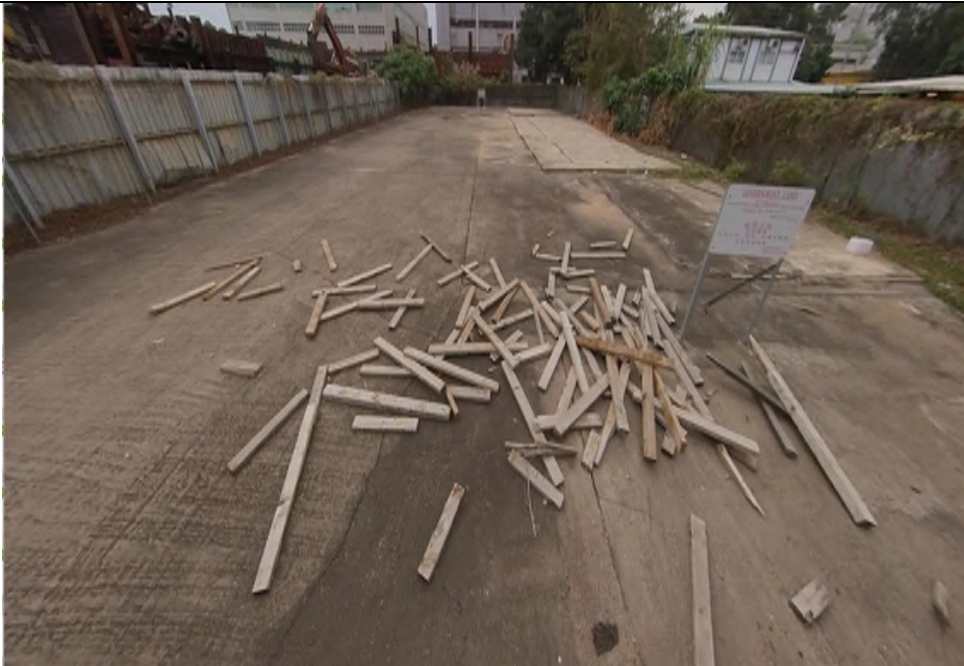
Photo EA-10: Existing Vacant Land (Previously Lot No. GLA-TPP 786 - CEDD's Site Office) – The land is paved with concrete floor in good condition with no oil stain observed.
