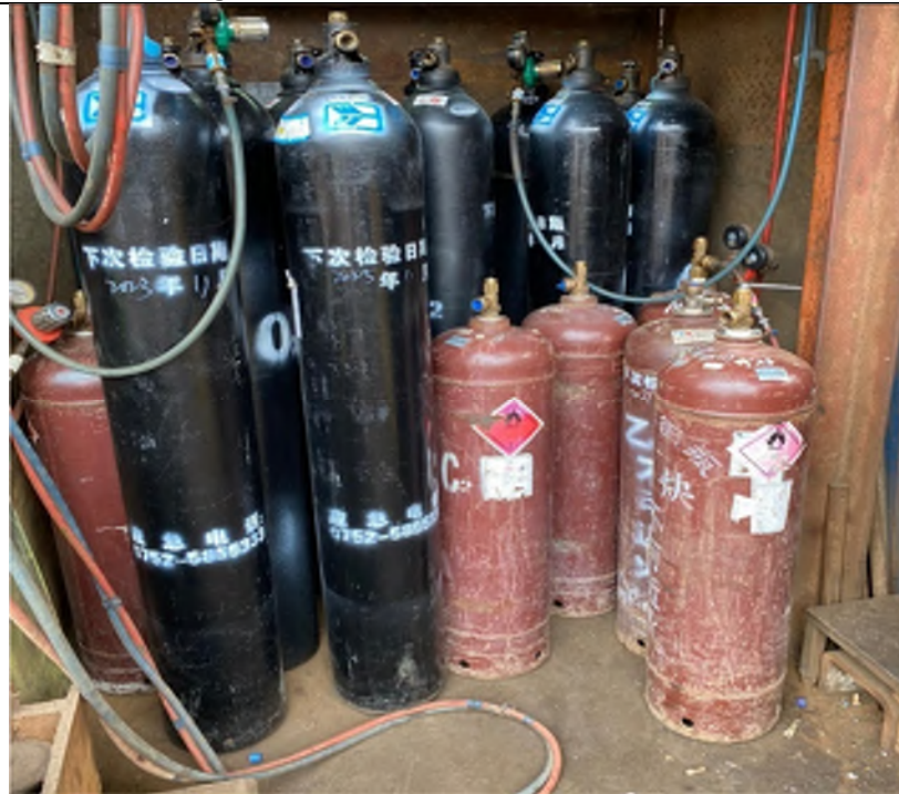
Photo EA-14: Lot No. STT 1450 - Existing C & H Import & Export Co. - Acetylene cylinders are stored in a wood cupboard.
