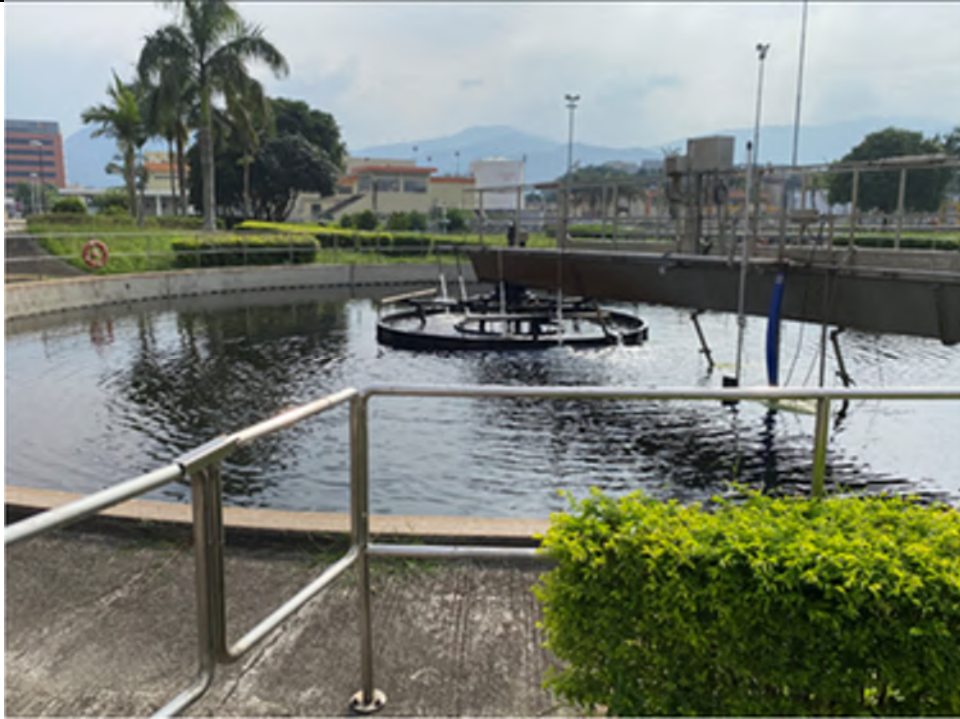
Photo WP-33: Final Sedimentation Tanks of West Plant - The tanks are located on concrete paved floor in good condition with no oil stain/stressed vegetation observed.
