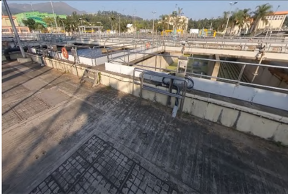
Photo WP-37: Aeration Tanks of West Plant - The tanks are located on concrete paved floor in good condition with no oil stain/stressed vegetation observed.
