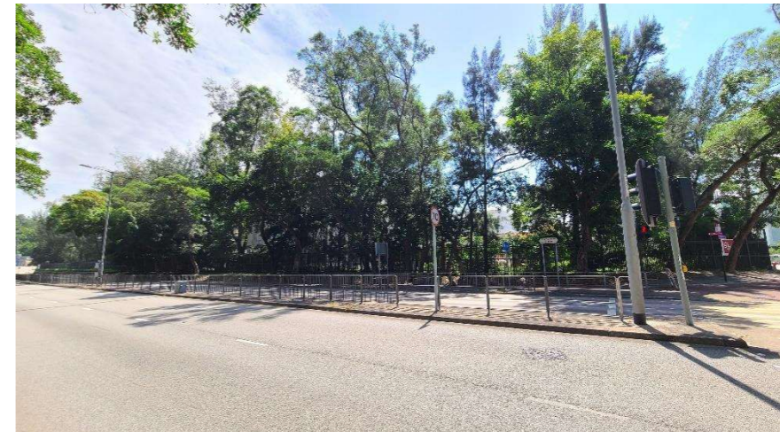
LR 5.1 – Ting Kok Road Roadside Amenity Planting
