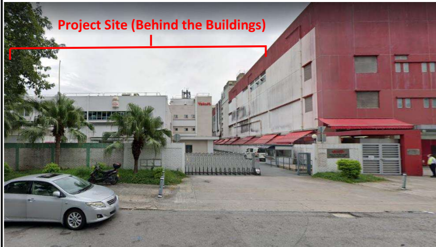
O1 – Occupants of Tai Po Industrial Estate (from North)
