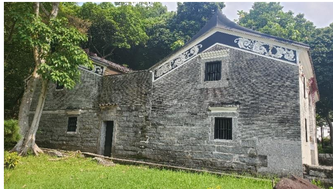
Side (Northwest) Façade of the Old House
