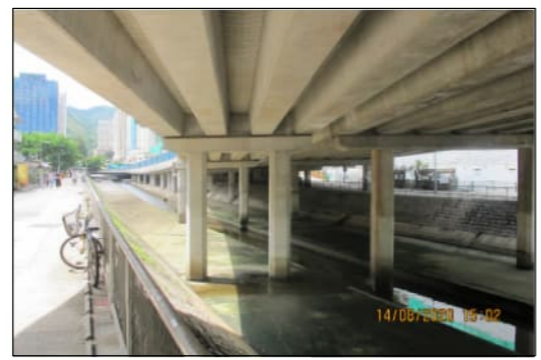
PHOTO 4131: FO TAN NULLAH UNDER FO TAN ROAD (DATE TAKEN: 14 AUGUST 2020)
