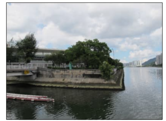
PHOTO 9494: SHING MUN RIVER CHANNEL (DATE TAKEN: 14 AUGUST 2020)
