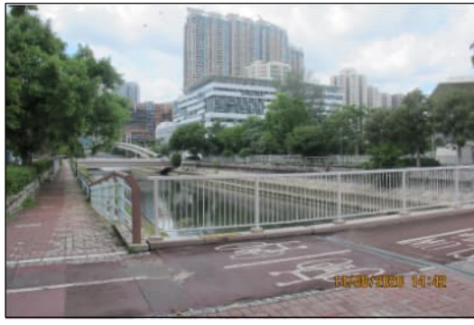
PHOTO 4114: CYCLING TRACK, FOOTPATH AND FOOTBRIDGE (DATE TAKEN: 14 AUGUST 2020)
