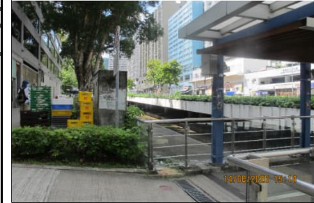
PHOTO 4153: FOOTBRIDGE AND FO TAN NULLAH (DATE TAKEN: 14 AUGUST 2020)
