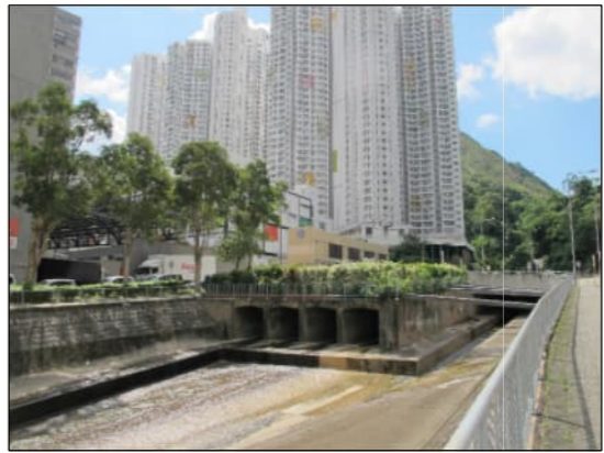
PHOTO 9537: BOX CULVERT OF FO TAN NULLAH (DATE TAKEN: 14 AUGUST 2020)
