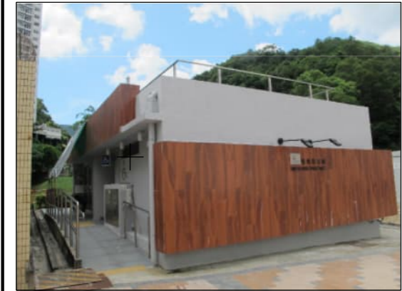
PHOTO 9544: KWEI TEI STREET PUBLIC TOILET (DATE TAKEN: 14 AUGUST 2020)
