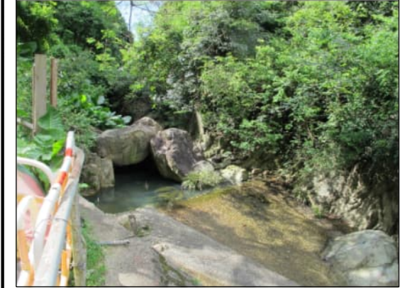
PHOTO 9551: UPSTREAM OF FO TAN NULLAH (DATE TAKEN: 14 AUGUST 2020)
