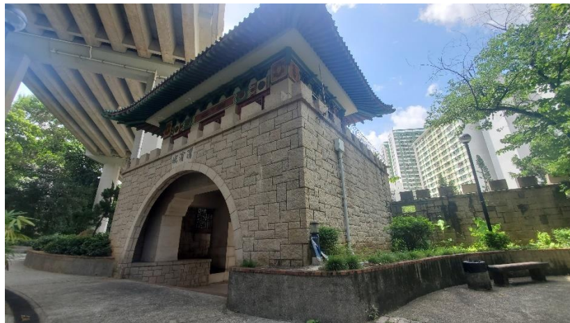
Gatehouse of Pok Ngar Villa (North Façade)
