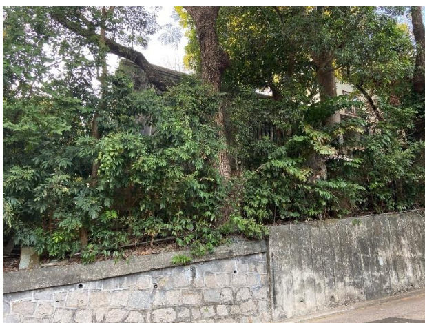
Stone Retaining Wall of Li Cottage
