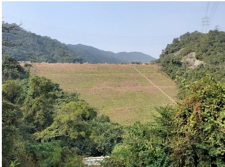
Dam of Lower Shing Mun Reservoir (Facing West)
