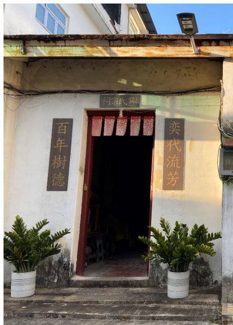
Tse Ancestral Hall (South Façade)
