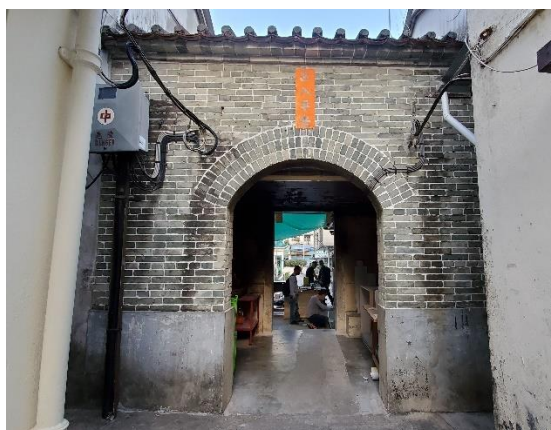
Entrance Gate of Chik Chuen Wai (Rear Doorway)
