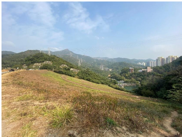
Dam of Lower Shing Mun Reservoir (Facing East)
