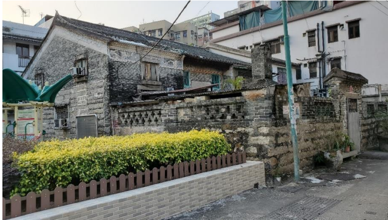
Nos. 1, 2 and 3 First Street
