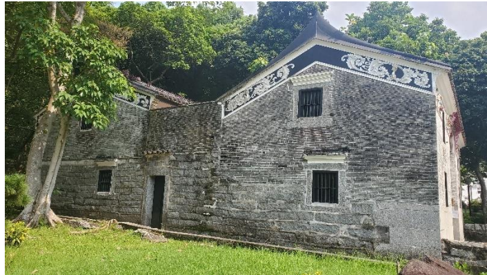
Side (Northwest) Façade of the Old House
