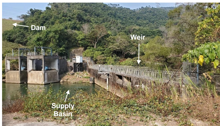
Weir of Lower Shing Mun Reservoir (Facing Northwest)
