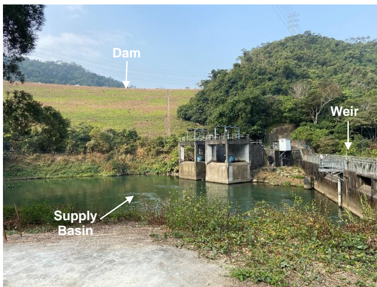
Supply Basin of Lower Shing Mun Reservoir (Facing West)
