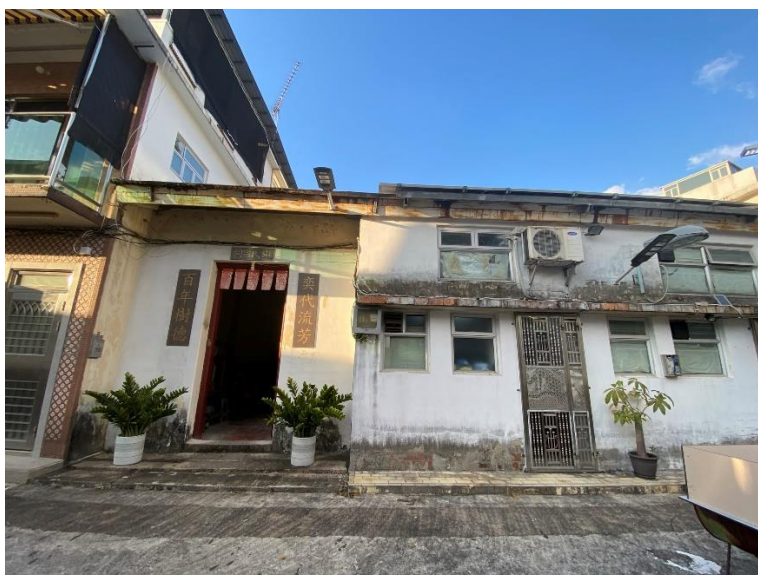
Tse Ancestral Hall and the Village houses on Two Sides (South Façades)
