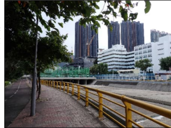
PHOTO 3461: FOOTPATH AND CYCLING TRACK AT TAI WAI NULLAH (DATE TAKEN: 31 OCTOBER 2022)
