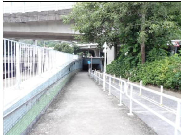
PHOTO 3464: PEDESTRIAN UNDERPASS (DATE TAKEN: 31 OCTOBER 2022)
