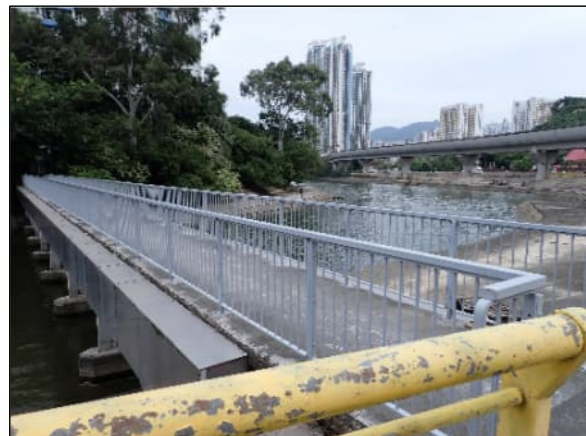
PHOTO 3450: FOOTBRIDGE AND TAI WAI NULLAH (DATE TAKEN: 31 OCTOBER 2022)
