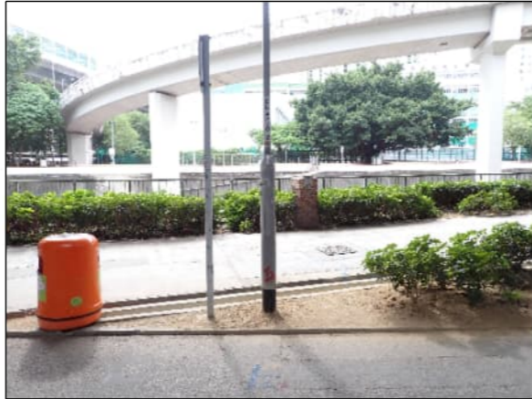
PHOTO 3465: LAMPOST BE4330 AND FOOTPATH (DATE TAKEN: 31 OCTOBER 2022)
