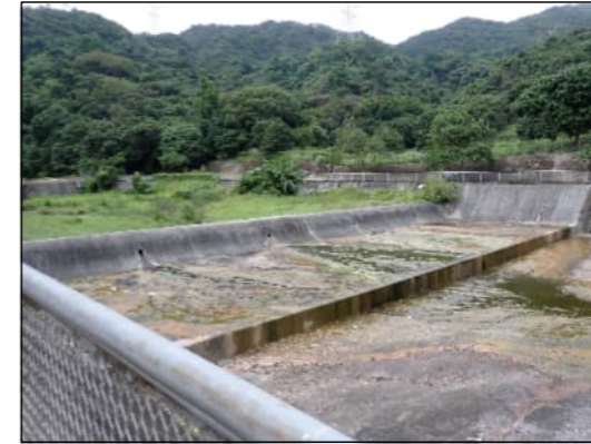
PHOTO 3521: UPSTREAM OF TAI WAI NULLAH (DATE TAKEN: 31 OCTOBER 2022)
