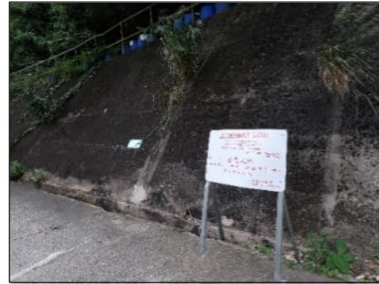
PHOTO 3552: SLOPE (7SW-D/C331) (DATE TAKEN: 31 OCTOBER 2022)
