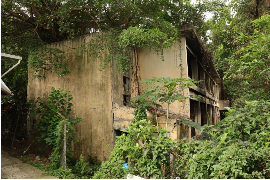
Side view of the school building from southwest
