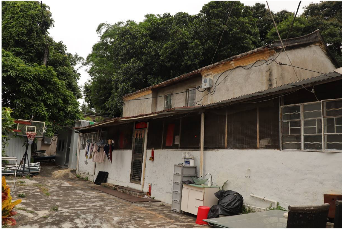
Side view from northeast
