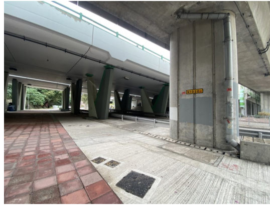
Photo 18: Pedestrian access underneath the elevated Tuen Mun Road
