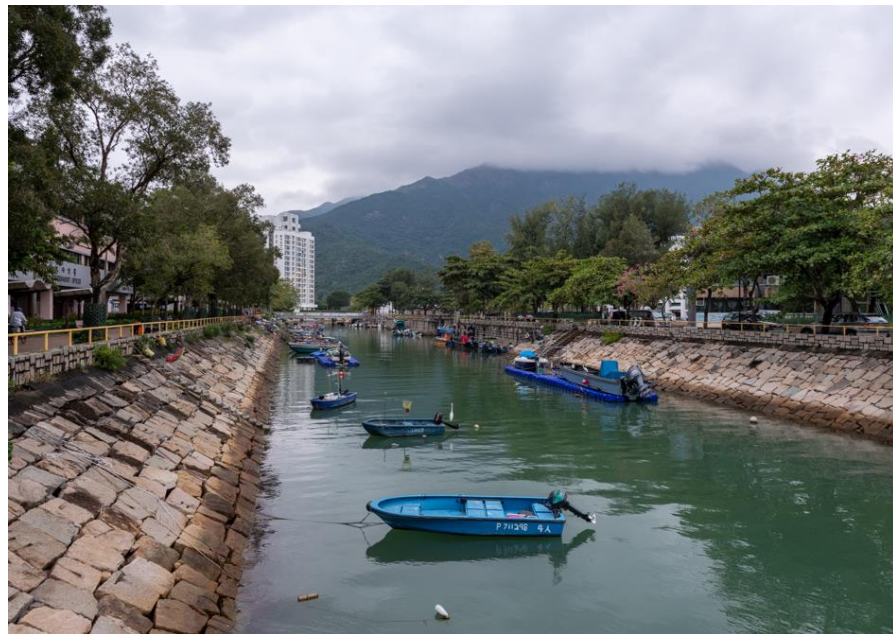
LR 10 - Channelised Watercourse
