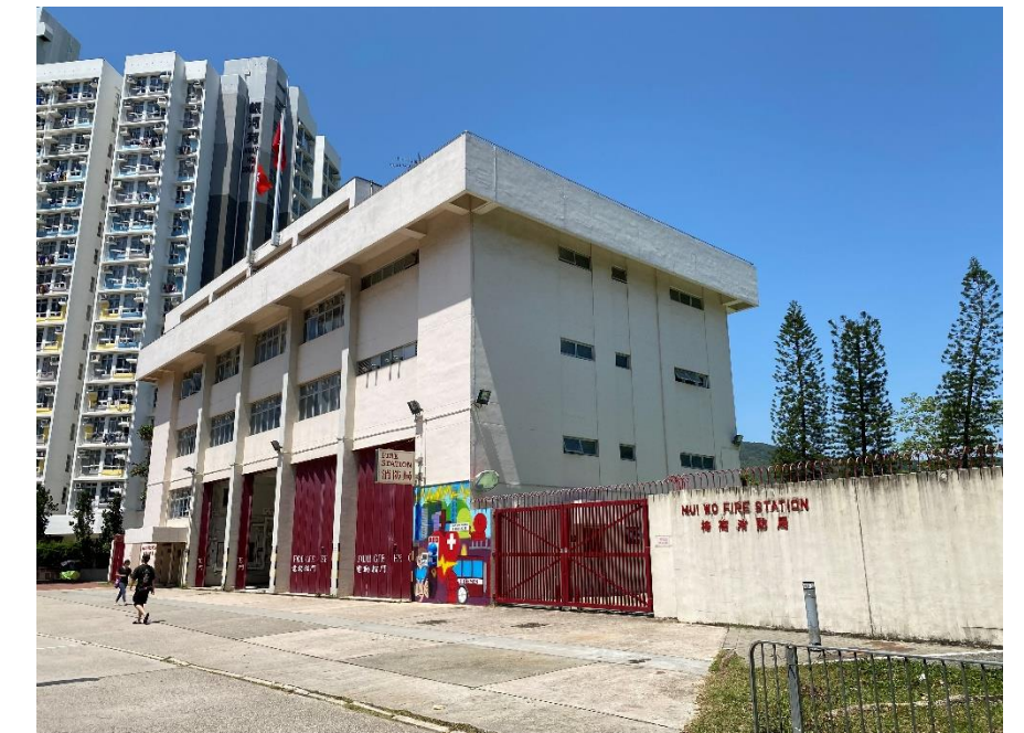
O6 - Mui Wo Fire Station
