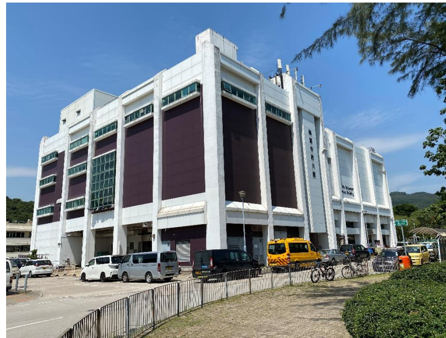
O5 - Mui Wo Municipal Services Building
