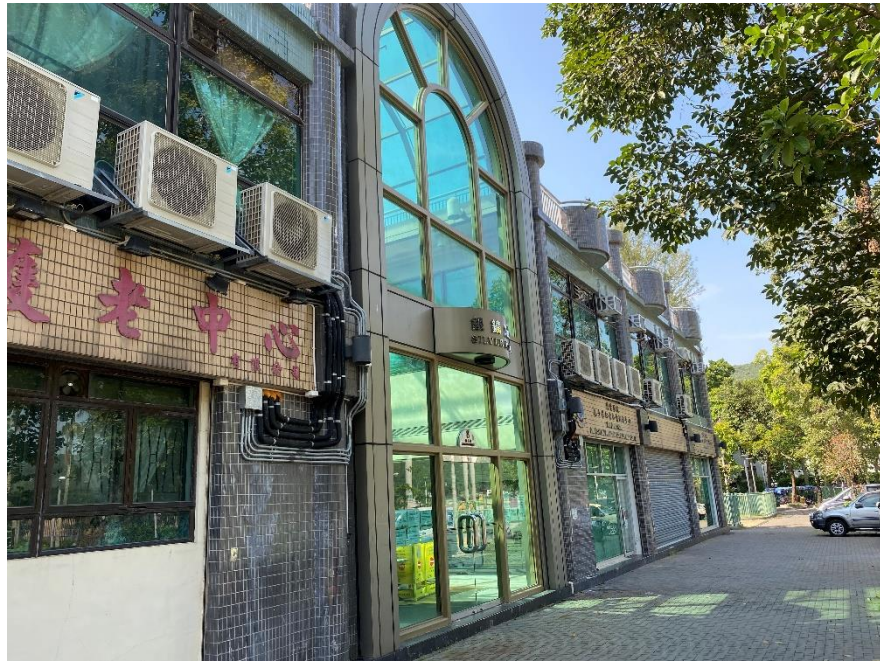
O1 - Silver Plaza (including Lai Lai Nursing Centre and Chan Shi Sau Memorial Social Service Centre)
