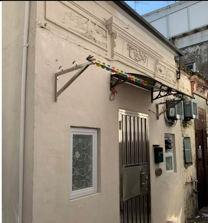
Figure 31. No. 25, Fan Tin Tsuen (FTT09). It is a traditional Chinese vernacular pitched roof brick house. It is in a one-half-one-courtyard plan. Plastered relief under eaves and on door canopy can be found.
