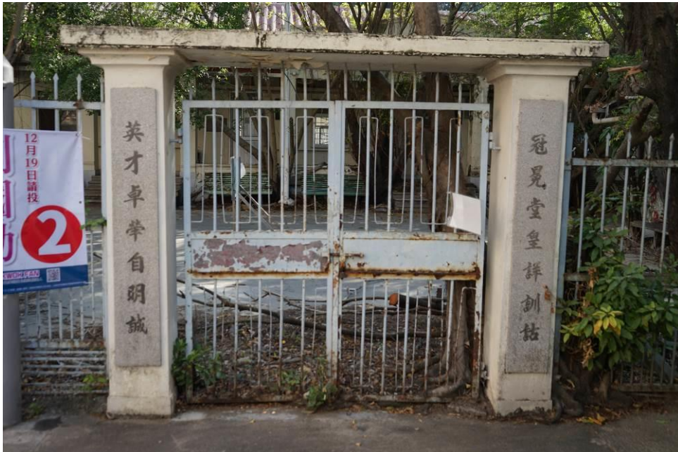
Figure 162. Former Koon Ying Public School (MPT20). The entrance gate of the school is flanked by a pair of terrazzo couplet.
