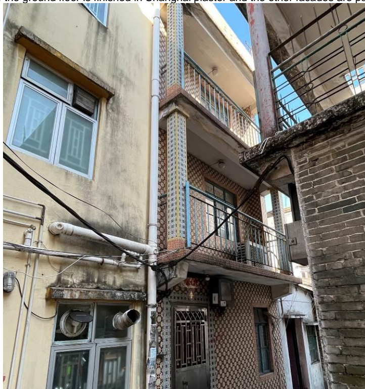
Figure 148. No. 17, Mai Po San Tsuen (MPT07), a three-storey village house with a flat roof. The building has a balcony with two square corner columns at the second and third storey. The front façade of the building is finished in mosaic tiles.
