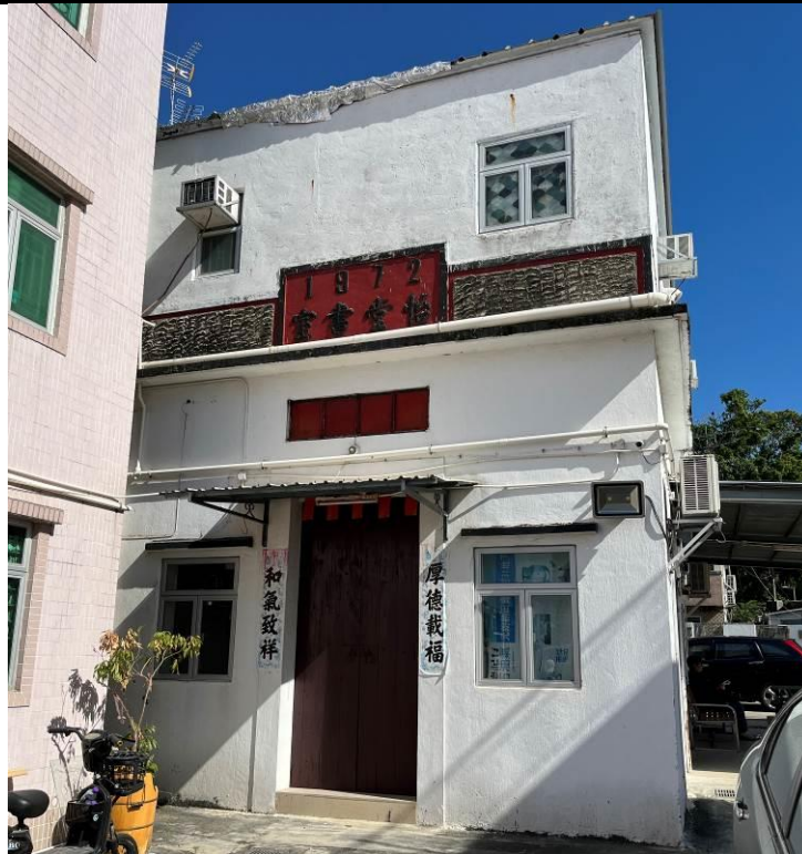
Figure 95. Yee Tong Study Hall, Tsing Lung Tsuen (TLT07), a two-storey village building with a flat roof. The building has a high-ceiling ground floor, the first floor is probably a later addition. Its parapet wall has decorative patterns and inscriptions of “1972 怡堂書室” (1972 Yee Tong Study Hall). The exterior is painted in white. Its significance in cultural heritage is noteworthy in architectural and social perspective for demonstrating the importance of education in the Man clan.
