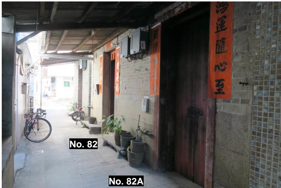
Figure 37. No. 82 and 82A, Fan Tin Tsuen (FTT18 and FTT19). No. 82 and 82A are traditional Chinese vernacular brick houses with a one-hall-one-courtyard plan. The building is decorated by plastered relief under eaves and on door canopy. Part of the front façade of No. 82A is finished with mosaic tiles.
