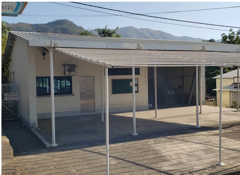
Figure 173. Sun Tin Vegetable Marketing Co-operative Society, Ltd. (SHT01). Built on an elevated platform, this building is a single-story building with a pitched roof of corrugated sheets. The front porch is extended with a simple structural frame formed by thin columns, providing more sheltered space in front of the building. The building is Utilitarian in style. A signboard with Chinese characters of “新田蔬菜產銷有限責任合作社 Sun Tin Vegetable Marketing Co-operative Society, Ltd.” is hung on the front wall.
