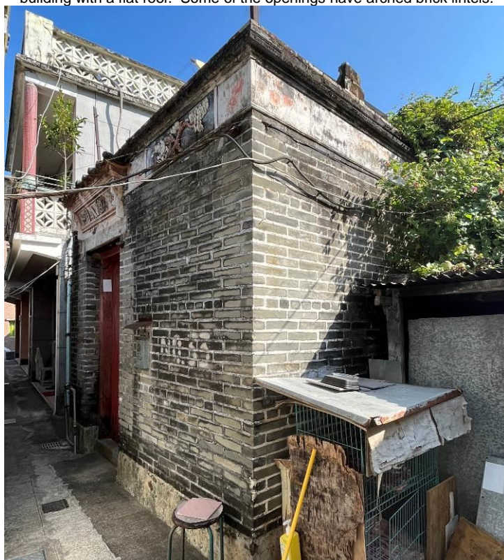
Figure 116. No. 50, Lok Ma Chau Tsuen (LMC13). It is a traditional Chinese vernacular brick building in a one-hall-one-courtyard plan. The building is relatively decorative – it has plastered mouldings of flora motifs on the door canopy and on the top of the wall on the front façade, as well as murals of flora motifs on the wall friezes from the front elevation extending to the side elevations.
