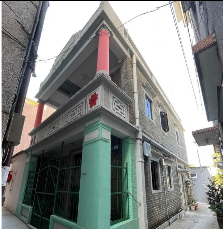
Figure 59. No. 106, Fan Tin Tsuen (FTT23), a two-storey brick house with a flat roof. The building has a two-storey front portico, the corner columns at ground level are in square shape. There are also two round columns and ornamental parapet of geometric pattern and flower symbols at balcony level. The parapet wall on the roof has “1957” inscribed indicating the construction year.
