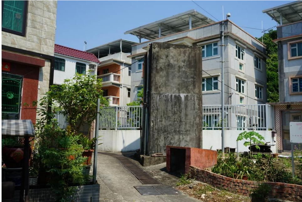
Figure 137. Pump House (PUT12). The pump house is located at the eastern end of the village. According to the villagers, it was possibly built in the 1960s. It was disused when tap water pipes were laid and connected to each house in the 1980s at Pun Uk Tsuen.
