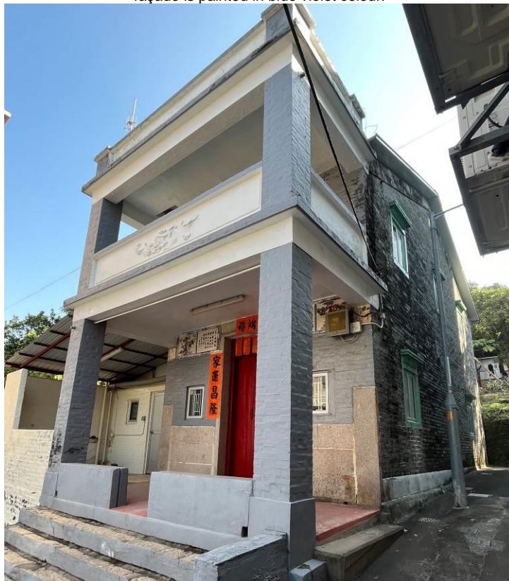
Figure 126. No. 51, Lok Ma Chau Tsuen (LMC14). All the window openings on the side elevations have label mouldings and rendered surrounds.
