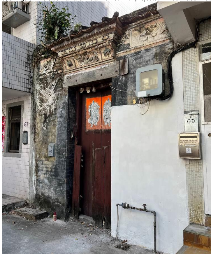
Figure 40. No. 88, Fan Tin Tsuen (FTT21), a traditional Chinese vernacular single-storey house. Plastered relief can be found under eaves and on door canopy.
