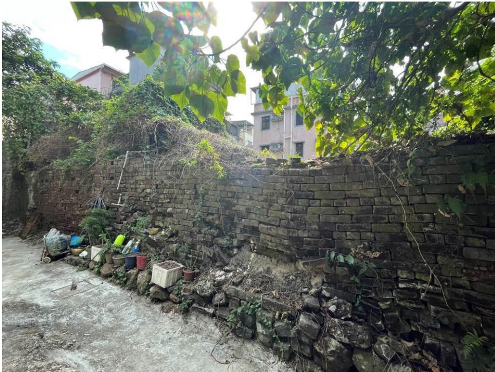
Figure 69. Northeast Enclosing Wall.
