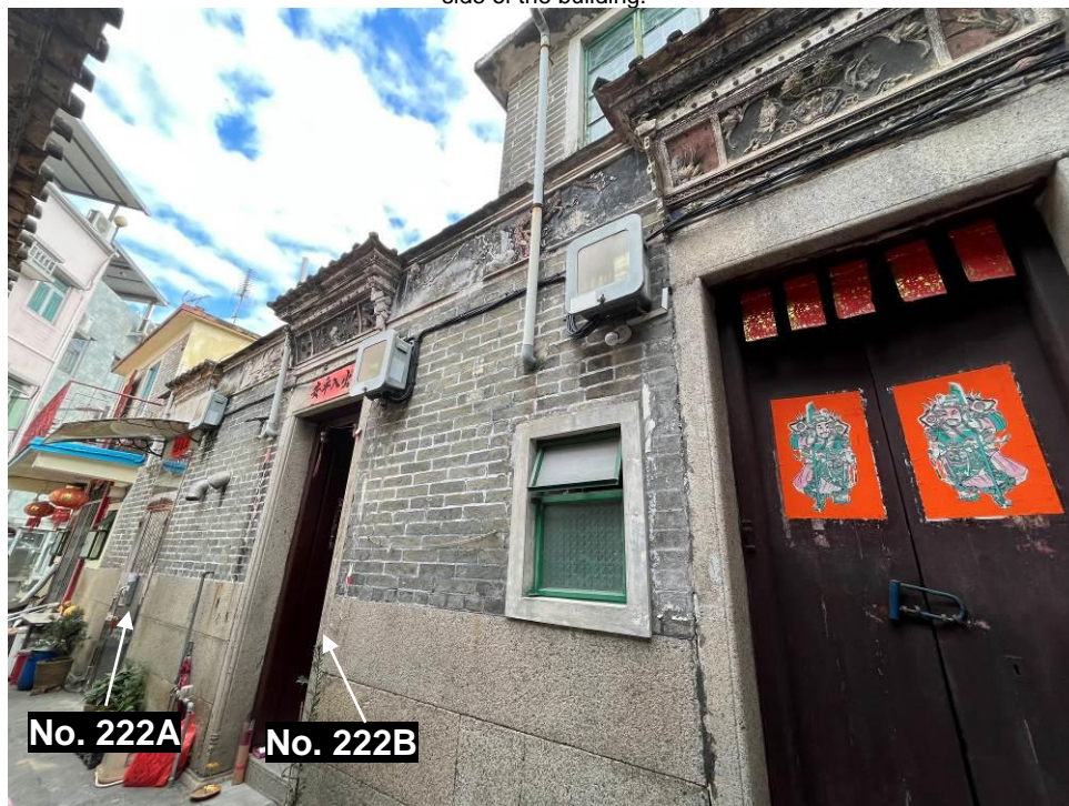
Figure 50. Nos. 222A and 222B (FTT39 and FTT40), Fan Tin Tsuen, front elevation. They are traditional Chinese vernacular houses with a one-hall-one-courtyard plan. The building is constructed of bricks with a granite base. Plastered relief can be found under eaves and on door canopy.
