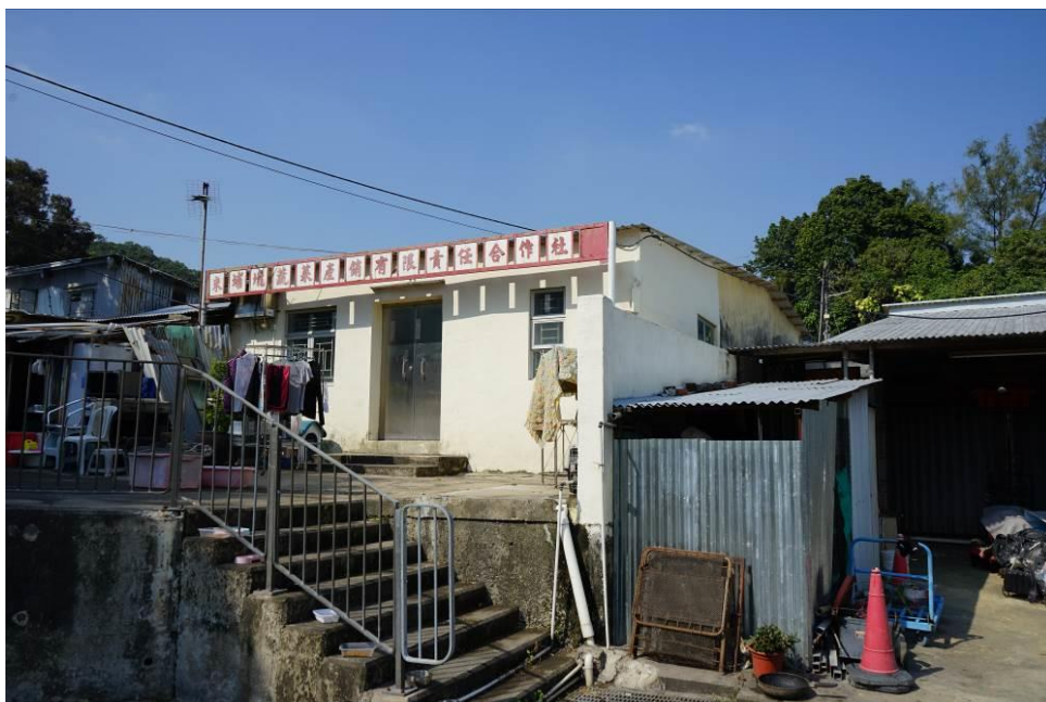
Figure 172. Mai Po Lung Vegetable Marketing Co-operative Society, Ltd. (MPL02), another structure opposite the road. It is a single storey building with a flat roof. The building is Utilitarian in style. The building also has a signboard with Chinese characters of “米埔隴蔬菜產銷有限責任合作社” (literally Mai Po Lung Vegetable Marketing Co-operative Society ) is placed on the roof. Simple staircase is attached to the front of the platform providing access. As one of the vegetable marketing cooperative societies, the Mai Po Lung Vegetable Station is a testimony of the agricultural cooperative movement in the New Territories in the latter half of the 20th century.
