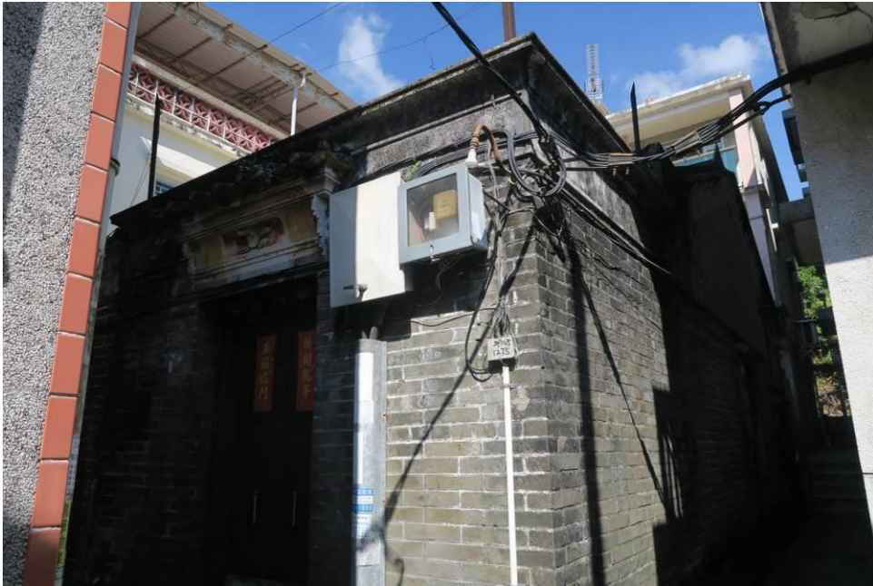
Figure 129. No. 1, Pun Uk Tsuen (PUT01), a traditional Chinese vernacular brick house. It is in a one-half-one-courtyard plan. The building is decorated by the plastered mouldings of auspicious motifs on the door canopy.
