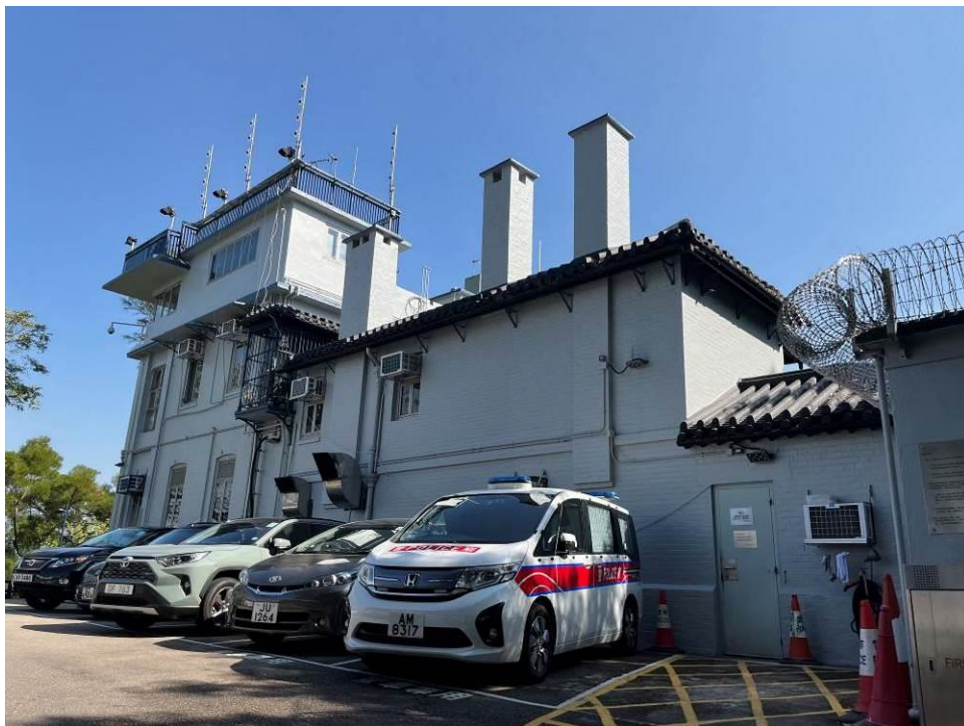
Figure 44. Side elevation. Original features such as Chinese pitched roofs and chimney stacks are retained.
