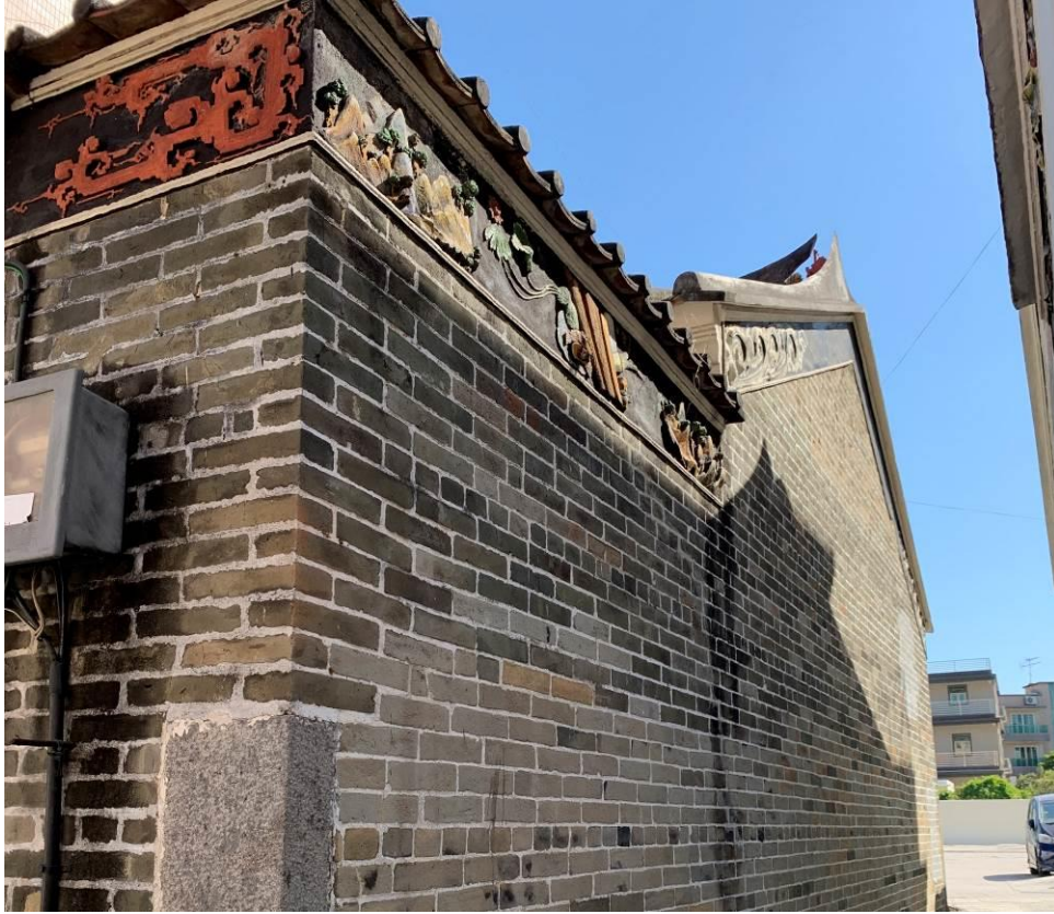
Figure 55. Side elevation (southwest façade).
