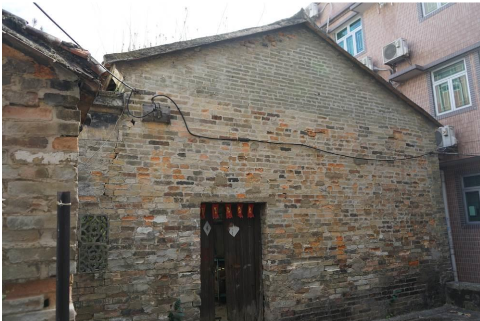
Figure 80. No. 32C, Wing Ping Tsuen (WPT04). The building is in a one-hall rectangular plan with its walls supporting the pitched roof.
