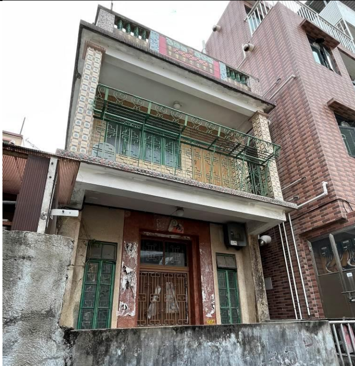
Figure 73. No. 235A, Fan Tin Tsuen (FTT44). It is a two-storey village house with a flat roof. The building has a balcony with two square columns finished in ceramic tiles. The front façade is finished in Shanghai plaster. Extensive use of geometric patterns is observed on the window grilles, entrance gate and the railings of the balcony.
