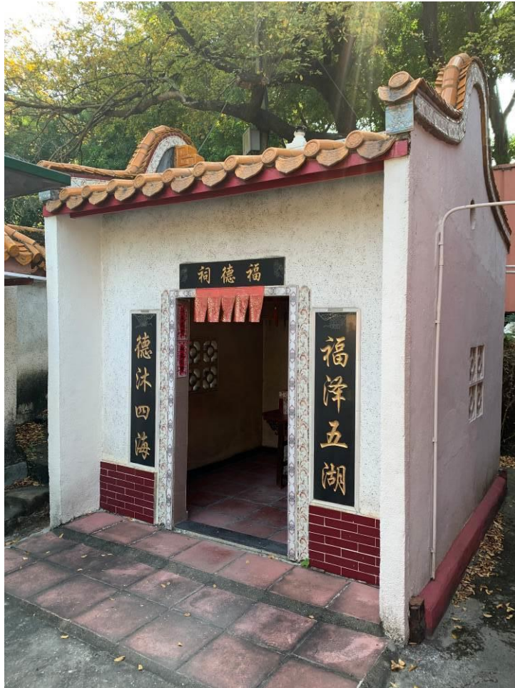
Figure 166. Fuk Tak Temple. The Temple is a one-bay structure with a pitched roof. It is the smallest temple in the compound. Its rounded gable wall is probably of "wood" nature in wuxing (五行木屬). The front elevation of the building is recessed and finished in Shanghai plaster and ceramic tiles. The entrance is flanked by a couplet on its sides and a horizontal plaque above.
