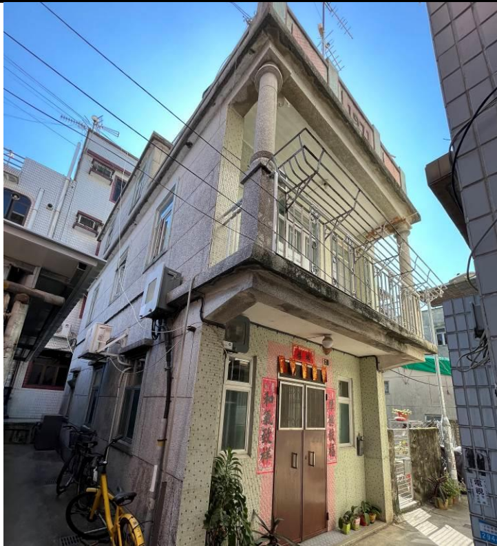
Figure 55. No. 20, Fan Tin Tsuen (FTT08). It is a two-storey village house constructed in 1971. The building has a balcony with two columns on both sides of the corners. The parapet wall on the roof has characters of “1971” indicating the construction year. The front façade is finished with mosaic tiles, while the other façades are finished with Shanghai plaster.
