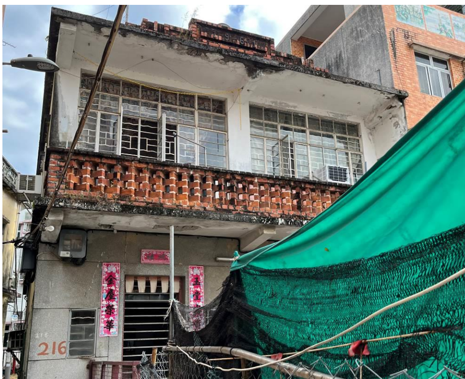
Figure 70. No. 216, Fan Tin Tsuen (FTT35), a two-storey village house with a flat roof. The parapet at the balcony is constructed of bricks which is layered in a way that allows ventilation. The ground floor is finished with Shanghai plaster. The first floor has large window openings with modern window grilles. The parapet wall on the roof is also constructed of bricks.
