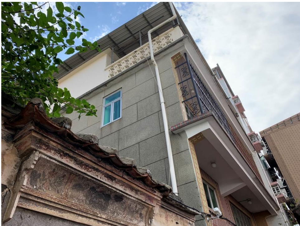
Figure 6. Nos. 17-18, Yan Shau Wai (YSW04), a two-storey village house comprising of two residential units. The building has a flat roof and a balcony at the first floor. The front elevation of is finished in ceramic tiles while the side elevations are finished in Shanghai plaster.
