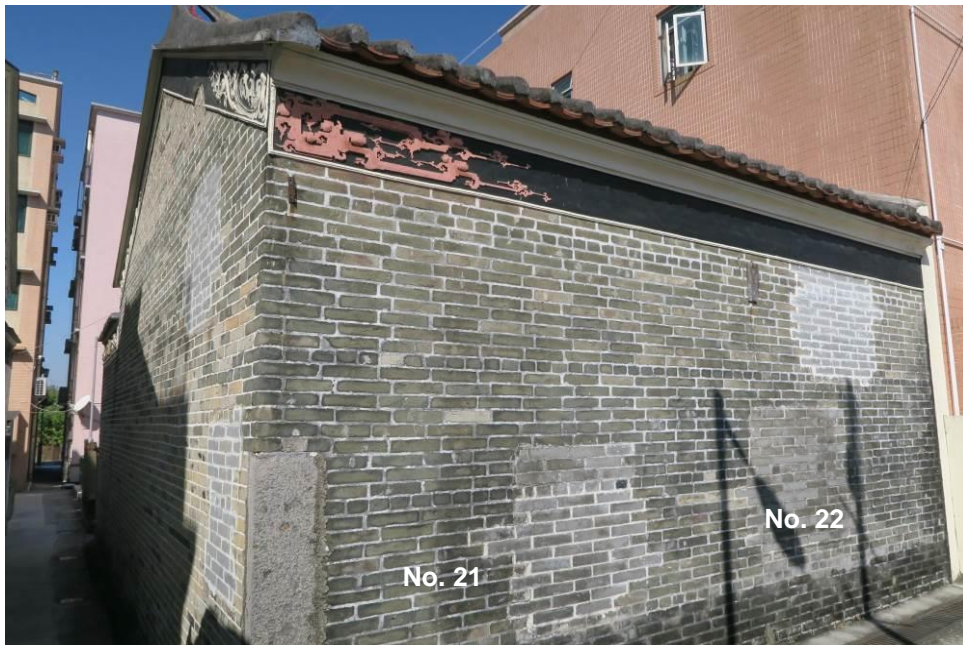
Figure 56. Back elevation (southeast façade).
