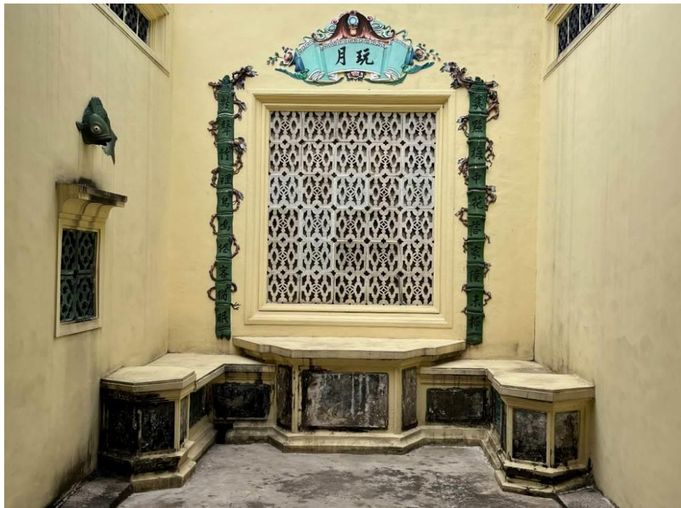
Figure 26. Enclosed Courtyard, East Annex. The Chinese characters “玩月” (literally meaning “Moon Watching”) is seen on the mortared horizontal plaque above.
