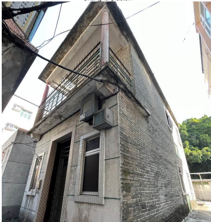
Figure 146. No. 8, Mai Po San Tsuen (MPT05), a two-storey village house with a flat roof. The building has a balcony with two round corner columns. The front façade of the ground floor is finished in Shanghai plaster and the openings are surrounded with mosaic tiles.
