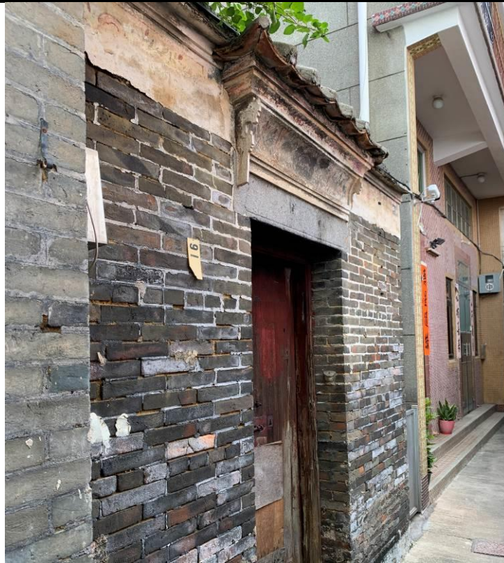
Figure 3. No. 16, Yan Shau Wai (YSW03), a traditional Chinese vernacular pitched-roof building. It is in a one-hall-one-courtyard plan. The building is decorated by the murals under eaves and on door canopy.
