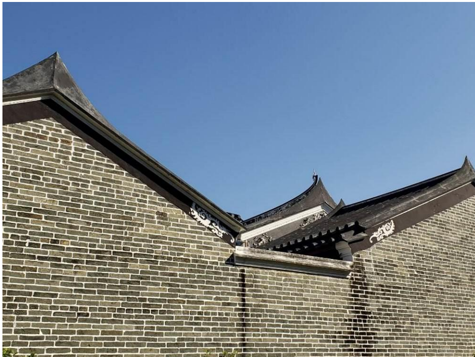
Figure 14. Side Elevation (Northwest Façade).
