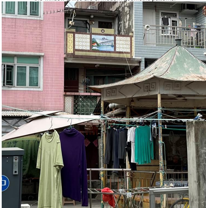
Figure 68. No. 194B, Fan Tin Tsuen (FTT32). It is a two-storey village house with a flat roof. The parapet at the balcony level is formed with ventilation tiles. The parapet wall on the roof is decorated with mosaic tiles and a drawing of scenery painted on tiles.
