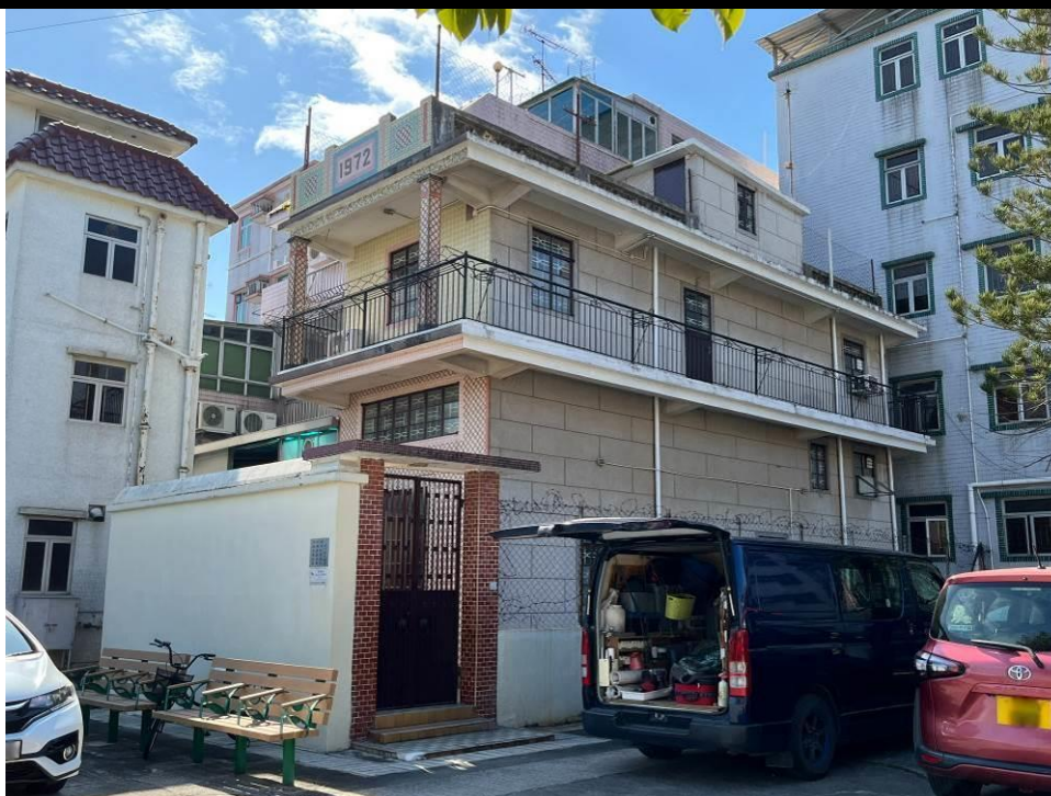
Figure 85. No. 22A, On Lung Tsuen (OLT02), a two-storey village house with a flat roof. The building has a high-ceiling ground floor and a balcony with two square corner columns finished in mosaic tiles. The balcony extends across the front elevation and the side elevation. The parapet wall on the roof, decorated by mosaic tiles, has a “1972” pattern indicating the construction year. The front façade is finished in mosaic tiles while the remaining façades are finished in Shanghai plaster.
