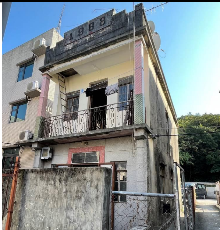
Figure 143. No. 2, Mai Po San Tsuen (MPT02), a two-storey village house. The building has a balcony with two square corner columns decorated with mosaic tiles. There is a staircase on the balcony connected to the flat roof. The parapet wall on the roof has “1968” inscribed indicating the construction year. The front façade of the ground floor is finished in Shanghai plaster and the first floor is painted in pale yellow.
