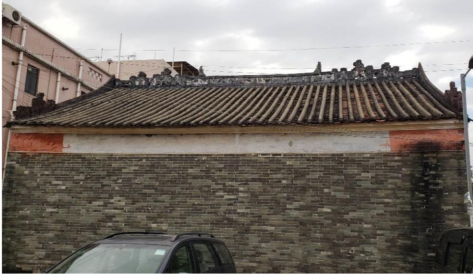
Figure 41. Back elevation (southeast façade).
