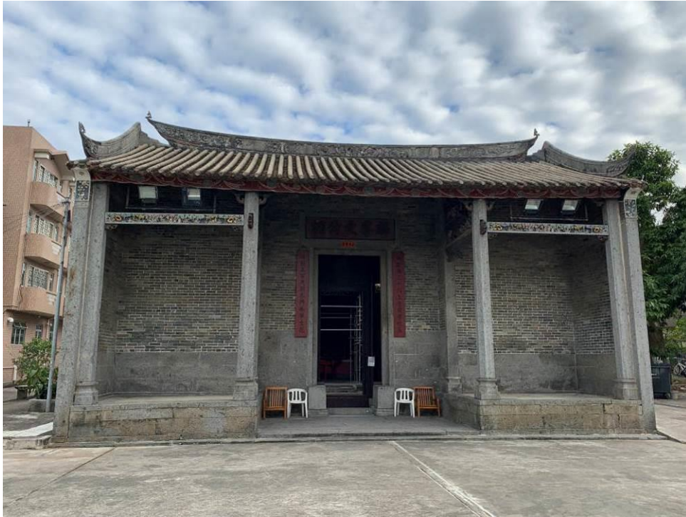
Figure 1. Front elevation (northwest façade).
