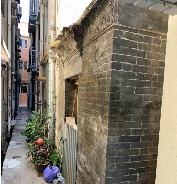
Figure 43. No. 138, Fan Tin Tsuen (FTT26), a traditional Chinese vernacular single-storey house. It is in a one-hall-one-courtyard layout. Plastered relief can be found under eaves and on door canopy. A plaster with Chinese characters of “泰山石敢當” (literally means Mount Tai Shigandang ) is painted on the right side of the front façade.
