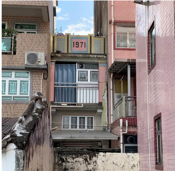
Figure 7. No. 34, Yan Shau Wai (YSW06), a two-storey village house with a flat roof. The building has a high-ceiling ground floor and a balcony with two square corner columns. The parapet wall on the roof has "1971" inscribed indicating the construction year. The façade is finished in mosaic tiles.
