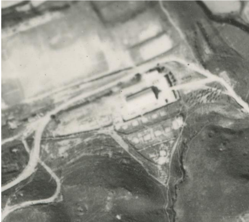
Plate 1. Construction of Gurkha Cemetery in 1956. (Source: Lands Department, 1956)
