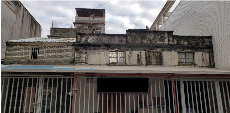
Figure 29. DD102 Lot 3186 RP (FTT06). Single-storey brick structure with a parapet wall. According to the characters on the parapet wall, the building was once a grocery named “San On Ho” (“新安號”).
