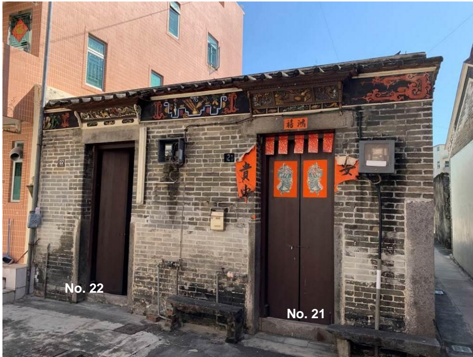
Figure 53. Front elevation (northwest façade).
