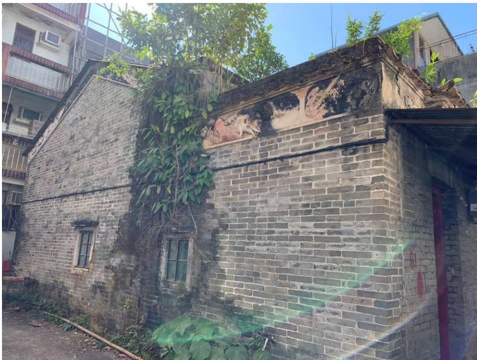
Figure 36. No. 81, Fan Tin Tsuen (FTT17). It is a traditional Chinese vernacular pitched roof brick house. It is in a one-hall-one-courtyard plan. The building is decorated by plastered relief under eaves and on door canopy.
