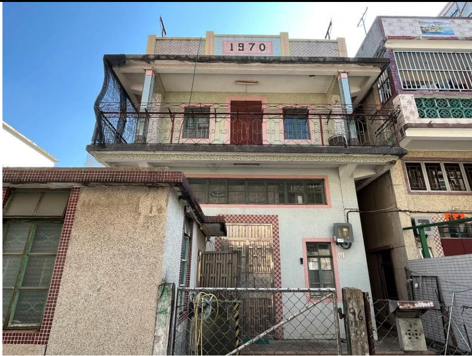
Figure 151. No. 96, Mai Po San Tsuen (MPT12), a two-storey village house with a flat roof. The building has a balcony extending across all the elevations of the building, two square columns are placed on the front façade. The parapet wall at the top has “1970” pattern formed by mosaic tiles. The front façade and the remaining facades of the first floor are finished in mosaic tiles.
