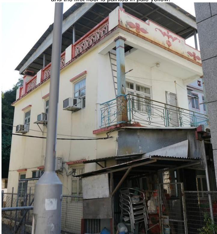
Figure 144. No. 3, Mai Po San Tsuen (MPT03), a two-storey village house. The building has a balcony with two square corner columns decorated with mosaic tiles. There is a staircase on the balcony connected to the flat roof. The parapet wall on the roof has plastered mouldings of flower and coin symbols. The exterior is painted in pale yellow.
