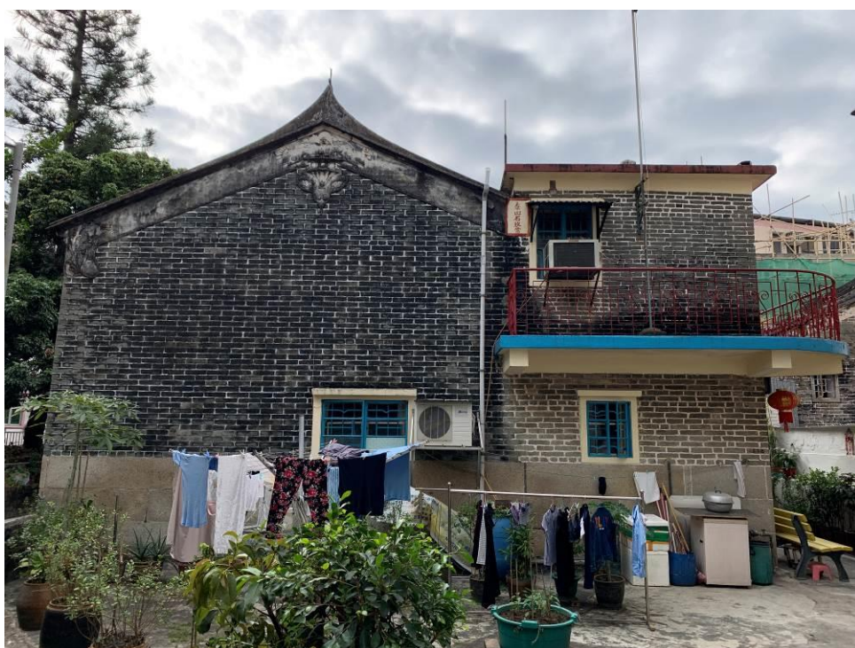
Figure 48. No. 222, Fan Tin Tsuen (FTT38), side elevation. It is a two-storey brick building with a granite base. The building was probably undergone alteration that the original front courtyard had been redeveloped into a two-storey flat-roof structure, while the back hall with pitched roof has been retained. A tablet with Chinese characters of “泰山石敢當” (literally means Mount Tai Shigandang ) is placed on the side elevation of the building. Plastered relief is observed under eaves.
