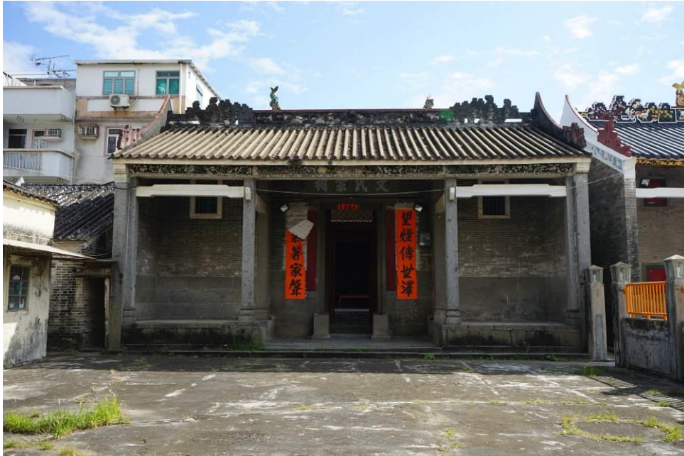
Figure 31. Front elevation (northwest façade) and the Annex Block to its left.
