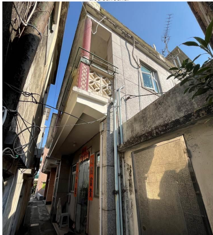
Figure 124. No. 49, Lok Ma Chau Tsuen (LMC12), a two-storey village house. The building has a balcony with round corner columns painted in red and a parapet wall on the flat roof. The exterior of the building is finished in Shanghai plaster
