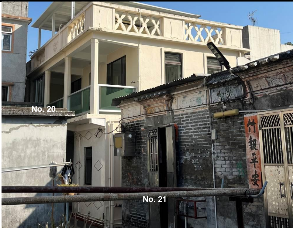
Figure 119. No. 20, Lok Ma Chau Tsuen (LMC04). It is a two-storey village house with a flat roof. The main entrance on the ground floor is recessed. The balcony on the first floor has three square columns with two at each corner and one in the middle. The parapet wall on the roof has plastered relief of flora motifs. The exterior is painted in pale yellow except the front façade of the ground floor is finished in Shanghai plaster with red diamond patterns.
