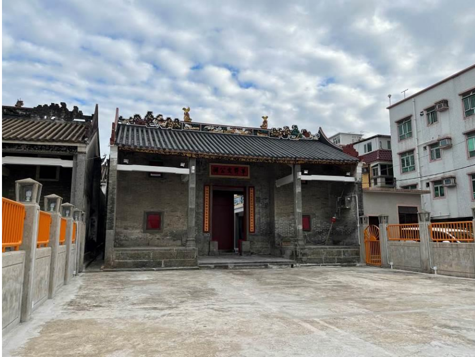
Figure 35. Front elevation (northwest façade).
