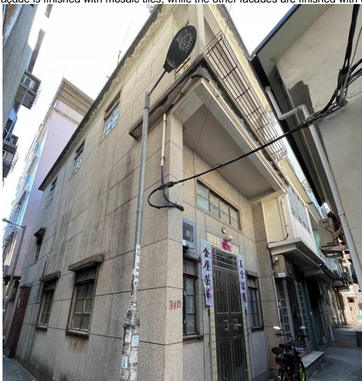
Figure 56. No. 31D, Fan Tin Tsuen (FTT12). It is a two-storey village house with a flat roof. The building has a high-ceiling first floor and a balcony with two square corner columns. The façades are finished with Shanghai plaster.
