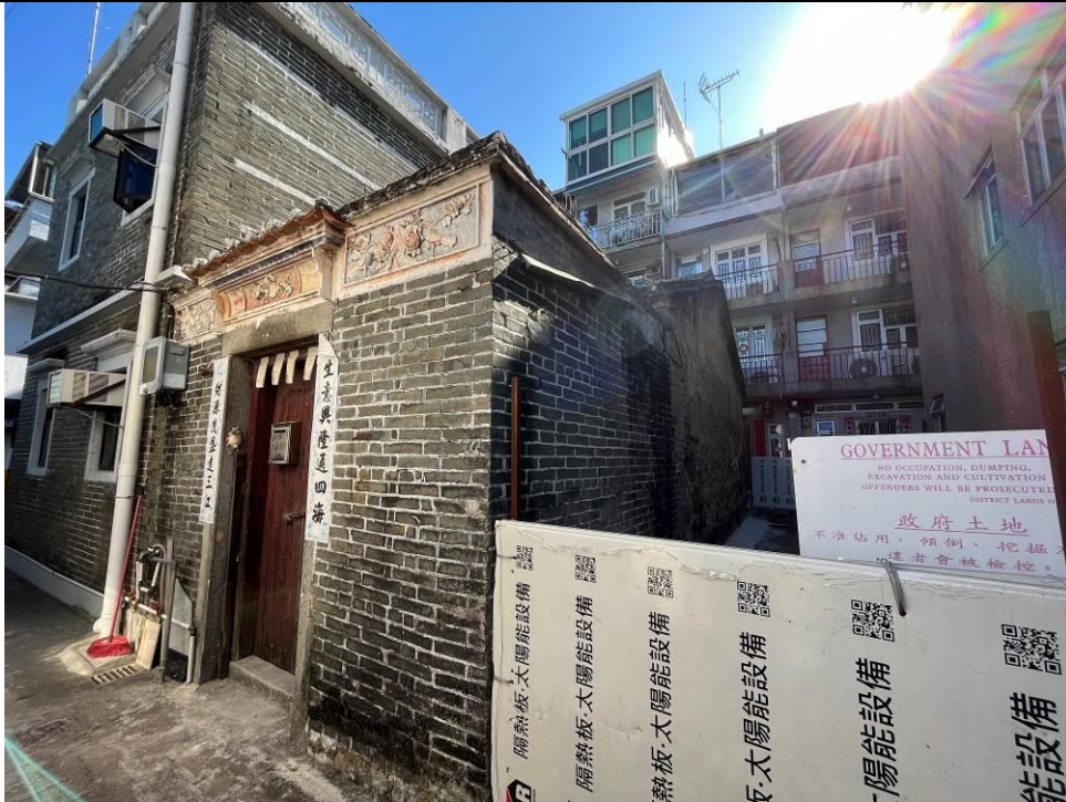
Figure 41. No. 105, Fan Tin Tsuen (FTT22). It is a traditional Chinese vernacular single-storey building. It is in a one-half-one-courtyard plan. Plastered relief is observed under eaves and on door canopy on the front façade.
