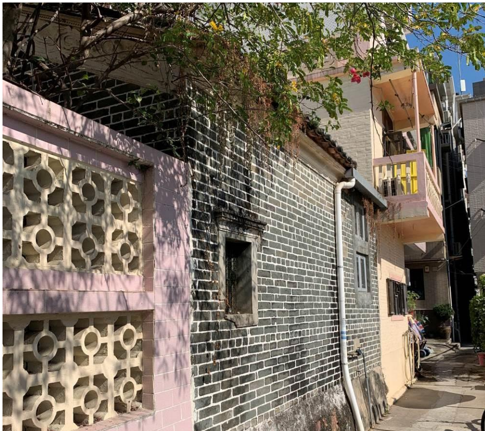
Figure 14. No. 7, Tung Chan Wai (TCW02), a traditional Chinese vernacular single-storey brick house. The building has a pitched roof and is decorated by the plastered relief of flora motif under eaves. The front elevation is not accessible.
