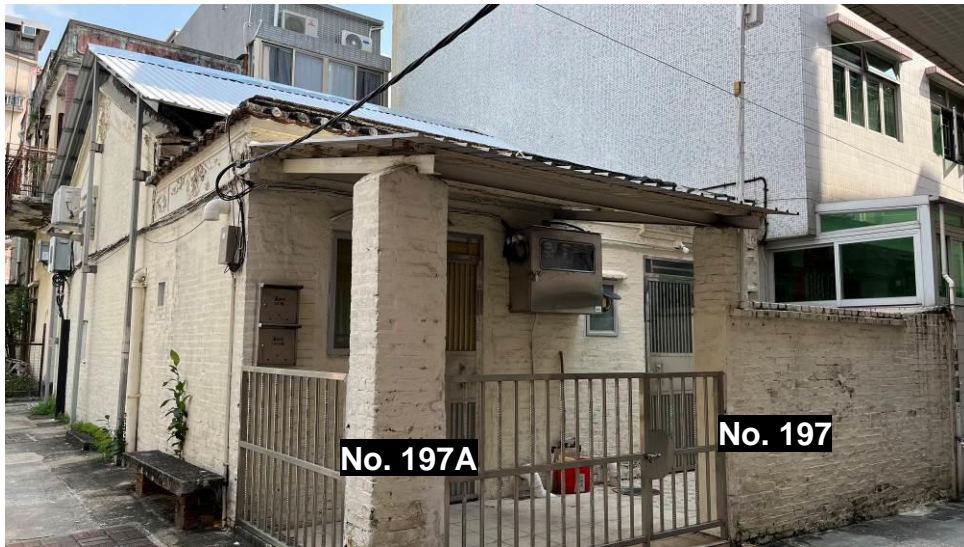
Figure 45. Nos. 197-197A, Fan Tin Tsuen (FTT33). It is a traditional Chinese vernacular single-storey house with two residential units. It is in a one-hall-one-courtyard plan. The exterior has been painted in white colour. Plastered relief can be found along the wall frieze on the front, back and side elevation. The units have a semi-enclosed front yard.
