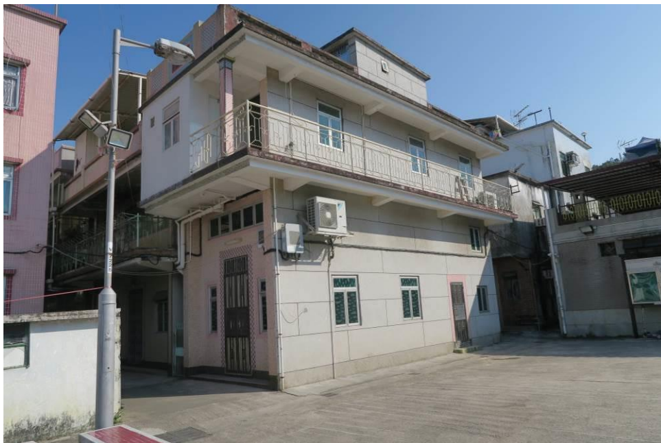
Figure 156. No. 125, Mai Po San Tsuen (MPT17), a two-storey village house with a flat roof. The building has a high-ceiling ground floor and a balcony with a square corner column at its front façade. The balcony extends from its front elevation across to the side elevation. The parapet wall on the roof has “1971” pattern created by mosaic tiles. The front façade is finished in ceramic tiles while the remaining facades are finished in Shanghai plaster. Alteration might have been carried out and enclosed half of the balcony space on the front elevation.
