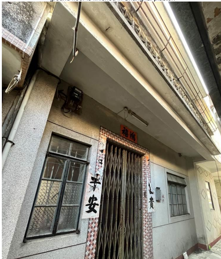
Figure 118. No. 19, Lok Ma Chau Tsuen (LMC03). It is a two-storey village house with a balcony at its first floor. The front façade of the ground floor is finished in Shanghai plaster. The entrance door has a decorative mosaic-tiled surround.
