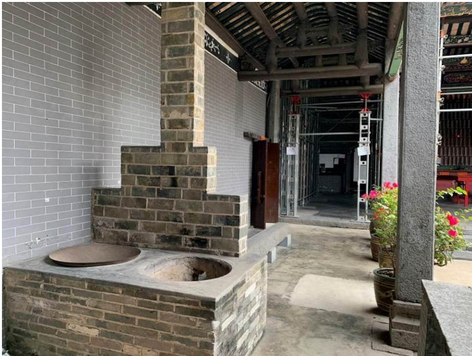
Figure 6. Left porch, first courtyard. A brick stove and chimney are installed.
