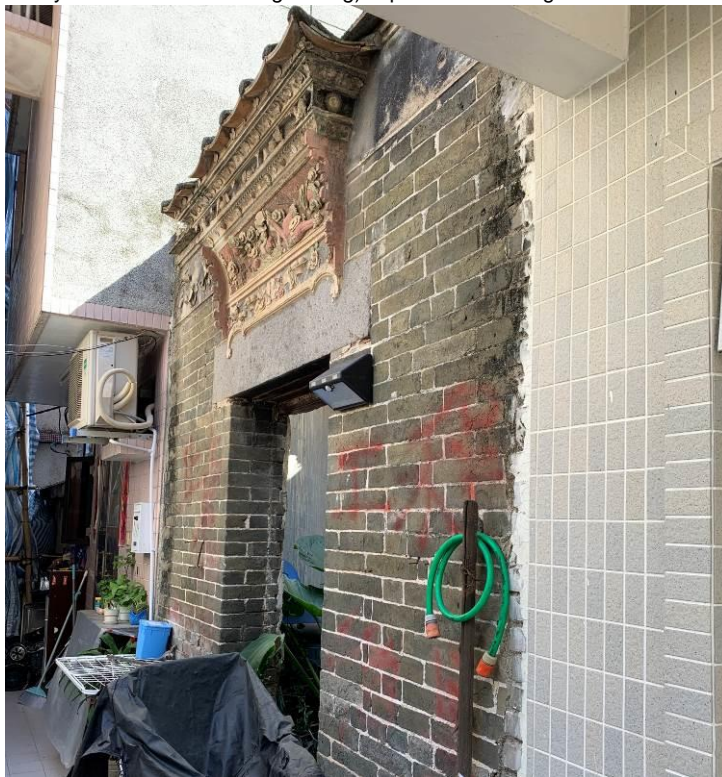
Figure 44. No. 178B, Fan Tin Tsuen (FTT30), a traditional Chinese vernacular single-storey house. It is in a one-hall-one-courtyard layout. Plastered relief can be found under eaves and on door canopy.
