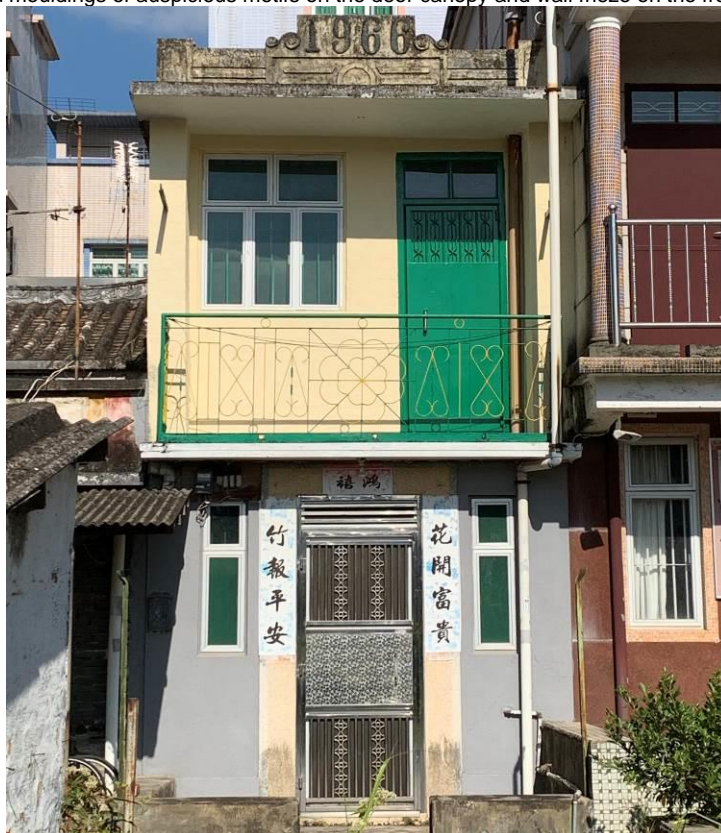
Figure 106. No. 4, Chau Tau Tsuen (CTT02), a two-storey village house with a flat roof. The building has a balcony at the first floor and a parapet wall on the roof. The barrier of the balcony and the parapet wall are decorated with geometric patterns, the parapet wall has inscription of "1966" indicating its construction year.
