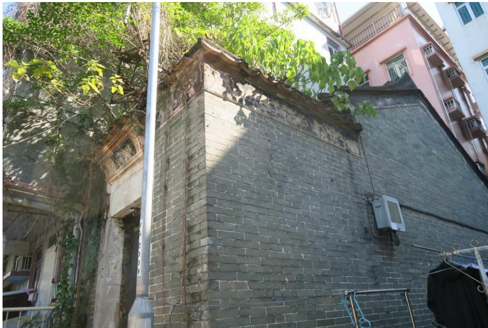
Figure 26. No. 12, Fan Tin Tsuen (FTT04). It is a traditional Chinese vernacular brick house with a one-hall-one-courtyard plan and pitched roof.
