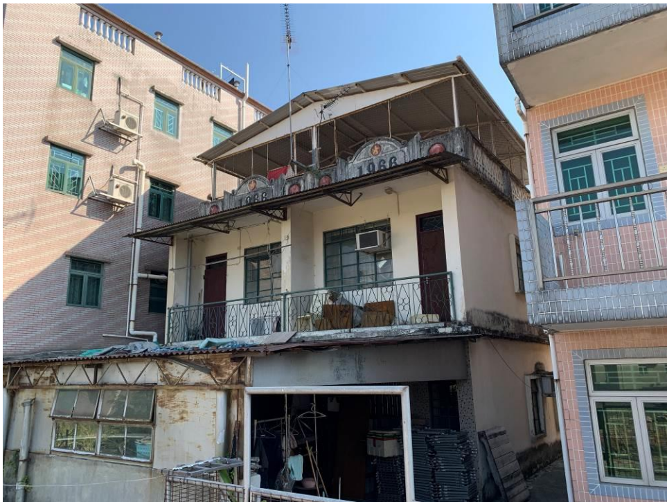
Figure 158. Nos. 131-132, Mai Po San Tsuen (MPT19), a two-storey village house with two residential units. The building has a balcony on its first floor. The parapet wall on the roof of each unit is semi-circular in shape and has plastered mouldings of “1966” pattern and a star within a red circle on top.
