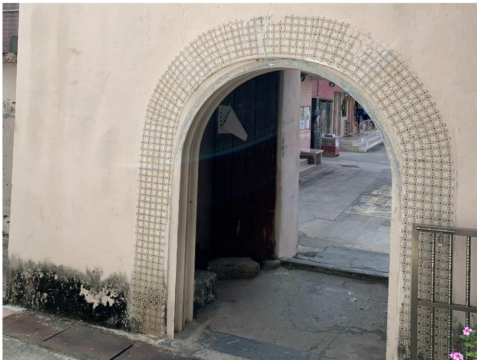
Figure 68. Internal Archway of the Entrance Gate.
