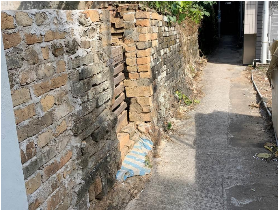
Figure 70. Southeast Enclosing Wall.
