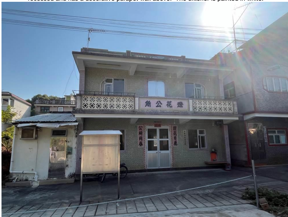
Figure 128. Village Office, Lok Ma Chau Tsuen (LMC16). The village office is a large two-storey village building. Its barrier of the balcony is formed by traditional Chinese coin pattern and has inscriptions of “燈花公所” (literally means “Candlelight Village Office”). The parapet wall on the roof is decorated by mosaic tiles and has a scenery painted on ceramic tiles in the middle, the mosaic tiles indicated the building was constructed in 1979. The front elevation is finished in ceramic tiles, while the remaining facades are finished in Shanghai plaster. Its significance in cultural heritage is noteworthy in terms of architectural and social perspective.
