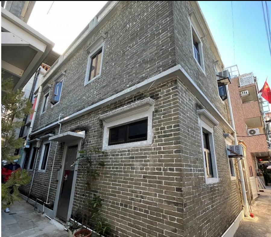
Figure 61. No. 106, Fan Tin Tsuen (FTT23), side and back elevation. All the windows have label mouldings and rendered surrounds.
