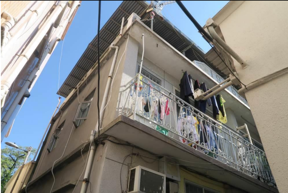
Figure 93. No. 35, Tsing Lung Tsuen (TLT05), a two-storey village house with a flat roof. The building has a high-ceiling ground floor and a balcony at the first floor. The parapet wall on the roof has inscription of “1966”. The front elevation is finished in Shanghai plaster.
