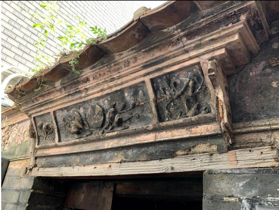
Figure 15. No. 12, Tung Chan Wai (TCW04), a traditional Chinese vernacular single-storey brick building. The building has a one-hall-one-courtyard plan. It is decorated by the plastered relief of flora motif under eaves and on door canopy.
