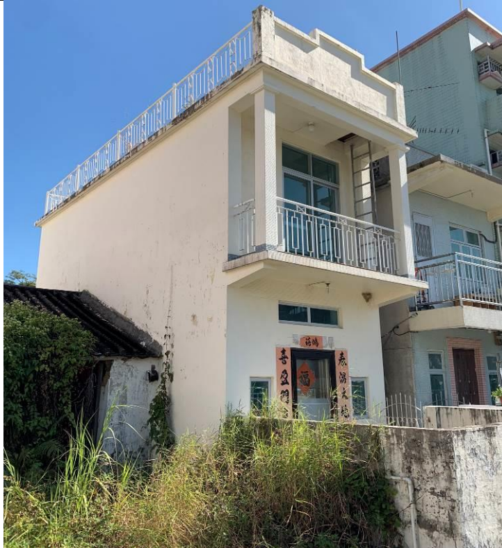
Figure 91. No. 5, Tsing Lung Tsuen (TLT02), a two-storey village house with a flat roof. The building has a high-ceiling ground floor and a balcony with two square corner columns. The building is painted in white.
