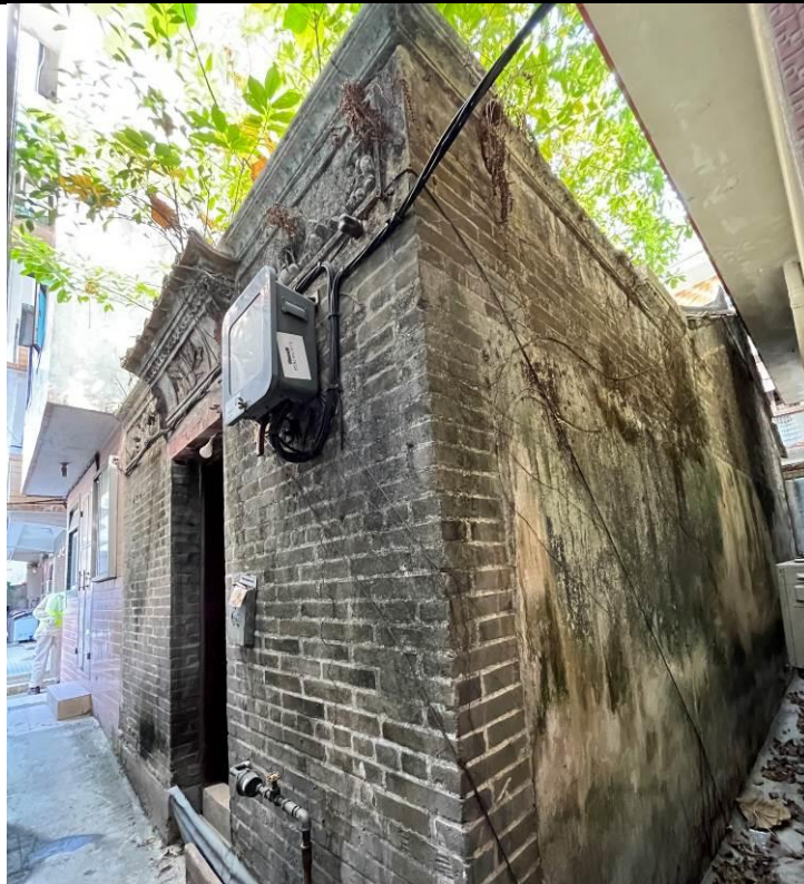
Figure 141. No. 74, Mai Po San Tsuen (MPT10), a traditional Chinese vernacular pitched-roof building. It is in a one-hall-one-courtyard plan. The building is decorated by the plastered mouldings and murals of auspicious motifs under eaves and on door canopy.
