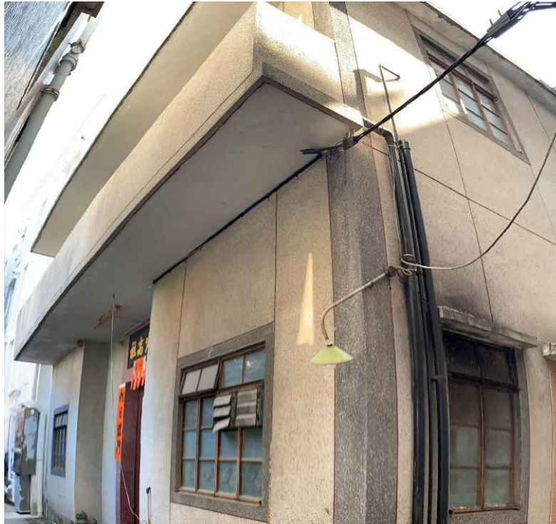
Figure 25. No. 185B, Fan Tin Tsuen (FTT03). It is a branch family ancestral hall building. It is two-storey high with a balcony on the first floor. The entrance door has a tiled-surround and a tablet with characters of “ Ding Gou Jo ” (“定高祖”) above the door. The exterior is finished in Shanghai plaster.
