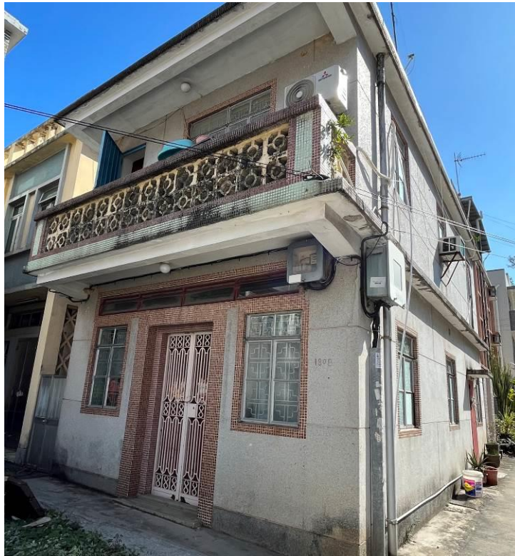
Figure 67. No. 180B, Fan Tin Tsuen (FTT31). It is a two-storey village house with a flat roof and a balcony on the first floor. The building is finished in Shanghai plaster. All the openings have decorative mosaic-tiled surrounds. The metal door gate and the window grilles are of modern geometric patterns.
