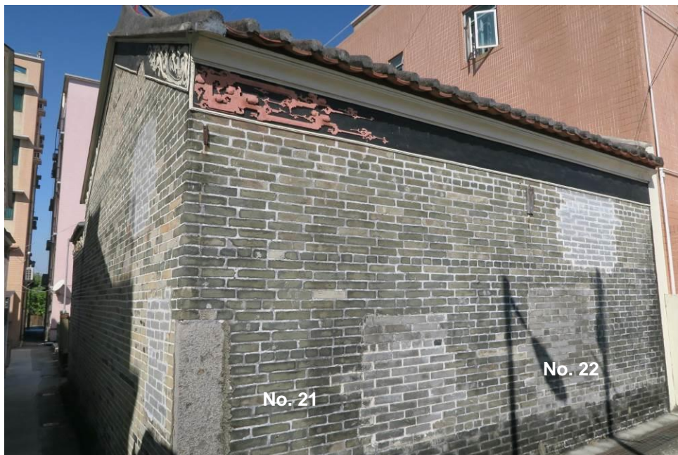
Figure 52. Back elevation (southeast façade).
