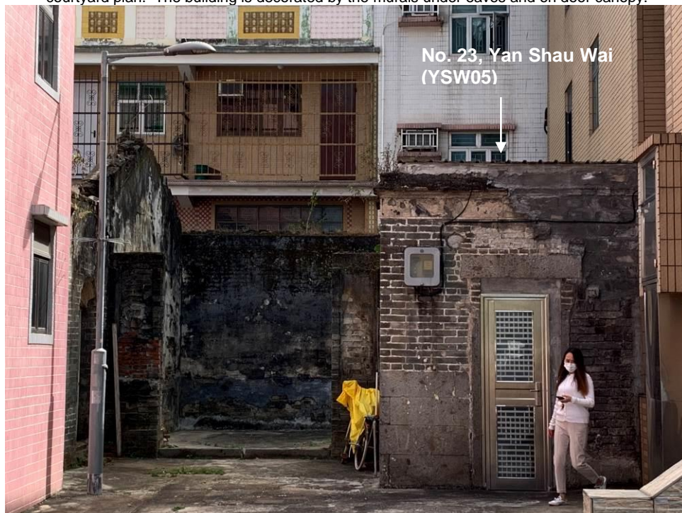
Figure 4. No. 23, Yan Shau Wai (YSW05), a traditional Chinese vernacular pitched-roof building. It is in a one-hall-one-courtyard plan. Although the building has minimal decoration, granite has been extensively used, such as the granite lintel above the entrance door, and the lower courses of the front wall. The building has experienced heavy alteration including replacement of a smaller metal front door and potentially reconstruction of the right side of front façade.
