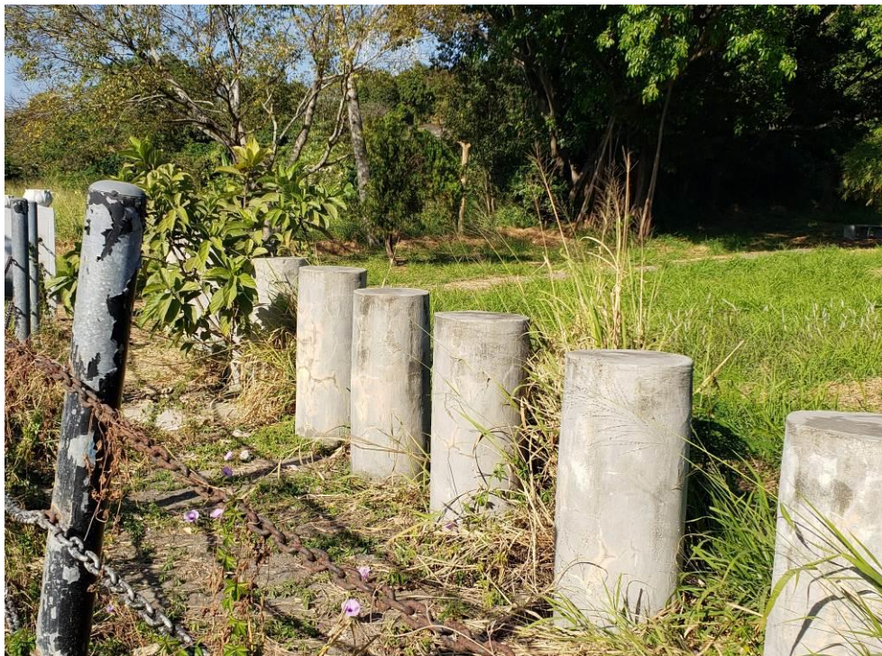
Figure 18. A row of circular concrete piles next to the road (BH07).
