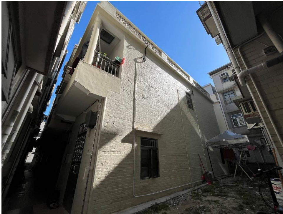
Figure 64. No. 151, Fan Tin Tsuen (FTT27). It is a two-storey village house with a flat roof. The building has a balcony with two round corner columns. The exterior of the building is painted in white. The front façade of the ground floor is finished in white tiles.
