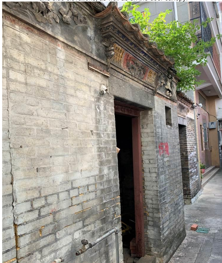
Figure 2. No. 15, Yan Shau Wai (YSW02), a traditional Chinese vernacular pitched-roof building. It is in a one-half-one-courtyard plan. The building is decorated by the plastered mouldings under eaves and the Chinese calligraphy mural on door canopy.
