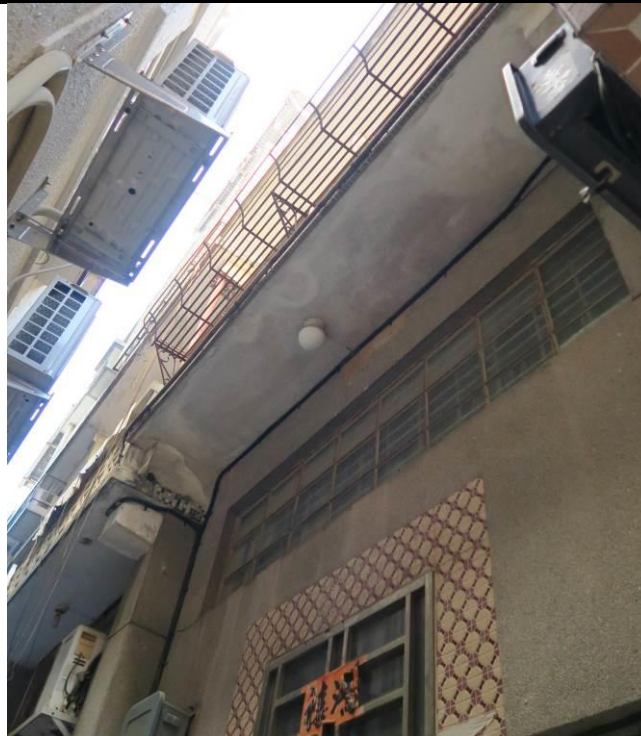
Figure 63. No. 119, Fan Tin Tsuen (FTT25). It is a two-storey village house with a flat roof. The building has a at the first floor. The exterior of the building is finished in Shanghai plaster. The entrance door has a decorative tiled surround.
