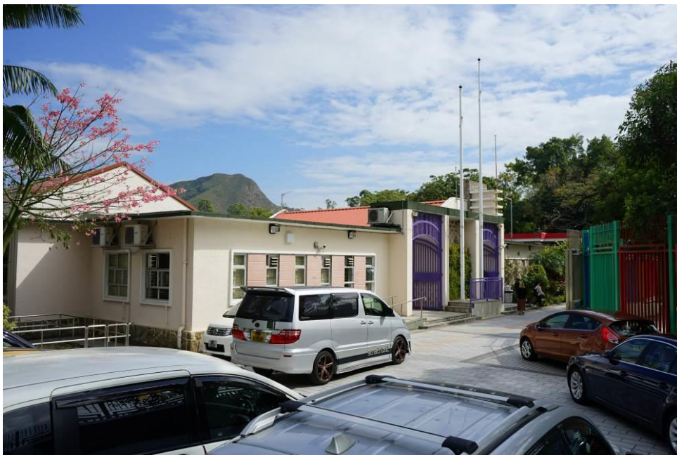
Figure 12. Southwest elevation of the main compound, comprises of two annex blocks and entrance gateway in between. Two flagpoles are erected on an elevated platform in front of the entrance gateway.
