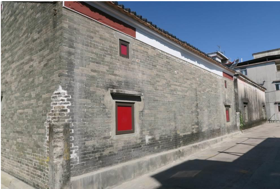
Figure 37. Back elevation (southeast façade).
