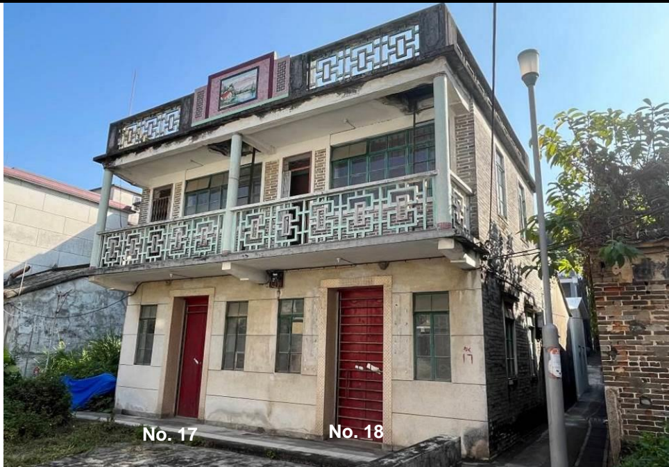
Figure 117. Nos. 17-18, Lok Ma Chau Tsuen (LMC02). It is a two-storey village brick house with two residential units. The building has a shared balcony with three round columns – two at each corner and one in the middle. The balcony has a cat ladder connected to the roof. The parapet wall on the roof has a scenery painted on ceramic tiles. The front façade of the ground floor is finished in Shanghai plaster.
