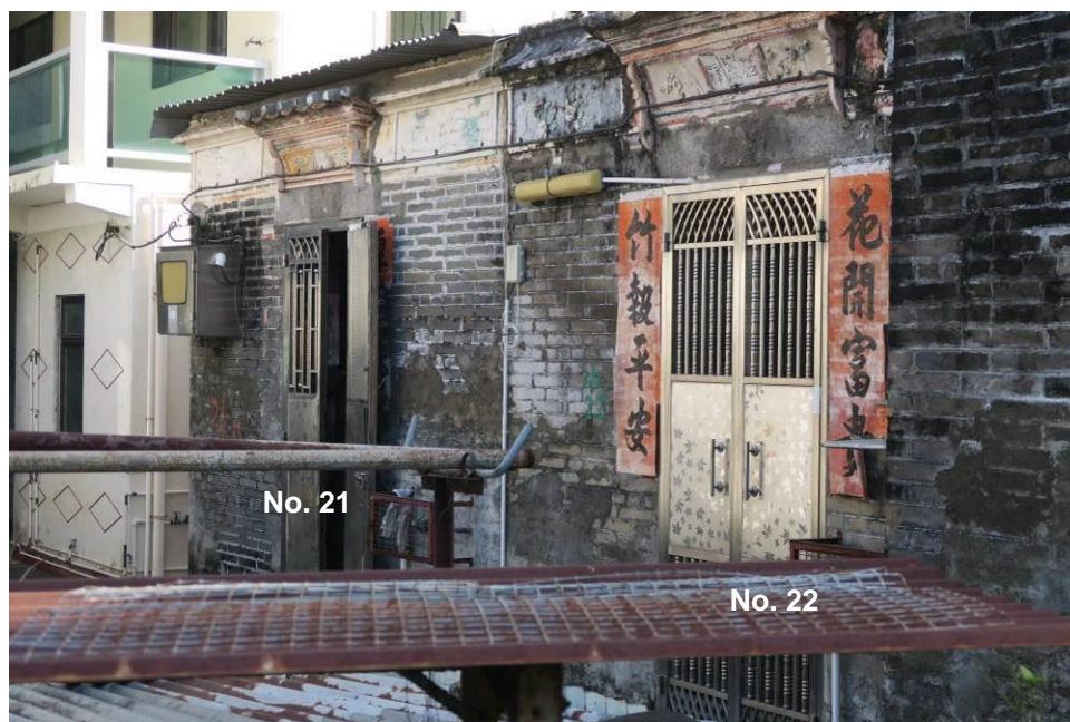
Figure 114. Nos. 21-22, Lok Ma Chau Tsuen (LMC05 and LMC06). They are traditional Chinese vernacular brick buildings in a one-hall-one-courtyard plan. No. 21 is decorated by the plastered mouldings of flowers and a coin symbol on door canopy and the murals of flora motifs on the top of the wall under eaves. No. 22 is decorated by plastered mouldings of flora and auspicious motifs on both the door canopy and top of the wall under eaves.
