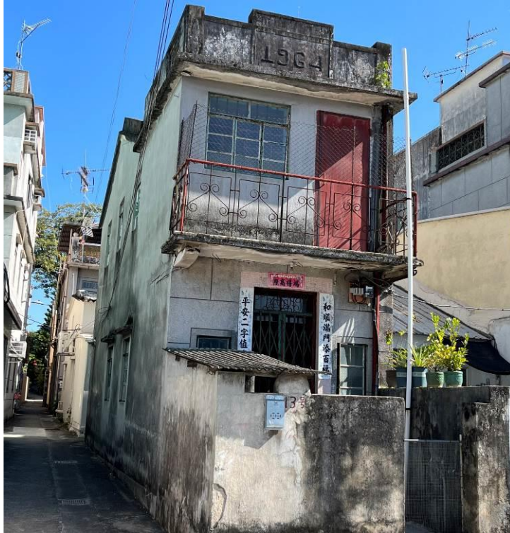
Figure 92. No. 13, Tsing Lung Tsuen (TLT03), a two-storey village house with a pitched roof. The building has a high-ceiling ground floor and a balcony on the first floor. Its parapet wall on the roof has "1964" moulded indicating the construction year. The front façade of the ground floor is finished in Shanghai plaster.
