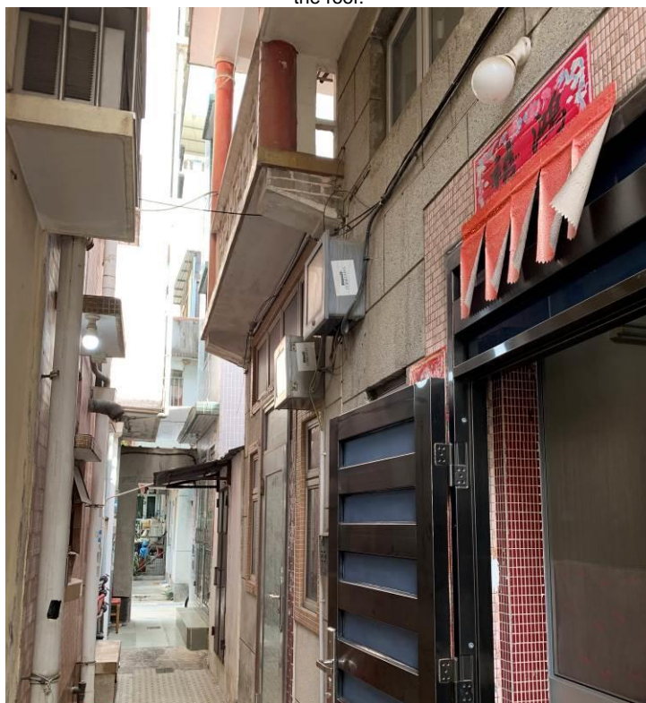
Figure 88. No. 57, On Lung Tsuen (OLT05), a two-storey village house. The building has a balcony with two red round columns at both corners. The front façade is finished in Shanghai plaster and the openings are framed by mosaic tiles.
