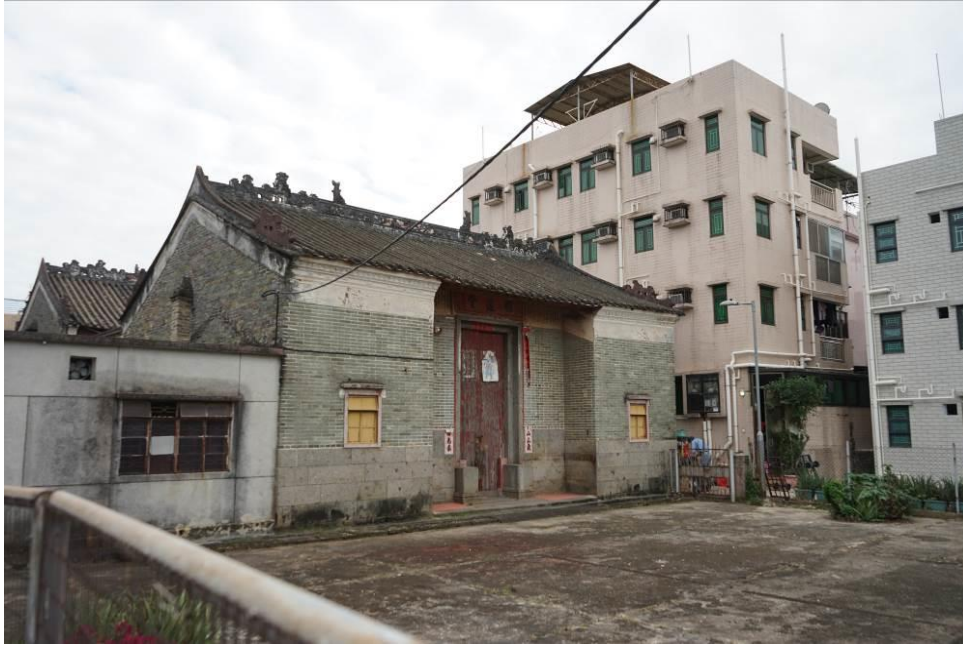
Figure 39. Front elevation (northwest façade).
