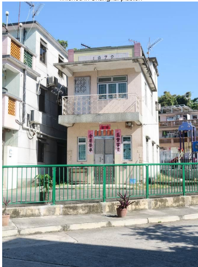
Figure 94. No. 57, Tsing Lung Tsuen (TLT06), a two-storey village house with a flat roof. The building has a balcony at the first floor with barrier of geometric patterns. The parapet wall on the roof is finished in mosaic tiles and has inscription of “1972”. The front elevation is finished in ceramic tiles.
