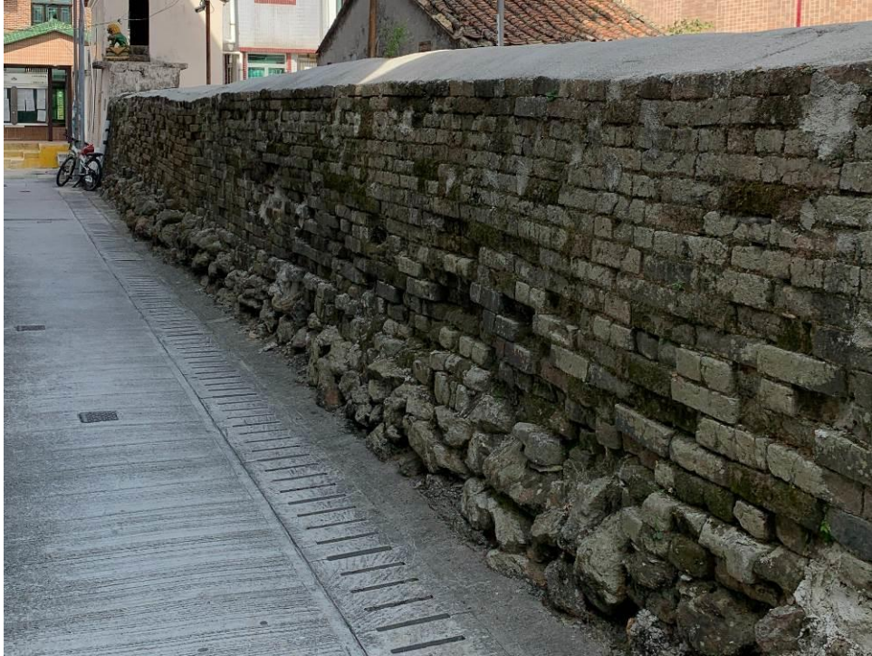
Figure 71. Southwest Enclosing Wall.
