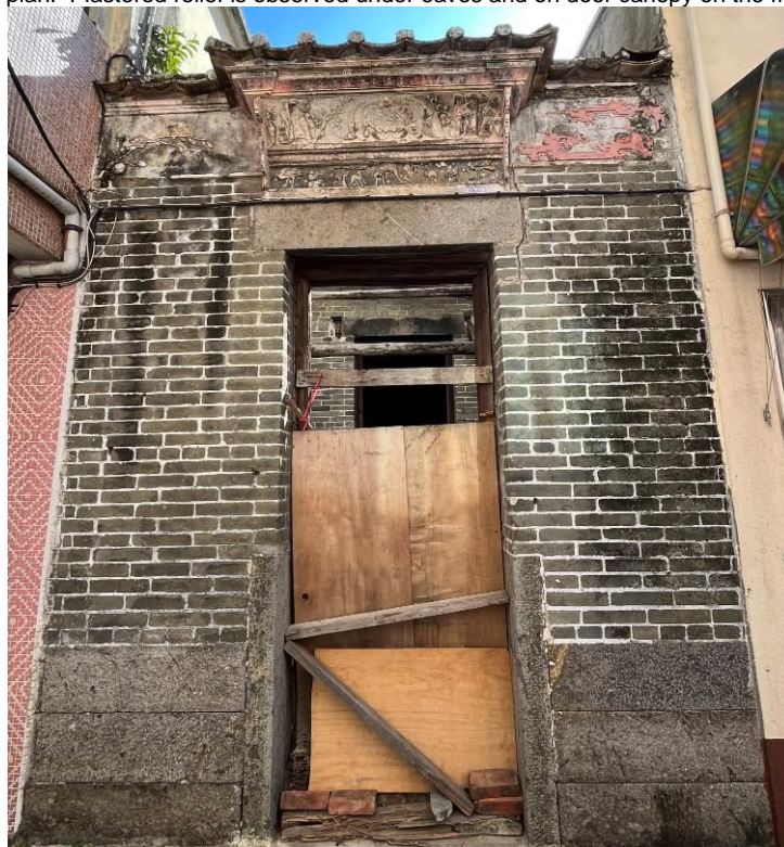
Figure 42. STL435 in Fan Tin Tsuen (FTT48), a traditional Chinese vernacular single-storey building. It is in a one-half-one-courtyard plan. Its front façade is granite-based. Plastered relief is observed under eaves and on door canopy.
