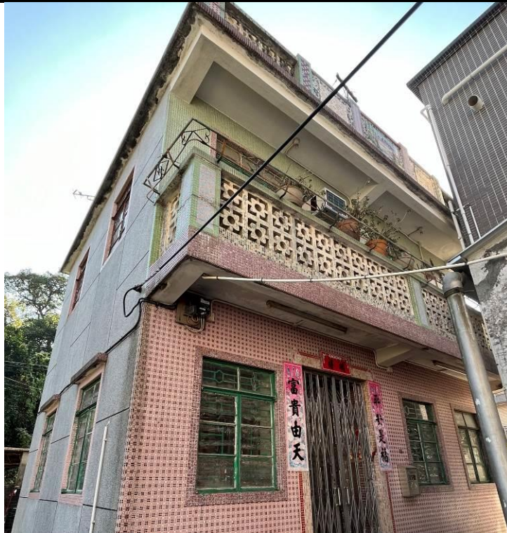
Figure 121. No. 35, Lok Ma Chau Tsuen (LMC09). It is a two-storey village house. The barrier of the balcony is formed with geometric patterns. The parapet wall on the flat roof is finished in ceramic tiles with landscape painted on tiles. The front elevation is finished in mosaic tiles while the remaining elevations are finished in Shanghai plaster. The window and door openings have mosaic-tiled surrounds.
