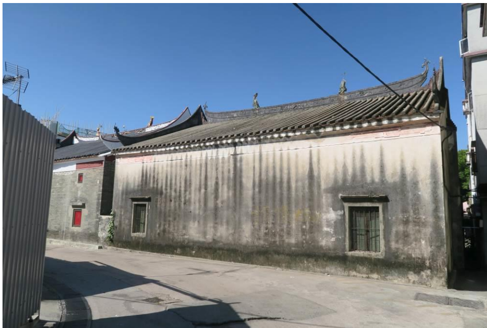
Figure 32. Back elevation (southeast façade).
