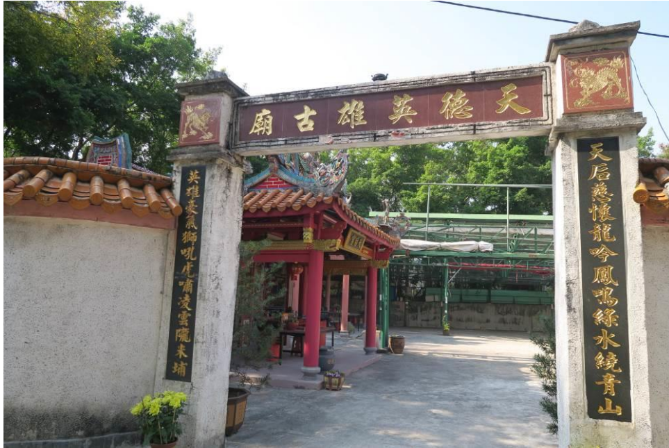
Figure 163. Entrance to the Tin Tak Heroes Temple (天德英雄古廟) (MPL01). An entrance gate is located to the east of the site. A couplet is embedded on the columns of the entrance gate.
