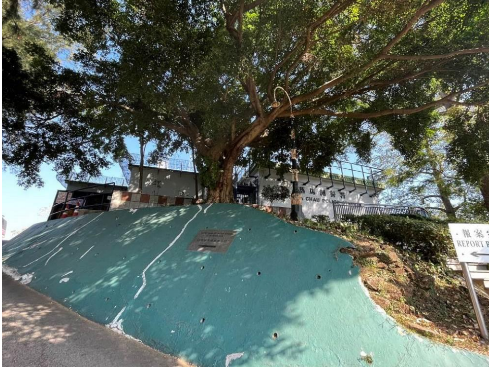
Figure 45. Back elevation and the annex block with inscriptions of “落馬洲警署 Lok Ma Chau Police Station” to the right.
