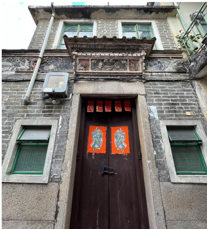
Figure 51. No. 223, Fan Tin Tsuen (FTT41). It is a traditional Chinese vernacular brick house with a granite base. It has probably undergone alteration that the new storey with a flat roof has been added to the original courtyard of the house. Plastered relief is observed under eaves and on the door canopy of the front façade of the ground floor.
