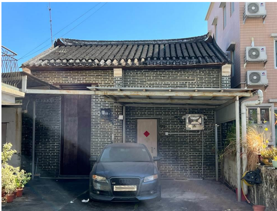
Figure 100. No. 37, San Lung Tsuen (SLT04), a traditional Chinese vernacular single-storey brick building. The building is constructed of grey bricks with its wall supporting its pitched roof. The building probably had two residential units before but one of the entrance door was filled with only the granite lintel left. Its main ridge has curled-up ends.
