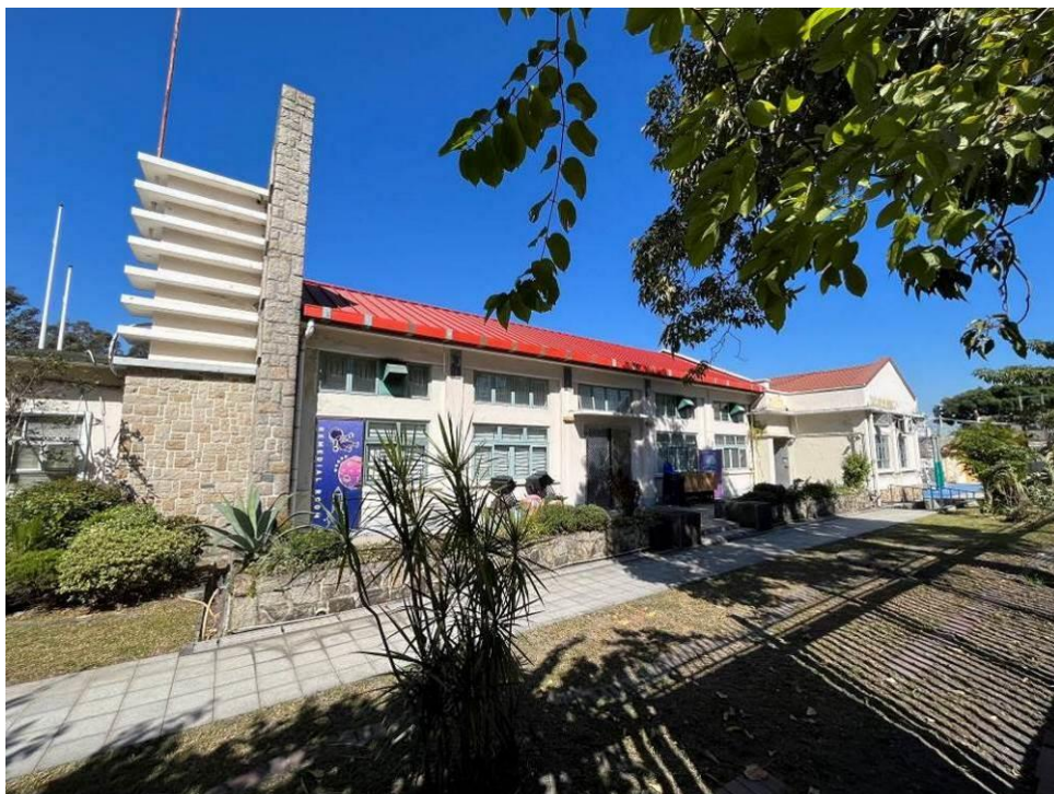
Figure 10. Southeast elevation of the main compound. The pitched-roof building is believed to be the hall of the school. It is connected to the south annex block to its left with the lighting rod (L-shaped granite wall) at the corner.
