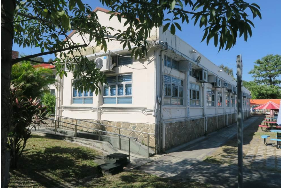
Figure 13. Northeast elevation of the main compound. The single-storey building is rectangular in plan with a red metal pitched roof and a granite base.
