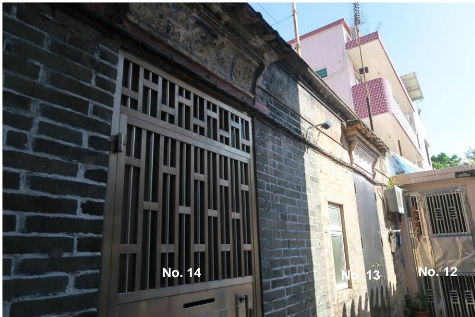
Figure 132. Nos. 12-15, Pun Uk Tsuen (PUT05, PUT06, PUT07 and PUT08). They are decorated by the murals on the decorative door canopy of each entrance door. A flat-roof annex had been added in front of the No. 12. No. 12 is painted in white while No. 13 is painted in orange. The exterior of No. 14 and No. 15 are fair-faced brick walls.
