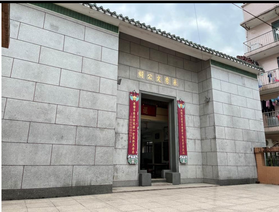
Figure 21. Ming Tak Tong (HB1355), front elevation. Ming Tak Tong Ancestral Hall is a branch ancestral hall of the Man clan. It was first built in 1811 to commemorate the 7 th generation ancestor Man Wing Sau (文永秀) and was reconstructed in 1973 13 . It is a concrete structure of Qing vernacular design having a two-hall-one-courtyard plan of three bays. The middle bay of the front façade is recessed. The ridge of its pitched roof has curled-up ends. The front elevation is finished in Shanghai plaster while other facades are plastered in pale yellow.
