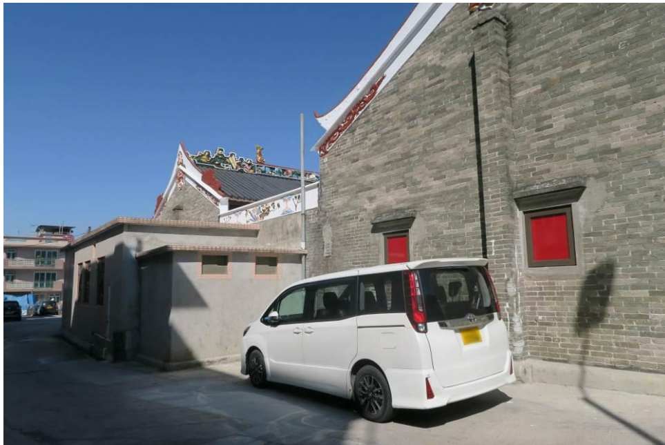
Figure 36. Side elevation (southwest façade).
