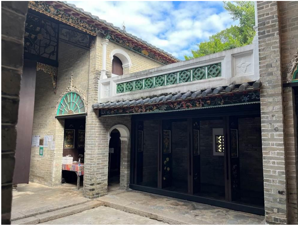
Figure 19. Eastern Side Room, Central Courtyard.
