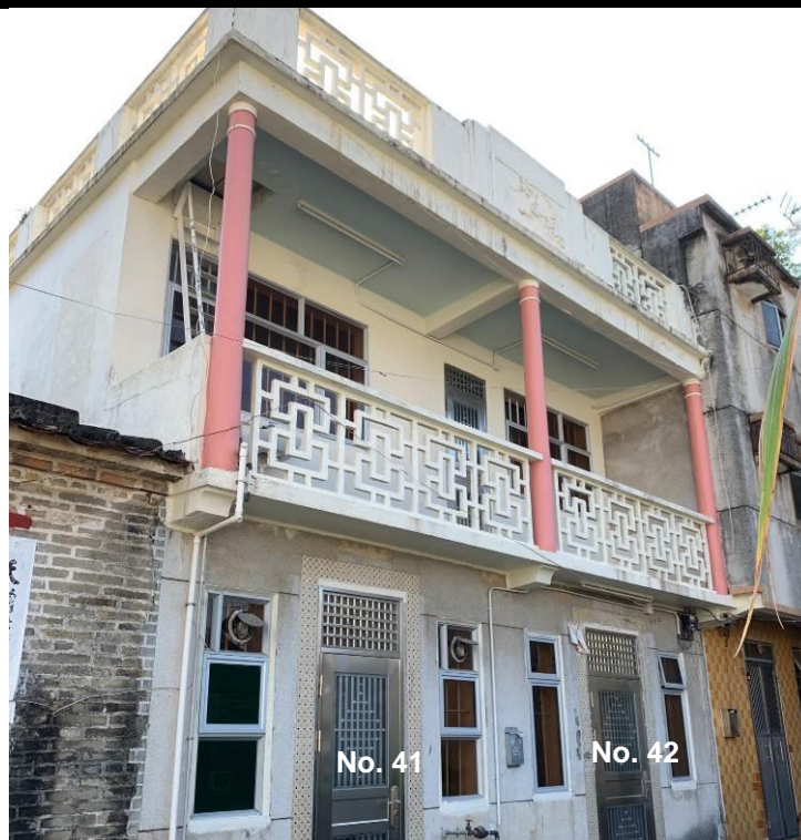
Figure 123. Nos. 41-42, Lok Ma Chau Tsuen (LMC11), a two-storey village house with two residential units. The building has a balcony with round columns at each corner and in the middle. The parapet wall on the roof has plastered relief of flower and bird motifs. The front façade of the ground floor is finished in Shanghai plaster, the door openings are decorated with mosaic-tiled surround.
