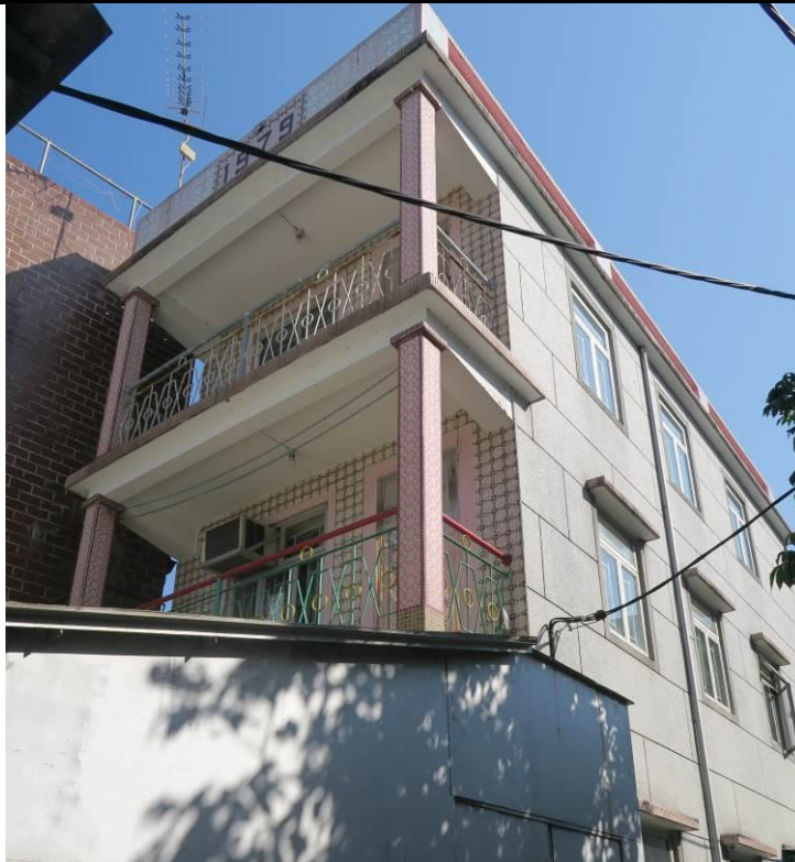
Figure 145. No. 4, Mai Po San Tsuen (MPT04), a three-storey village house with a flat roof. The building has a balcony with two square corner columns decorated with mosaic tiles at the second and the third storey. The parapet wall on the roof has a “1979” pattern formed by mosaic tiles. The front façade is finished in ceramic tiles and the other facades are finished in Shanghai plaster.
