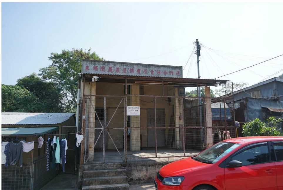
Figure 171. Mai Po Lung Vegetable Marketing Co-operative Society, Ltd (MPL02). Built on an elevated platform, this building is a single-story building with a pitched roof. Its front porch is sheltered covered by corrugated sheets. The building is Utilitarian in style. A signboard with Chinese characters of Mai Po Lung Vegetable Marketing Co-operative Society (“米埔隴蔬菜產銷有限責任合作社”) (literally Mai Po Lung Vegetable Marketing Co-operative Society ) is placed on the roof. Simple staircase is attached to the front of the platform providing access.
