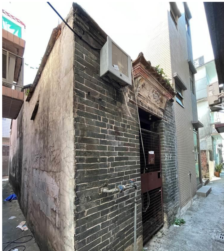
Figure 90. No. 23, Tsing Lung Tsuen (TLT04), a traditional Chinese vernacular single-storey brick building. The building has a one-hall-one-courtyard plan. It is decorated by the plastered relief of flora motif on the door canopy.
