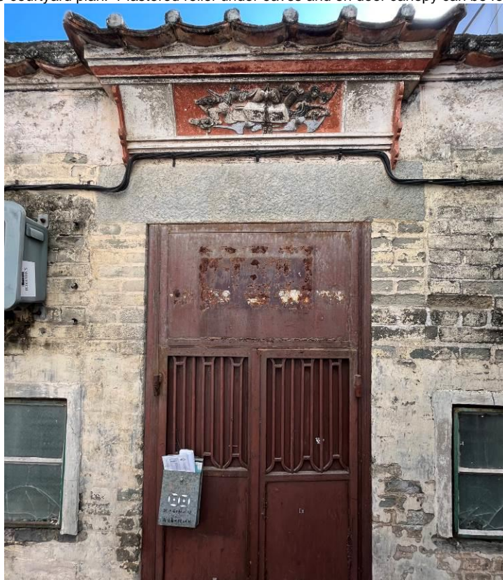
Figure 32. No. 26, Fan Tin Tsuen (FTT10), a traditional Chinese vernacular single-storey house. Plastered relief can be found on door canopy.
