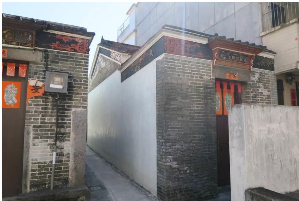
Figure 99. No. 20, San Lung Tsuen (SLT03), a traditional Chinese vernacular single-storey brick building. The building has a one-half-one-courtyard plan. It is decorated by the plastered relief of auspicious motif on the door canopy. A wall frieze is running on the front and side façade of the building with plastered mouldings of ruilong (夔龍) and other patterns. Its flat main ridge on the pitched roof has curled-up ends. The side façade of the building is painted in white. The building is similar architectural style as No. 21 and No. 22 nearby (grade 3 historic buildings).
