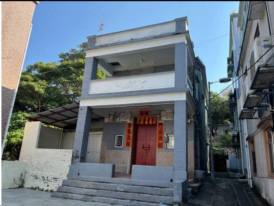
Figure 125. No. 51, Lok Ma Chau Tsuen (LMC14). The two-storey building is a traditional Chinese vernacular architecture with a pitched roof and a verandah in front supported by two columns below. The building is constructed of grey bricks. The base of the front façade is finished with granite plates. The parapet wall on the verandah has plastered relief of auspicious motifs. All the window openings on the side elevations have label mouldings and rendered surrounds. The brick surface on the front façade is painted in blue violet colour.
