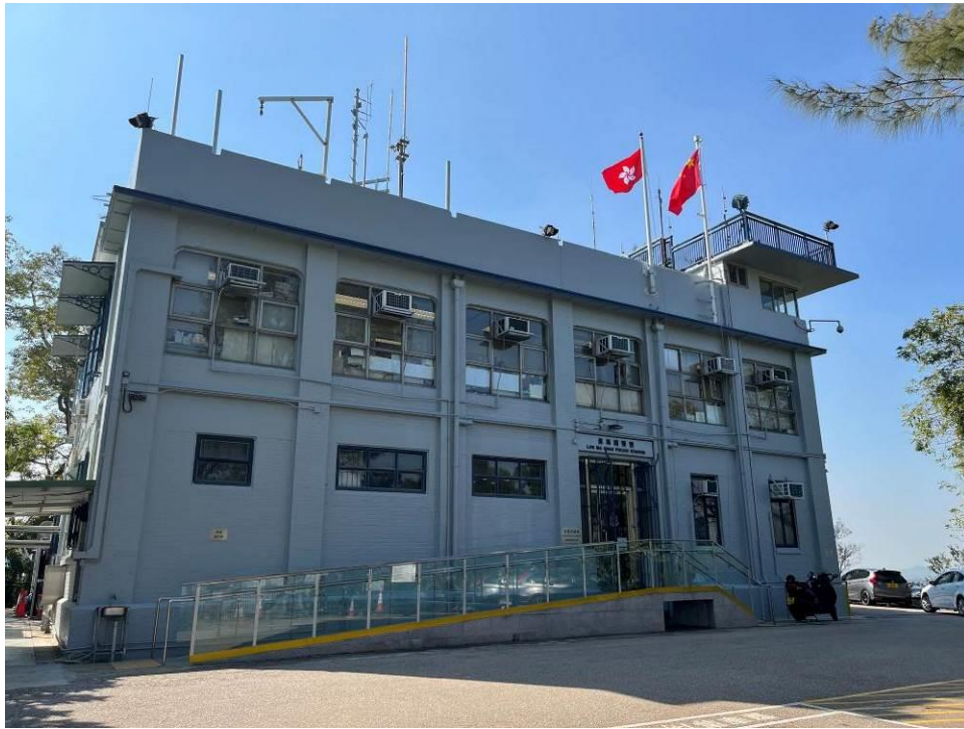
Figure 43. Front elevation, the original verandahs had been enclosed. The roof has been altered into flat roof and added with an additional storey.
