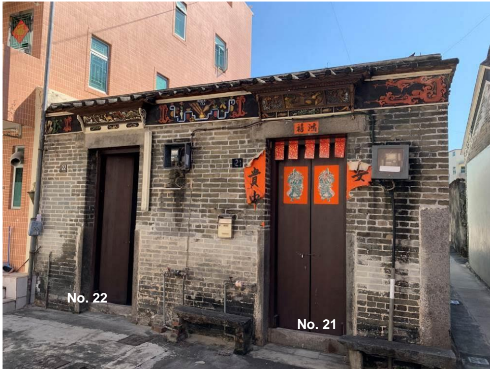
Figure 51. Front elevation (northwest façade).
