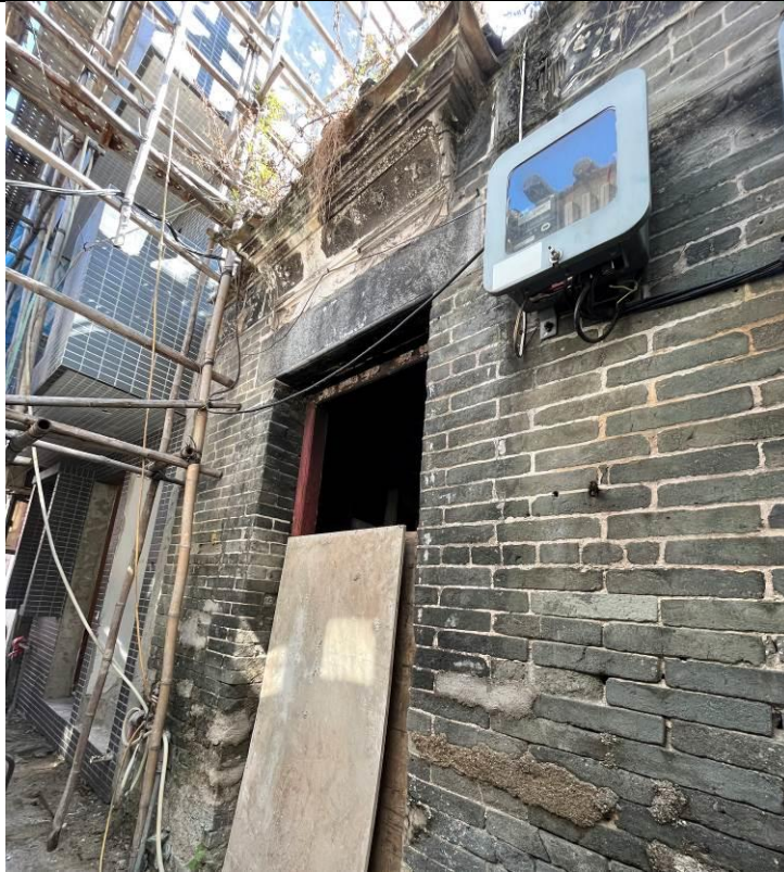
Figure 53. No. 91, Fan Tin Tsuen (FTT46), a traditional Chinese vernacular single-storey house with a one-hall-one-courtyard layout. Plastered relief can be found under eaves and on door canopy.
