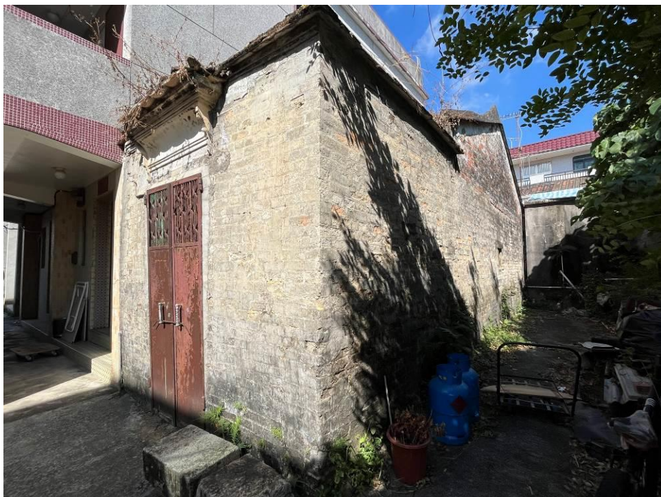
Figure 133. No. 26, Pun Uk Tsuen (PUT09), a traditional Chinese vernacular brick house in a one-hall-one-courtyard plan. The building is decorated by the murals on the decorative door canopy but the colours are fading.
