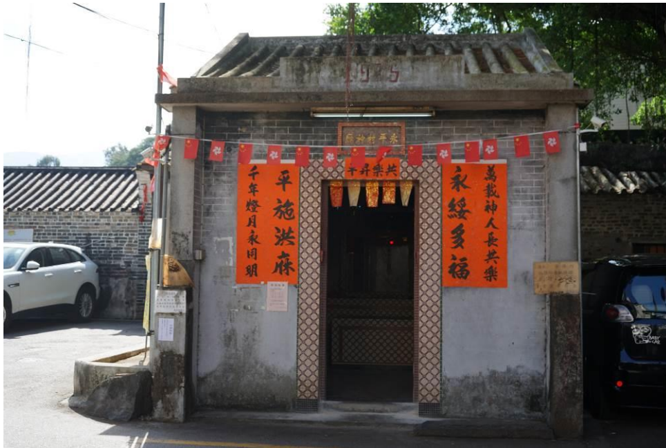
Figure 77. Hall of Gods, Wing Ping Tsuen (WPT02), a Chinese vernacular pitched roof building in a one-bay plan. The front façade has drawn brick lines while the remaining walls are plastered. The entrance door has a mosaic-tiled surround. The parapet wall on the roof has inscription of “1975”. Its significance in cultural heritage is noteworthy in terms of cultural perspective.
