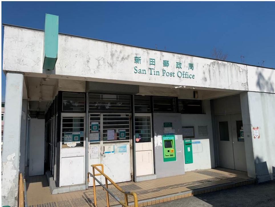
Figure 5. Main entrance to San Tin Post Office.
