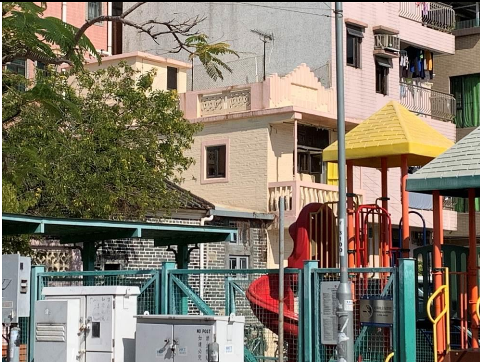
Figure 19. No. 8, Tung Chan Wai (TWC03), a two-storey village house with a flat roof. The building has a balcony with two thin corner columns. The parapet wall on the roof has "1962" inscribed indicating the construction year. The building is painted in pale yellow and pink.
