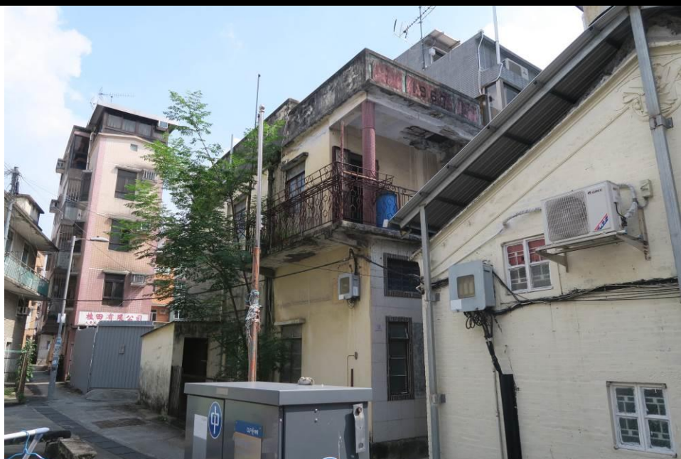
Figure 69. No. 206A, Fan Tin Tsuen (FTT34). It is a two-storey village house with a flat roof. It has a balcony on the first floor extending from the front elevation to the side elevation, with two circular columns at front. The exterior is plastered except the front elevation of the ground floor which is finished in Shanghai plaster. The parapet wall on the roof indicated it was built in 1967. Spalling concrete with the metal rebar exposed is observed on the ceiling of the balcony.
