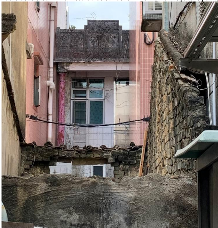
Figure 12. No. 92, Yan Shau Wai (YSW11), a two-storey village house with a flat roof. The building has a balcony with two red round columns at both corners and a parapet wall on the roof. The front façade is painted in pink. The openings at the first floor have been installed with modern aluminium windows and door.
