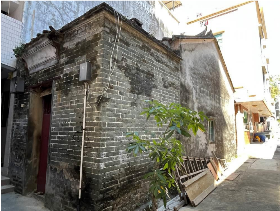
Figure 103. No. 55, Chau Tau Tsuen (CTT04), a single-storey brick house in a one-hall-one-courtyard plan. The building has a pitched roof and its main ridge has curled-up ends. The building has a decorative door canopy.
