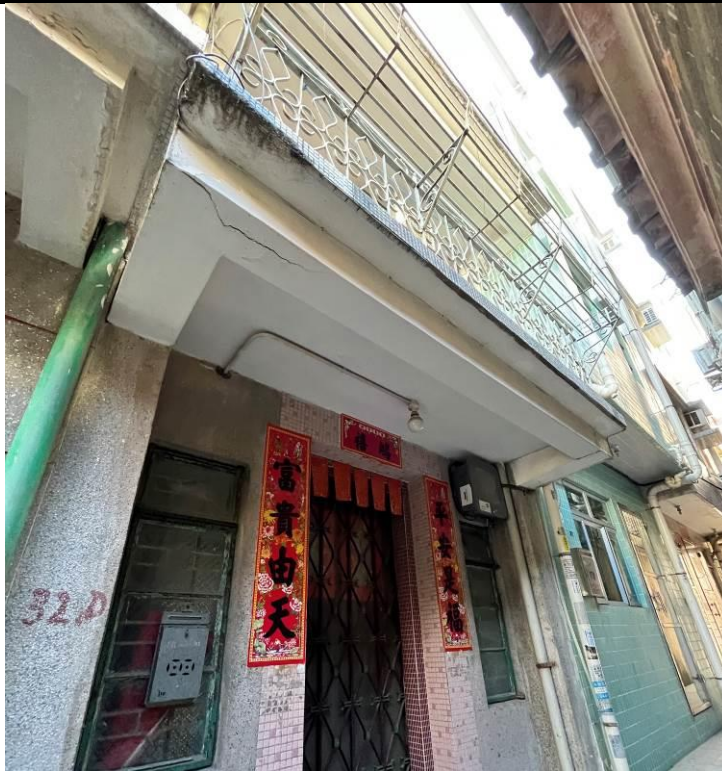
Figure 57. No. 32D, Fan Tin Tsuen (FTT13). It is a two-storey village house with a flat roof. The building has a high-ceiling first floor and a balcony on first floor. The entrance door has a decorative tiled surround. The front elevation is finished with Shanghai plaster. The metal door gate and the barrier of the balcony are of modern geometric patterns.
