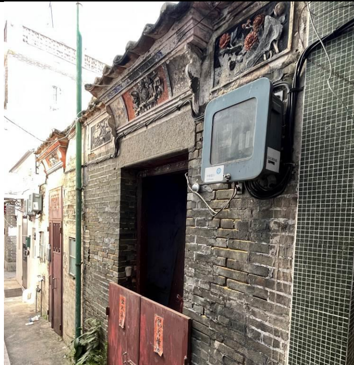
Figure 33. No. 27, Fan Tin Tsuen (FTT11), a traditional Chinese vernacular single-storey house. Plastered relief can be found under eaves and on door canopy.
