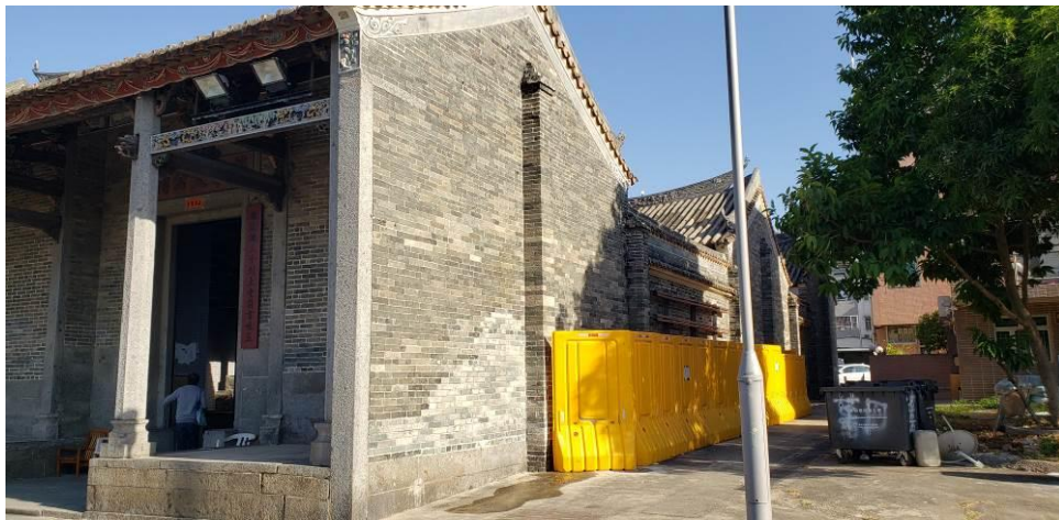
Figure 2. Side elevation (southwest façade).
