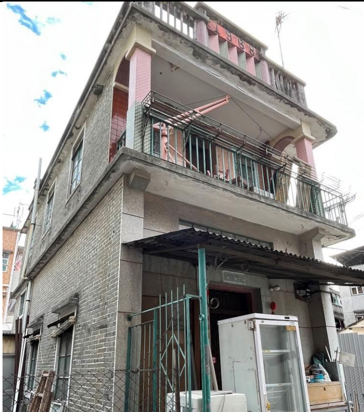
Figure 75. No. 239A1, Fan Tin Tsuen (FTT45). The parapet wall on the roof has “1968” inscribed indicating the construction year. The front façade of the building is finished in Shanghai plaster and ceramic tiles, while the remaining façade is fair-faced brick wall.
