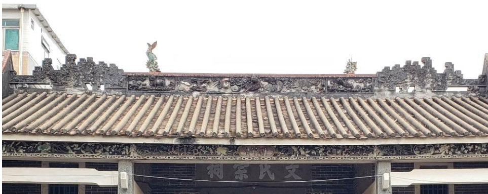
Figure 34. Main ridge details.
