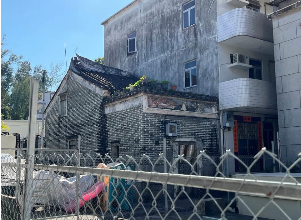
Figure 35. No. 77, Fan Tin Tsuen (FTT16). It is a traditional Chinese vernacular pitched roof brick house. It is in a one-hall-one-courtyard plan. Main roof ridge has curled-up end. The building is decorated by plastered relief under eaves.
