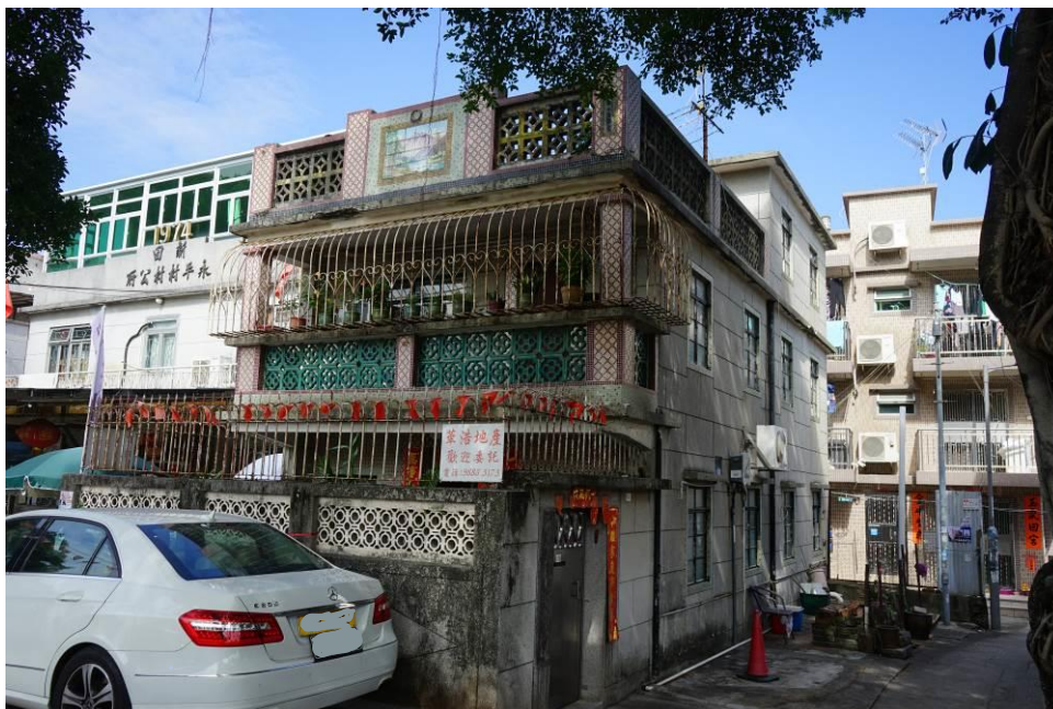
Figure 82. No. 102, Wing Ping Tsuen (WPT05), a two-storey village house with a flat roof. The building has a balcony with two corner columns decorated with mosaic tiles. The exterior is finished in Shanghai plaster. This parapet wall on the roof is decorated with mosaic tiles and a scenery painted on ceramic tiles.
