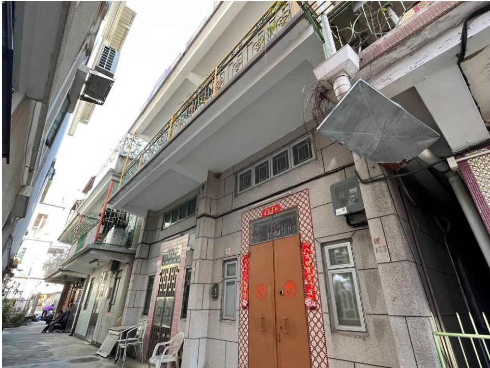
Figure 155. Nos. 122-123, Mai Po San Tsuen (MPT16), a two-storey village house with two residential units. The building has a high-ceiling ground floor and a shared balcony with thin round corner columns. The front façade of the ground floor is finished in Shanghai plaster.
