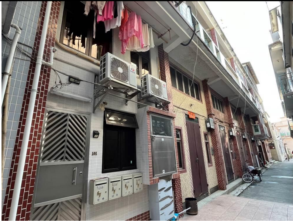
Figure 153. Nos. 101-108, Mai Po San Tsuen (MPT14), a row of two-storey village houses. These buildings have high-ceiling ground floor and a connected balcony with square columns defining each unit. The front façades are finished in ceramic tiles. It is speculated this row of houses were constructed at once.
