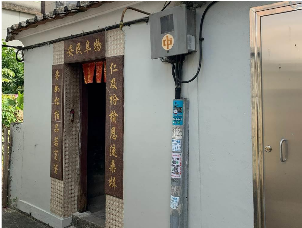
Figure 73. Front Elevation of the Shrine (Northwest façade).
