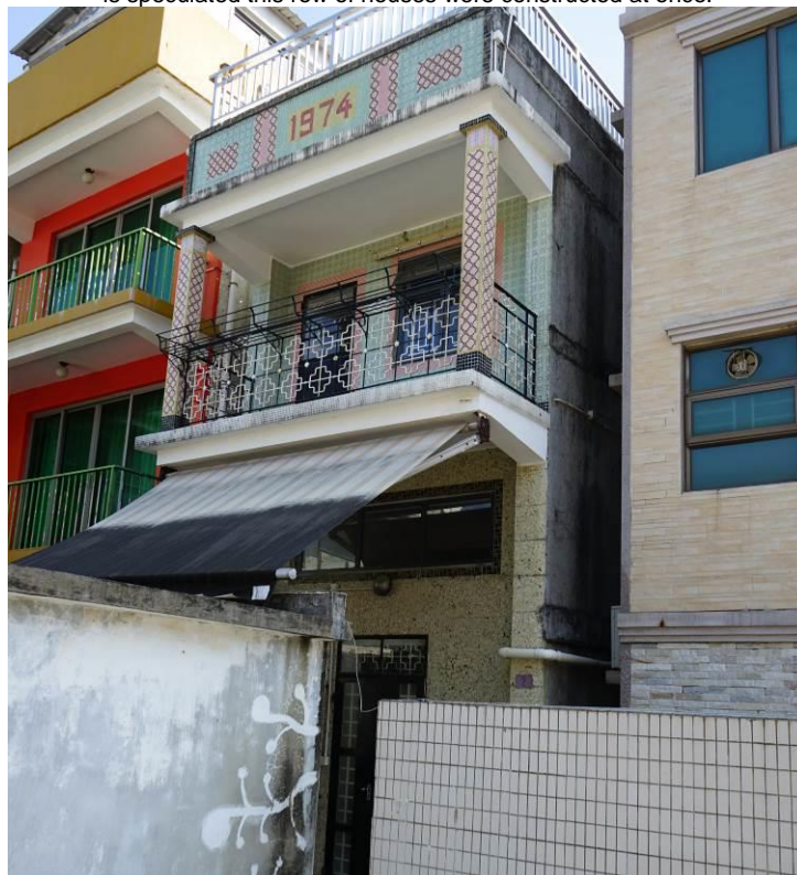
Figure 154. No. 117, Mai Po San Tsuen (MPT15), a two-storey village house with a flat roof. The building has a high-ceiling ground floor and a balcony with two square corner columns. The parapet wall on the roof has a “1974” pattern created with mosaic tiles. The front façade of the ground floor is finished in terrazzo while the first floor is finished in ceramic tiles.
