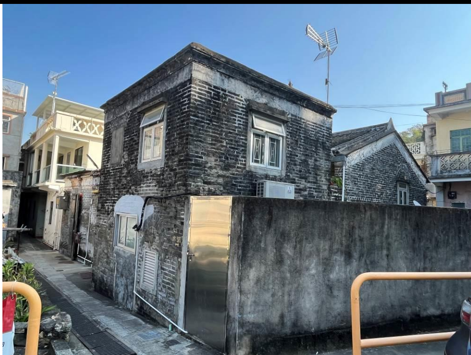
Figure 115. No. 23, Lok Ma Chau Tsuen (LMC07). The building had probably undergone alteration works, the traditional pitched-roof brick hall is retained at the back while the original front courtyard has been reconstructed into a two-storey brick building with a flat roof. Some of the openings have arched brick lintels.
