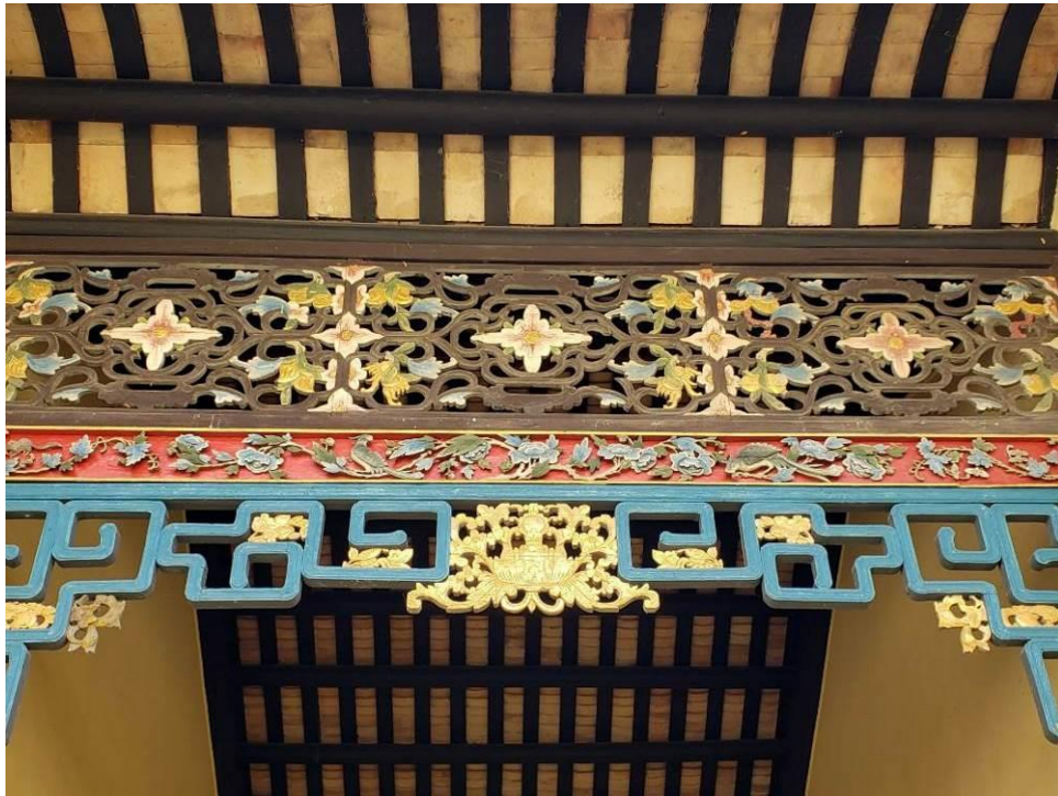
Figure 25. Decorative Timber Surround of Parlour, East Annex.
