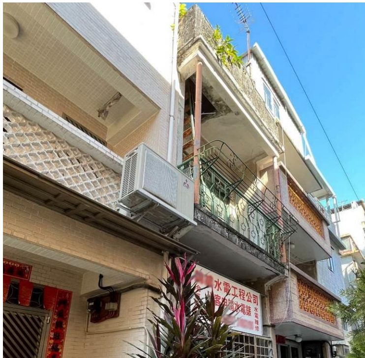
Figure 66. No. 168A, Fan Tin Tsuen (FTT29). It is a two-storey village house with a flat roof. The building has a balcony with two red thin round columns at both corners. The parapet wall on the roof has “1966” inscribed indicating the construction year.
