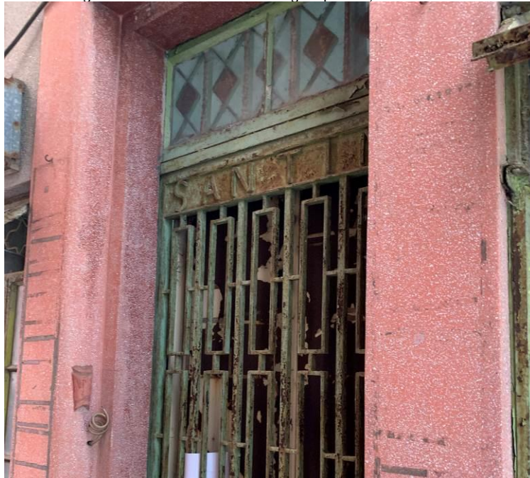
Figure 10. No. 64, Yan Shau Wai (YSW08). The entrance door has a red terrazzo surround and a green metal gate with modern geometric patterns and inscription of "SANTIN".
