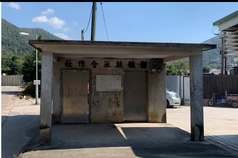
Figure 177. Subsidiary station of San Yau Vegetable Marketing Co-operative Society, Ltd. The San Yau Vegetable Marketing Co. Soc. Ltd. (新墟蔬菜產銷有限責任合作社) was established on 18th November, 1953 45 . This subsidiary station was first appeared in 1963 46 as a single-storey building with a sheltered front porch. The existing structure was probably rebuilt in the mid 1970s 47 . Constructed of reinforced concrete, it is a single-storey building with a flat roof and a covered front porch.
