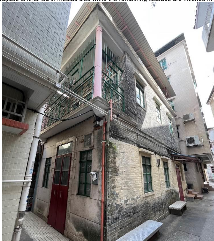
Figure 86. No. 52A1, On Lung Tsuen (OLT03), a two-storey village house with a flat roof. The building has a balcony with two round corner columns on its front façade and a staircase connected to the roof. The front façade of the ground floor is finished in Shanghai plaster while the remaining façades are generally fair-faced brick walls.
