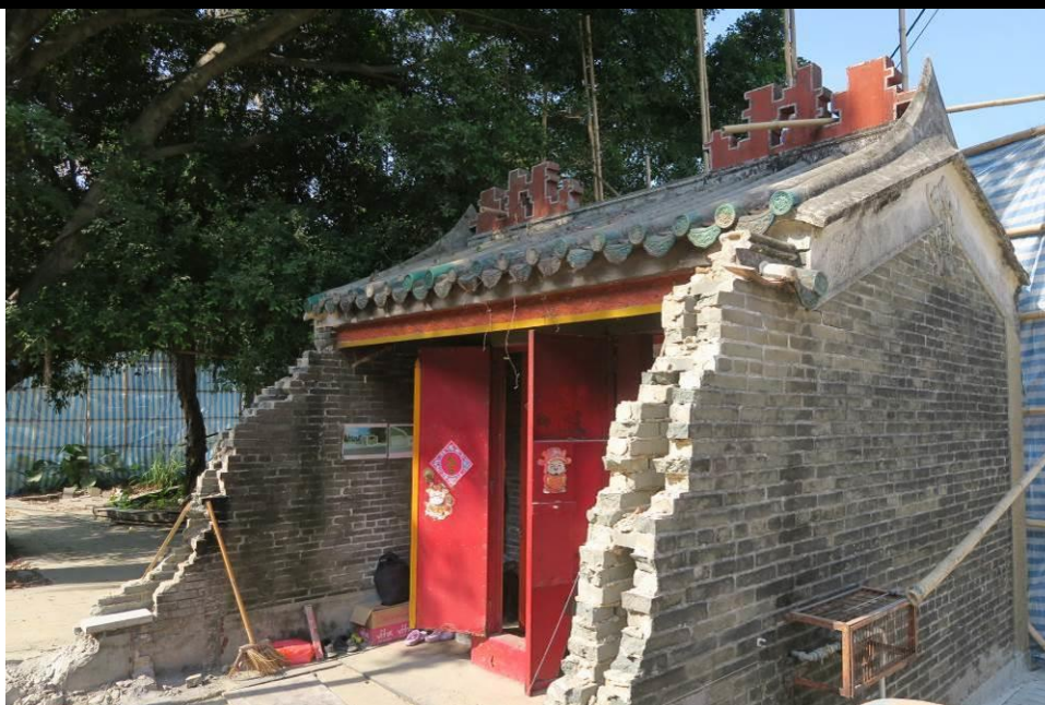
Figure 139. Yeung Hau Temple (San Tin) (MPT01) next to Castle Peak Road. It was probably erected over 200 years ago for fung shui reasons and had renovated or reconstructed in 1858, 1902, 1954 and 1969. 32 It was originally a traditional Chinese brick building in a two-hall-one-courtyard plan of one bay. The building was undergoing reconstruction during visit. The front hall still existed during visit, it has a pitched roof with a flat main ridge. A screen door is located in the middle of the first hall.
