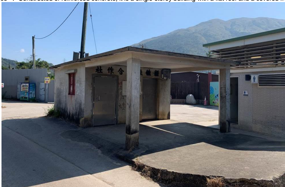
Figure 178. Side elevation of the subsidiary station. The building is Utilitarian in style with no decoration. The significance in cultural heritage of the station is embodied in historical perspective. Together with other Vegetable Marketing Co-operative Societies in Hong Kong, these venues are a testimony of the government's effort in improving the agricultural industry, as well as the agricultural cooperative movement within farmers in the New Territories in the latter half of the 20th century. The erection of a subsidiary station reflects the thriving vegetable farming in Ngau Tam Mei area.
