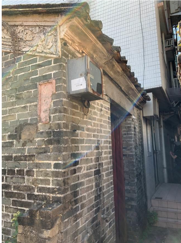
Figure 16. No. 43A, Tung Chan Wai (TCW06), a traditional Chinese vernacular single-storey brick building. It is decorated by the plastered relief of flora motif under eaves on its side elevation.
