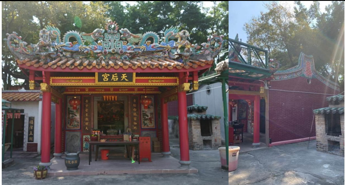
Figure 167. Front façade (left) and side façade (right) of the Tin Hau Temple. The building is a one-hall concrete structure with a front porch. It has a pair of polygonal gable wall which is probably of “fire” nature in wuxing (五行火屬). The building is richly decorated with paintings, sculptures and patterns of folklores and auspicious motifs. The front porch of the Temple was added in 2003. 39 It is believed the existing temple is a reconstruction.
