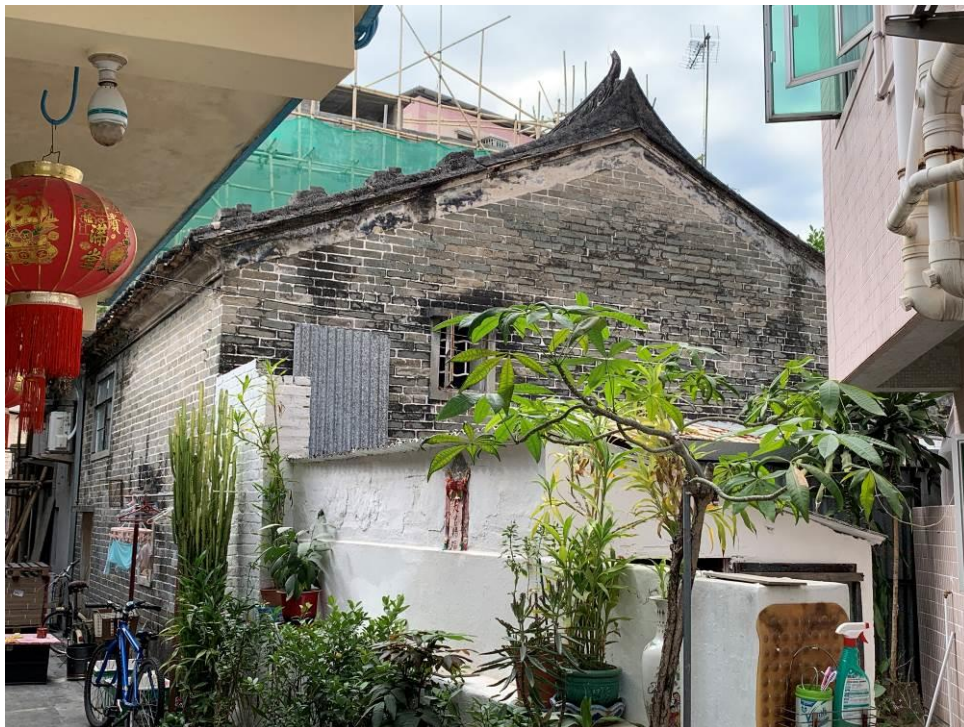
Figure 47. Nos. 220-221 Fan Tin Tsuen (FTT36 and FTT37), side elevation. It is a pitched-roof building. Its main ridge has curled-up ends.
