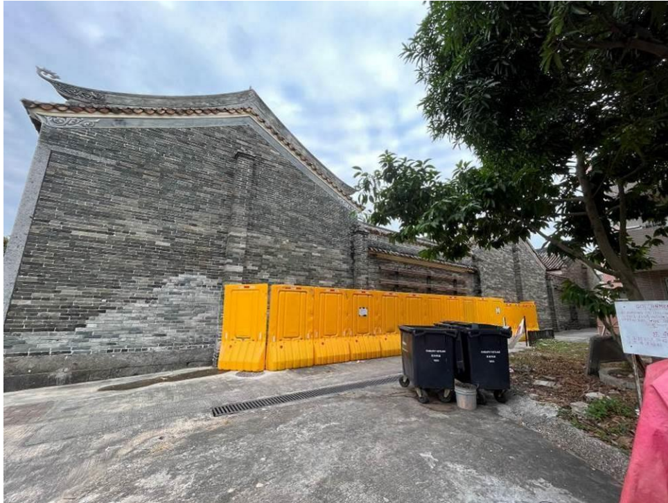
Figure 3. Side elevation (northeast façade).
