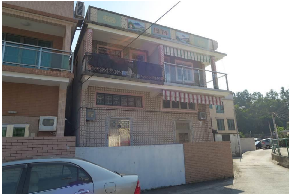
Figure 157. No. 127-128, Mai Po San Tsuen (MPT18), a two-storey village house with two residential units. The building has a high-ceiling ground floor and a balcony with square columns defining each unit. The parapet wall on the roof has a “1974” pattern created by mosaic tiles, it also has scenery painted on ceramic tiles which could be the culture of people originated from Fujian (鶴佬) according to the village elders. The front façades are finished in ceramic tiles.
