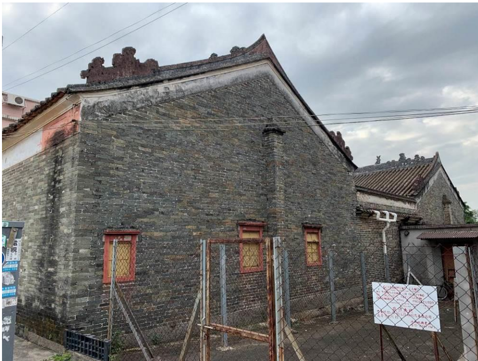
Figure 40. Side elevation (northeast façade).
