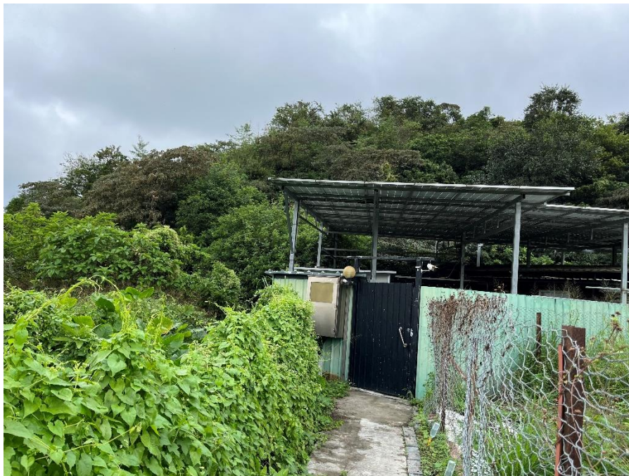
Photo A7.4 Footpath to Field Scanning Area A7 was blocked by temporary structure.
