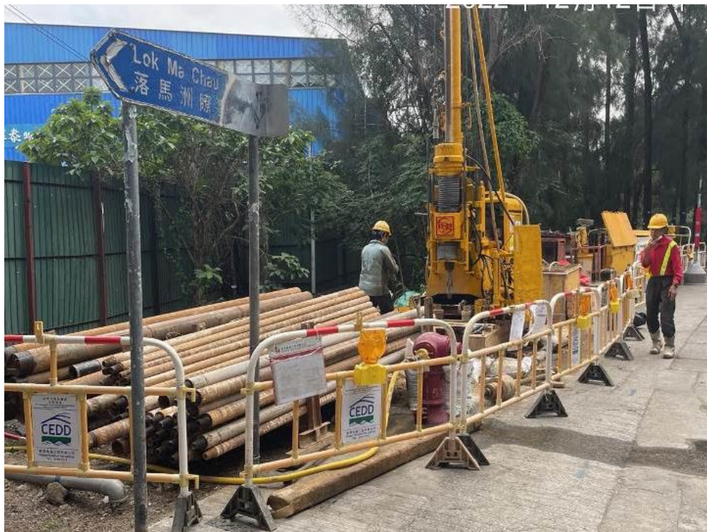
Photo 2: Drill Rig setup at EDH06
