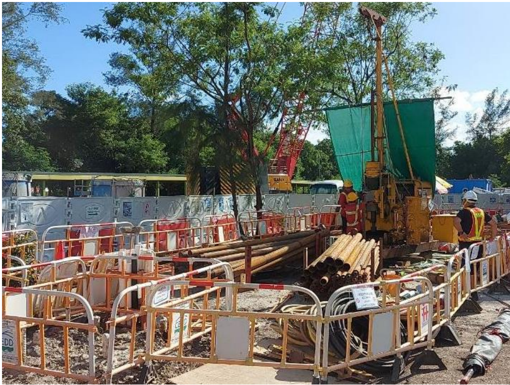
Photo 1: Drill Rig setup at EDH04
