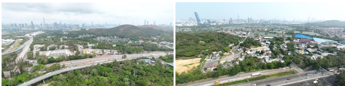
Northern Project Area at the north of San Tin Highway and Fanling Highway
