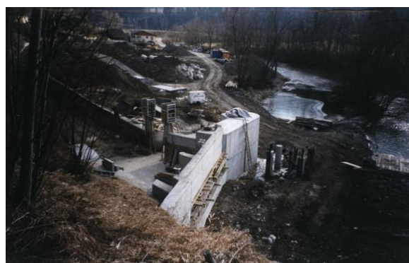
Construction of Hydropower plant in Austria 355
