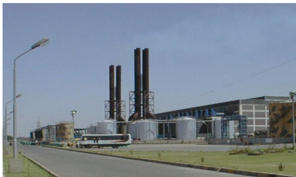
Kohinoor Energy Power Project 106
