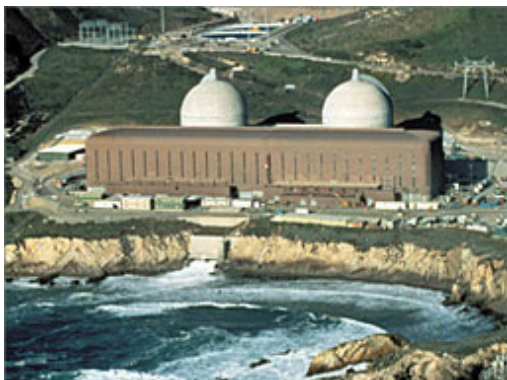
Nuclear power plant 168
