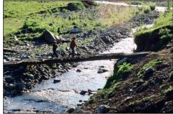
Improvement of Flood Protection in Azerbaijan 374
