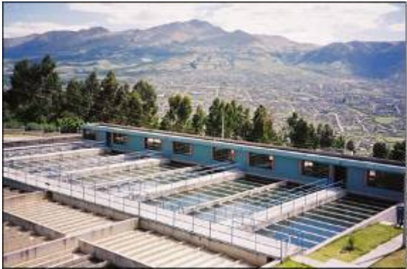
A new treatment plant in Southern Quito 390
