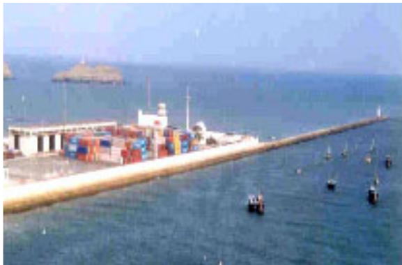
Pakistan Deep Water Container Port 89
