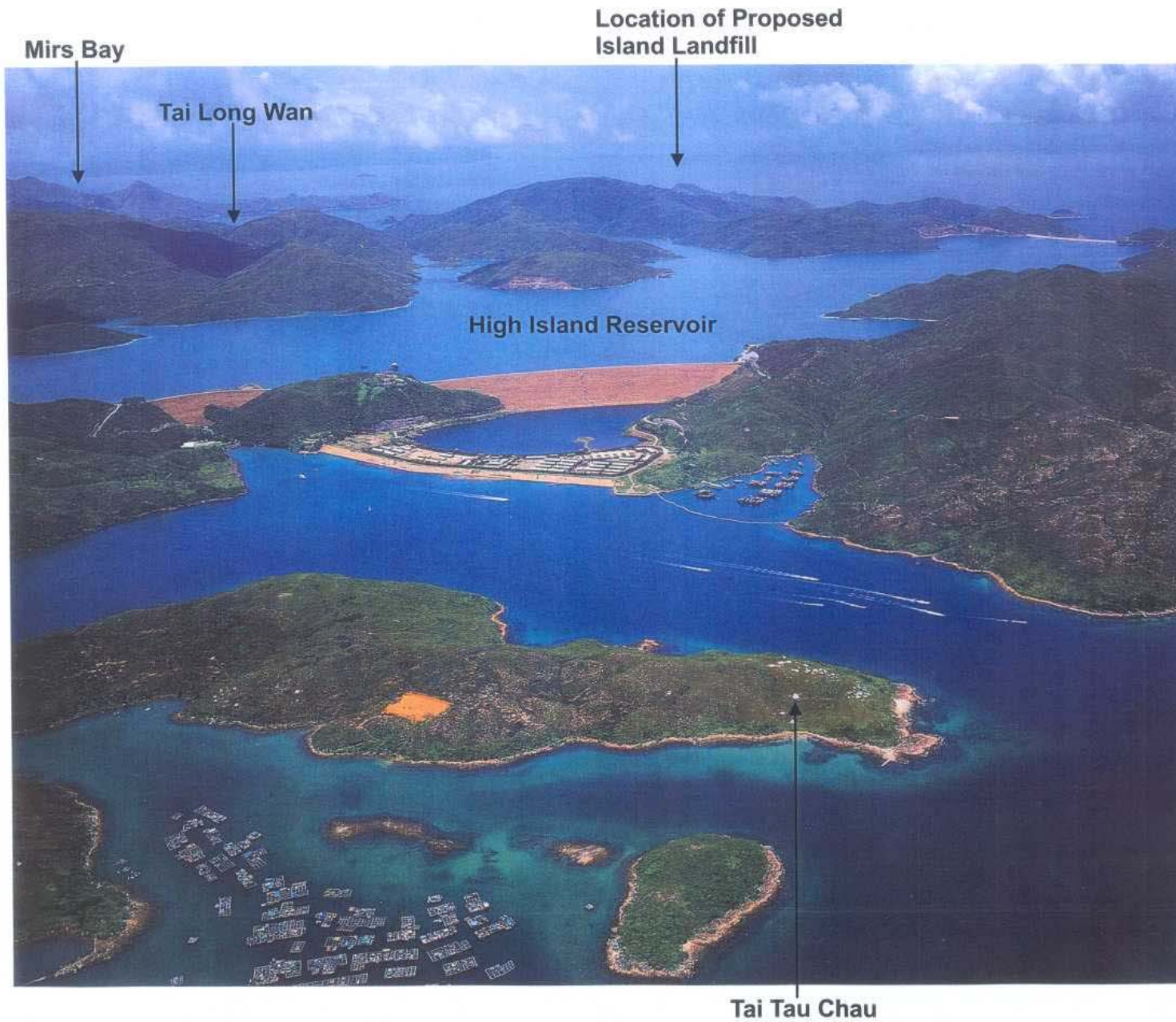
Figure 14.3 Tai Long Wan Offshore Island Landfill - Landscape Context
