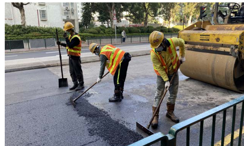
| Paving PMSMA6 surface at Wu Chui Road, Tuen Mun
