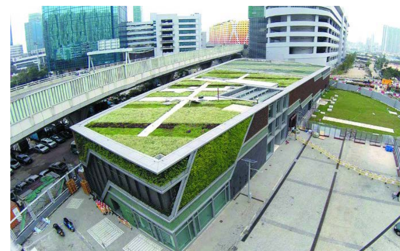
Energy Saving and Green Buildings – District Cooling System at Kai Tak Development
