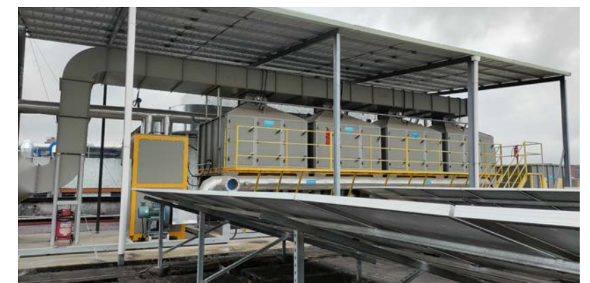
A combination of activated carbon concentrator and catalytic oxidation technology to remove VOCs in exhaust gas from printing process
