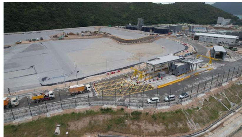
| SENT Landfill extension (first operation day on 21 November 2021)
