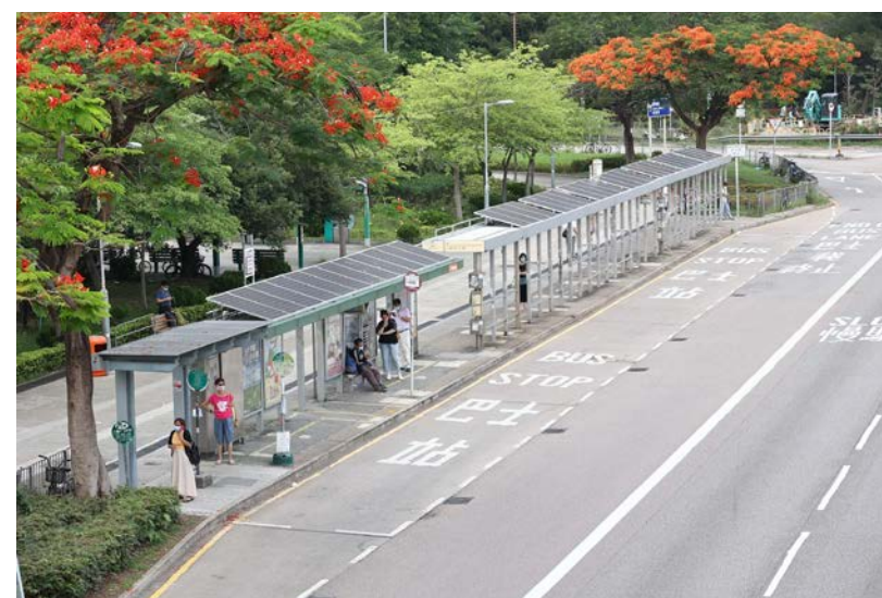
| The FiT Scheme has encouraged the private sector to develop RE. The Kowloon Motor Bus Company (1933) Limited and Long Win Bus Company Limited have installed solar panels on bus shelters to supply electricity for lighting at bus stops.
