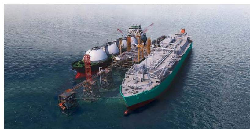
Offshore Liquefied Natural Gas (LNG) Terminal under construction (Artist's Impression)
