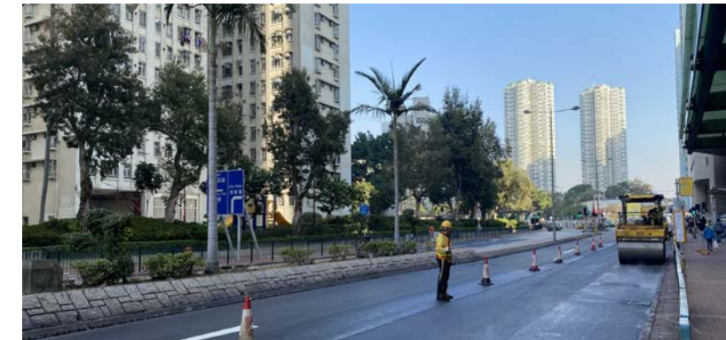
| Road surfacing works at Wu Chui Road, Tuen Mun
