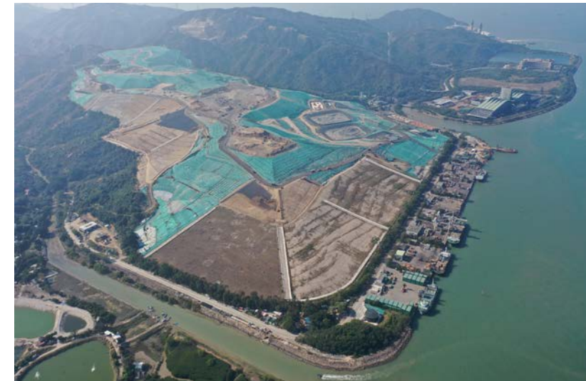
| WENT Landfill and its Extension
