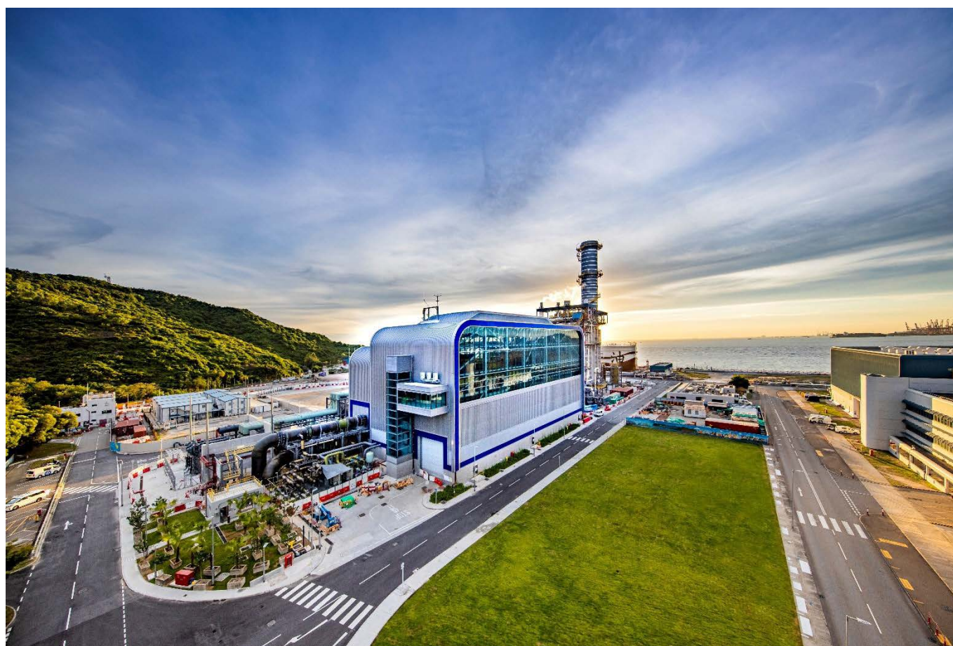
| New gas-fired generation unit at Black Point Power Station
