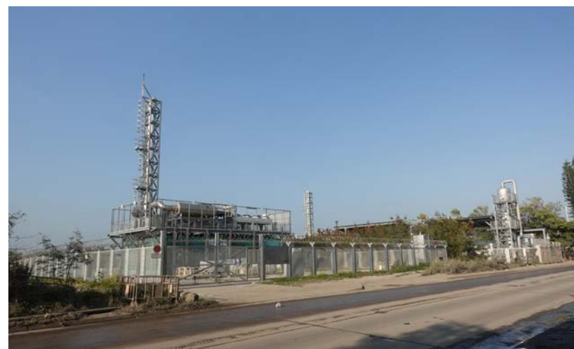
| WENT Landfill Gas Utilisation Facility
