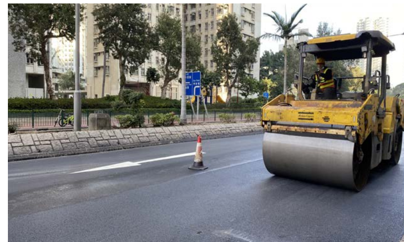
| Compressing the just-laid PMSMA6 surface at Wu Chui Road, Tuen Mun
