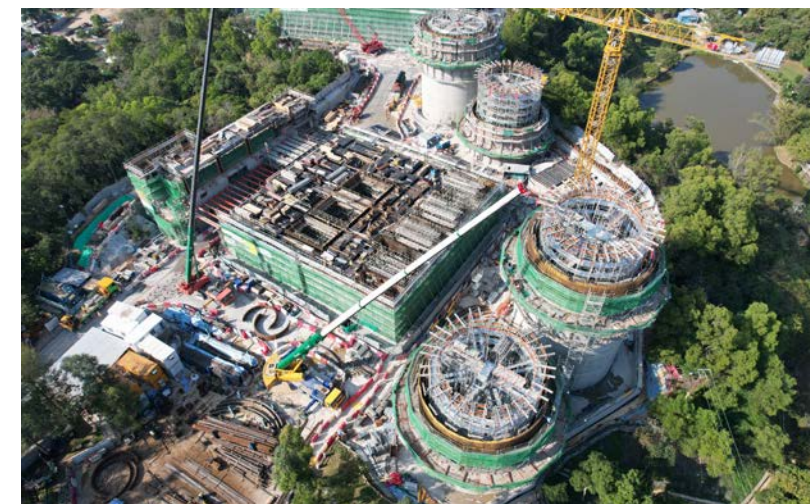
Construction in progress at O-PARK2 (December 2021)
