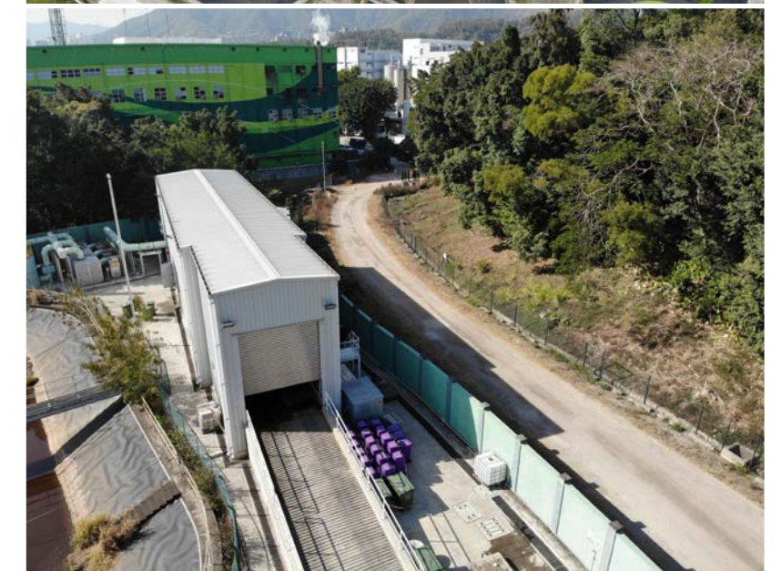
Food Waste Pre-treatment Facilities for food waste / sewage sludge anaerobic co-digestion trial scheme at Tai Po Sewage Treatment Works
