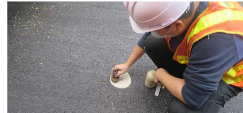
| Measuring the engineering performance of PMSMA6 right after the re-surfacing works
