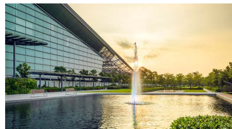
T-PARK combines advanced technologies including sludge incineration, power generation, seawater desalination, wastewater treatment, together with community amenities and an education centre
