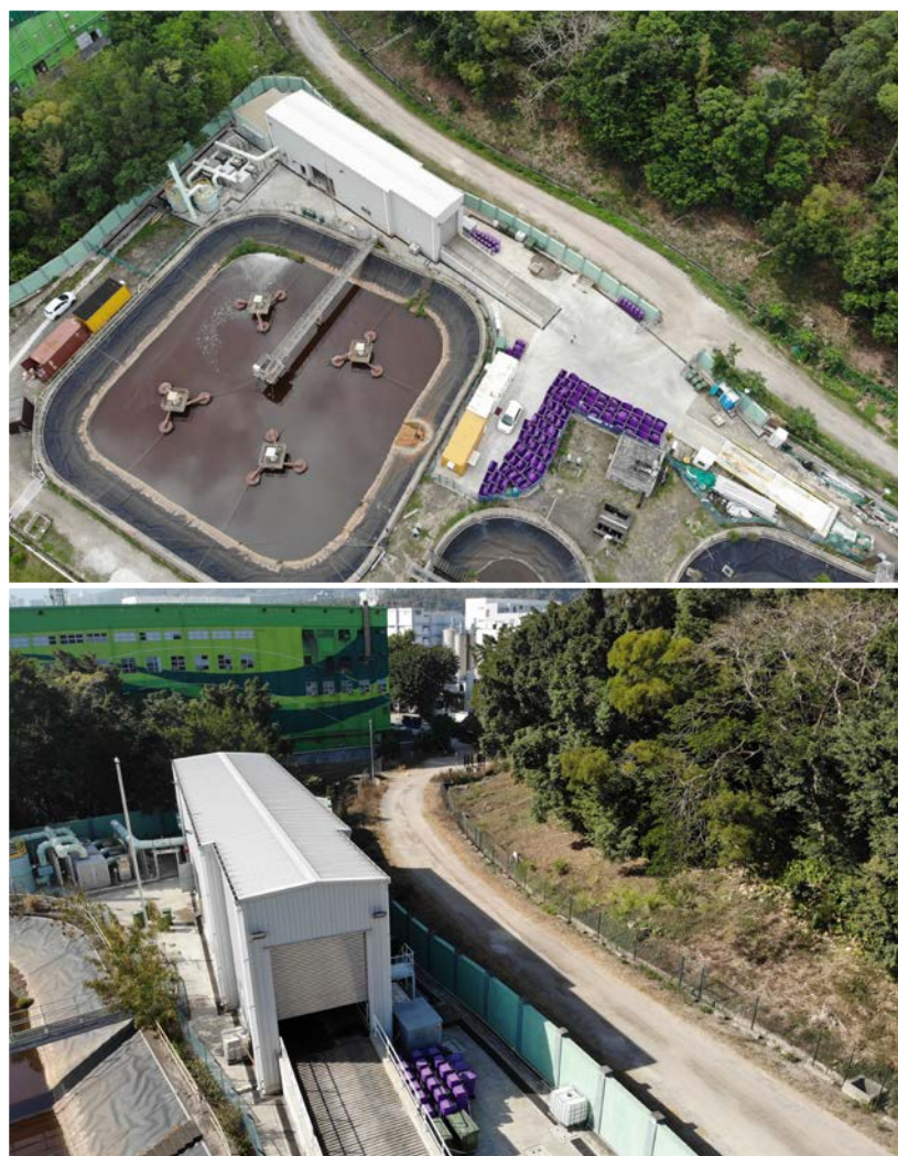
The Food Waste Pre-treatment Facilities for the food waste/ sewage sludge anaerobic co-digestion trial scheme at TPSTW
