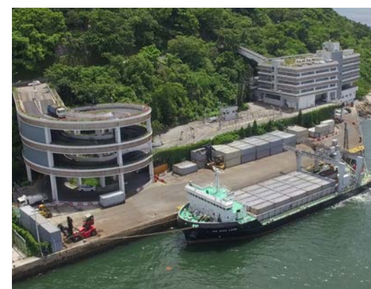
Island West Transfer Station
