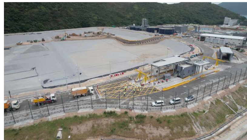
SENT Landfill extension (1 st operation day on 21 November 2021)
