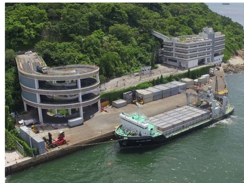
Island West Transfer Station
