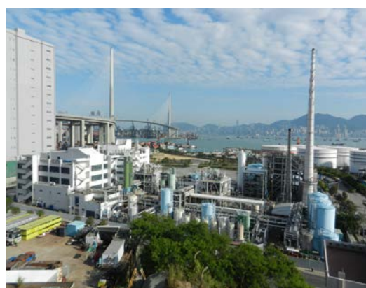
Chemical Waste Treatment Centre
