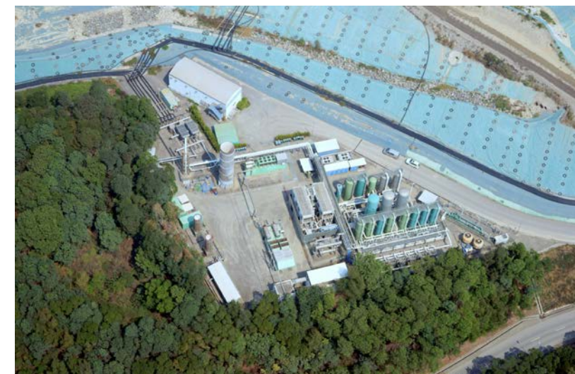
| Landfill Gas Treatment Facility at the NENT Landfill
