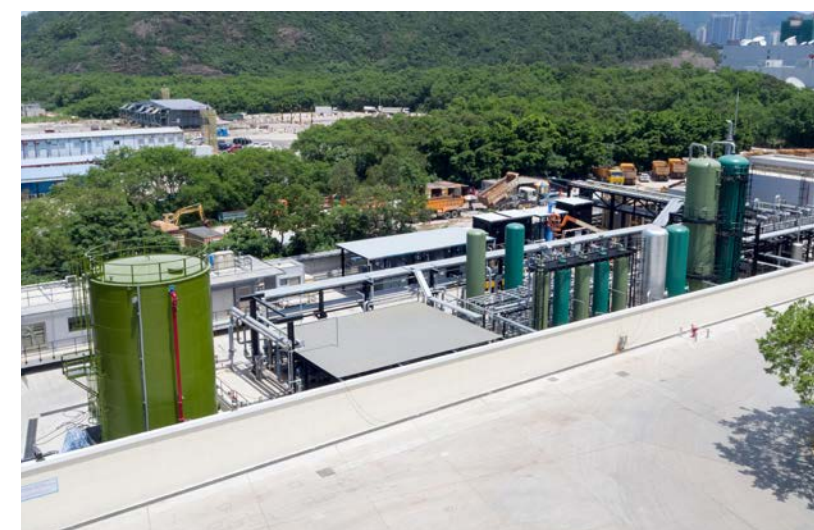
| Landfill Gas Utilization Plant at the SENT Landfill
