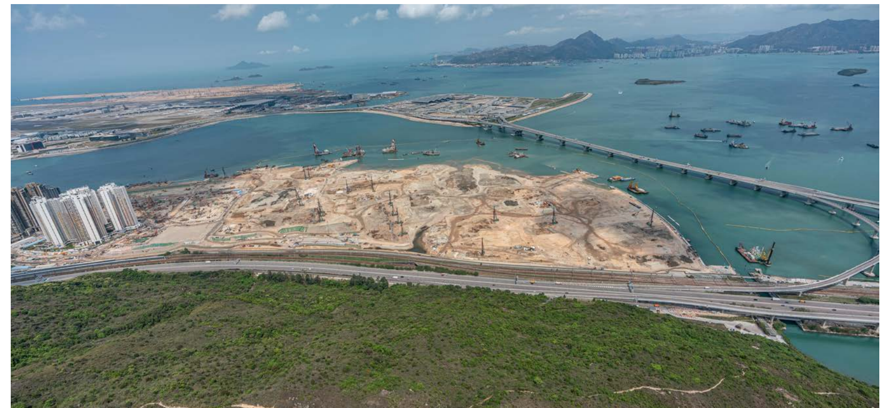
| Tung Chung East Reclamation Works
