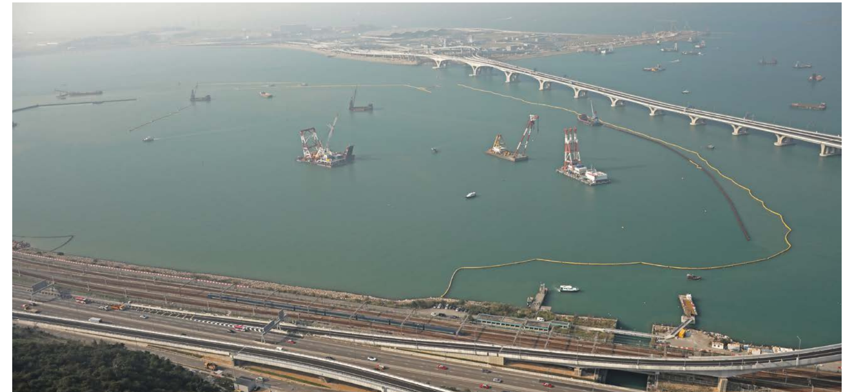
Perimeter silt curtain to enclose the reclamation works areas
