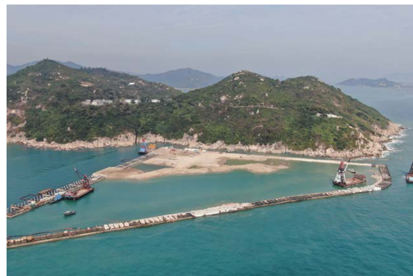
Reclamation of artificial island in progress at I-PARK (December 2020)
