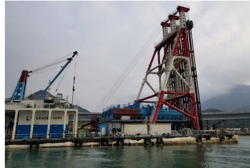
Deep cement mixing barges
