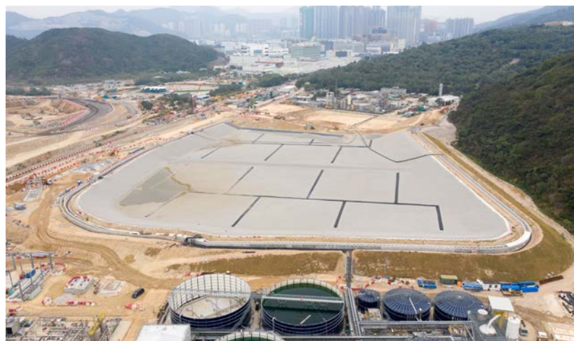
| Construction of the SENT Landfill extension in progress
