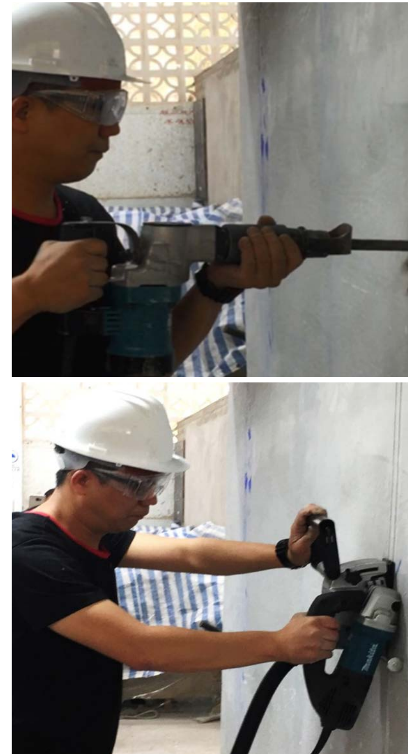
Wall chaser (bottom) performs with less noise and dust than the conventional breaker (top)
