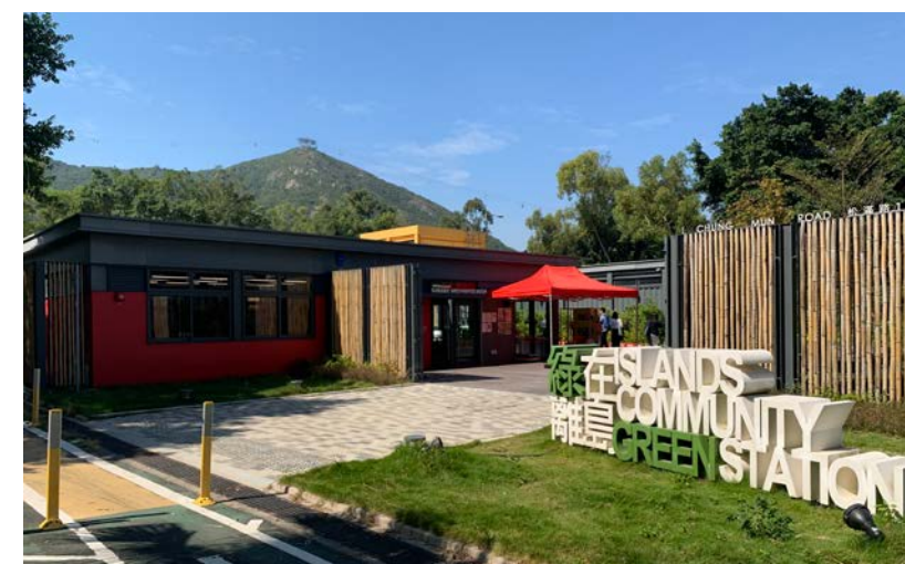
A new Recycling Station GREEN@ISLANDS has commenced service to the public since 2020
