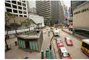
Roadside Air Monitoring Station at Central
