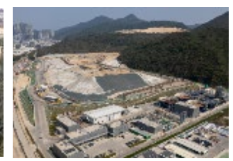
SENT Landfill Extension
