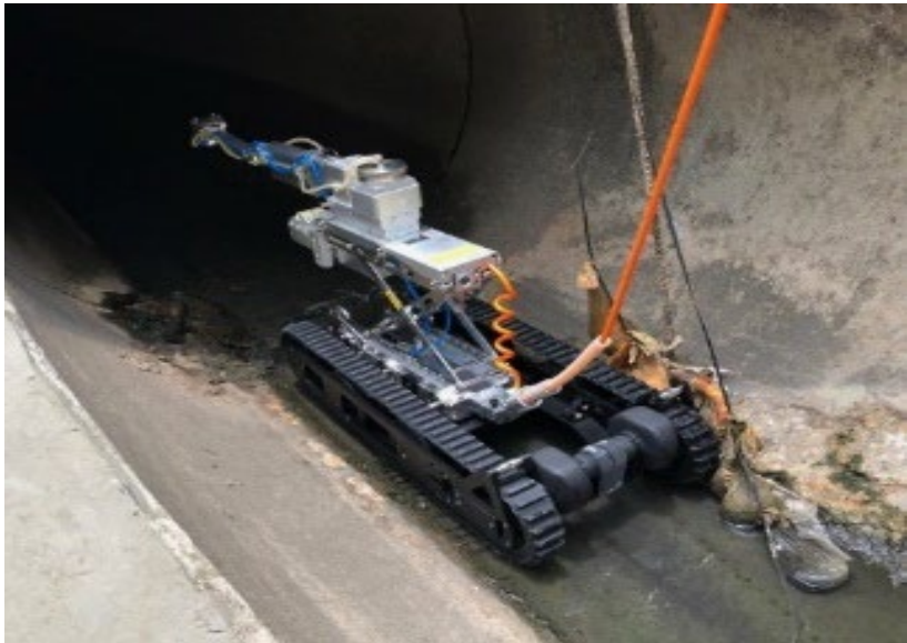
Multi-terrain robot in tracing the pollution at underground drainage systems
