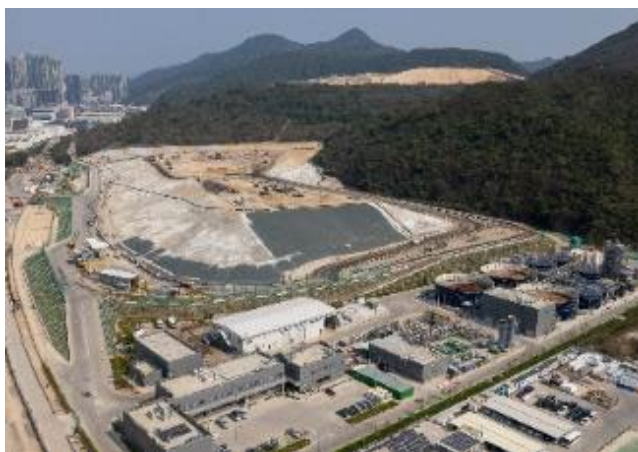
SENT Landfill extension
