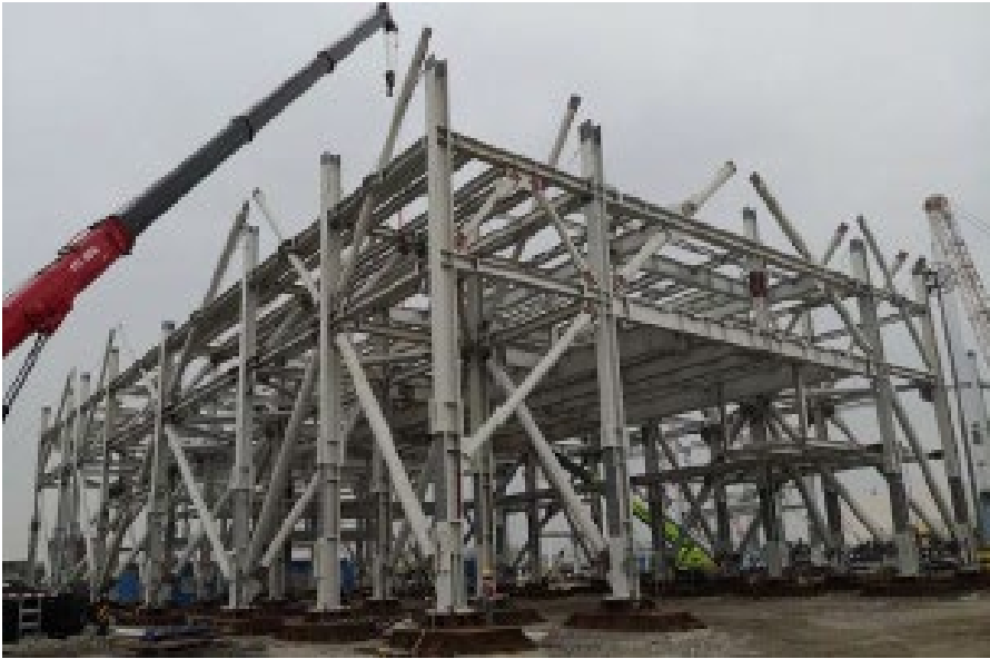
Off-site prefabrication of huge electrical and mechanical units at Zhuhai (2022)
