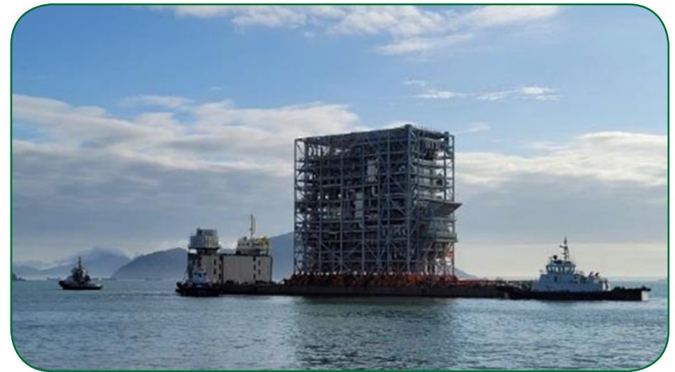
I-PARK1's main electrical and mechanical equipment modules setting sail to Hong Kong from Zhuhai (2023-2024)
