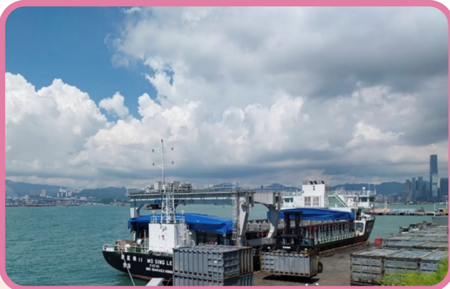
A new diesel-electric-powered waste container vessel equipped with lightweight screen cover berthing at Island West Transfer Station
