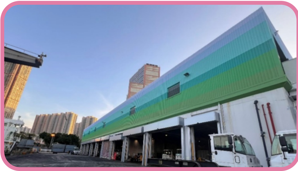
The facade of Transfer Building at Island East Transfer Station repainted with a gradient of greens and blues to blend harmoniously with the surroundings
