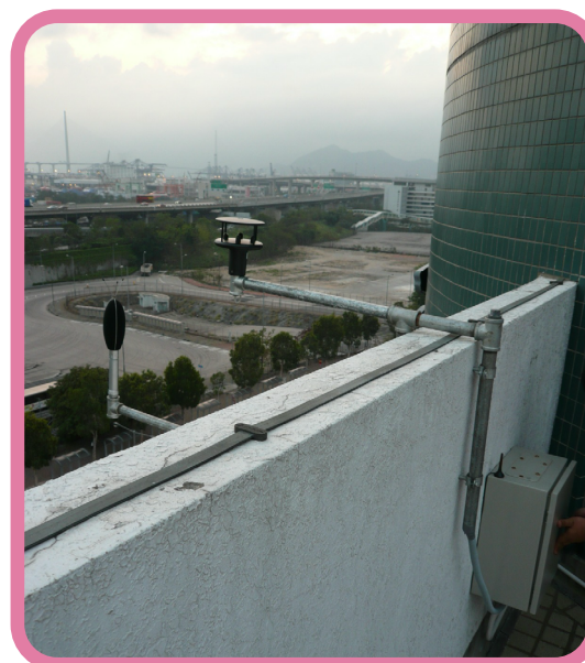
Putting concept into practice – continuous construction noise monitoring at the Hong Kong Section of XRL. (Photo courtesy of MTR Corporation Limited)
