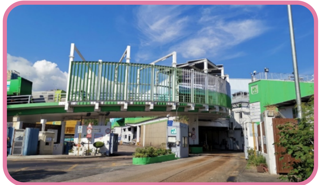
A stylish ramp canopy at West Kowloon Transfer Station
