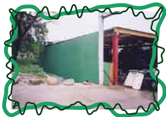
改善後 After Improvement
