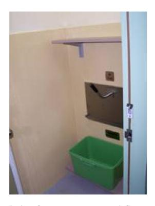
In the refuse storage room on each floor, a shelf was installed on the wall for stacking waste paper, and a plastic container was placed below the refuse chute inlet for collecting metals/plastics.
