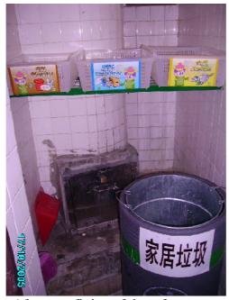
After retrofitting of the refuse storage room on each floor, a rack was installed above the refuse chute inlet for placing three plastic containers for collecting waste paper, metals and plastics.
