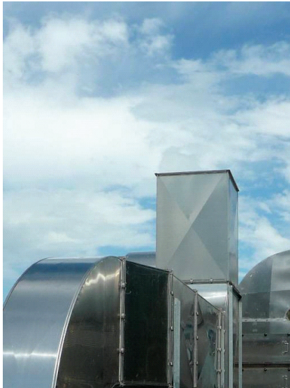
Fig.5: Exhaust outlet should be properly located away from air sensitive receivers.
