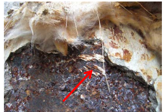
Asbestos cloth remnants on flue that has been re-insulated with non-asbestos cement render and glass fibre insulation
