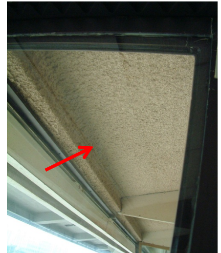
Coarse textured sprayed ceiling coating
