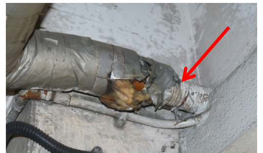
Asbestos rope pipe insulation beneath glass fibre insulation
