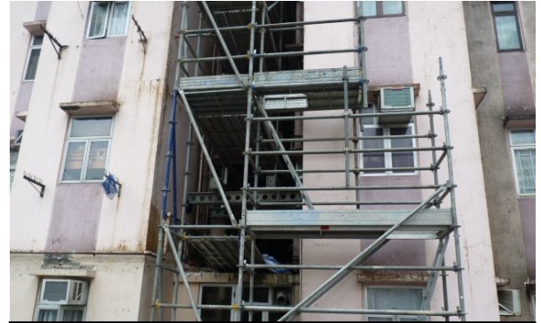
Metal scaffold should be used. Ensure a separate external staircase for access for work inspection
