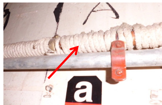
Asbestos rope pipe insulation
