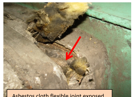
Asbestos cloth flexible joint exposed by removal of glass fibre
