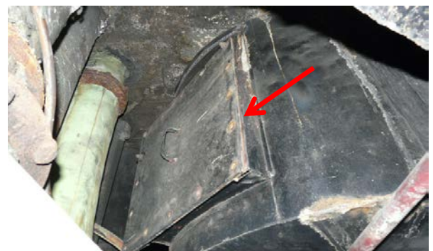
Access plates to flues and chimneys can also contain asbestos gasket seals. These can complicate thorough inspection and should not be disturbed until removal
