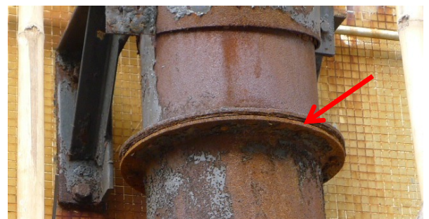
Uninsulated flues – and flues after insulation removal should be dismantled at flange joints to inspect for and remove any asbestos gaskets
