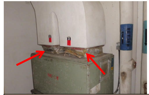
Asbestos cloth flexible joints to free standing air handling unit.
