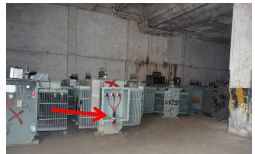
Electrical distribution transformers in storage. All units should be uniquely marked to enable tracing during abatement and disposal
