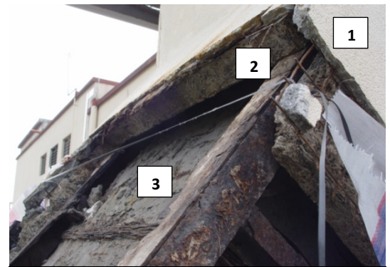
Chimney consisting of external non-asbestos cement render (1) on top of compressed timber board (2) with asbestos plaster to rectangular flue inside (3)
