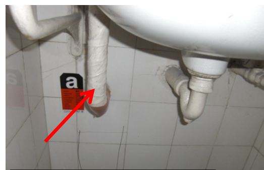
Asbestos plaster pipe insulation
