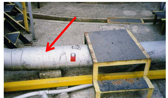
Bituminous asbestos and hessian wrap to external pipes
