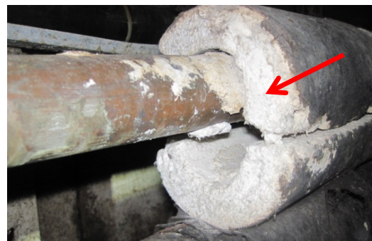
Sectional asbestos plaster pipe insulation
