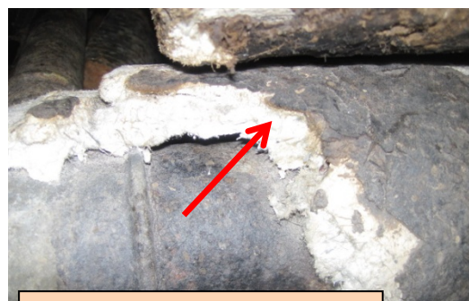
Asbestos plaster pipe insulation
