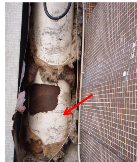
Asbestos plaster flue insulation covered by glass fibre insulation
