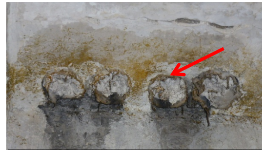
Cut off remnants of pipes through floor slab with asbestos plaster pipe insulation
