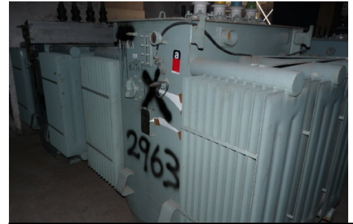
Electrical distribution transformer asbestos hazard labelled prior to disposal
