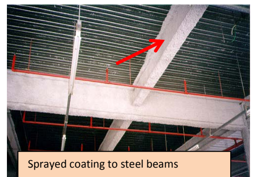
Fine textured sprayed ceiling coating
