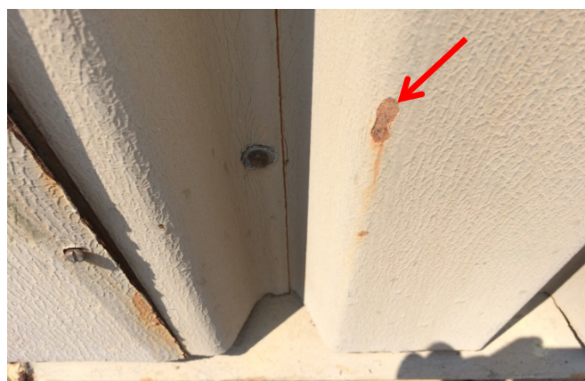
“Galbestos” asbestos coating to profiled metal wall sheeting is only discernable with close-up inspection as a slightly thickened textured outer layer to the metal sheet
