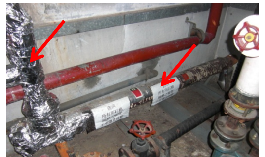
Asbestos cloth pipe insulation beneath glass fibre insulation partially wrapped in metal foil
