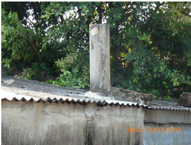
CACS roof is associated with other ACMs (An asbestos cement flue as shown in the example above).
