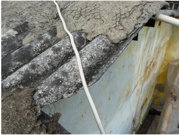
CACS roof covered with a layer of cement screeding.
