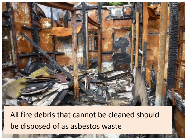
Small scale debris scattered around a fire site will need clearing prior to work zone erection
