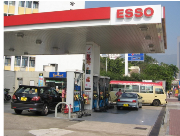
Petrol filling station
