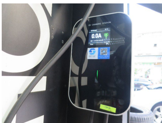
7.2 kW AC charging facility
